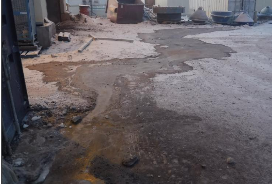
Photo 1. Overflow spill on ground surrounding WWTP.
