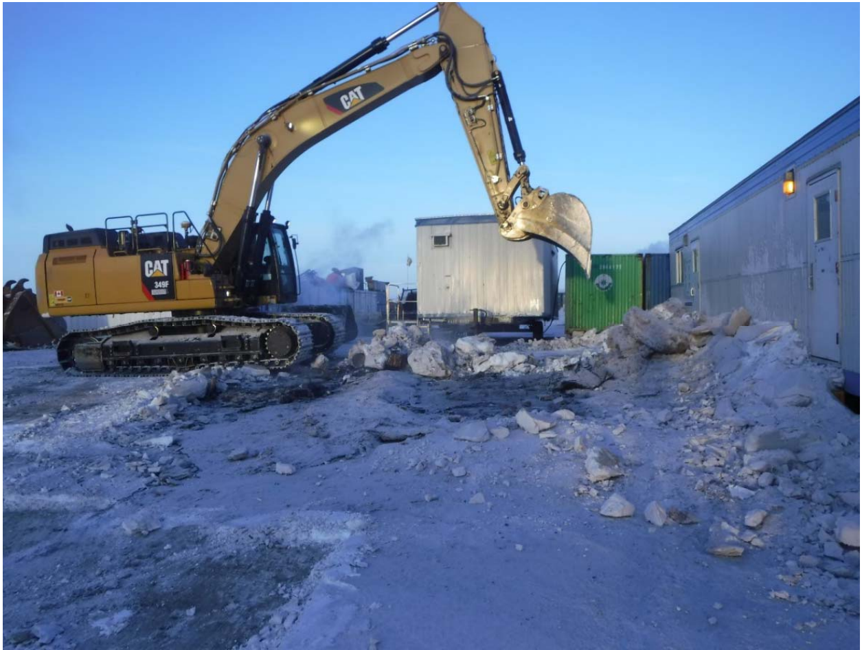
Photo 2 – Impacted ice/snow being scrapped up by excavator
