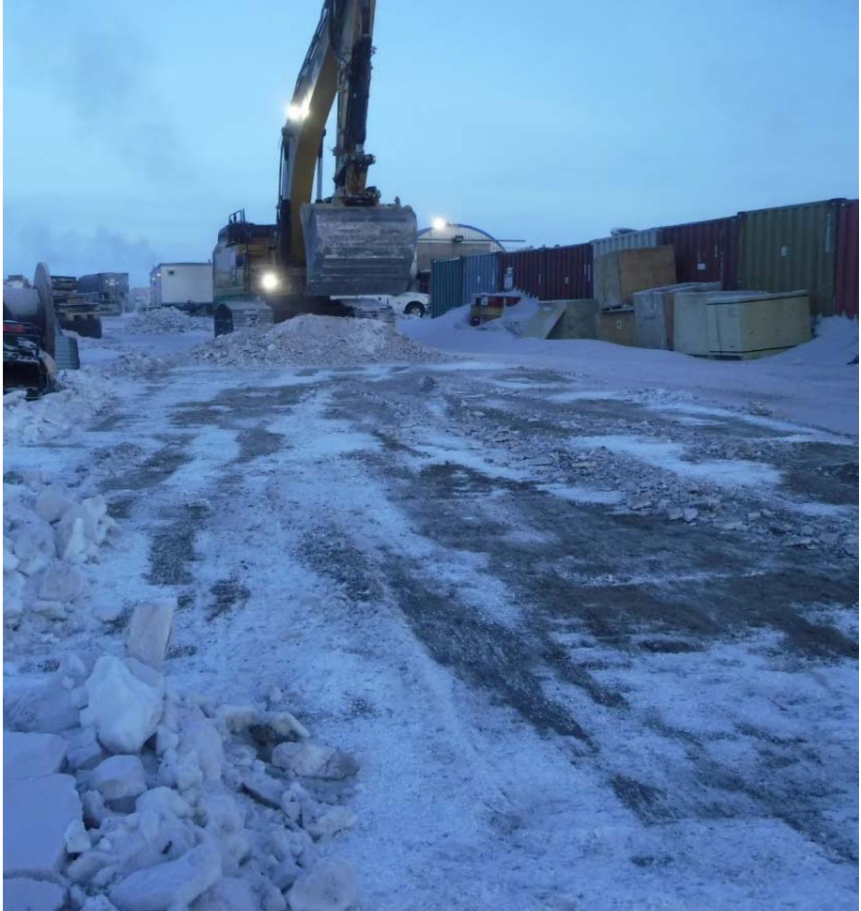
Photo 3 – Impacted ice/snow being scrapped up by excavator
