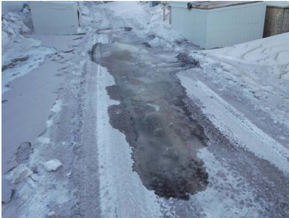
Photo 1. Overflow spill on ground outside MSC AA South lift station
