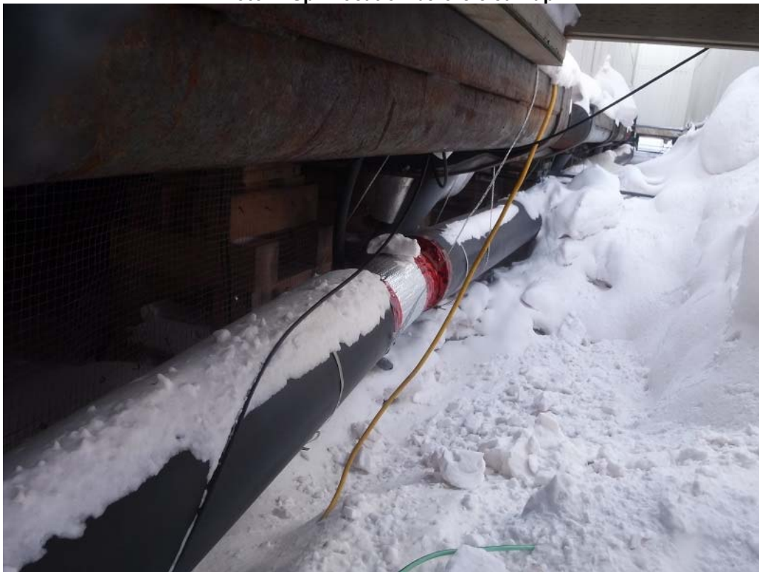
Photo 2. Gravity Drain Line after repairs completed
