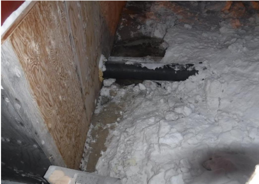
Photo 1. Overflow spill on ground outside Weatherhaven lift station
