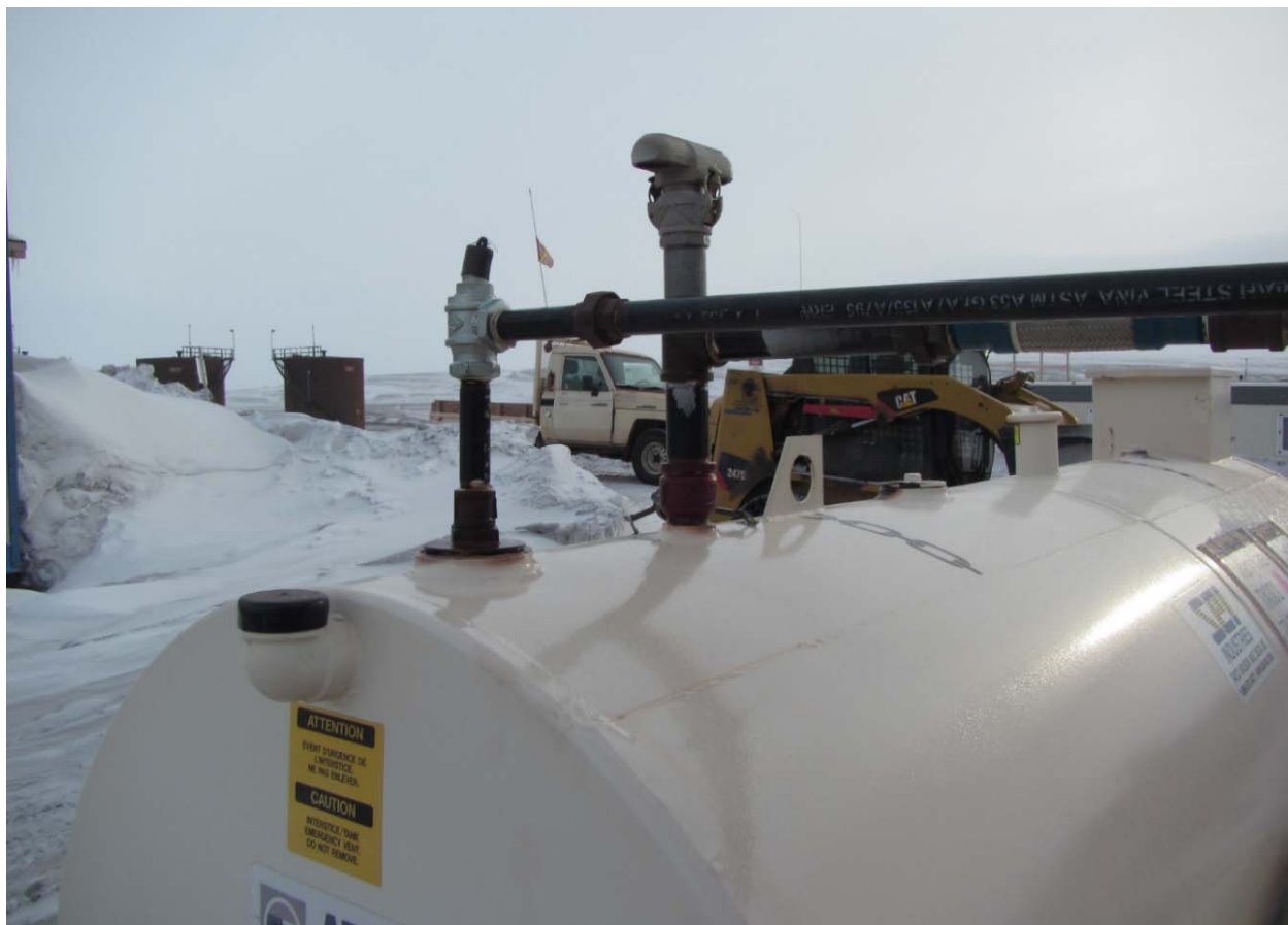
Photo 3. Vent pipe and whistle before retrofit
