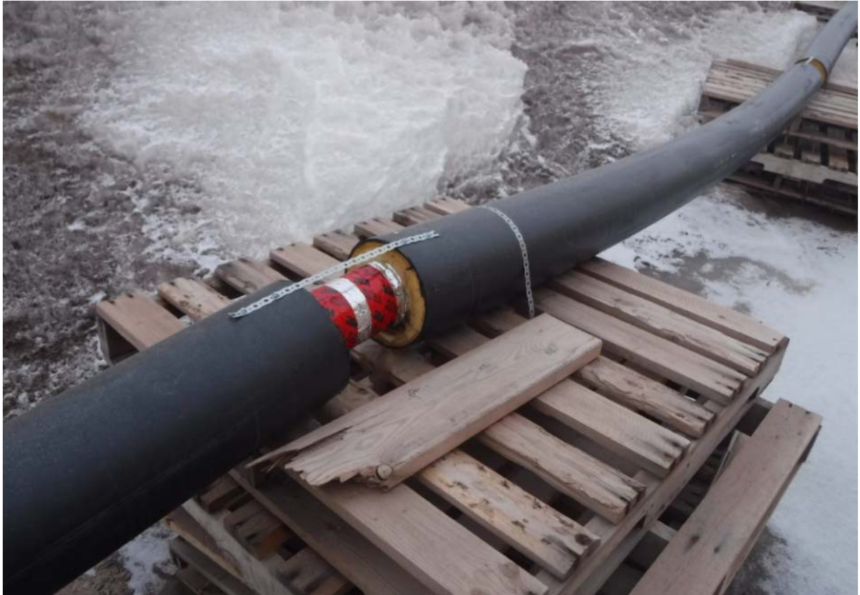
Photo 2. Lift station discharge line after repairs were completed.
