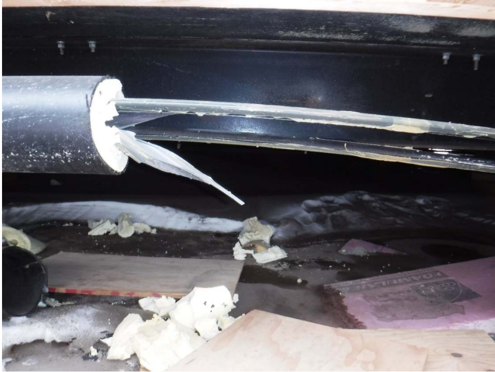
Photo 1. Discharge line in need of repair for approx. 20 feet
