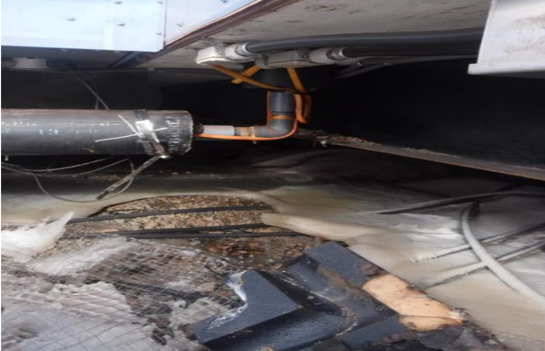
Photo 1. Discharge line before elbow repair
