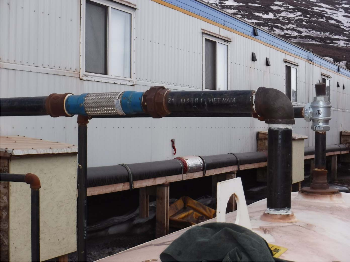
Photo 5. Return line without audible whistle fitting on main tank
