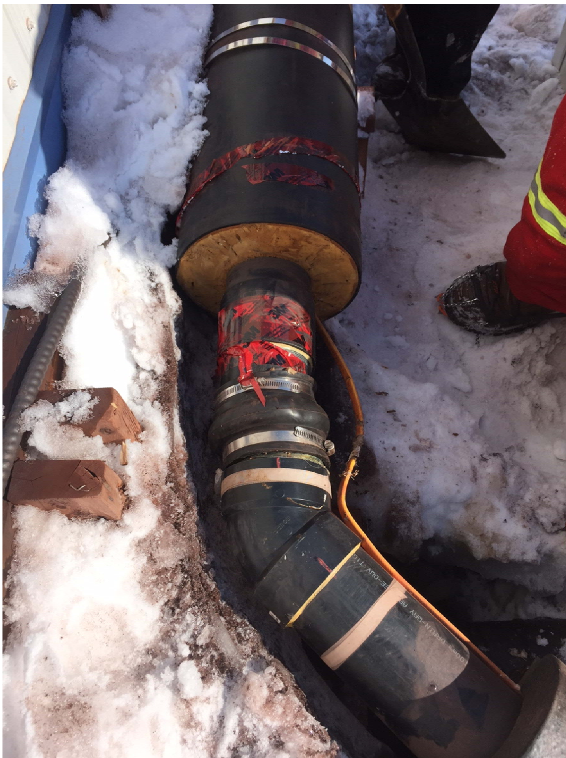
Photo 1: Gravity drain line following repair of the separated coupling.
