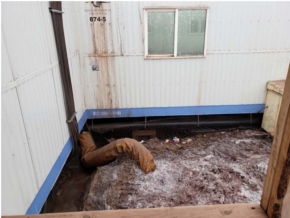
Photo 2. Discharge pipe problematic location
