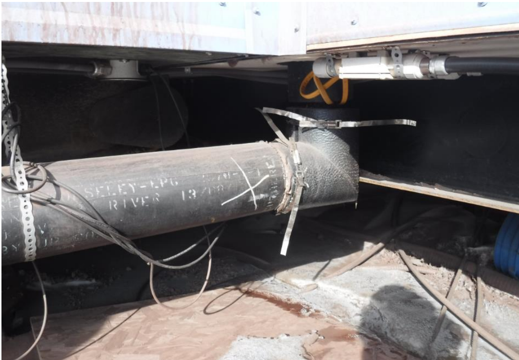
Photo 2. Discharge line following elbow repair
