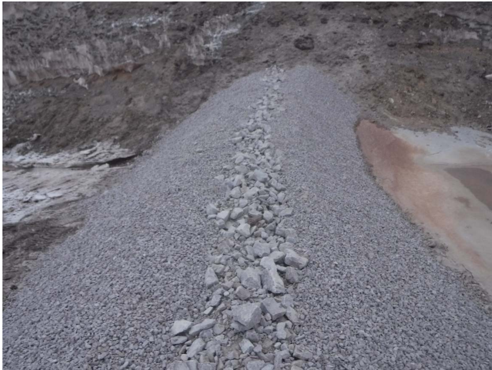
Photo 4. May 22, 2018: Typical check dam/berm cross section
