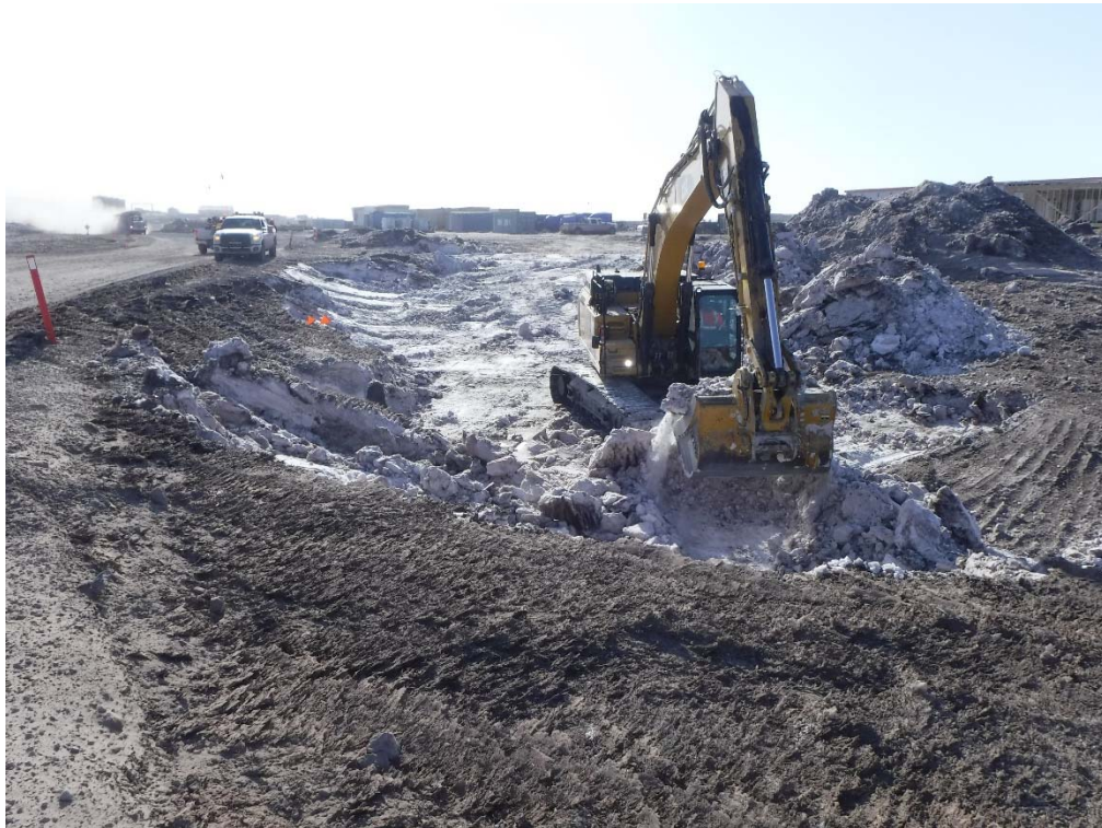
Photo 4. May 9, 2018: Removal of excess snowpack from road crossing above SDLT
