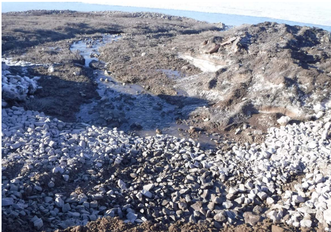
Photo 4. June 6, 2018: Bank armoring with riprap
