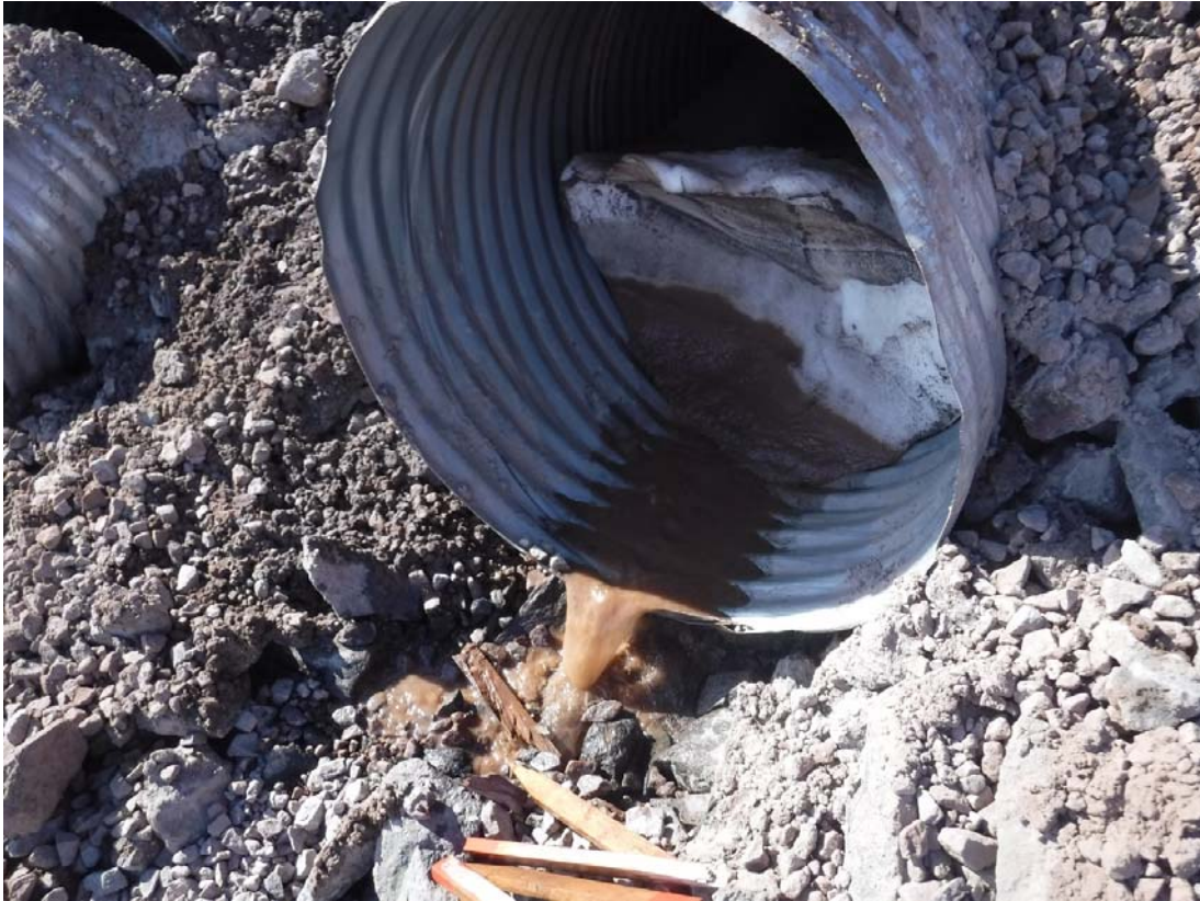
Photo 3. June 10, 2018: Minimal flow from culvert outlet after inlet was blocked off to divert runoff from the Mine Haul Road
