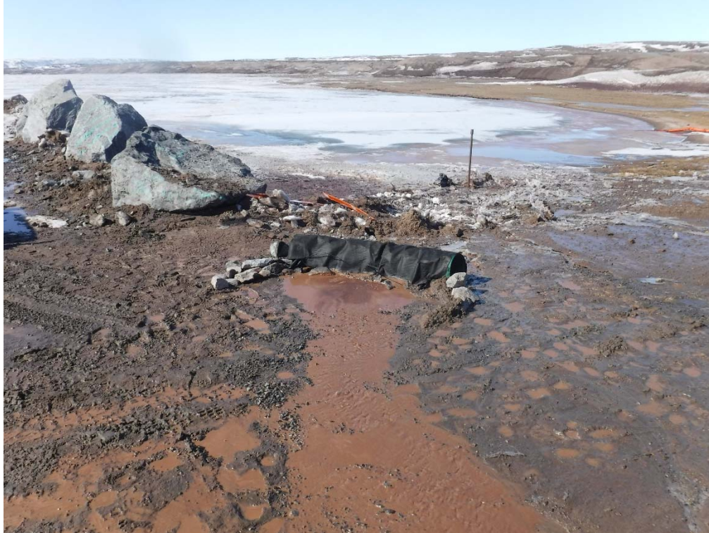
Photo 1. May 15, 2018: Sediment-laden water flowing into spring berm before entering Camp Lake
