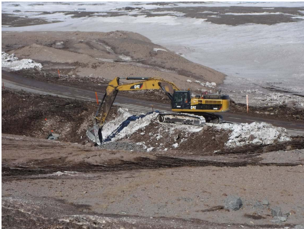
Photo 6. May 13, 2018: Removal of excess snowpack from road crossing above CLT
