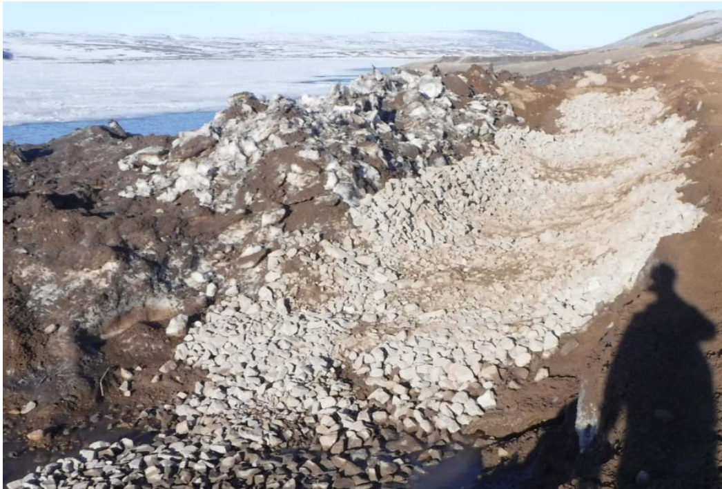
Photo 3. June 6, 2018: Bank armoring with riprap
