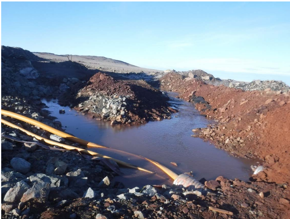
Photo 2. June 20 th , 2018 – West drainage ditch inflow into the Waste Rock Stockpile Pond following berm reinforcement.
