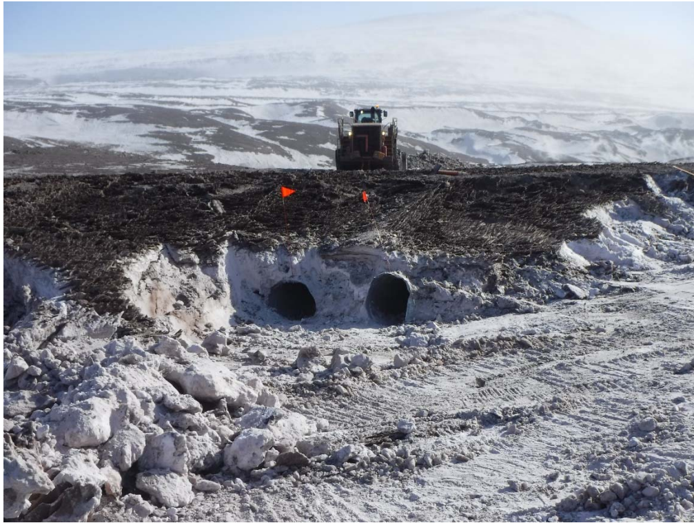
Photo 3. May 9, 2018: Removal of excess snowpack from road crossing above SDLT
