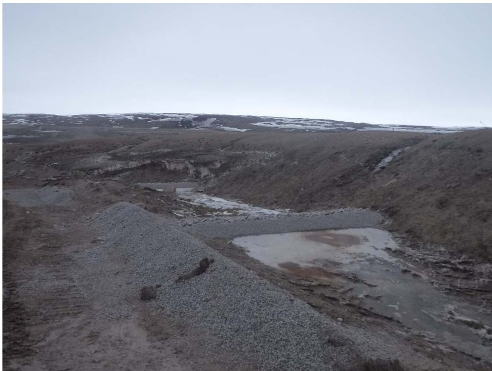
Photo 2. May 22, 2018: Camp Lake Jetty access road drainage channel check dam
