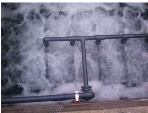
Proper air scouring in membrane tank
