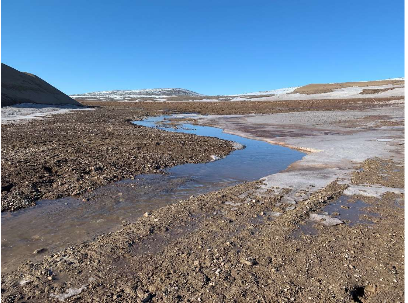
Figure E.14.2: Stream Crossing with Culvert Removed, Historic Roadway Regraded to Restore Natural Drainage, May 2019
