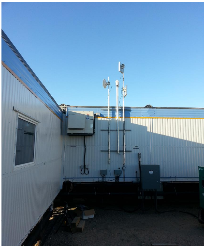
Figure 14: Mary River camp WS600-UMB sensor installed on outside wall of server room trailer (photo taken during 2014 trip)
