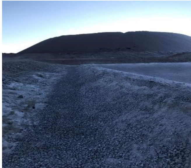
Type 5 in Base of Crest Trench Compacted
