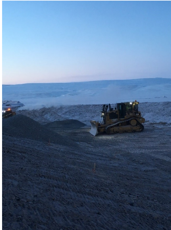
Placing Type 5 in Slope
