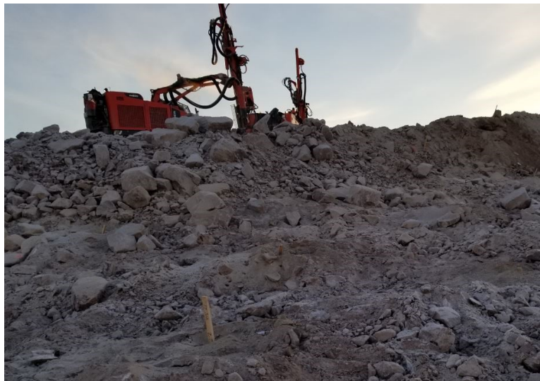
Blast Pattern Drilling Ongoing
