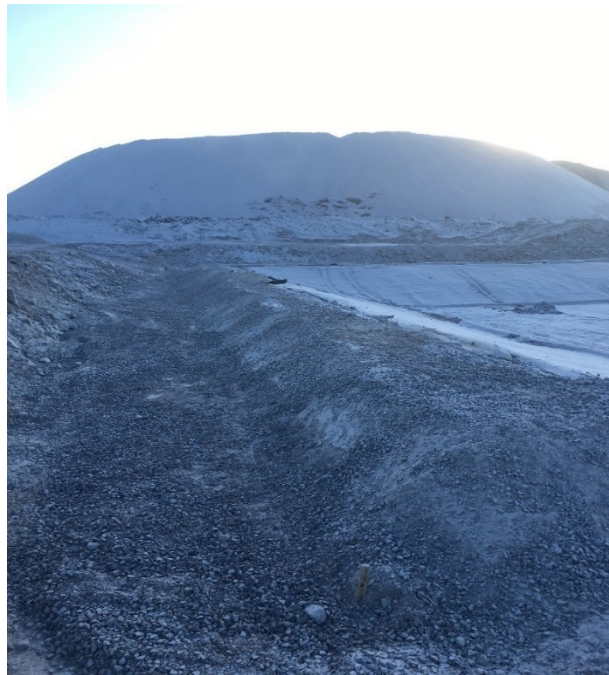
Pond 1A Backfill Key Trench with Type 5 and Trimming Backslope
