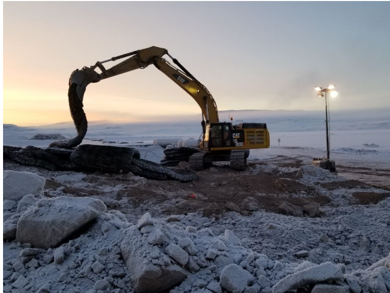
Blast Mat Positioning
