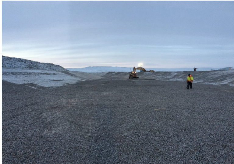
Placing Type 5 Material Pond Floor View from Floor Level
