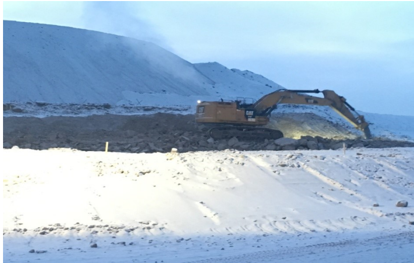
Ripping Frozen Material from Backslope Southeast
