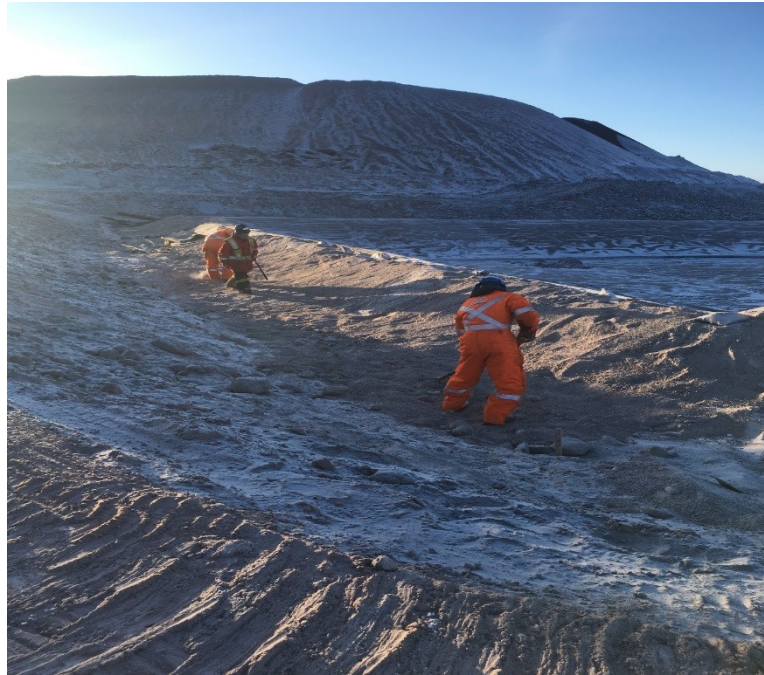
Placing Type 9 in Key Trench
