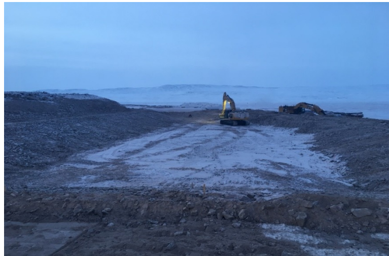
Trimming Slope and Pond Floor
