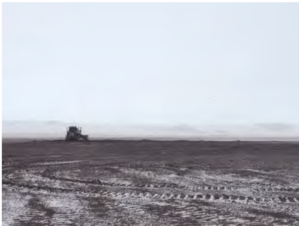
Figure 4-9: Placing Sacrificial Waste Iron Ore
