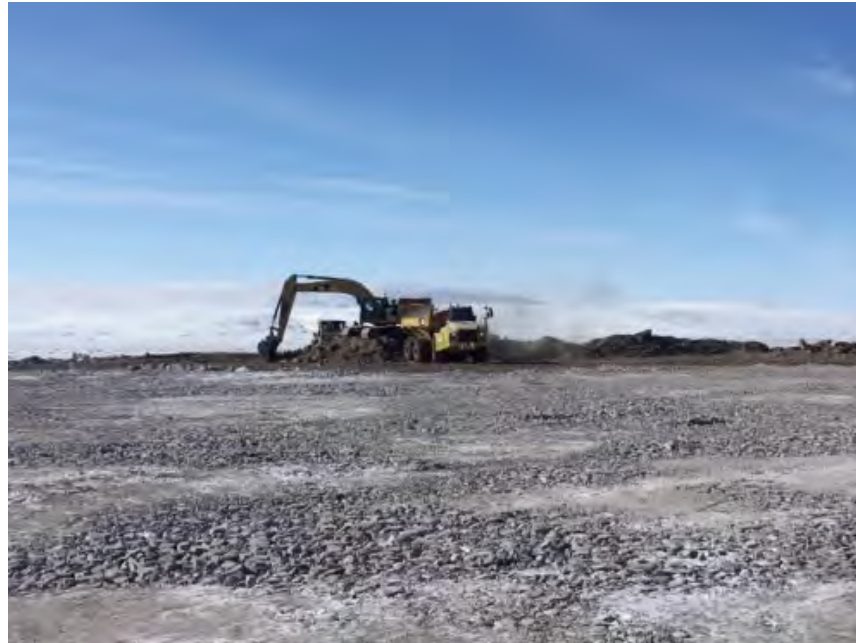
Figure 4-5: Removing Overburden
