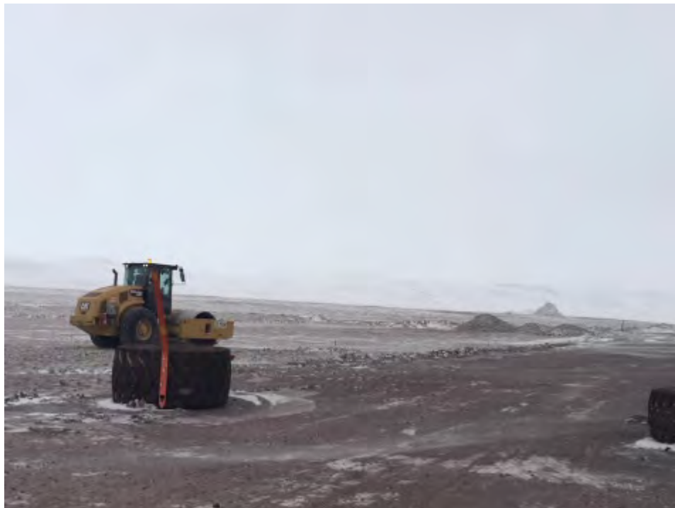
Figure 4-8: Compacting Type 8
