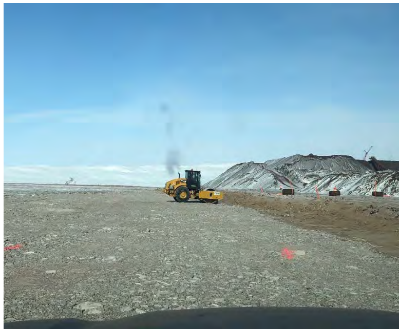
Figure 4-2: Compacting Rock Fill
