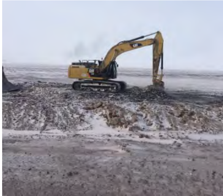
Figure 4-1: Ore Pad Excavation
