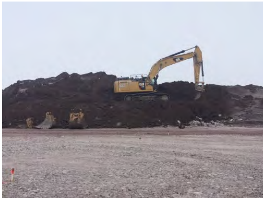
Figure 4-6: Ripping Frozen Waste Ore Stockpile
