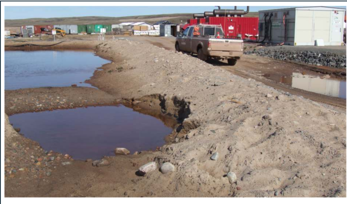
Figure 30: View of minor slope problem at the south-east corner of the berm at the Genset pond
