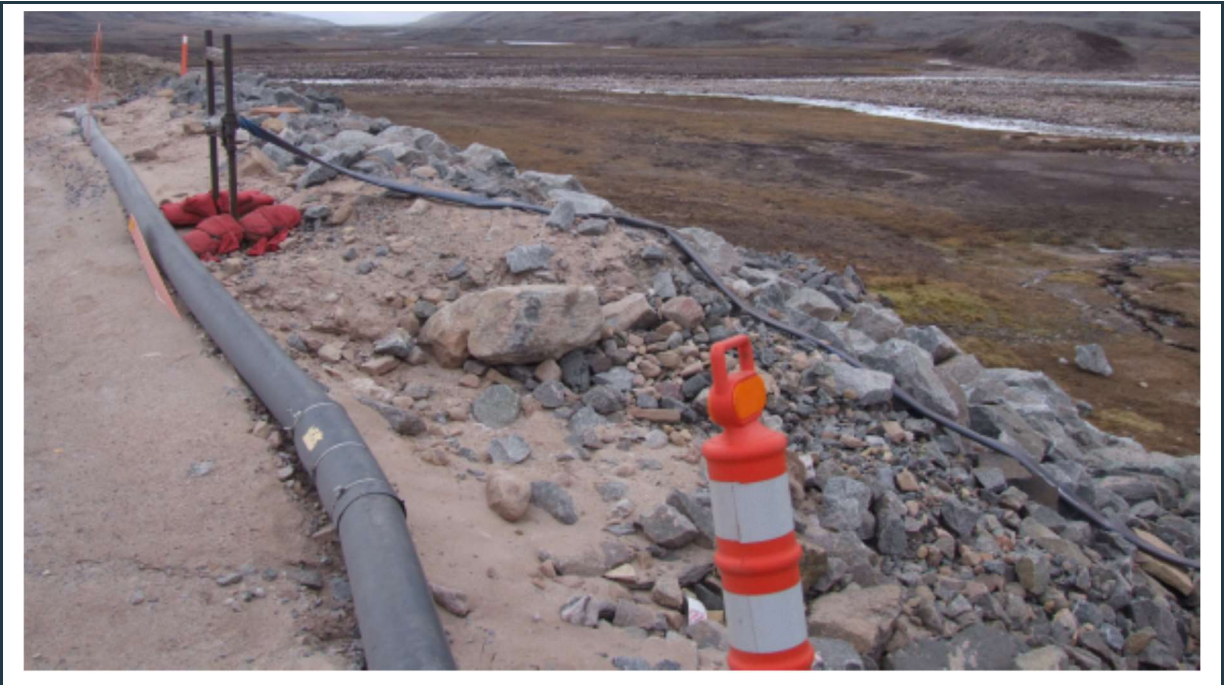
Figure 37: Water (effluent) discharge area. Stable slope, comprising a mix of crushed rock and soils.
