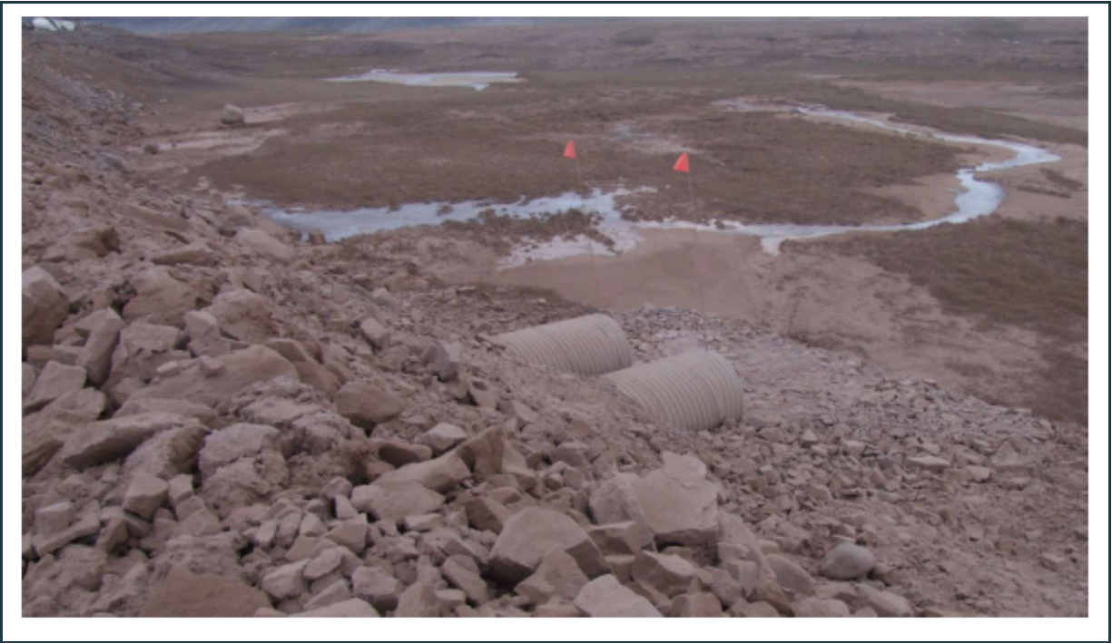
Figure 59: Water seepage through and beneath the road embankment near the tote road culverts.
