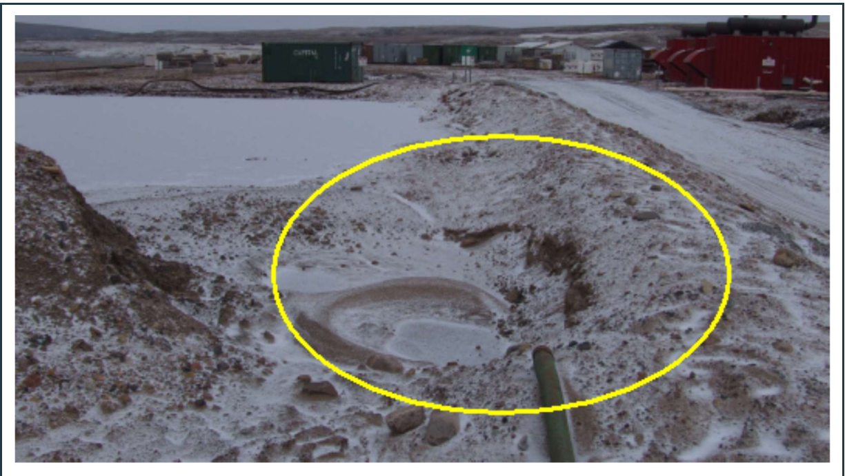
Figure 28: View of minor slope problem at the south-east corner of the generator berm.
