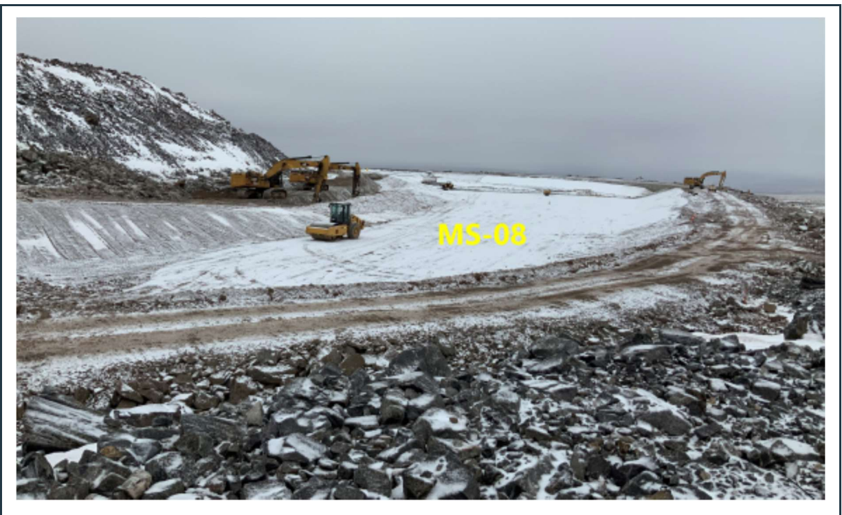
Figure 24: Construction of the new MS-08 pond, immediately adjacent to the waste rock dump.
