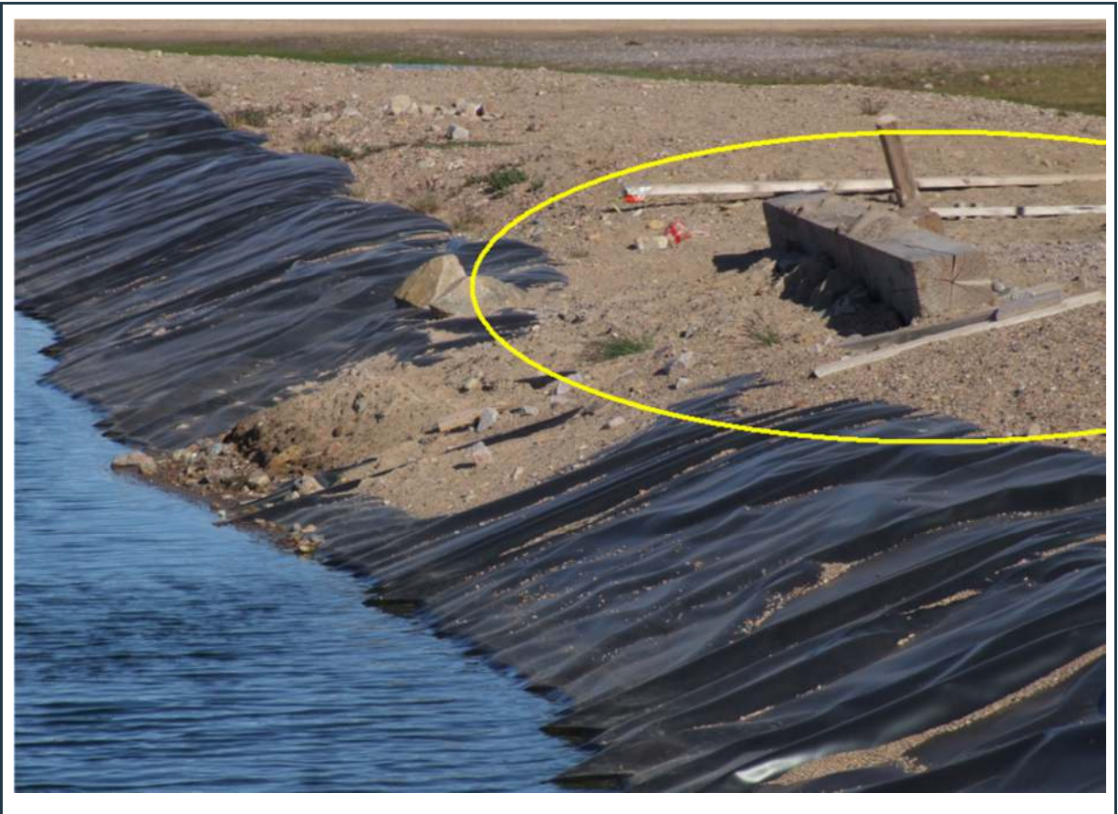
Figure 8: PWS pond #2 – Lower crest elevation caused by truck traffic at the water discharge point (yellow circle)
