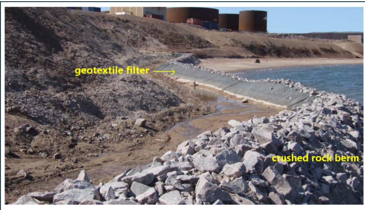
Figure 61: View of the freight dock check dam/berm with geotextile filter on the upstream face of the crushed rock berm, to retain silt
