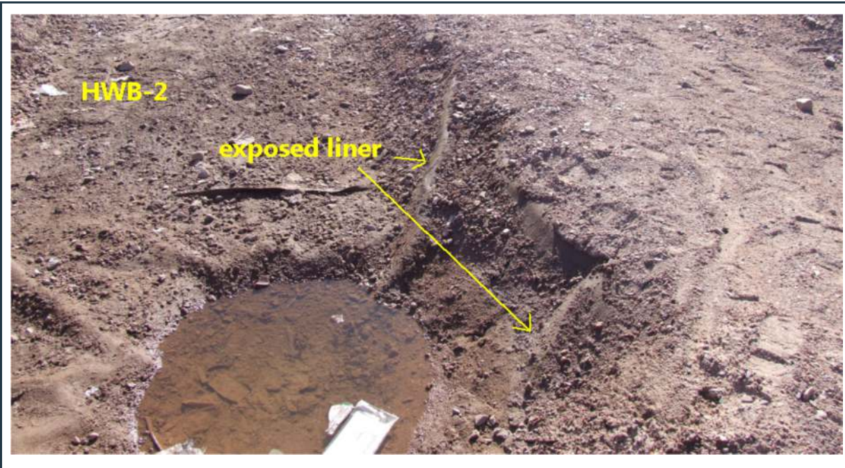
Figure 44: Small area of ponding water within the HWB-2 cell with locally exposed liner
