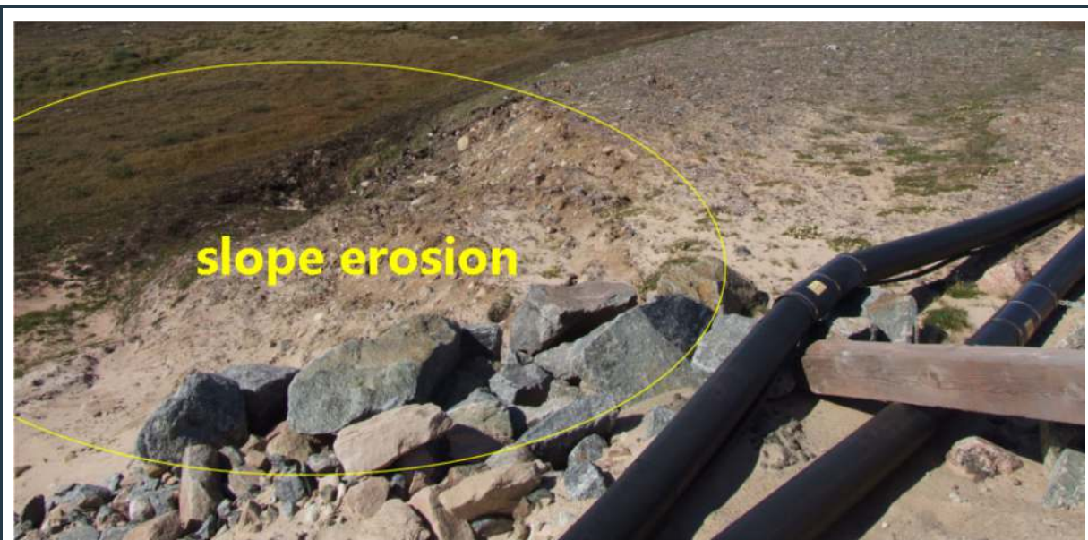
Figure 41: Minor slope erosion adjacent to the water discharge area.
