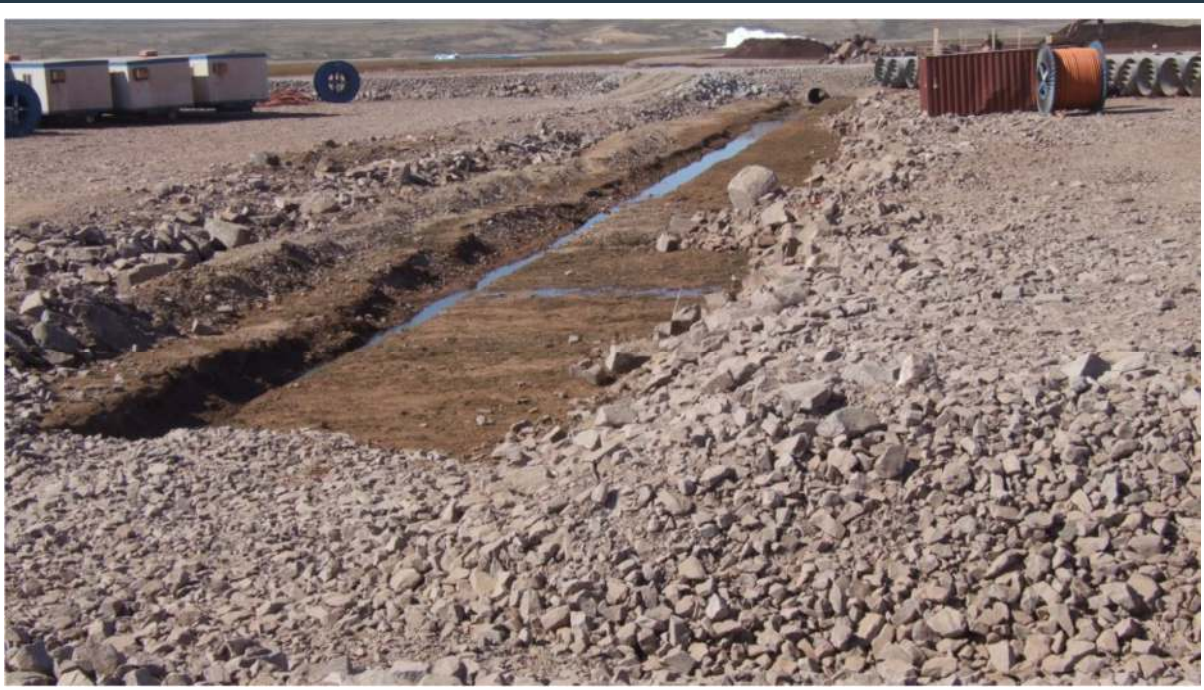
Figure 66: W13-W14 surface water collection ditch (under construction)
