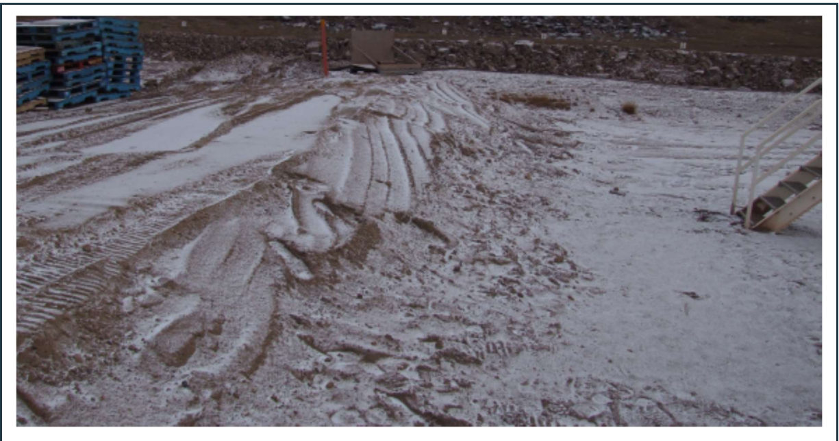
Figure 30: Recently placed granular fill on the berm's crest, to protect the previously exposed liner.
