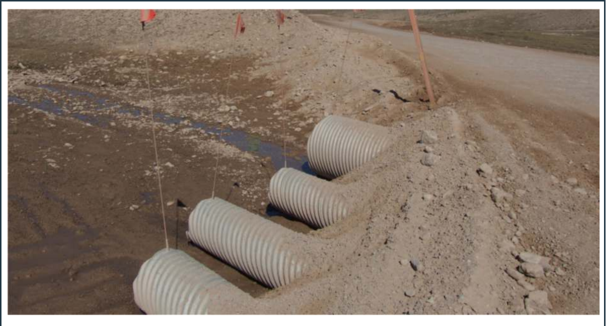
Figure 90: View of culvert(s) 102 (outlet) in excellent conditions
