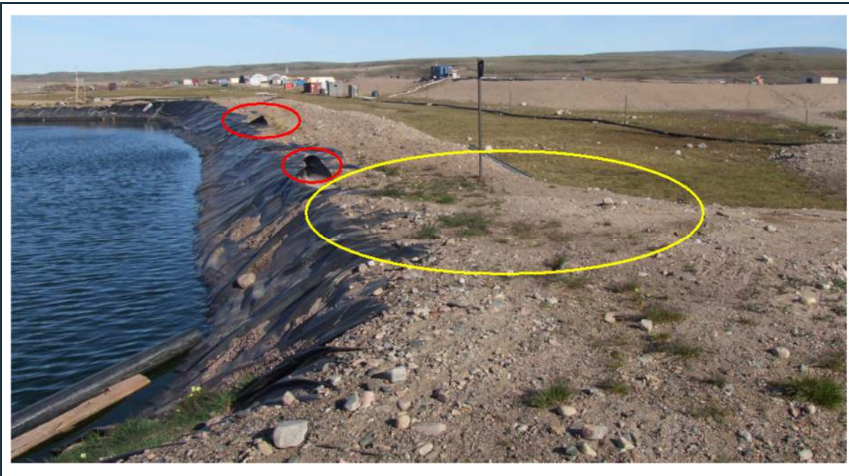
Figure 7: PWS pond #1 – Lower crest elevation (yellow circle) and damages to the liner (red circles)
