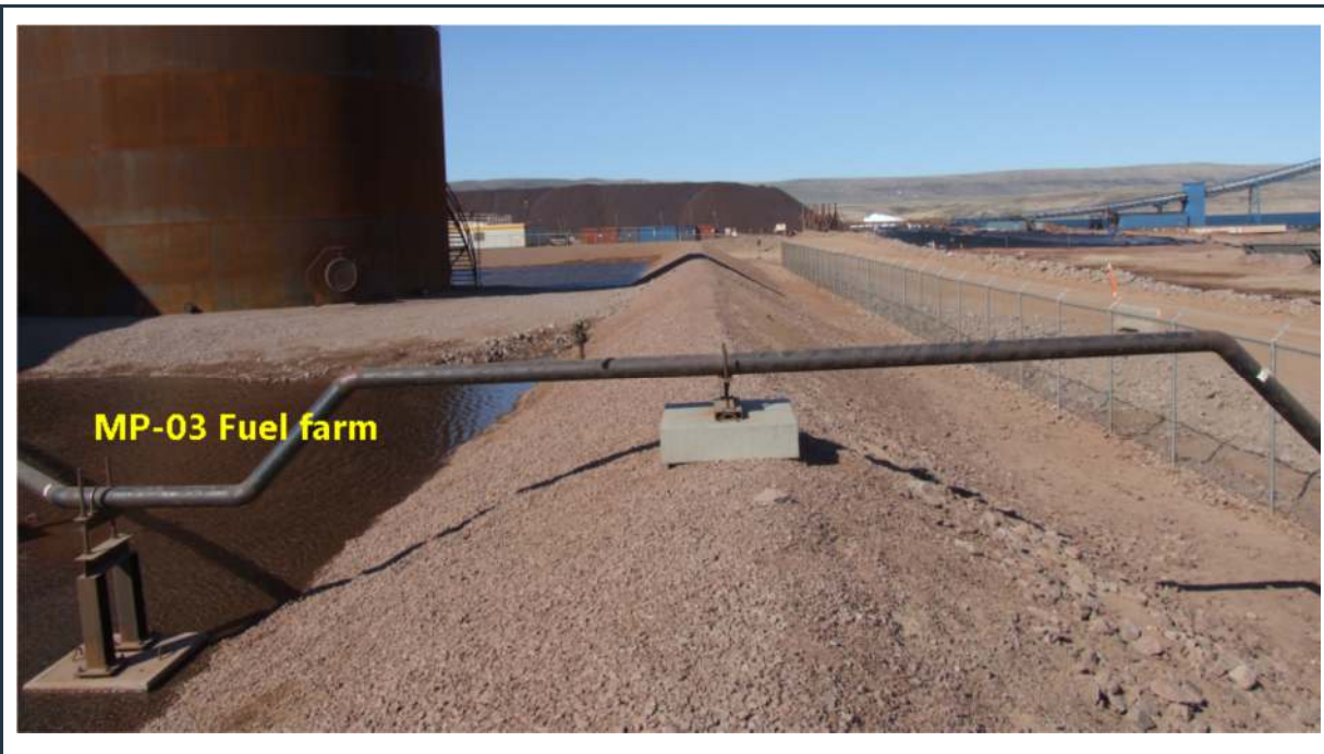
Figure 51: View of stable, well maintained berms around the MP-03 fuel tank farm
