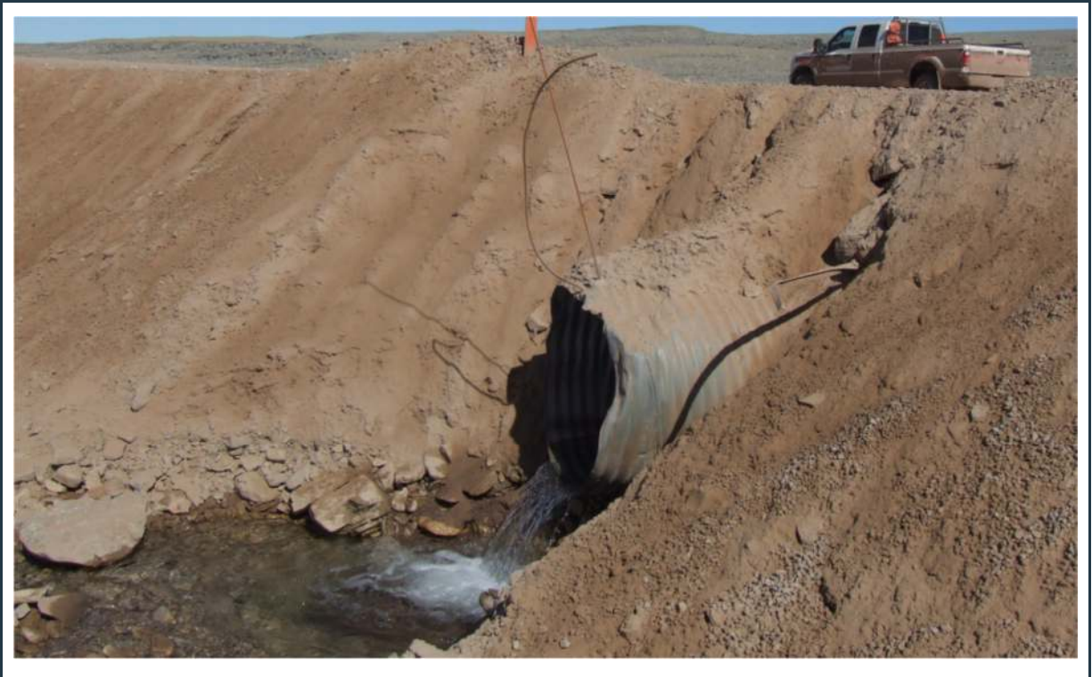
Figure 86: View of culvert 083 (outlet) with some slope erosion
