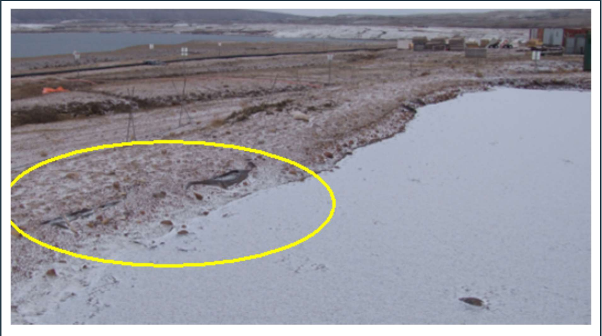
Figure 27: View of the locally low generator berm (high water level with frozen surface).
