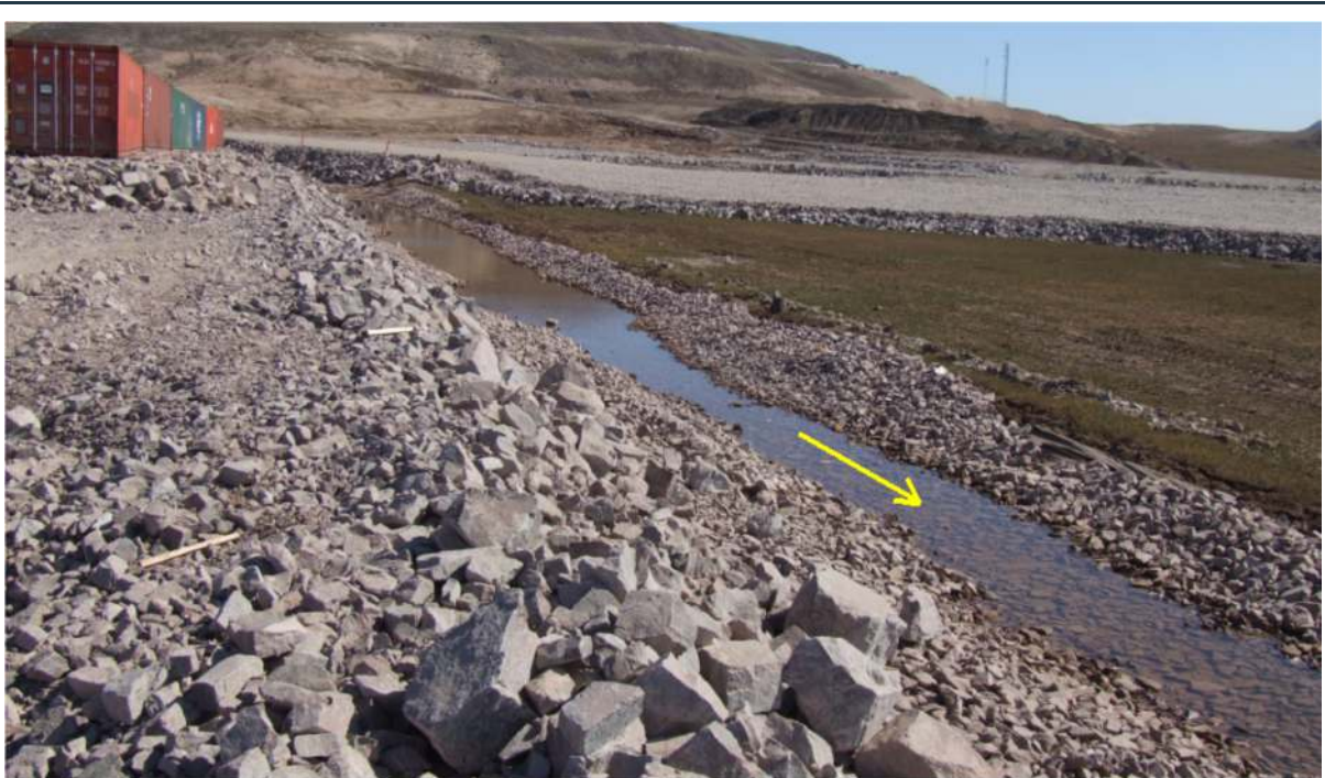
Figure 67: 380 M surface water collection ditch (under construction)
