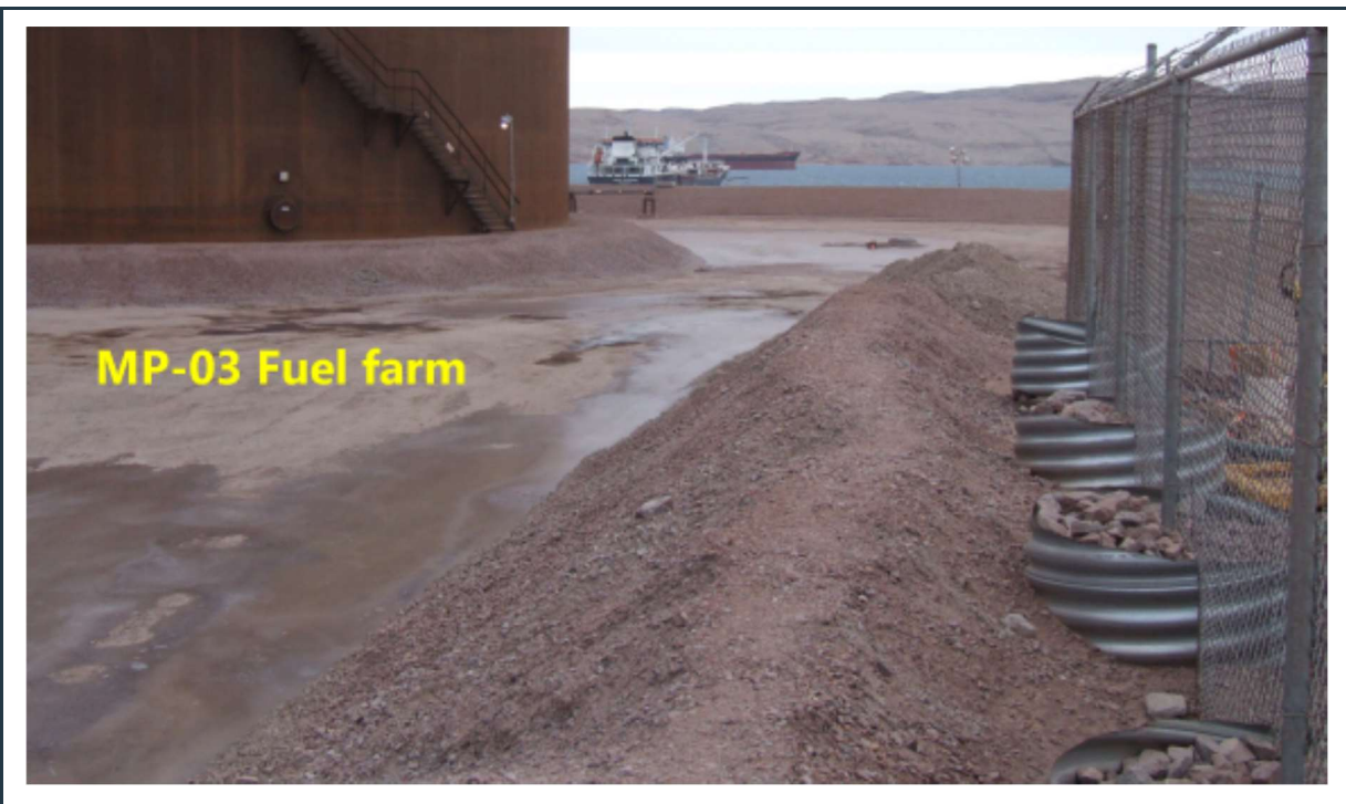
Figure 46: View of stable, well maintained berms around the MP-03 fuel storage.
