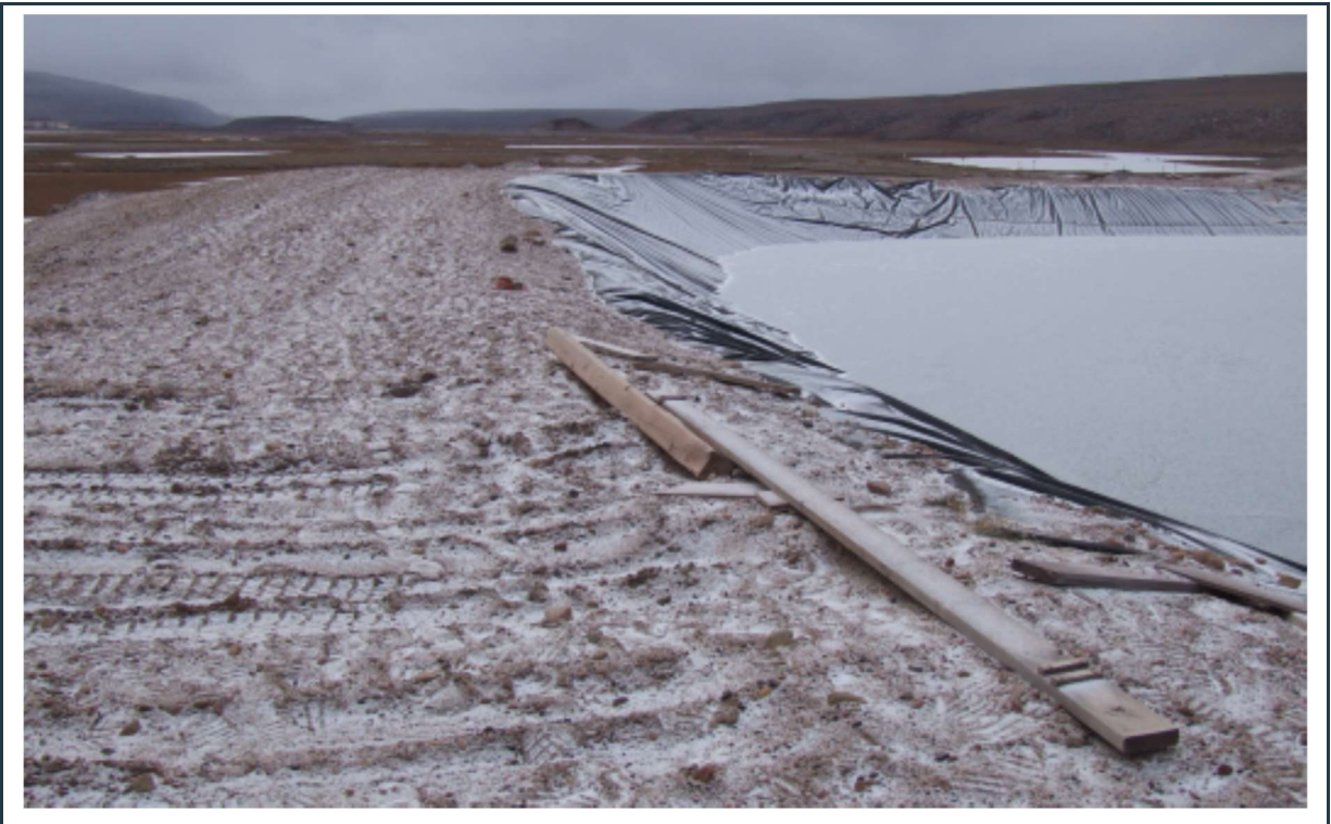
Figure 7: PWS pond #3 – Timber/lumber debris visible on the crest that should be removed.
