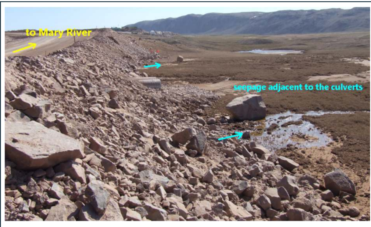
Figure 70: Water seepage through the road embankment adjacent to the tote road culverts
