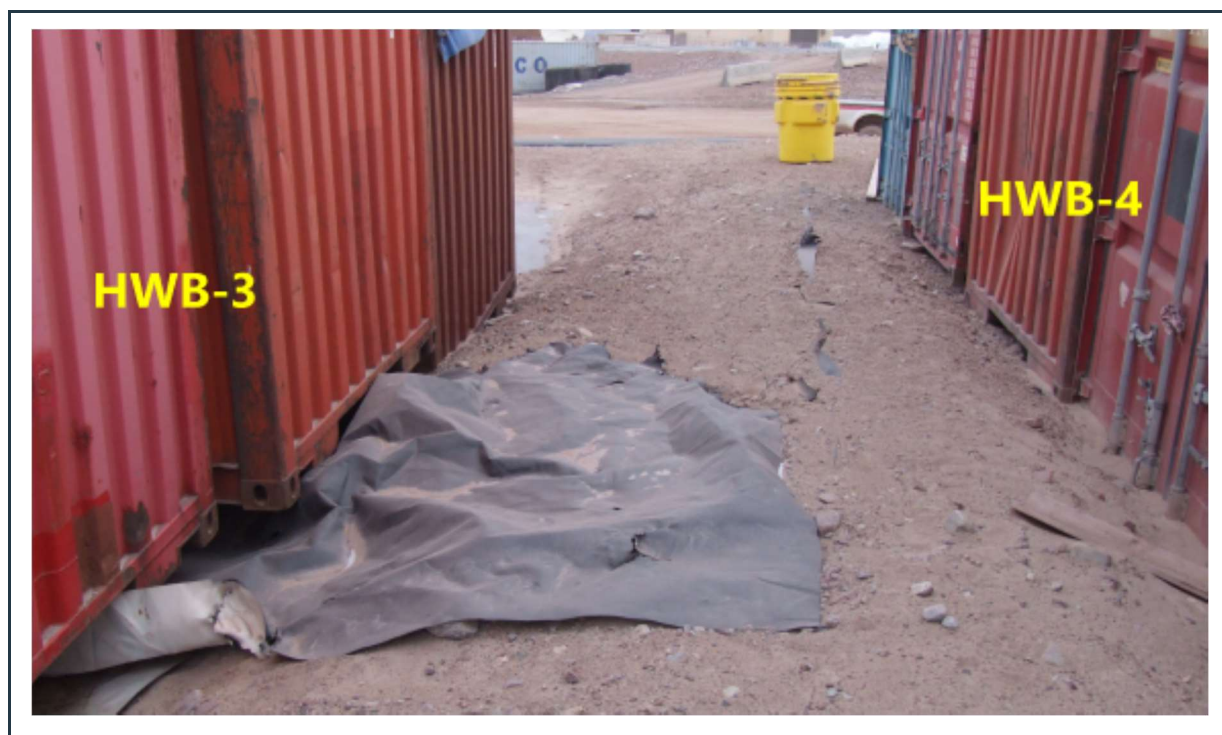
Figure 44: Exposed liners between the HWB-3 and HWB-4 cells.
