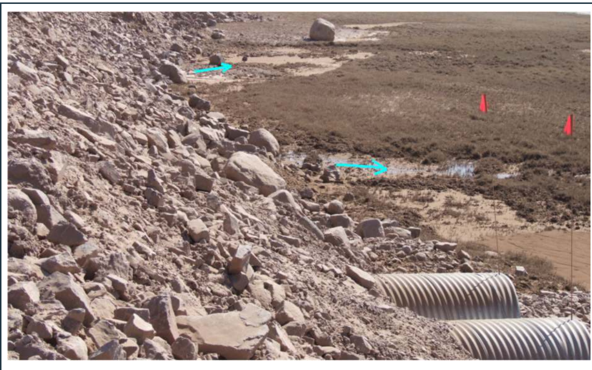
Figure 71: Water seepage through the road embankment adjacent to the tote road culverts
