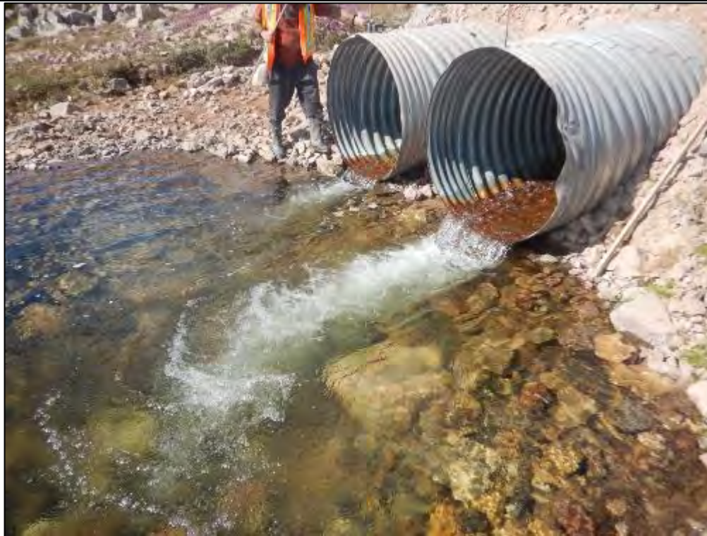
Photos 8: Photograph of the downstream end the perched culvert before remediation at CV-225. Remediation could not be completed in 2019.
