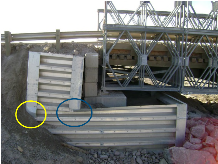
Photo 33 (2712): KM 64 Bridge, south abutment. Note tilting of upper bin wall, buckling of back bin wall corner post (yellow) and bending of upper plate in the lower bin wall (blue).
