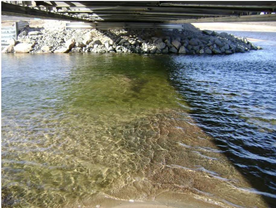
Photo 35 (2718): KM 80 Bridge, road surfacing gravel that has fallen through the centerline joint in the bridge deck and is visible in the river.
