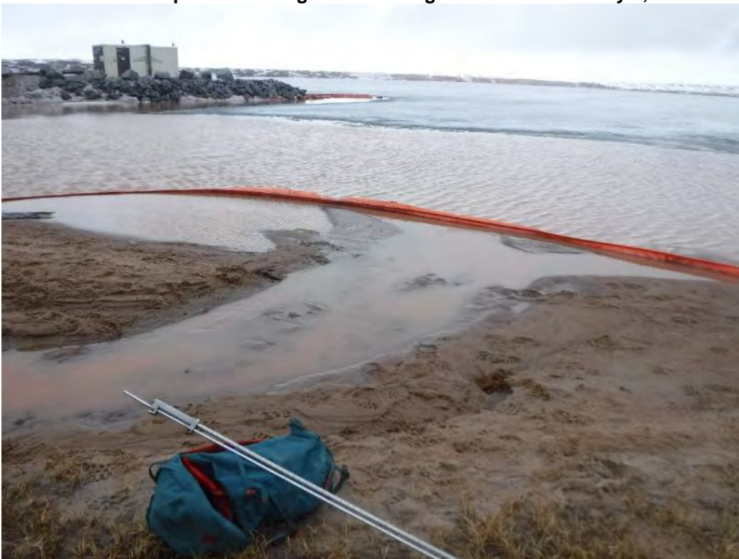
Photo 4. CLSP Outfall into silt curtain on May 9, 2019
