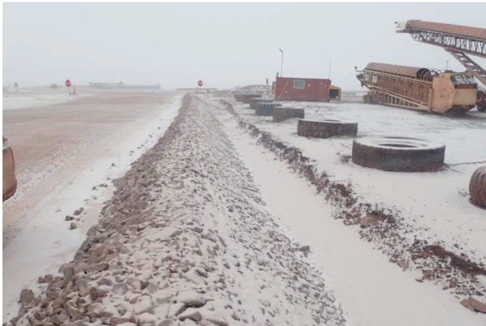
Figure 2. Restored ditches on the South East corner of the Milne Ore Pad to the Entrance Road. (Photo looking south west)
