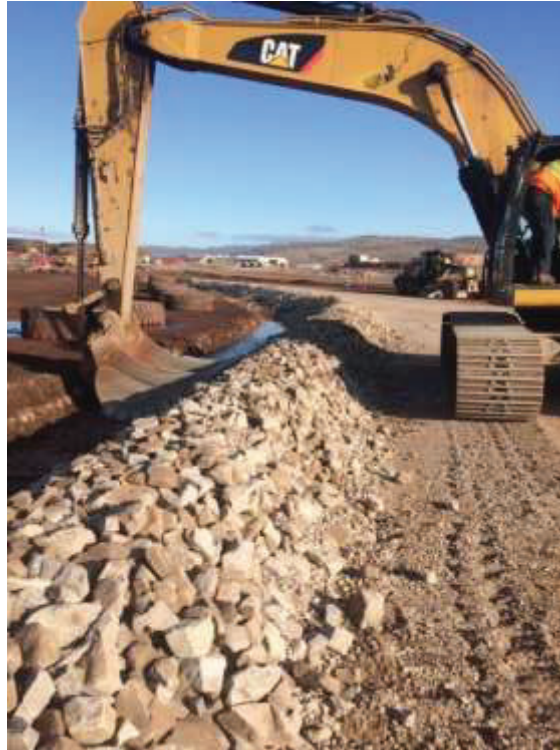
Figure 1. Southeast Ore Pad ditch restoration. (Photo looking north-east)
