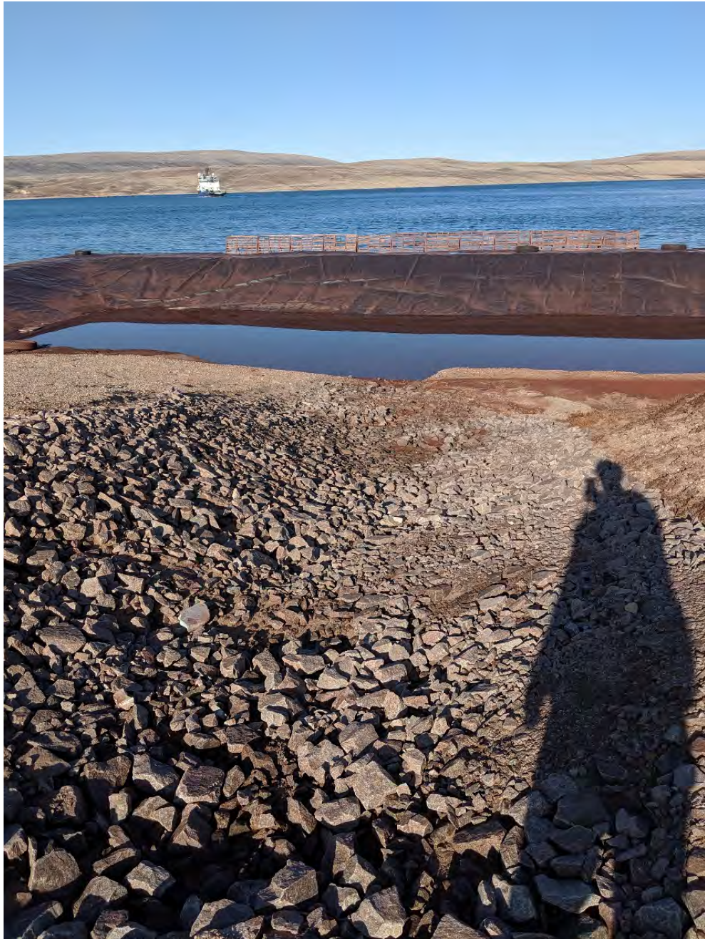
Photo 4: MP-06 Liner Key-In Repairs
