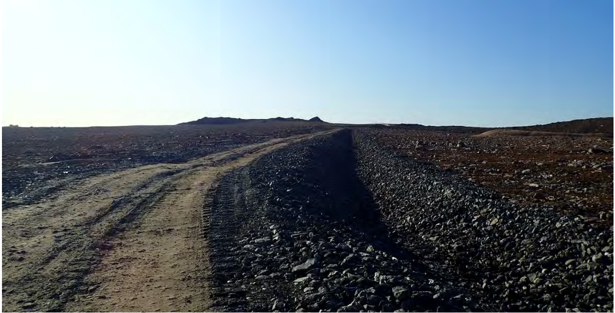
Photo 1: Ongoing Construction of WRF East Perimeter Road and Collection Ditch
