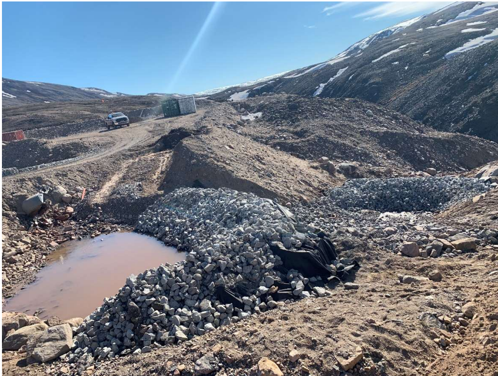
Figure 3: 2019 KM106 Check Dam and Gabion Basket Upgrades
