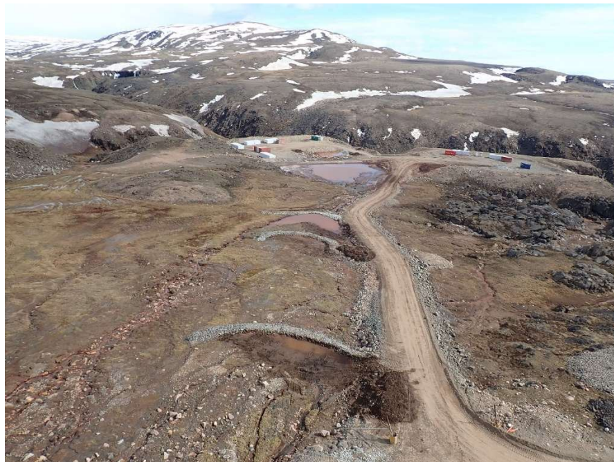
Figure 2: 2019 KM 106 Check Dam Upgrades from Above
