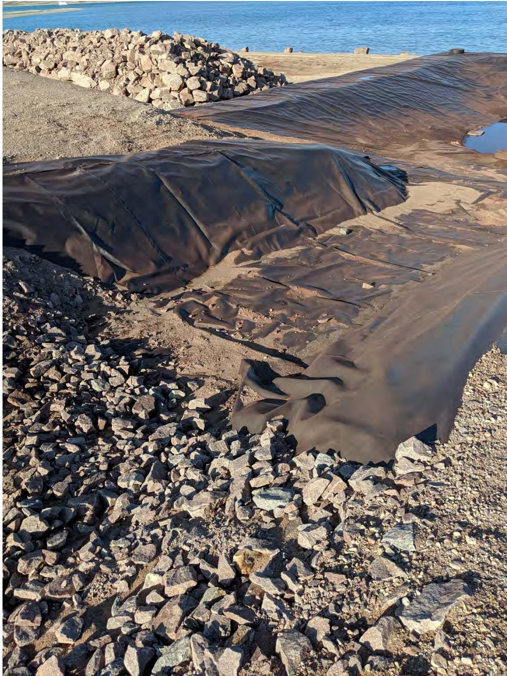
Photo 3: MP-06 Liner Key-In Repairs
