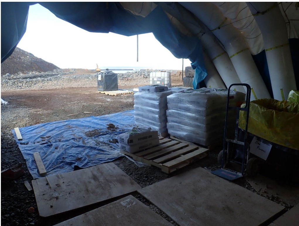
PHOTO 4 – Lime secondary containment at WRF Water Treatment Plant
