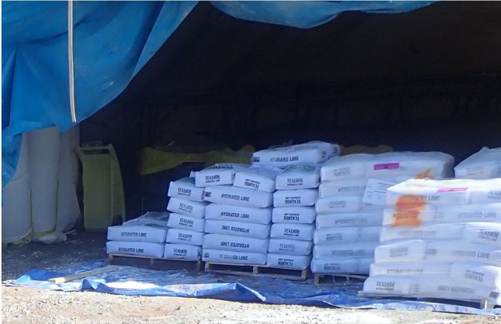
PHOTO 5 – Lime placed on secondary containment at WRF Water Treatment Plant
