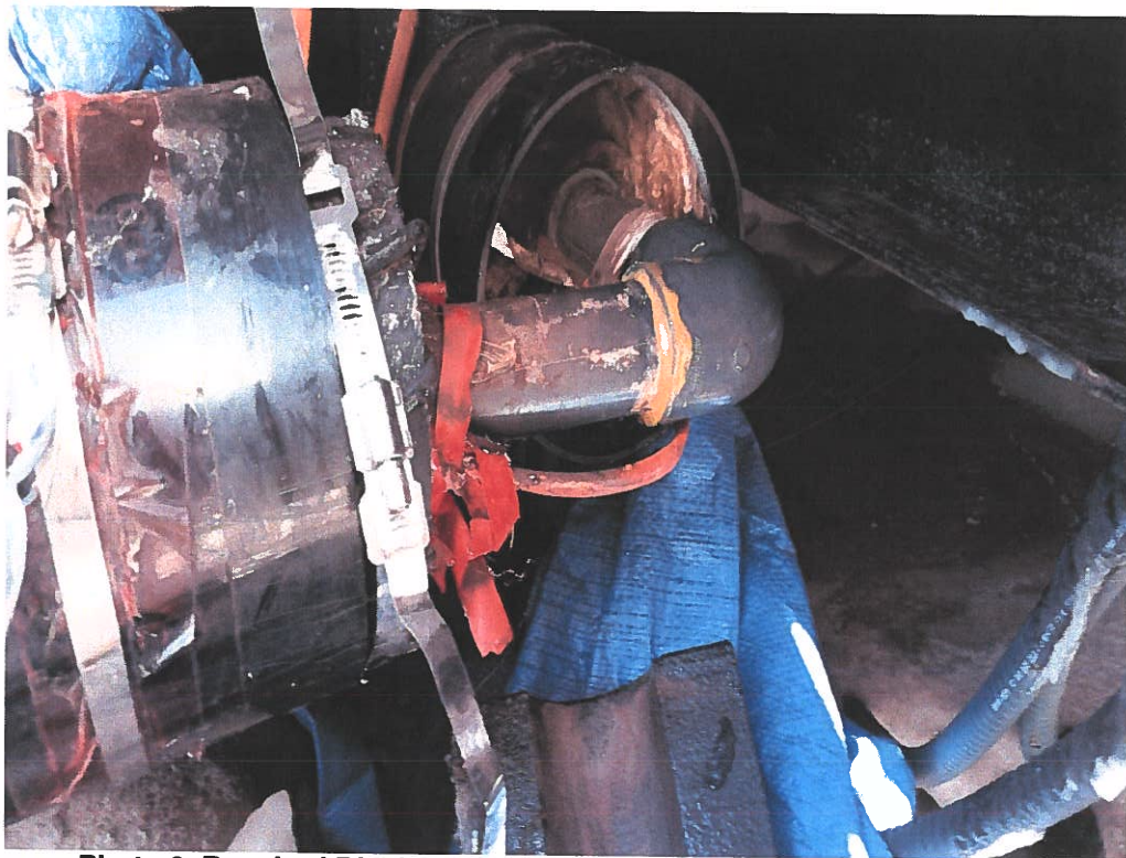
Photo 2. Repaired Discharge Line under AD wing prior to reinsulation.
