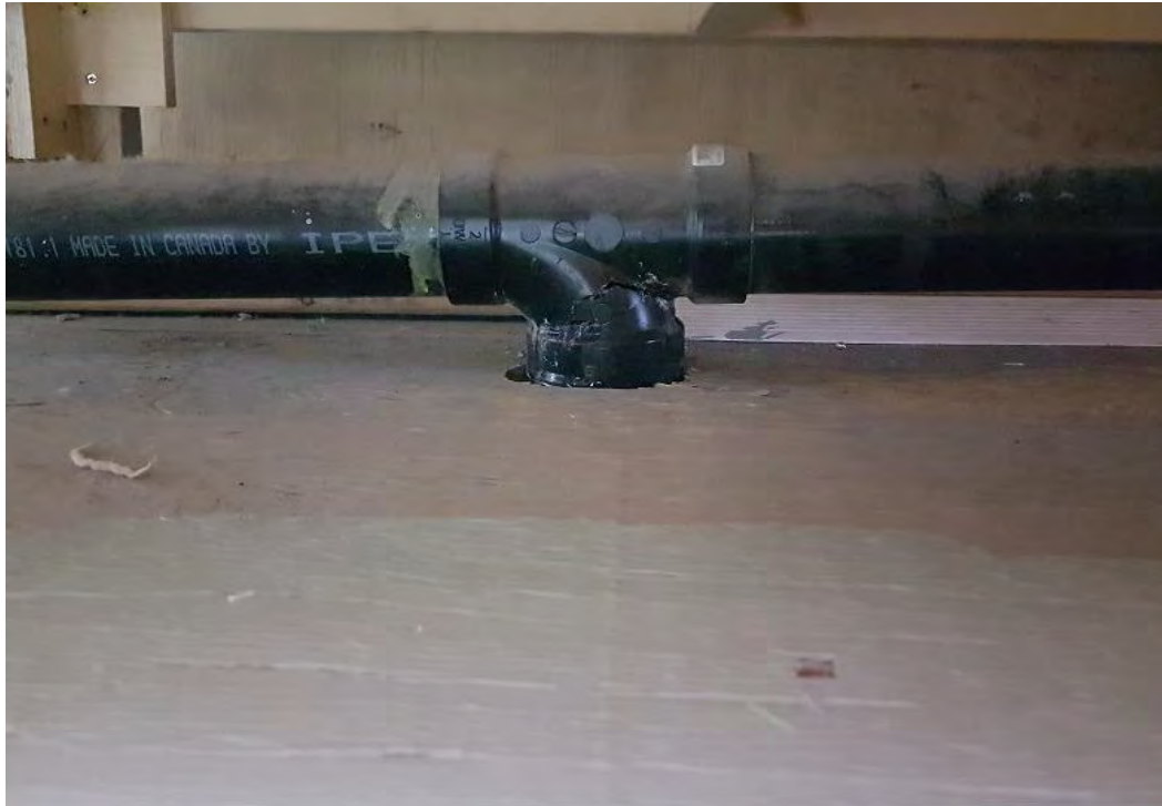
Photo 1. Damaged drain below women's bathroom.
