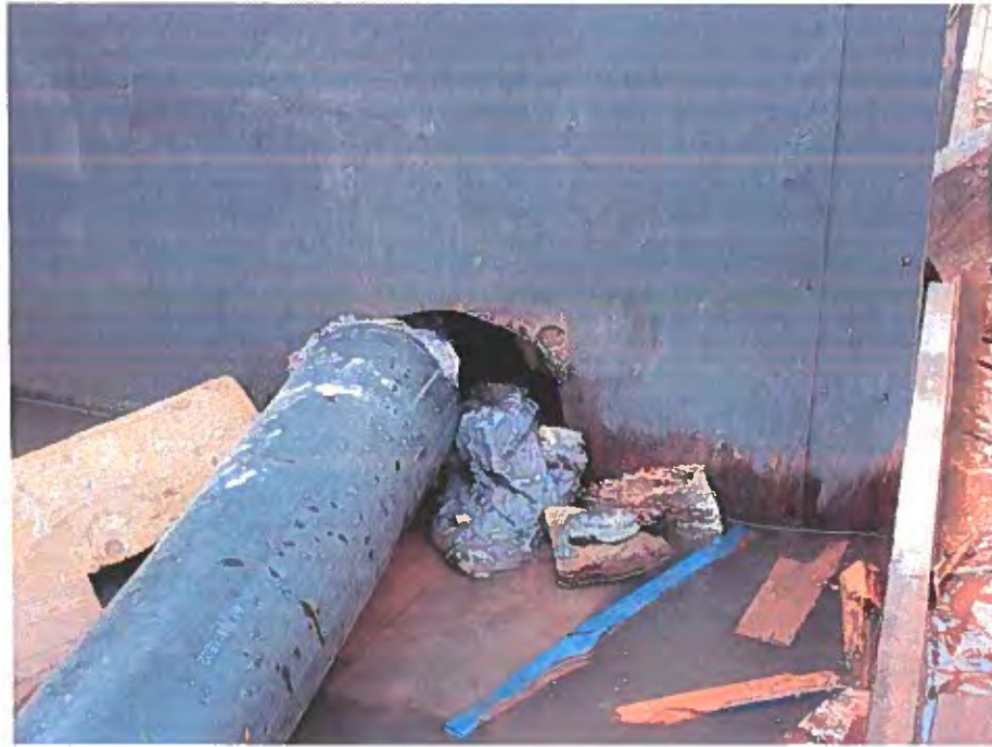
Photo 1. Separated Discharge Line under Weatherhaven lift station.
