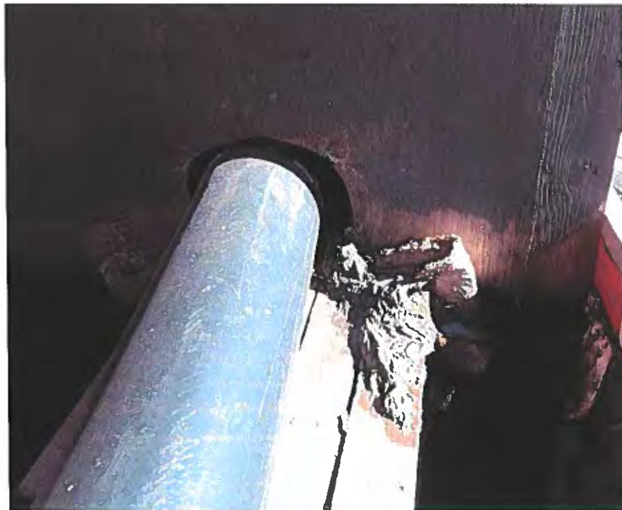
Photo 2. Repaired Discharge Line under Weatherhaven lift station.
