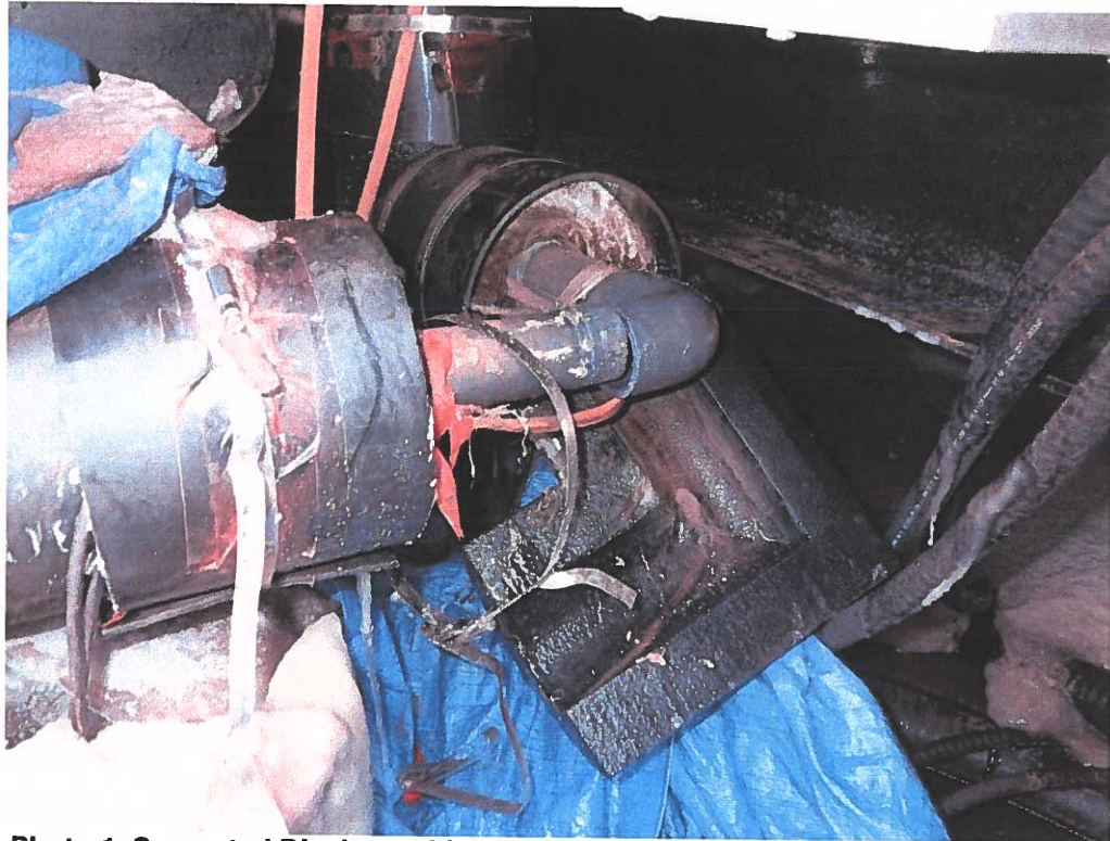
Photo 1. Separated Discharge Line under AD wing following insulation removal.
