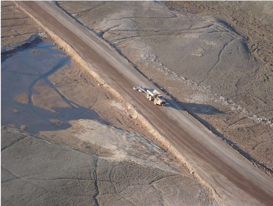
PHOTO 3 – 740 Tire Drag for Dust Suppression – September 2019
