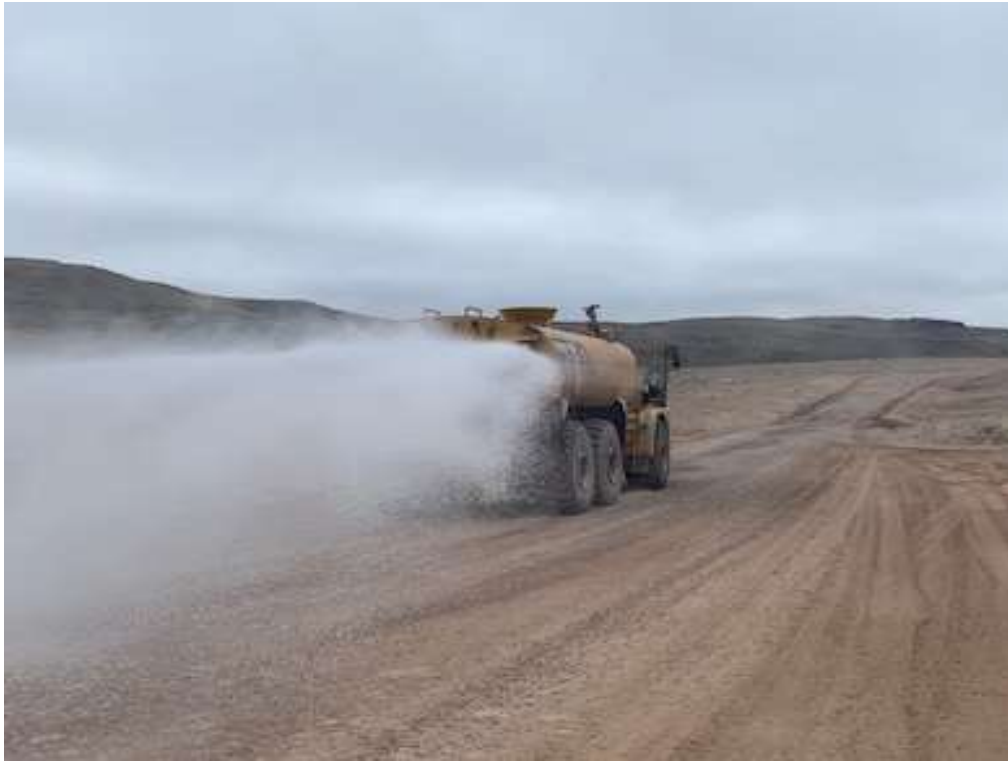
PHOTO 1 – Dust Suppression Water Truck on Tote Road – August 2019
