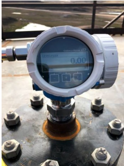
Photo 4-11: Radar Level Gauge
