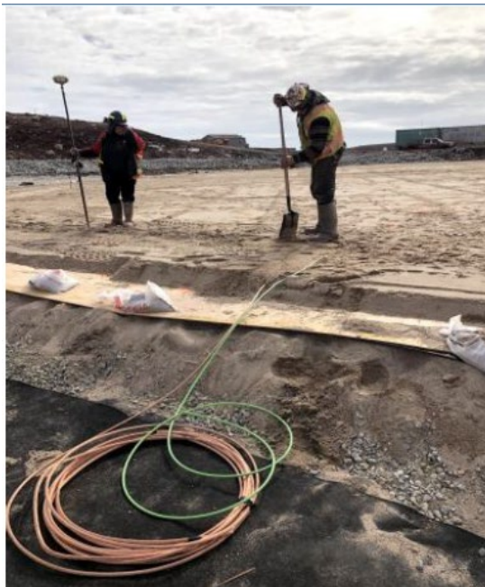
Photo 4-2: Grounding Grid Installation
