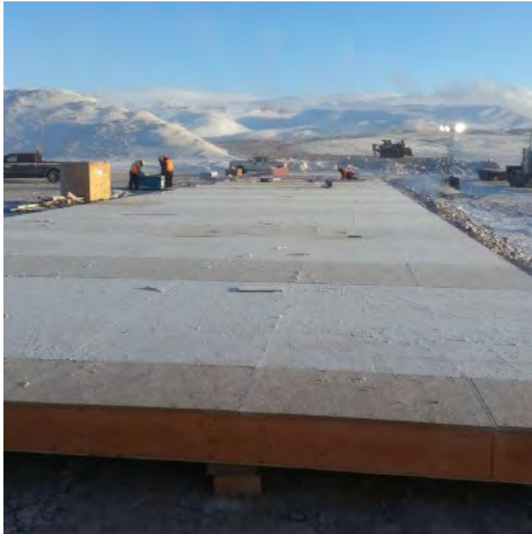
Photo 4-3: Floor Panel Placement
