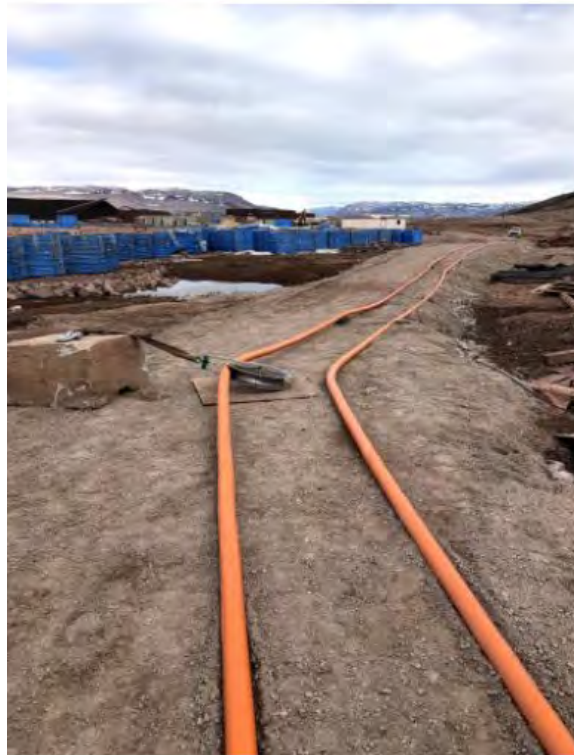
Photo 4-9: Power Supply Cables
