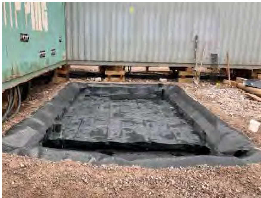
Photo 4-12: Transformer Containment
