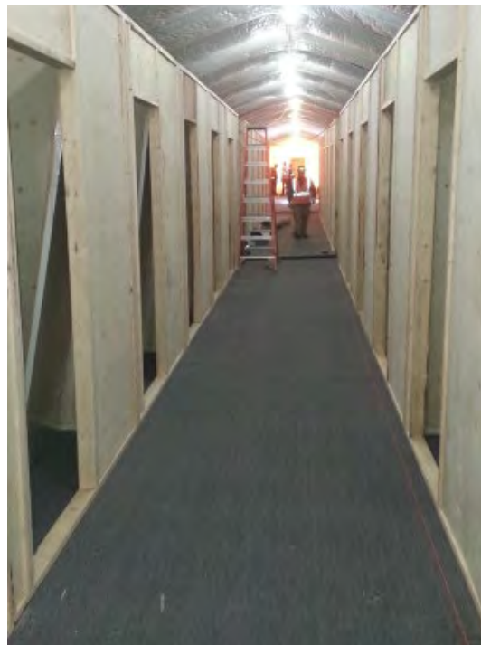
Photo 4-6: Dorm Wall Installation
