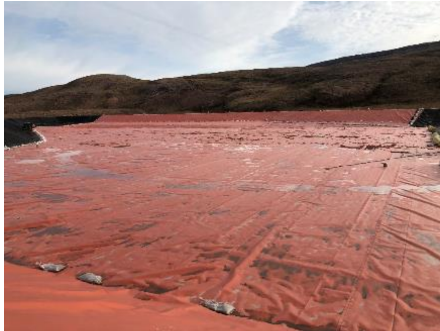
Photo 4-6: Liner Installation (remaining area)
