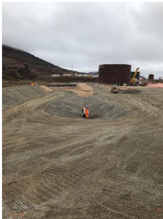
Photo 4-7: Earthworks Including One Sump
