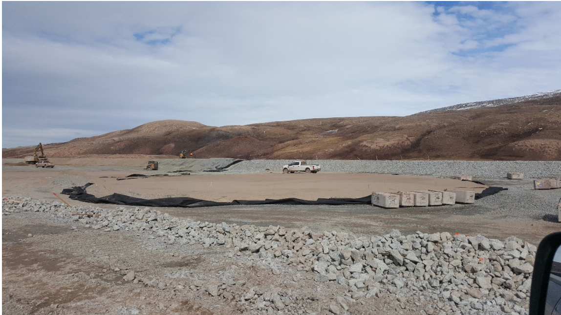
Photo 4-2: Preparing Pad for Tank 005
