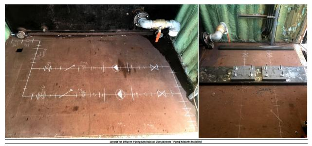
Photo 4-14: Effluent Pump Station Layout
