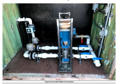
Photo 4-16: Effluent Pump Station Piping
