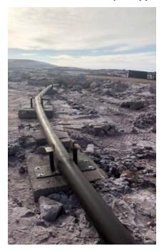
**Photo 4-8: Effluent Line Supports**
