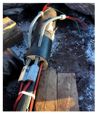
Photo 4-12: Effluent Line Heat Tracing
