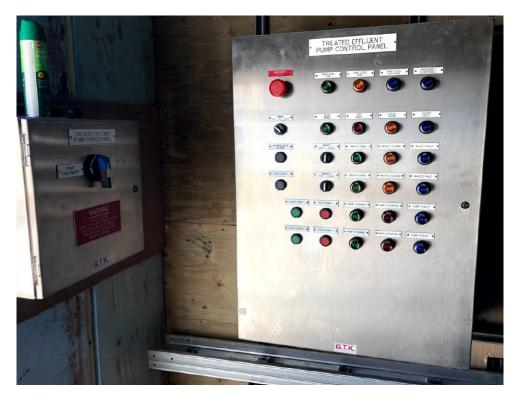
**Photo 4-17: Pump Station Control Panel**
