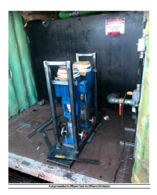
Photo 4-15: Effluent Pumps Installation
