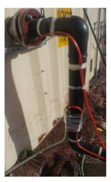
Photo 4-9: Effluent Line Heat Tracing
