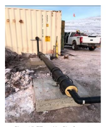
**Photo 4-7: Effluent Line Pipe Supports**
