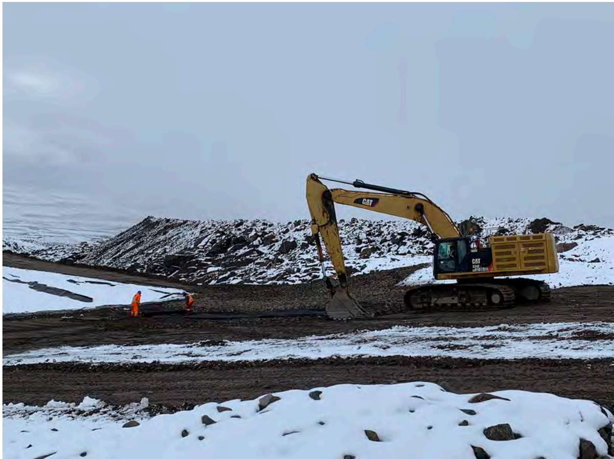
Placing Geotextile Fabric and Fine Riprap at Inlet - 12Sep20
