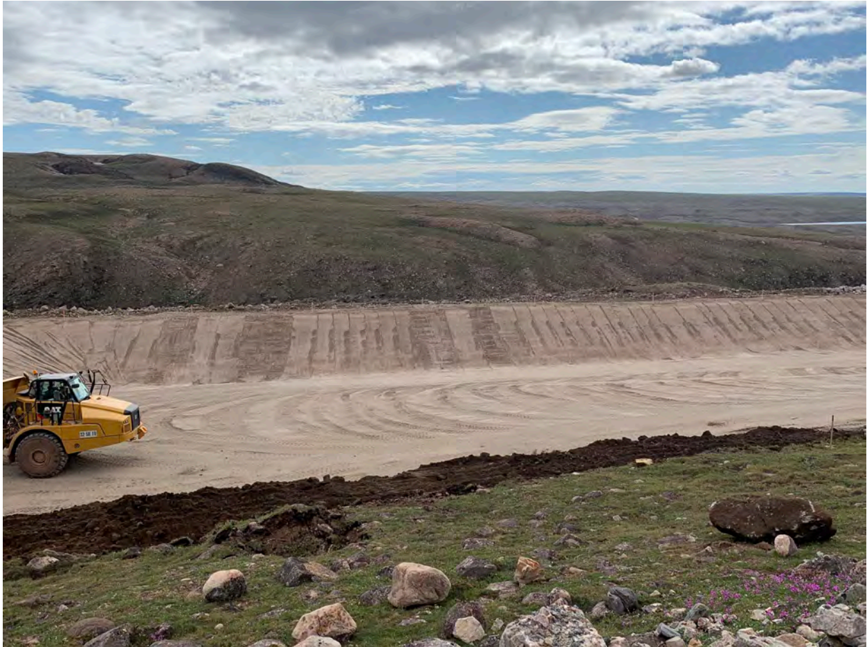
Preparing North Liner Anchoring - 21Jul20
