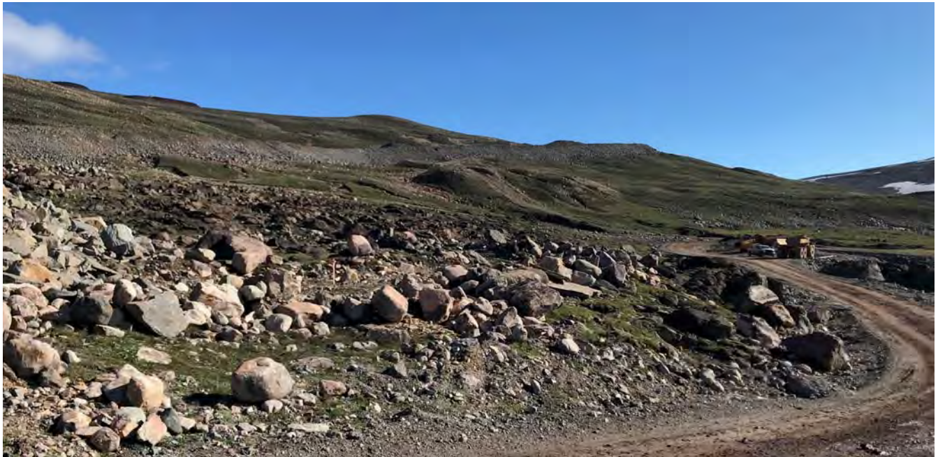
Location of Diversion Berm Where High Point Prevent Drainage Along Design Alignment
