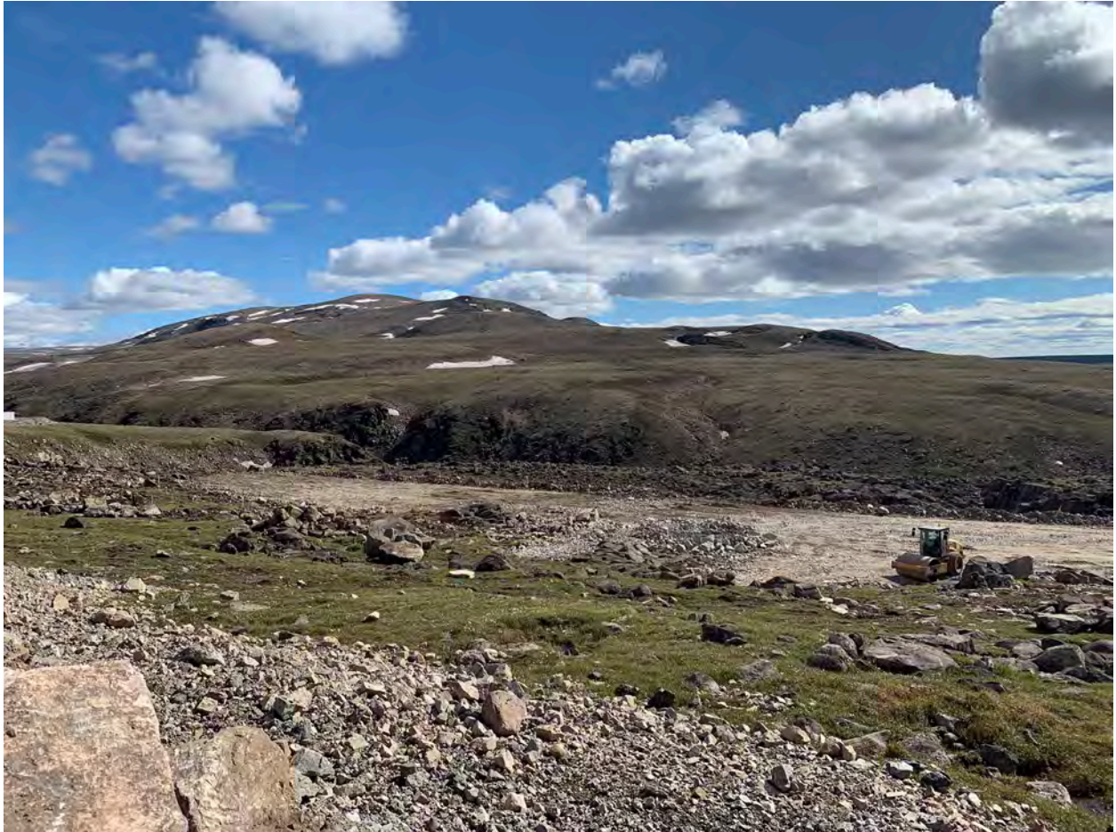
Placing 150mm minus material in Existing Crevices - 8Jul20
