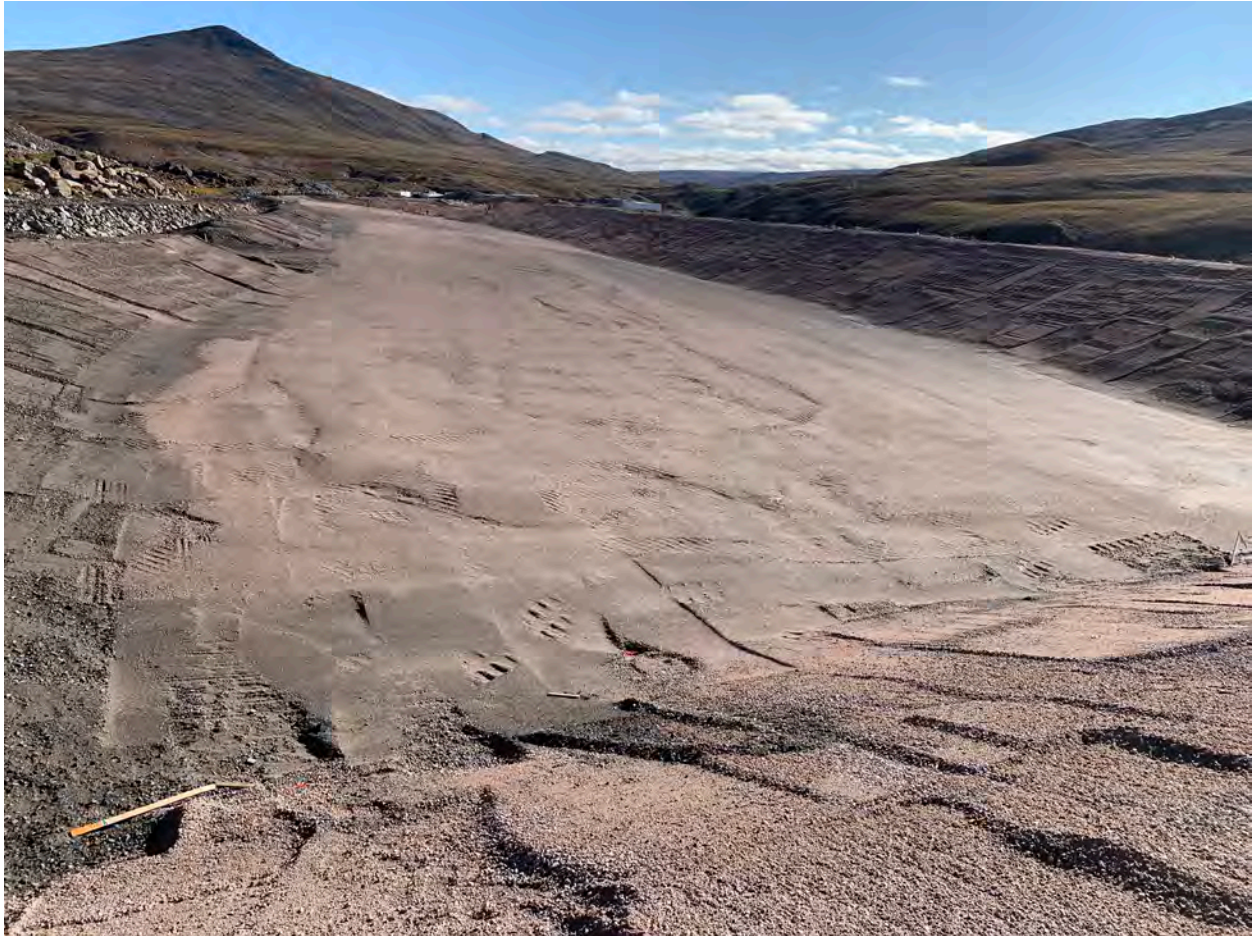
Placement of Intermediate Bedding - 20Aug20
