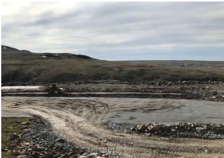
150mm Placement to the slopes
