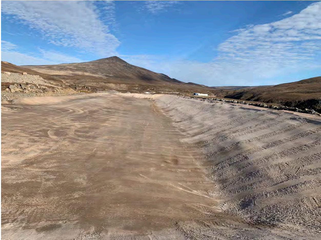
Completed Intermediate Bedding on Pond Bottom - 2Sep20
