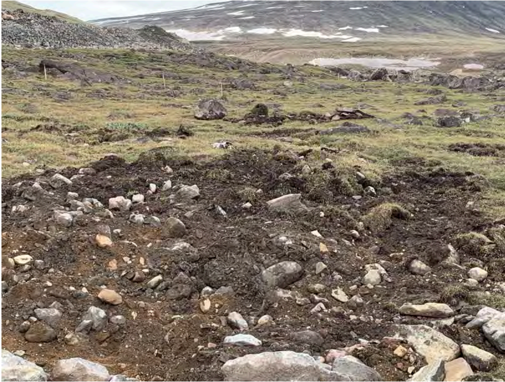
Prepare Foundation – Removal of Organic Material – 1Jul20
