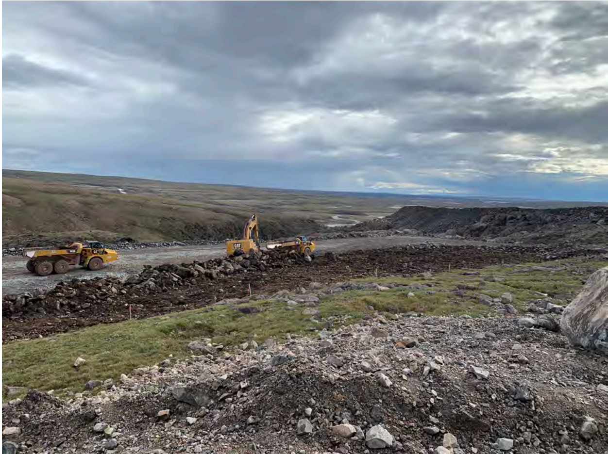
Pond Bottom Original Ground Preparation - 10Jul20
