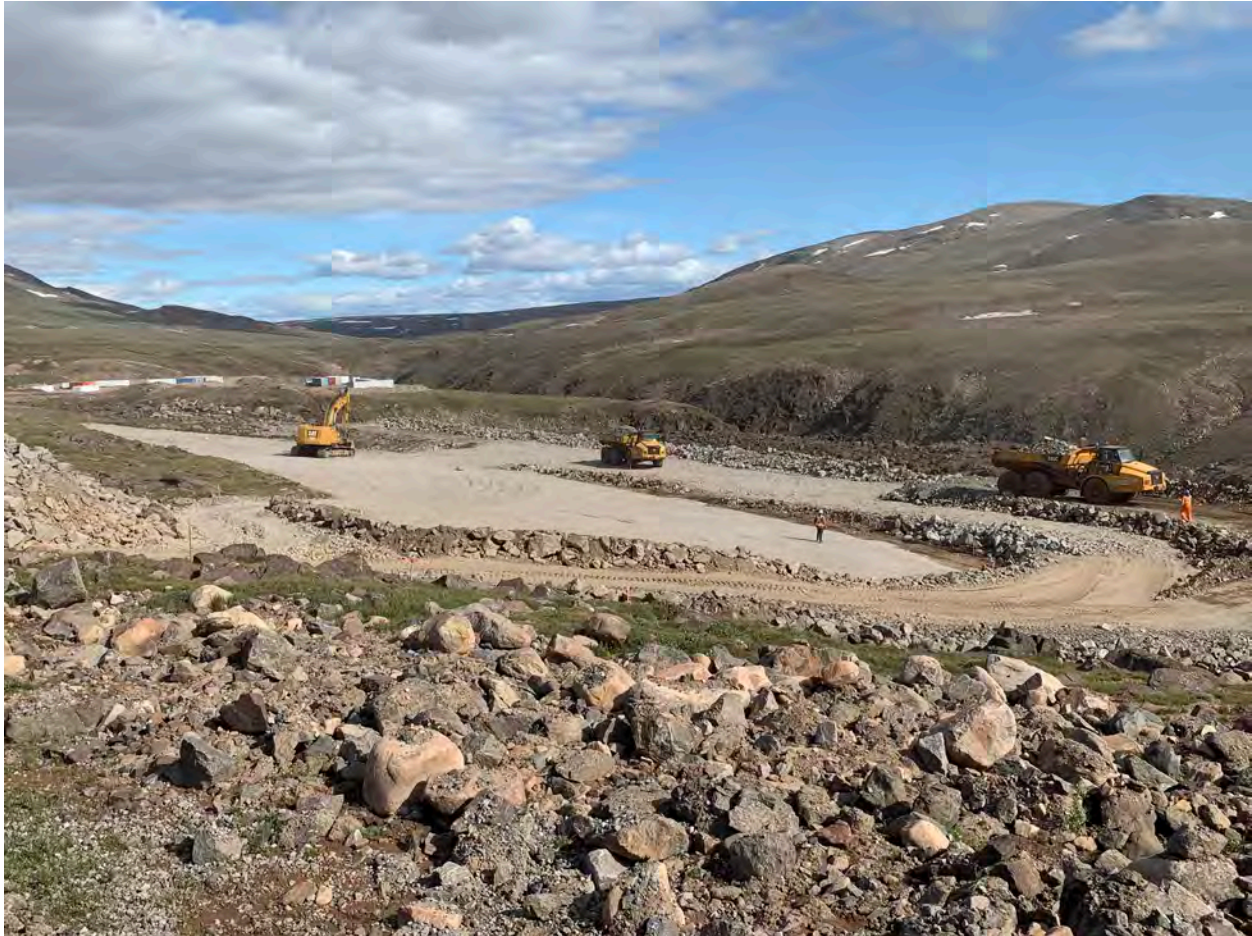
Placing ROQ on Berm and Placing 32mm minus Pond Bottom Layer - 13Jul20
