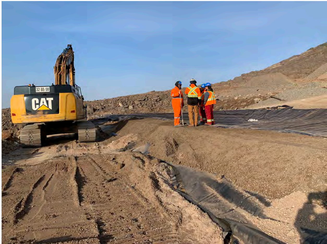
Backfilling Liner with \frac{3}{4} " minus Material in Anchor Trench - 9Sep20
