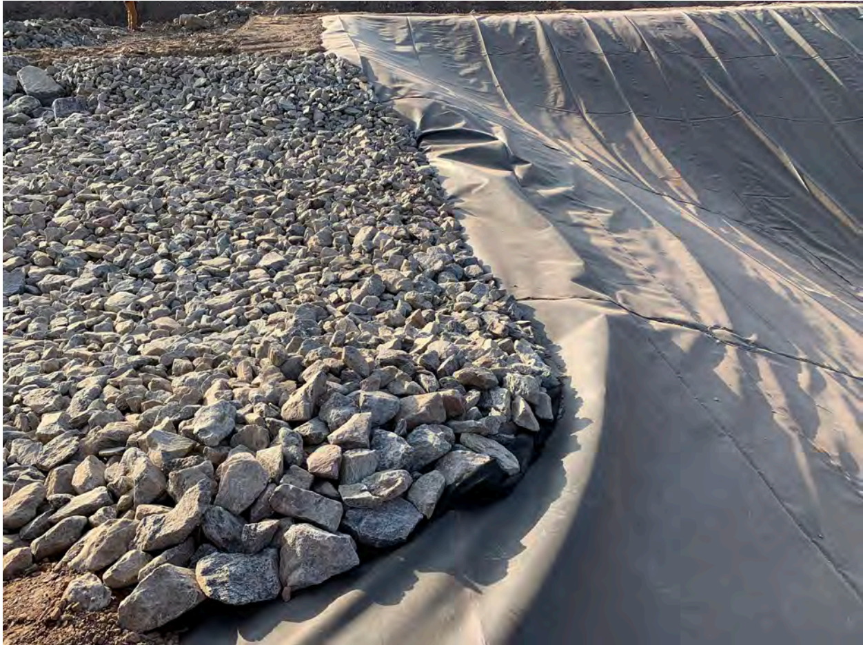
Photo of Spillway and Liner Transition - 9Sep20
