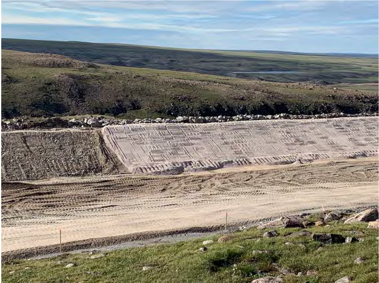
Placement of Intermediate Bedding - 20Jul20
