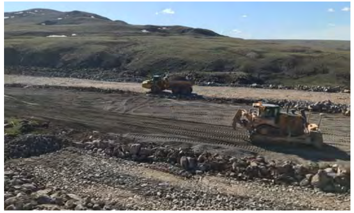
32mm placement to the floor
