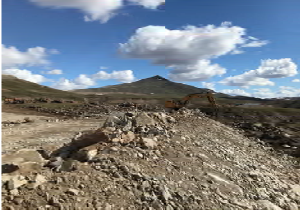
Trimming ROQ South slope
