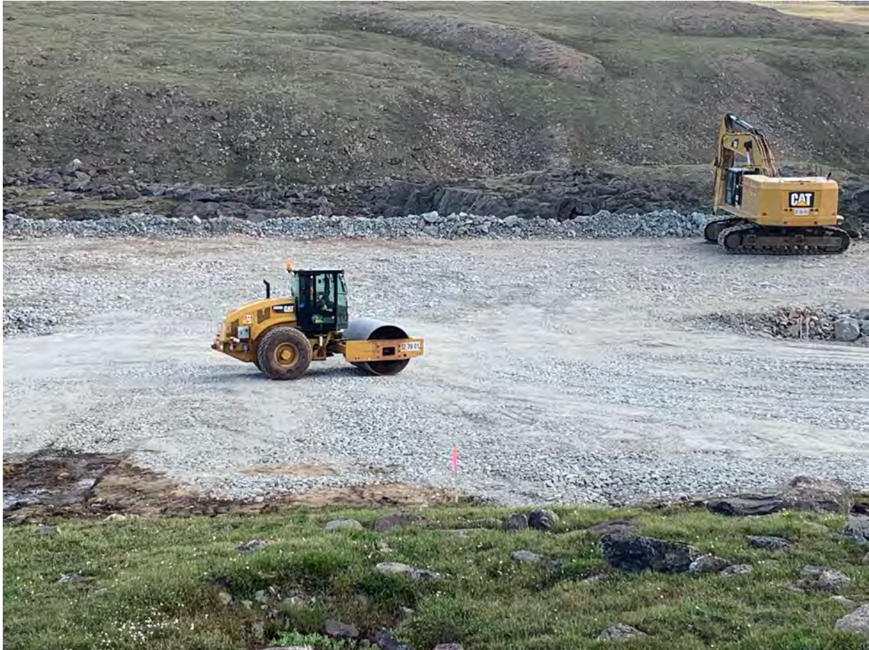
Placing 32mm minus layer on Pond Bottom - 12Jul20
