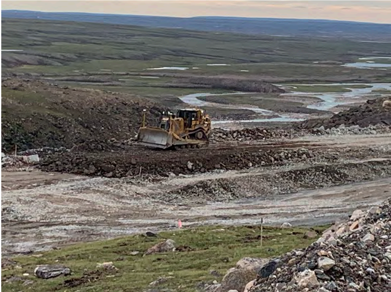
Placing ROQ in Layers on Berm - 15Jul20
