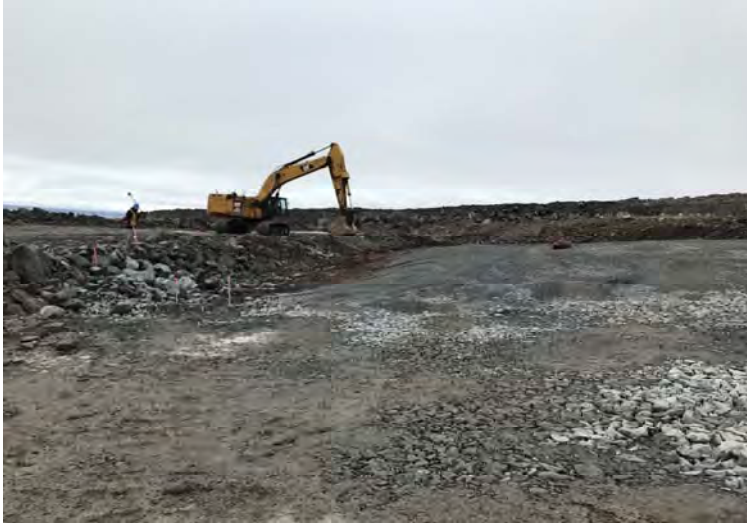
Trimming ROQ in preparation for 150mm placement
