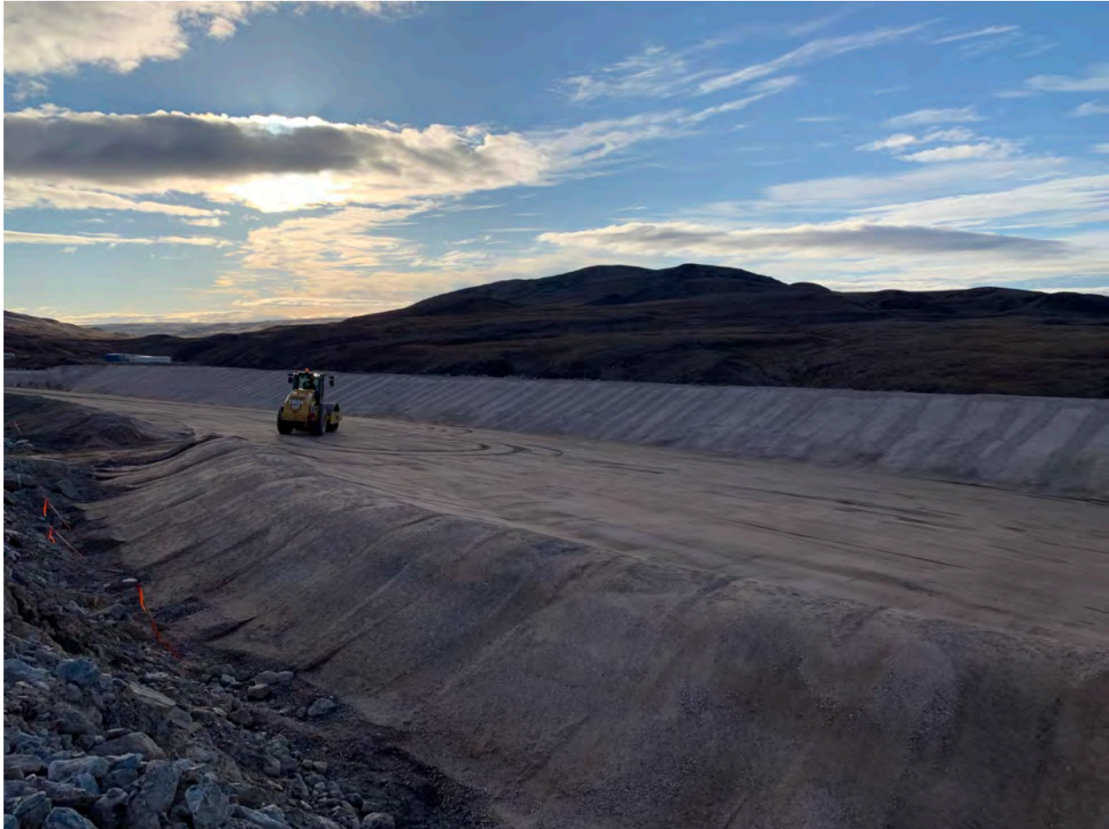
Compacting Intermediate Bedding - 3Sep20
