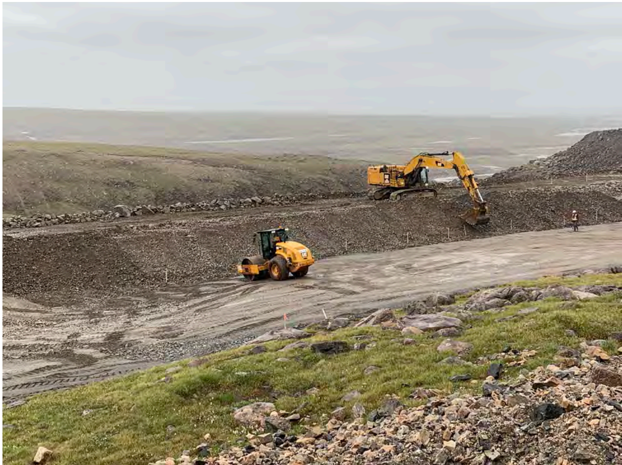
Placement of 150mm Minus on Upstream Side of Berm - 17Jul20
