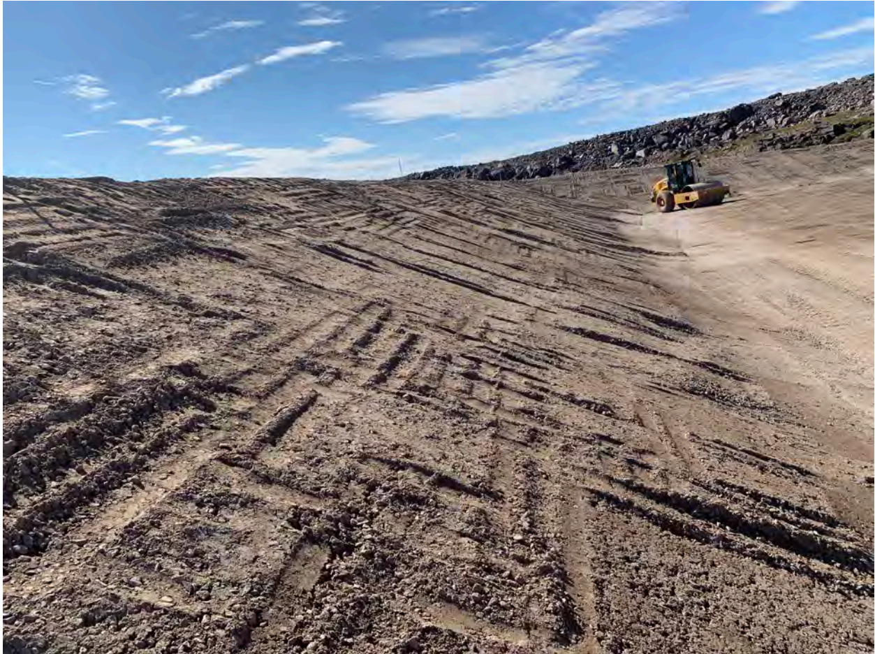
Placement of Intermediate Bedding Prior to Compaction - 19Jul20
