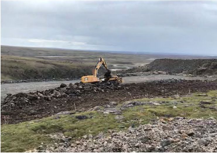
Boulders and Organics Removal / Waste Dump
