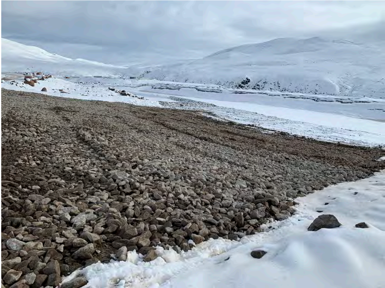
Completed Fine Riprap Placement at Inlet - 16Sep20
