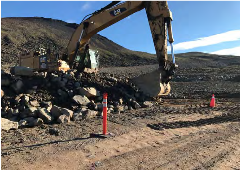
Trimming Berm Around 150mm Pad Next to Mag Road
