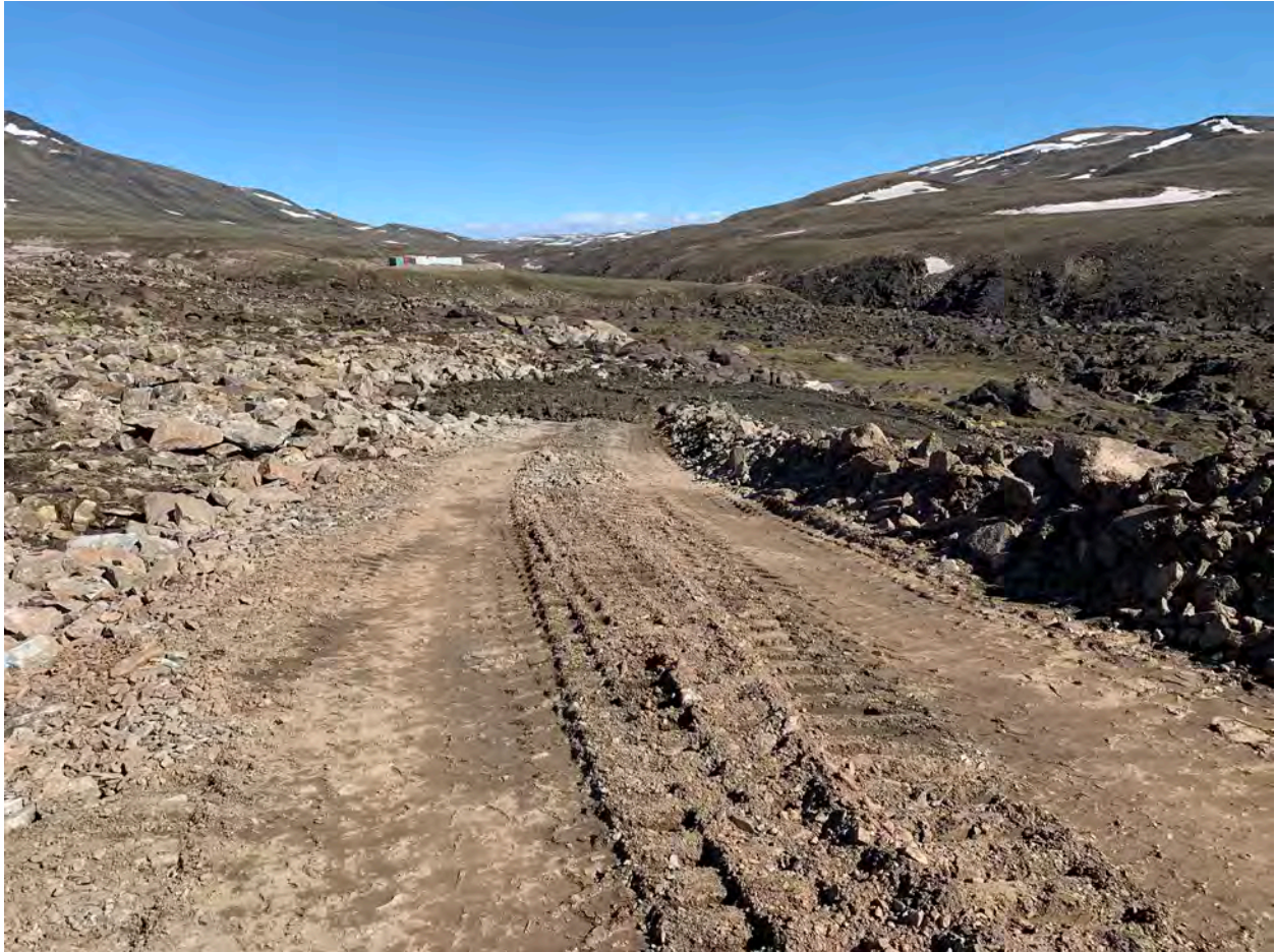
Extending 2 nd Layer of Berm Rise – 2Jul20
