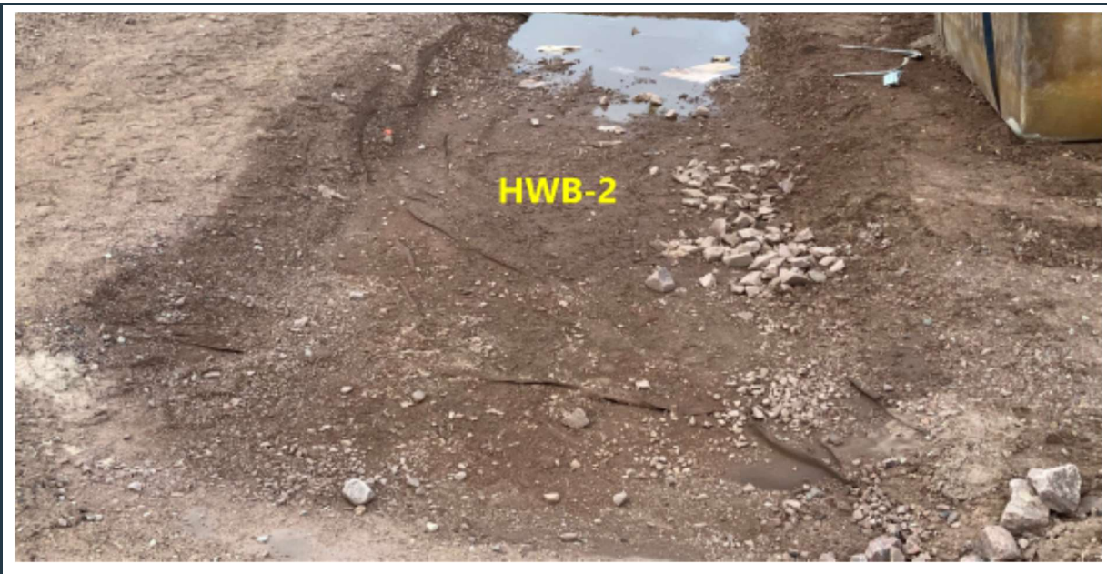
Figure 44: Ponding water in the empty HWB-2 cell with locally exposed geotextile and liner. Empty containers stored immediately adjacent to the cell.
