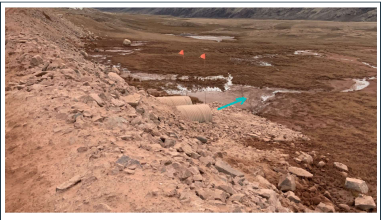
Figure 72: View of twin culverts, draining surface water from the quarry under the tote road (outlet).
