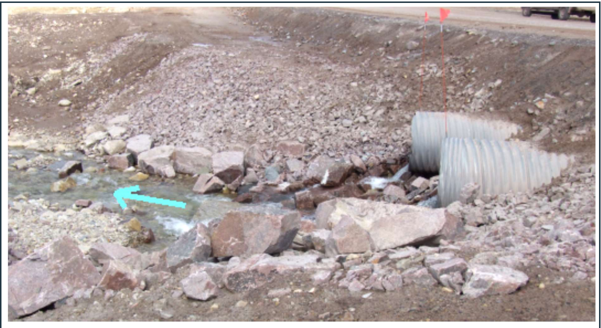
Figure 104: View of culvert(s) 094 (outlet) in good condition.
