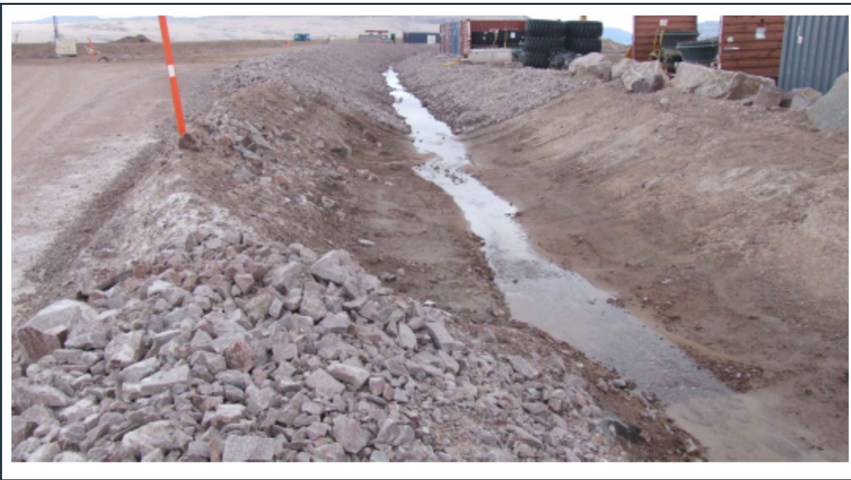
Figure 78: P-SWD-5 – "Q01-North" surface water collection ditch. Riprap is missing at one section.
