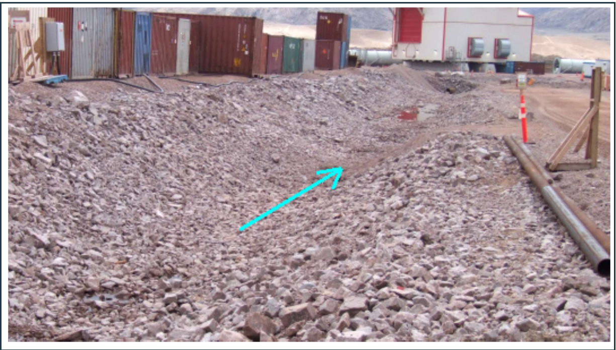
Figure 84: View of the east section of the 380 M surface water collection ditch, in good condition.
