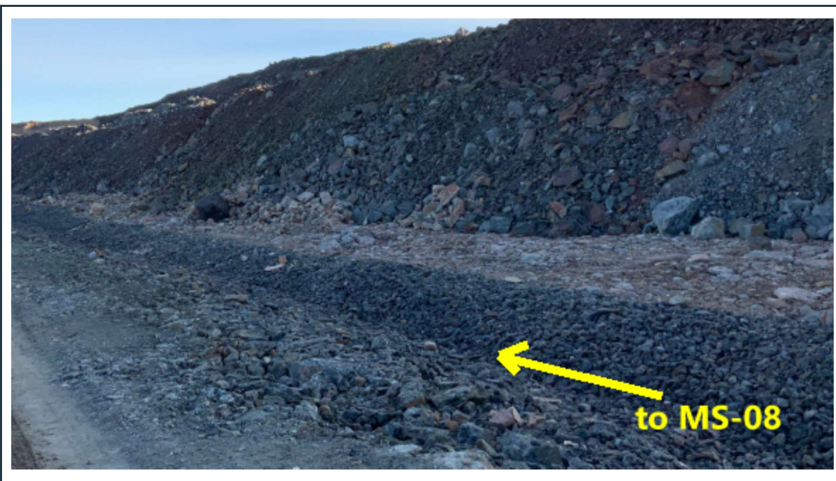
Figure 26: Well-maintained drainage ditch along the west side of the waste rock facility.
