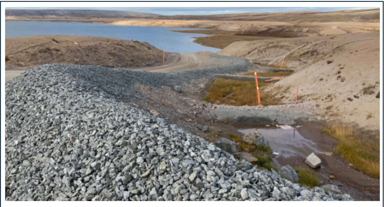
Figure 34: Camp Lake check dams and berms, forming efficient silt sedimentation cells
