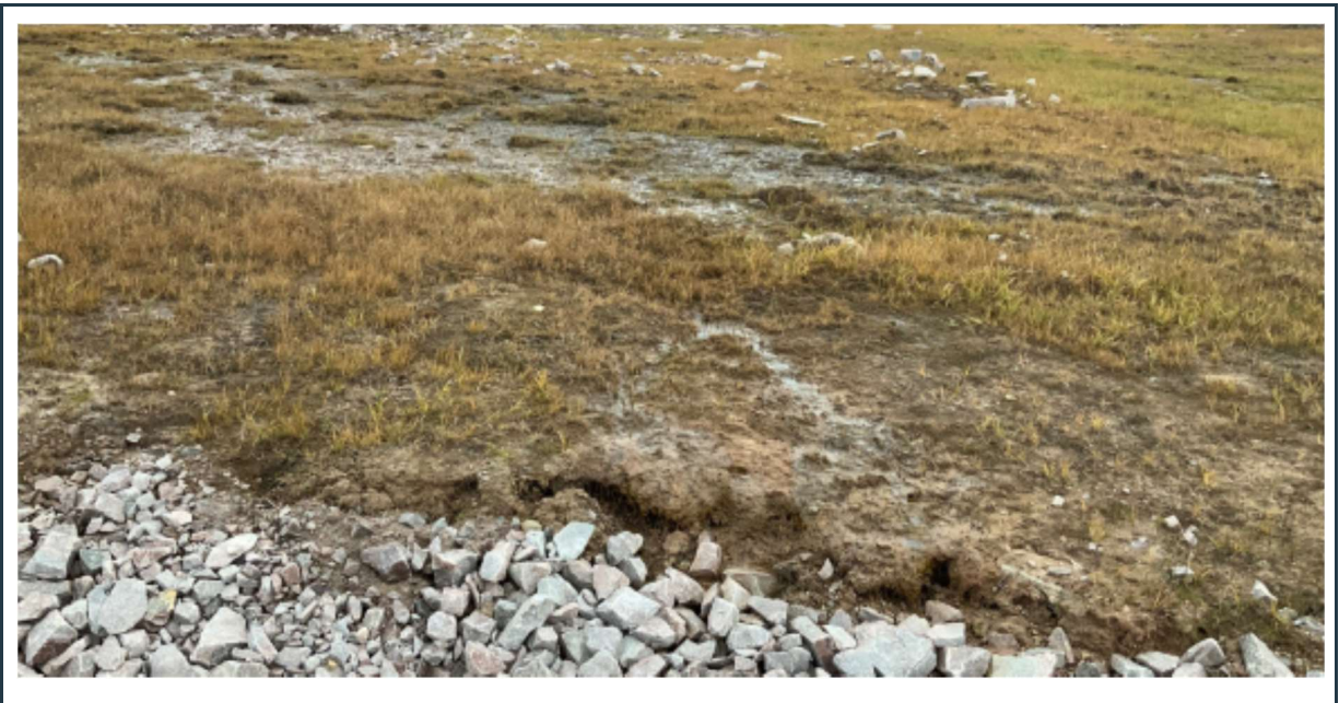
Figure 62: Continuous sheet flow of surface water from a large area, resulting in sloughing of one side of the P-SWD-3 ditch.
