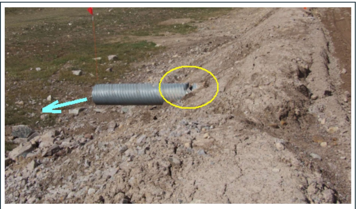
Figure 110: View of culvert 110A (outlet) with minor damage on the top of the pipe (yellow circle).
