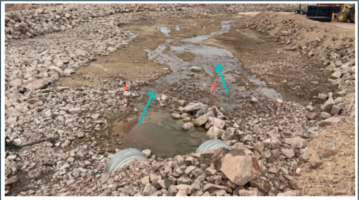
Figure 66: View of the P-SWD-7 surface water collection ditch and culverts (outlet).
