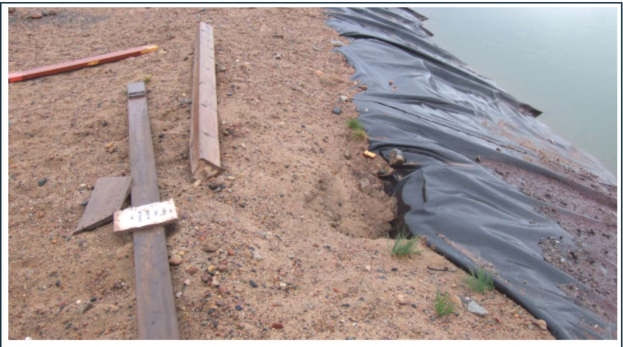
Figure 10: PWS pond #3 – Timber/lumber debris visible on the crest. Note the loss of some finer berm material (sand) into the voids of rock fill. The “sinkhole” should be filled and the debris removed.
