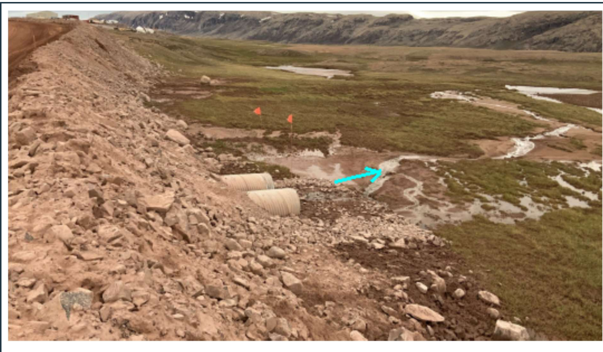
Figure 88: View of twin culverts, draining surface water under the tote road (outlet).
