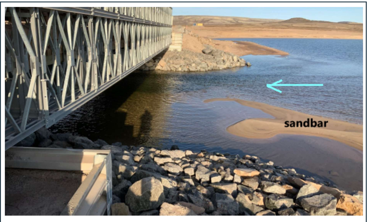
Figure 78: View of bridge 80, looking north. Note the sandbar in the river, blocking some of the flow.
