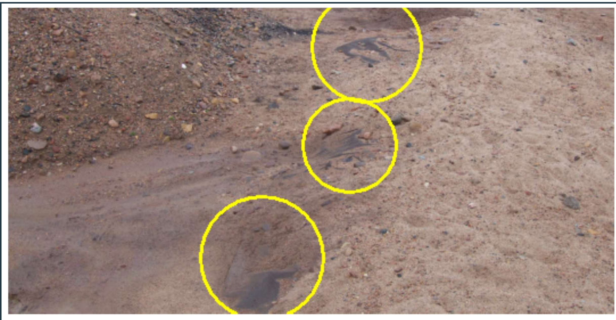
Figure 34: View of the south-east berm that needs to be repaired (raised and regraded). Note the exposed geotextile and liner that shall be covered with sand/gravel during berm rehabilitation.
