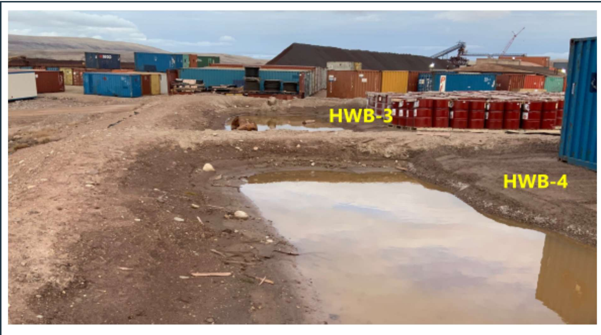
Figure 47: Stable berms around and ponding water within the HWB-3 and HWB-4 cells.
