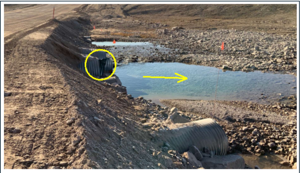
Figure 84: View of culvert(s) 078 outlet (looking south). Minor damage visible on one of the pipes (second from north - yellow circle).
