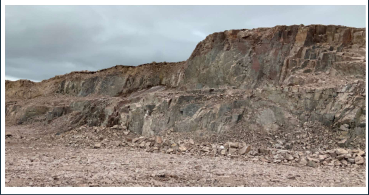
Figure 75: View of stable highwalls in the Q01 quarry.
