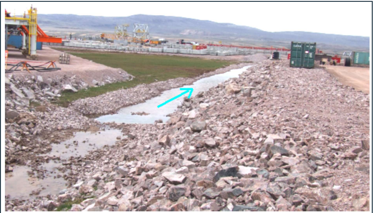
Figure 83: View of the south section of the 380 M surface water collection ditch, with minor riprap sloughing/rolling in the foreground.
