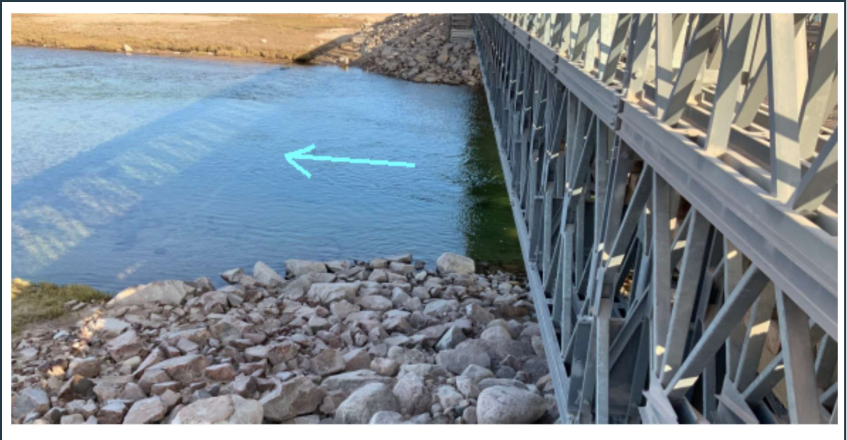
Figure 73: View of the north side of "bridge 17". Note the rip-rap scour protection at the abutments.
