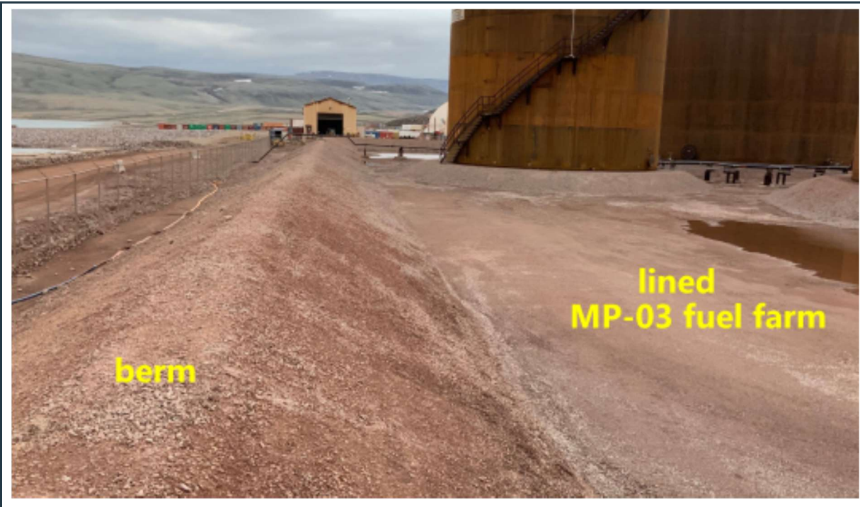
Figure 61: View of stable, well maintained berms around the MP-03 fuel tank farm.
