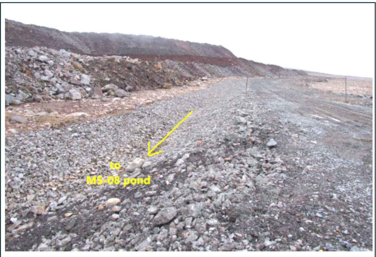
Figure 30: Well-maintained drainage ditch along the west side of the waste rock dump
