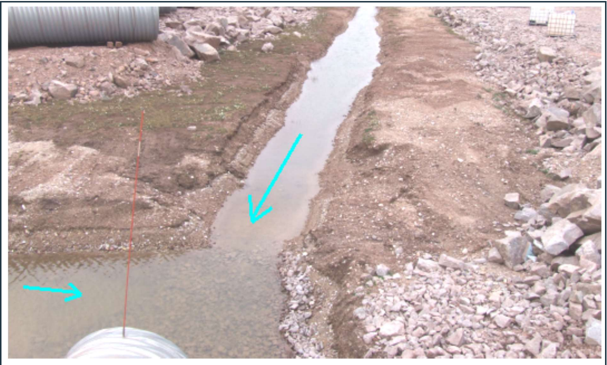
Figure 82: View of the W3/W14 surface water collection ditch and culvert inlet.
