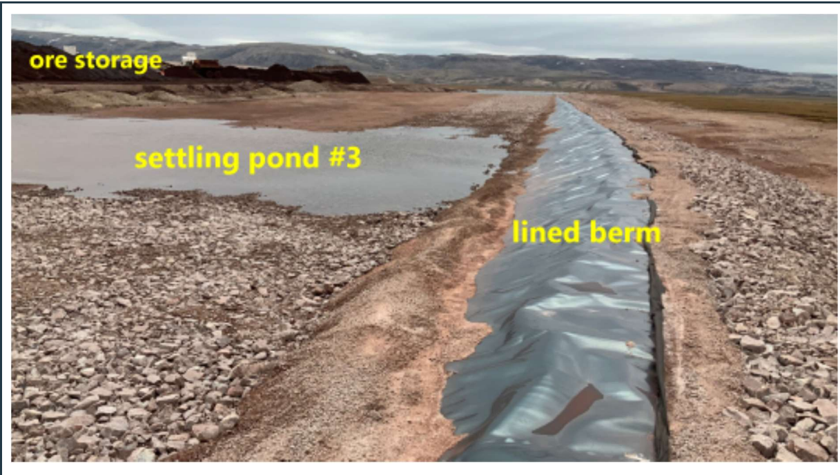
Figure 73: View of the lined, stable berm along the west side of settling pond #3.
