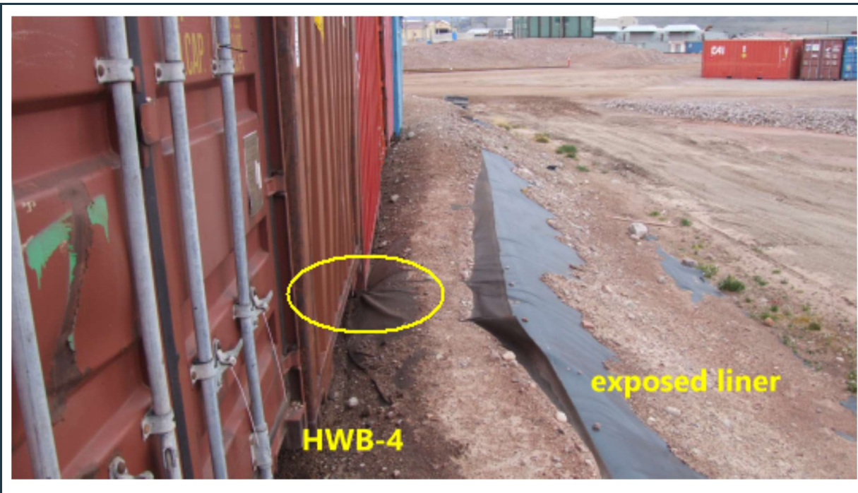
Figure 59: Exposed geotextile and liner at the HWB-4 cell, with location of potential damage to liner.
