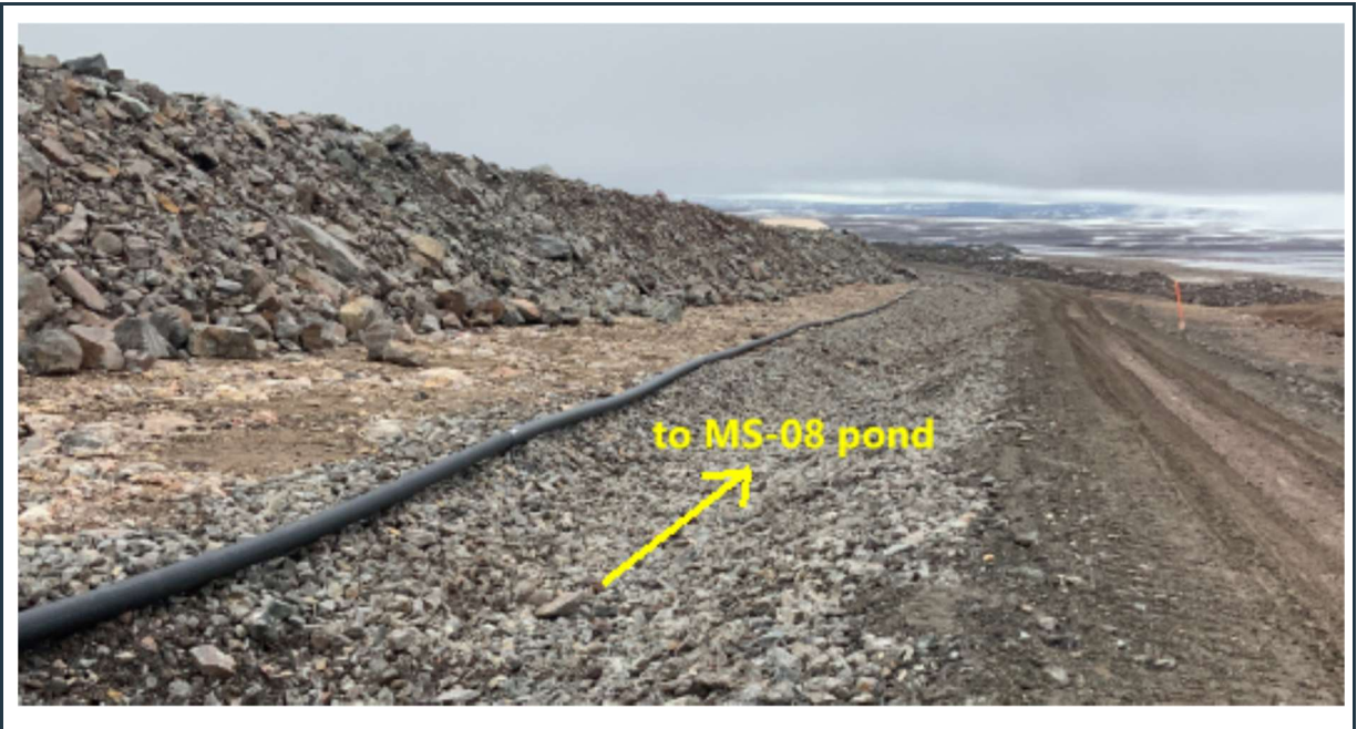
Figure 29: Well-maintained drainage ditch along the east side of the waste rock dump
