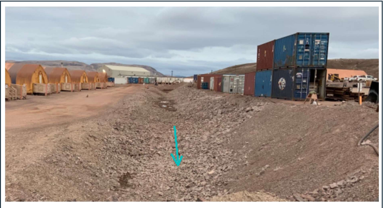
Figure 69: View of the east section of the 380 M surface water collection ditch, in good condition.
