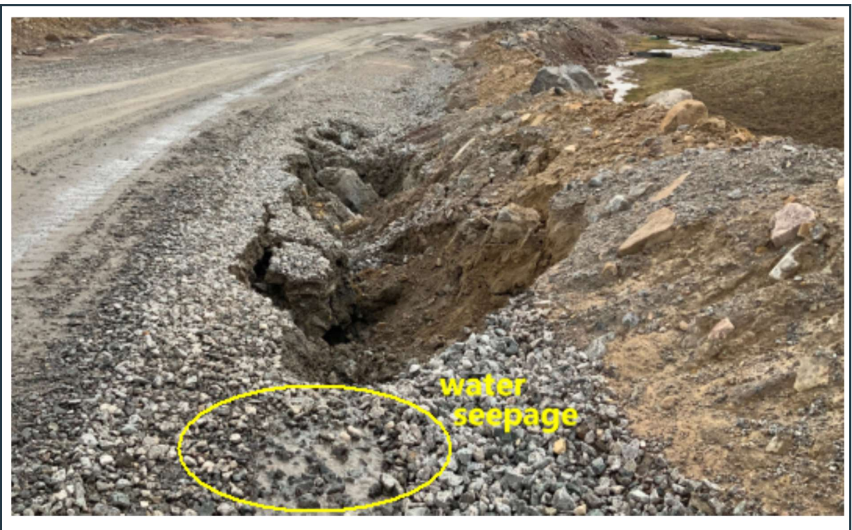
Figure 48: Surface water flowing from the quarry area along the road resulted in a failure of the edge of the access road leading to the quarry. Immediate repair was requested to prevent accidents.
