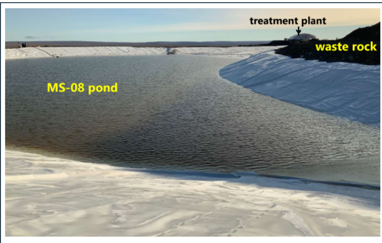
Figure 24: View of the robust, stable berm around the MS-08 pond with shallow slopes and intact liner.
