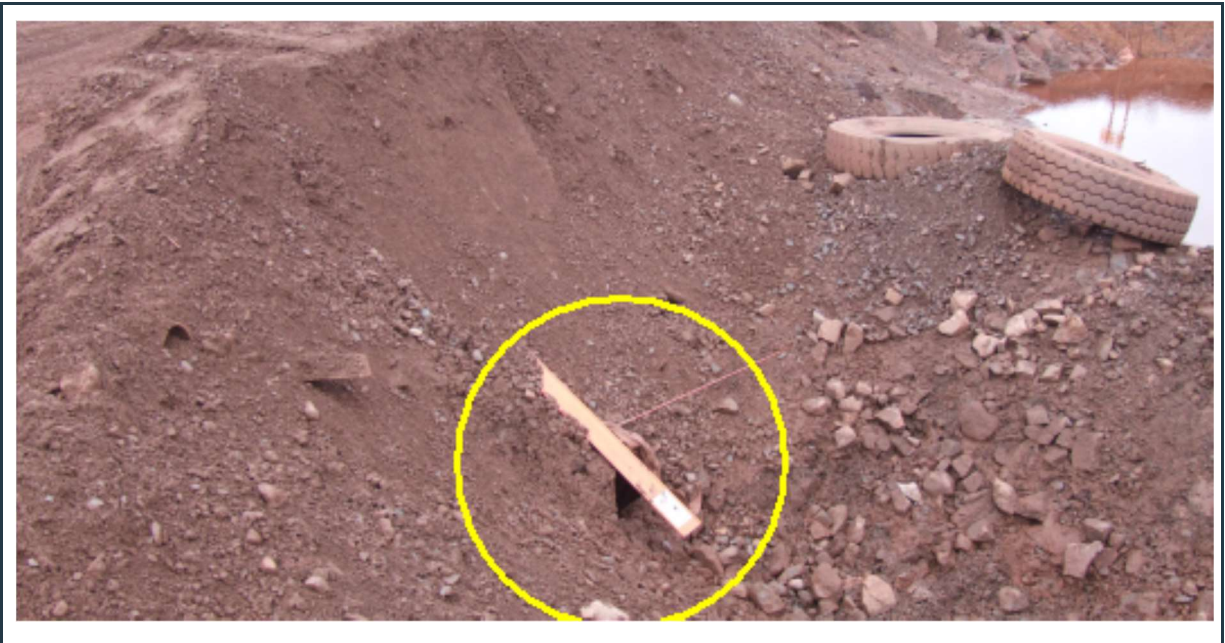
Figure 25: Partially clogged inlet of a culvert, located under the access road next to the truck weighing scale. It drains surface-water from the crusher area to the MS-06 pond.
