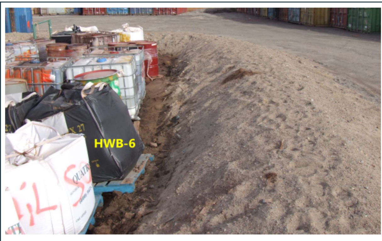
Figure 18: View of the recently upgraded stable berm around HWB-6.
