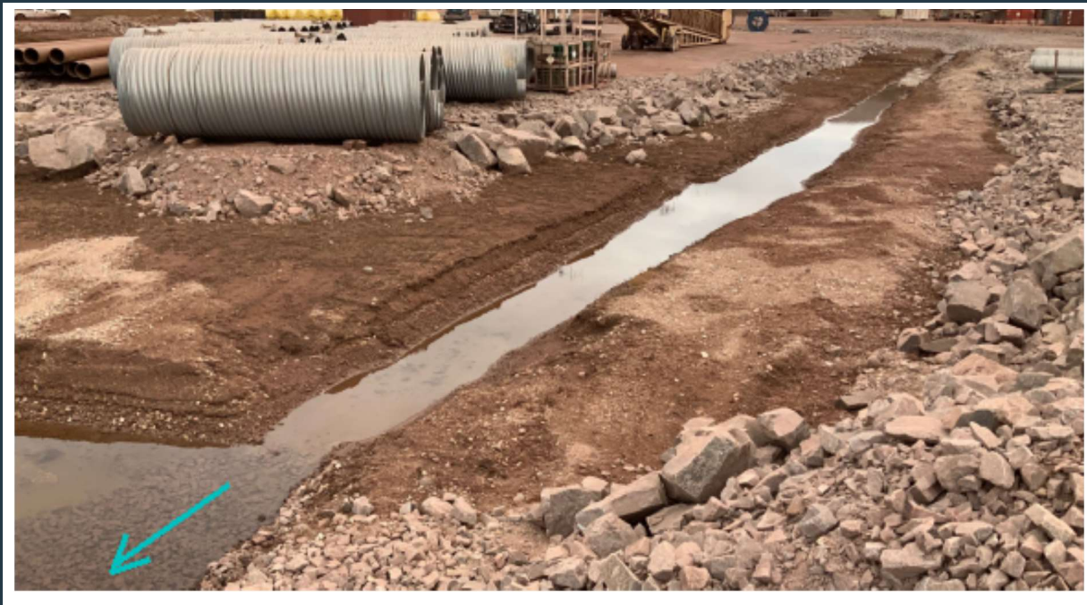
Figure 67: View of the W3/W14 surface water collection ditch.
