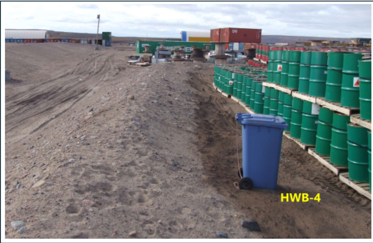
Figure 16: View of stable berms at HWB-4 next to HWB-3, with jet-fuel barrels stored on wooden pallets.
