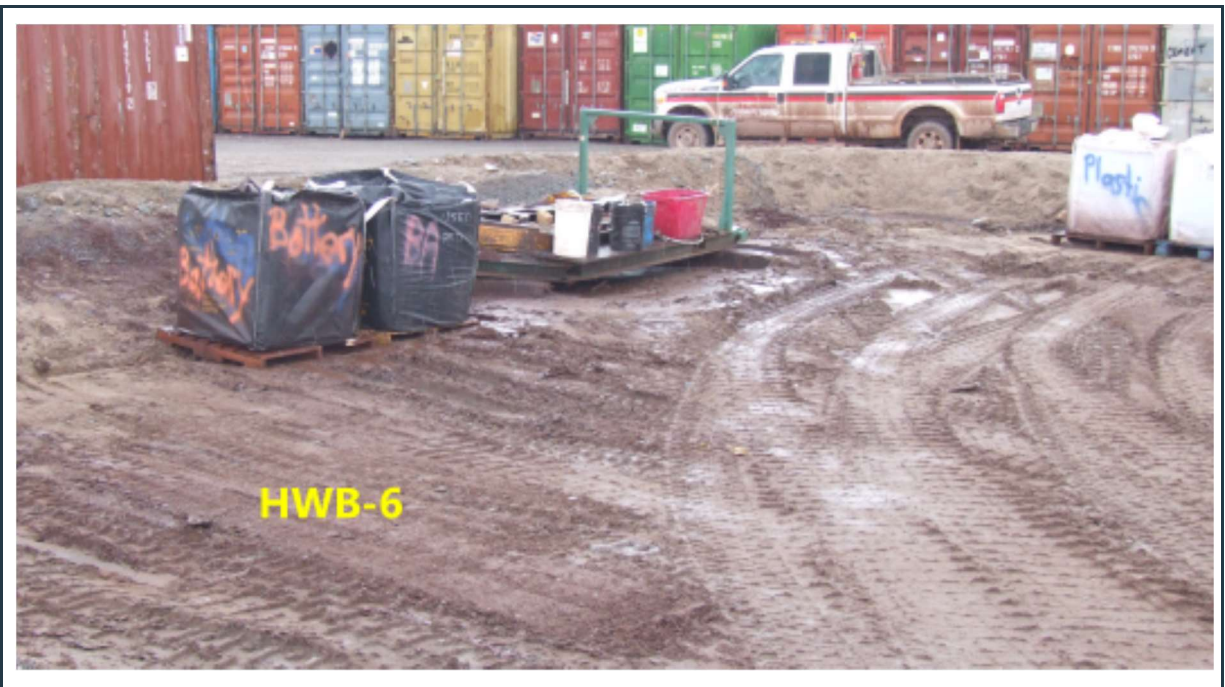
Figure 18: View of HWB-6. Note the well maintained “floor” (protecting the liner) within the cell.
