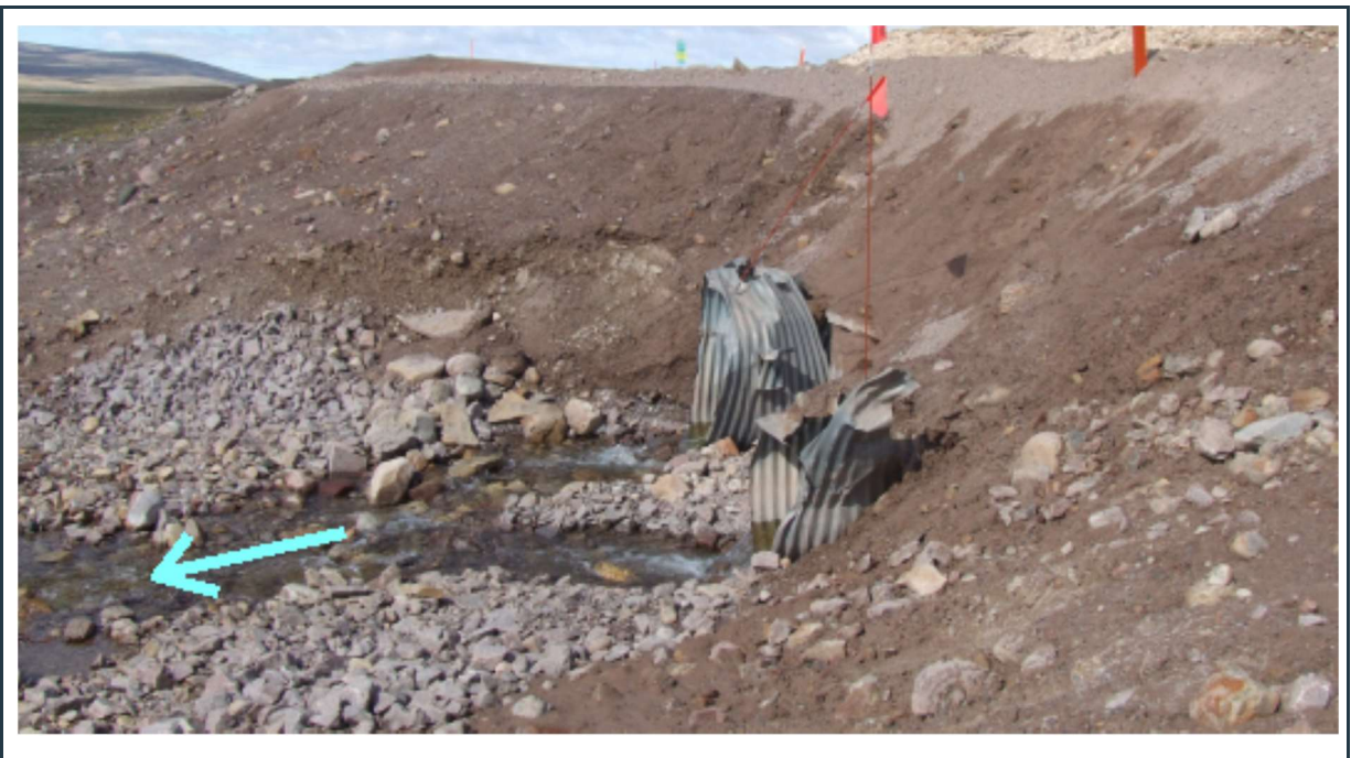
Figure 116: View of culvert(s) 114D (somewhat damaged outlet). Repair of both pipe ends required.
