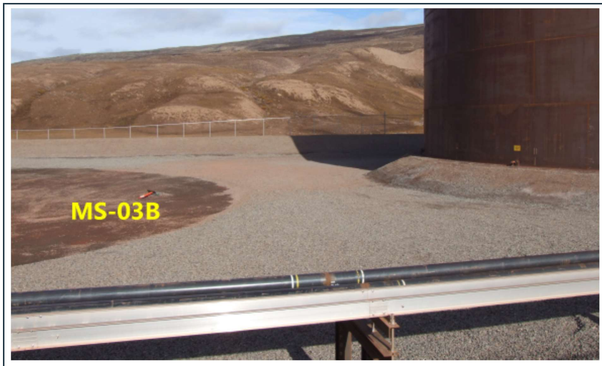
Figure 32: View of the recently completed fuel tank farm with well-constructed stable perimeter berms.
