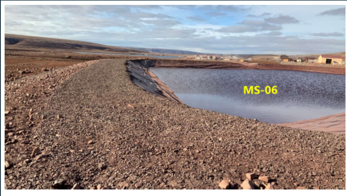
Figure 21: MS-06 surface-water collection pond with robust, stable berms and intact liner.
