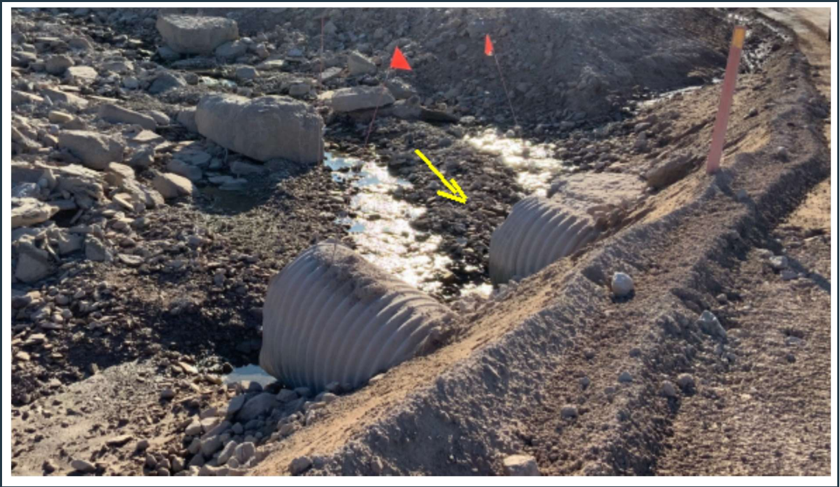
Figure 87: View of culvert(s) 094 inlet, in good condition (looking south).
