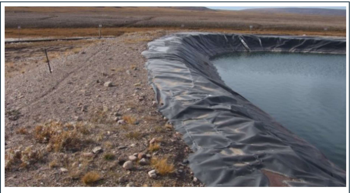
Figure 10: PWS pond #1. Well maintained stable perimeter berm and liner.
