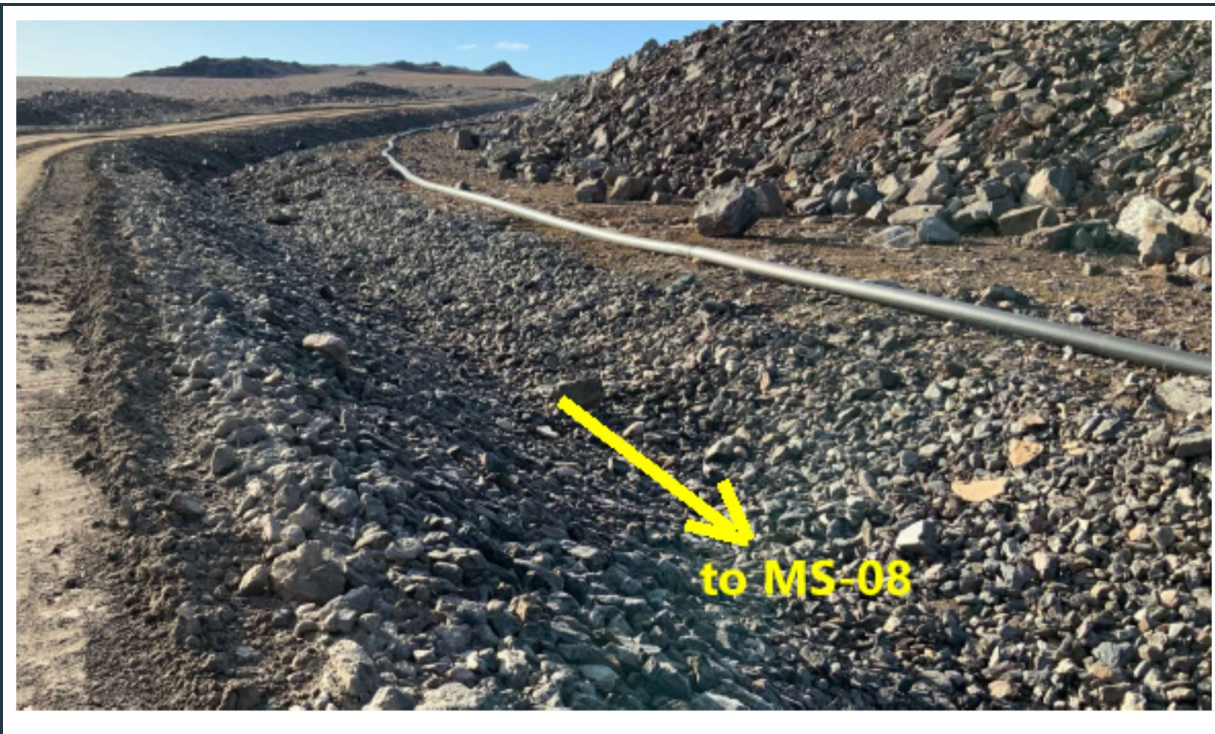
Figure 25: Well-maintained drainage ditch around the east side of the waste rock facility.
