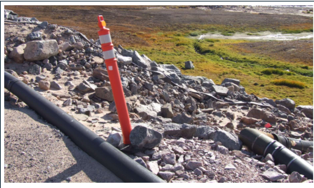
Figure 35: Minor slope erosion (cobbles and boulders rolling down the slope) at the water discharge area.
