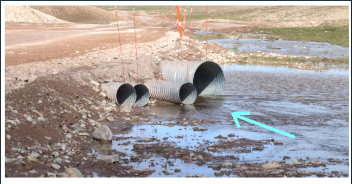
Figure 105: View of culvert(s) 102 (inlet) in good conditions.
