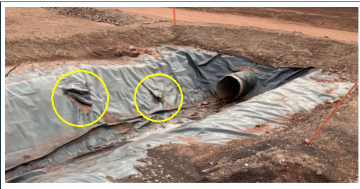
Figure 54: Some liner damage on the slope of the southern intake channel to the MP-05 settling pond.
