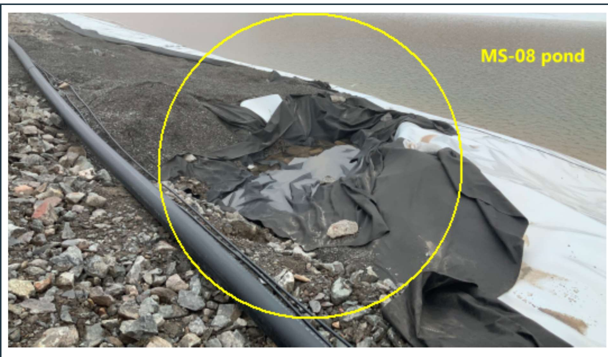
Figure 28: Area of minor fine-soil migration into the underlying rock fill at the northern section of the berm. The geotextile should be rearranged and the hole filled with fine crushed aggregate.
