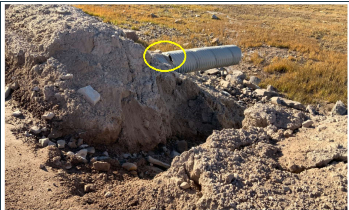
Figure 94: View of culvert 110A outlet (looking south-west). Note the minor damage on the top of the pipe (yellow circle), and the recent erosion of the road embankment adjacent to the culvert.
