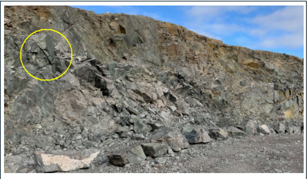
Figure 38: Stable rock face with some minor potential hazards (weak dike, loose boulders and sliding rock wedges). Boulders placed along the toe of the "rock face" block access to the slope.
