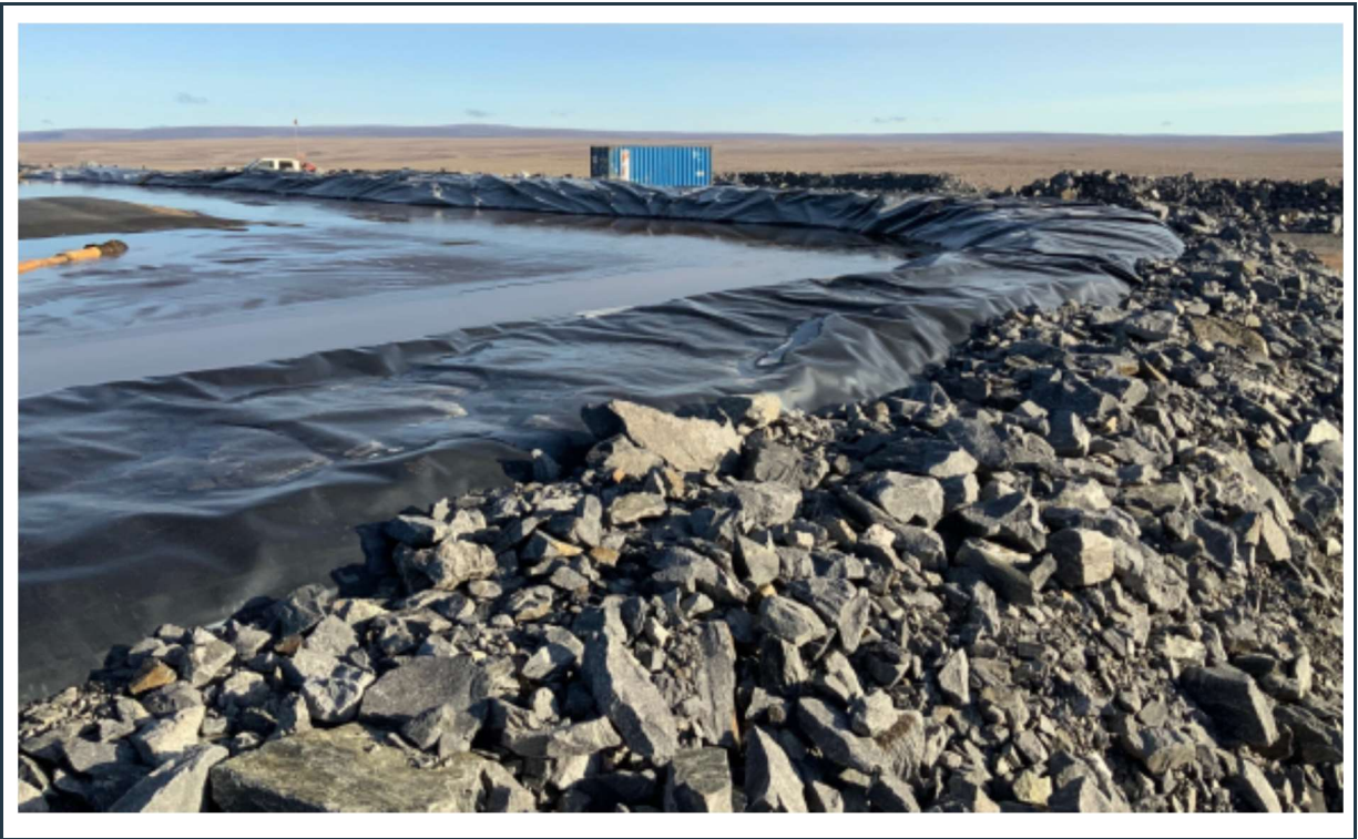
Figure 27: Stable rock fill berm at the water treatment pond adjacent to the waste rock facility.
