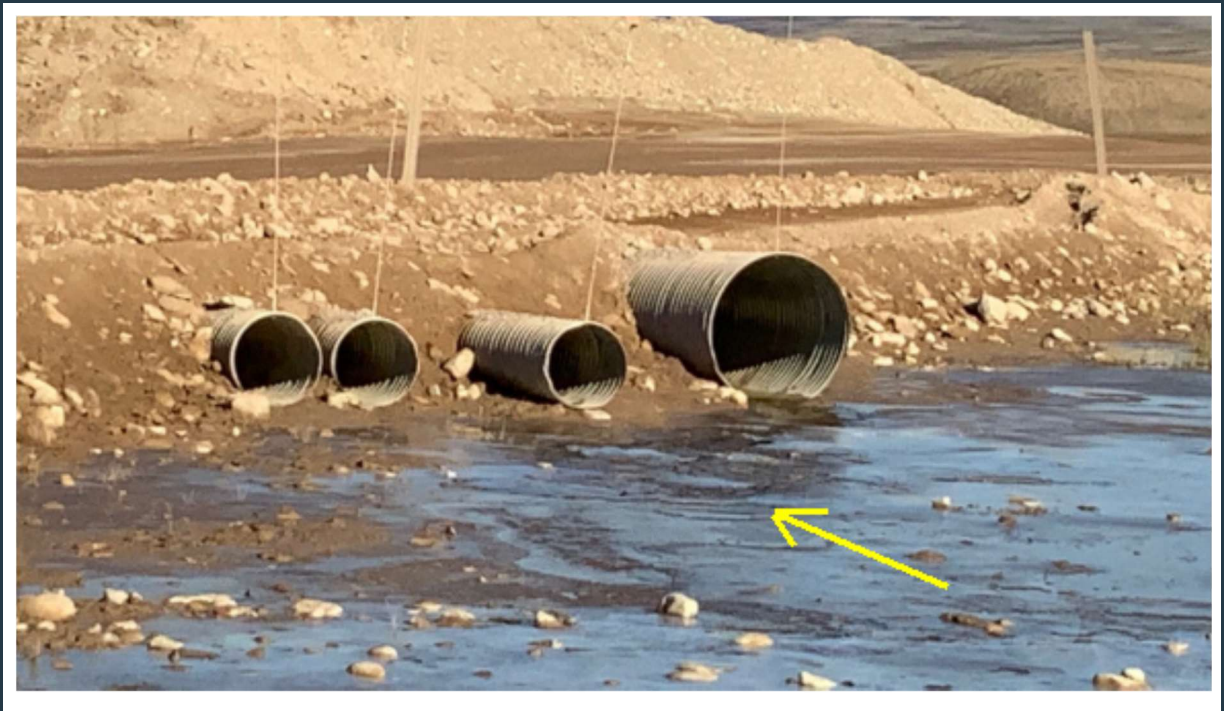
Figure 89: View of culvert(s) 102 inlets in good condition (looking west).
