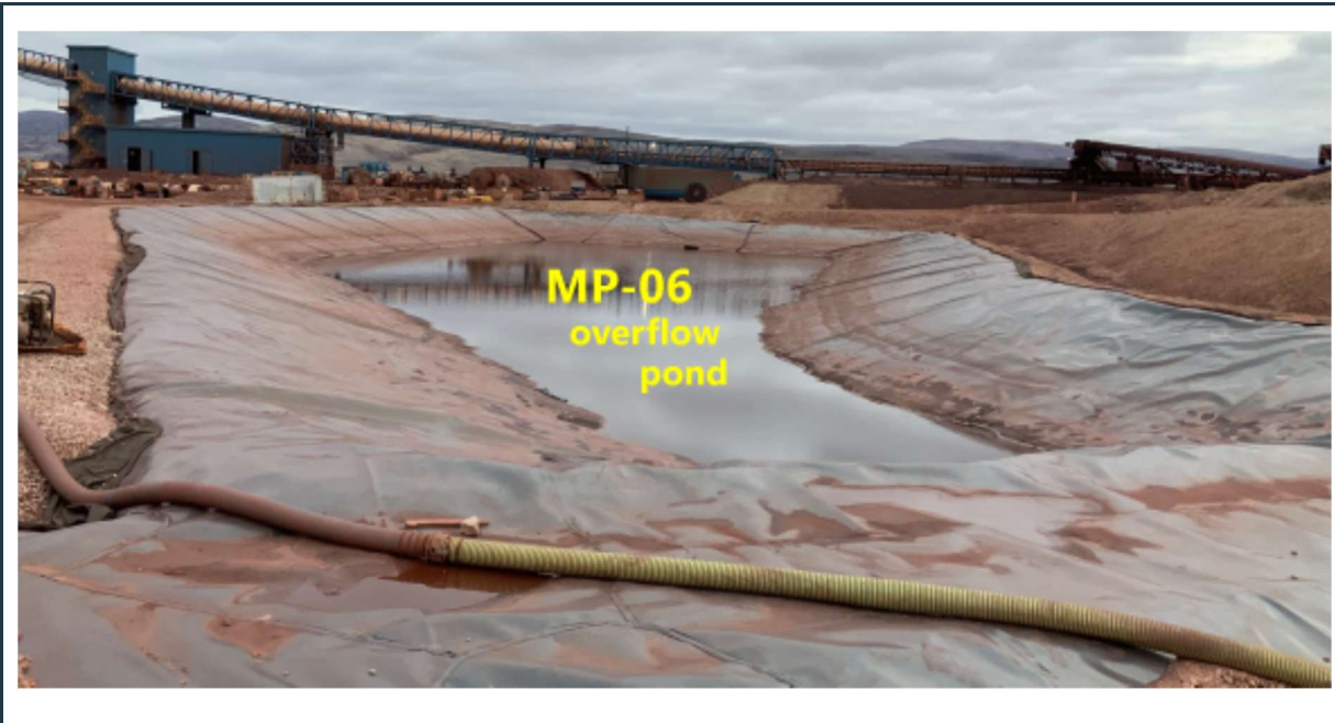
Figure 57: View of the lined MP-06 overflow pond, with stable berms.
