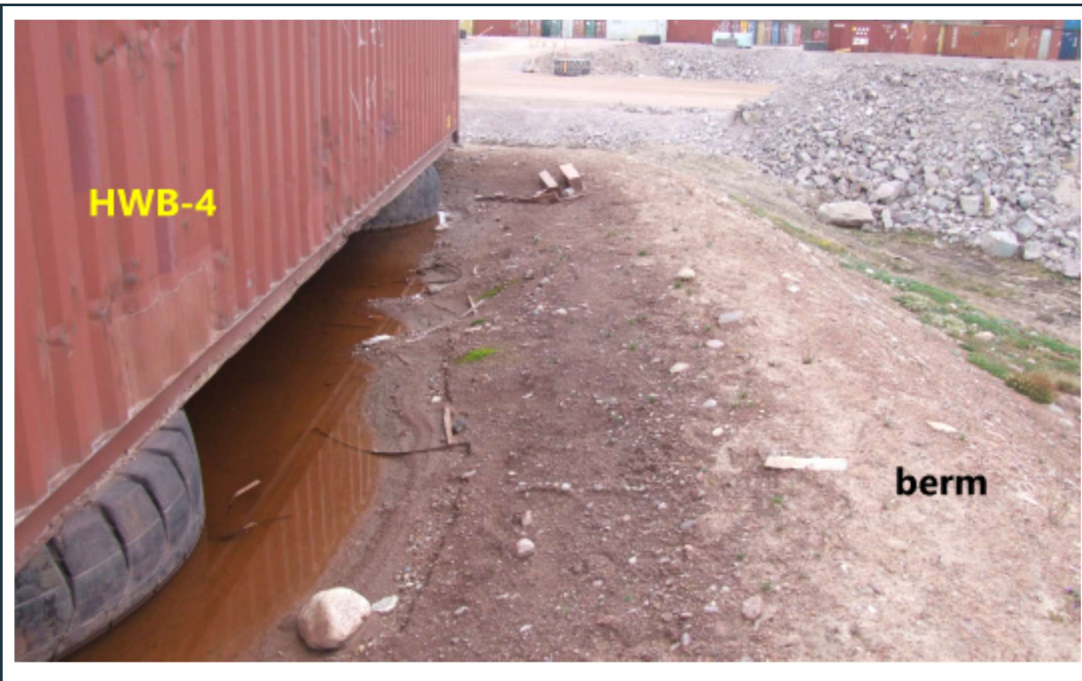
Figure 57: Stable berm around, and ponding water within the HWB-4 cell.
