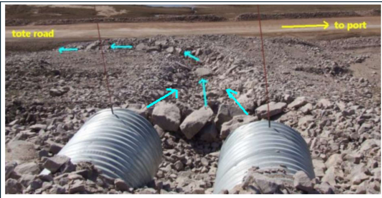
Figure 86: Culverts and drainage ditch, conveying surface water from the P-SWD-6 "Q01 South" ditch toward the tote road.
