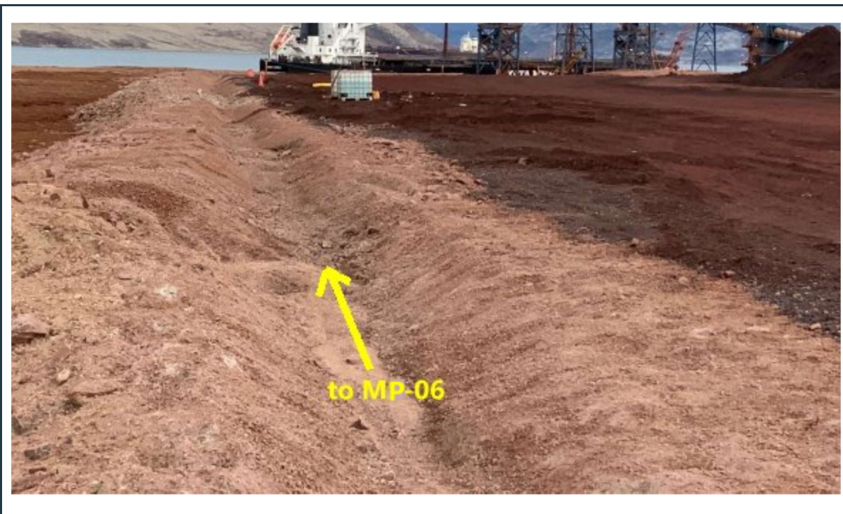
Figure 58: Surface water collection ditch adjacent (west) to the crushed ore storage area, draining to the MP-06 pond.
