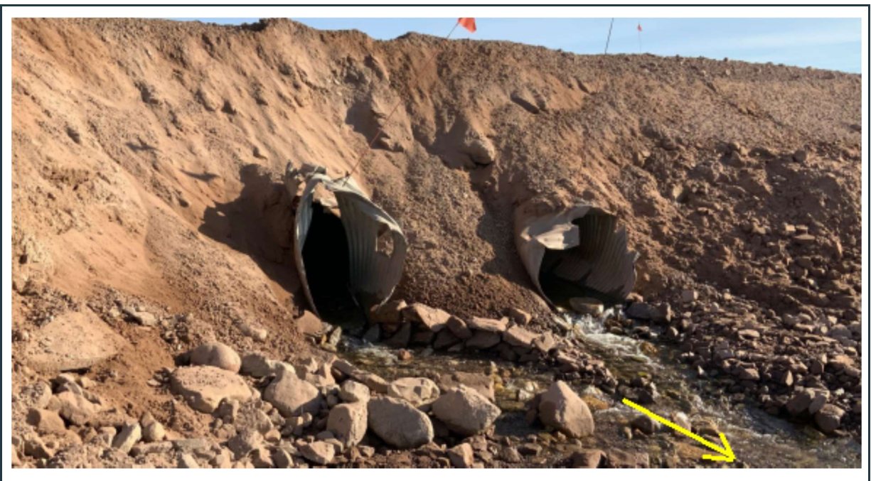
Figure 100: View of culvert(s) 114D damaged outlets (looking south-east). Repair of both pipe ends is required.
