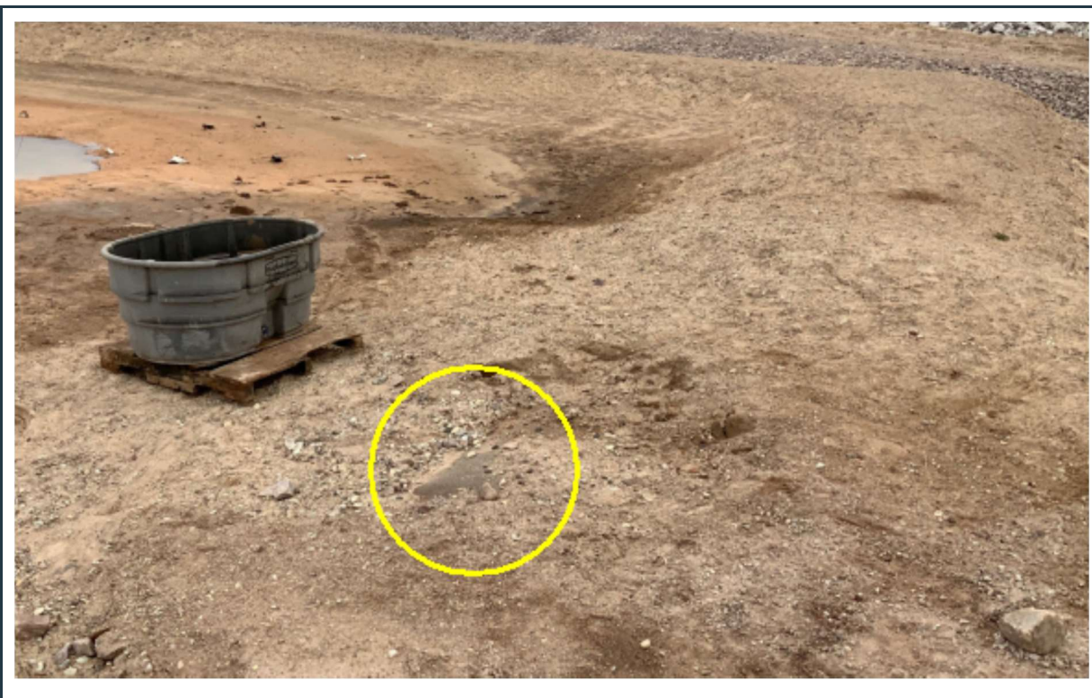
Figure 52: Condition of the ramp to the MP-04A snow dump, with exposed liner (yellow circle).
