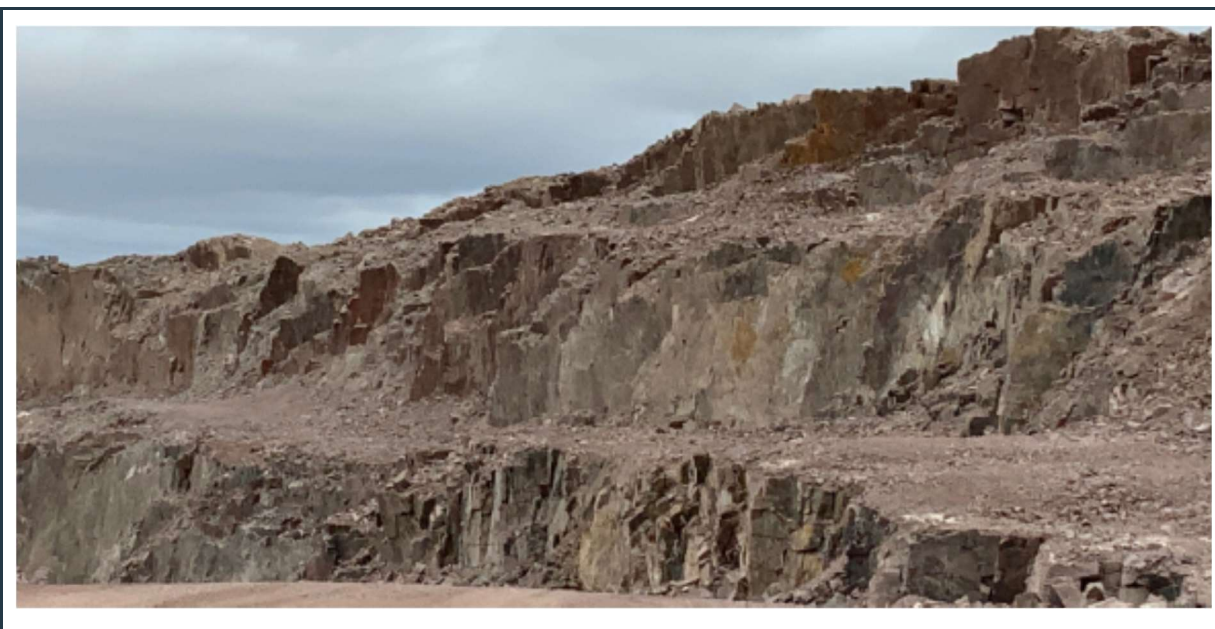
Figure 60: View of stable highwalls with minor weathering and bench erosion in the Q01 rock quarry.
