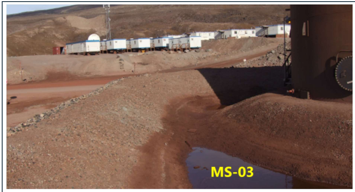
Figure 31: View of the well-maintained stable berm around the MS-03 diesel fuel farm.
