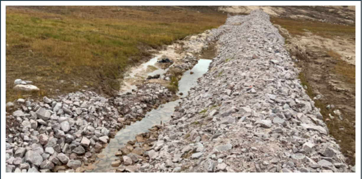
Figure 61: View of the “P-SWD-3 surface water collection ditch with failing side slope. The sloughing is caused by the uncontrolled water flow into the ditch along its alignment (see the next image).
