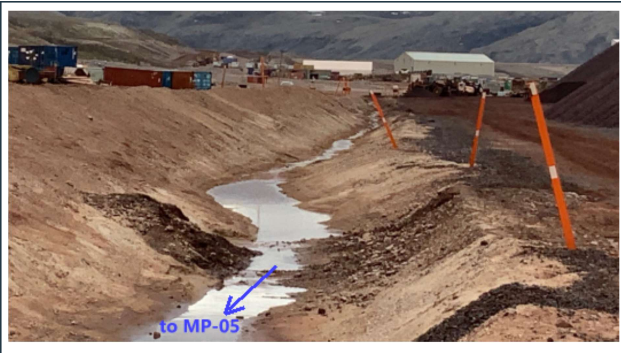
Figure 69: Surface water collection ditch adjacent to the crushed ore storage, draining to MP-05 pond.
