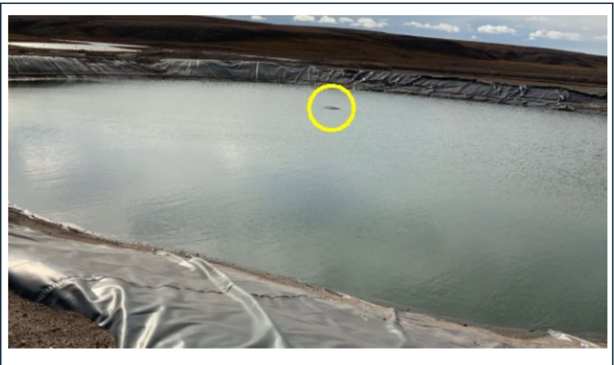
Figure 12: Stable perimeter berms at the PWS pond #3 – A small “floating” section of the liner is visible in the pond (yellow circle).
