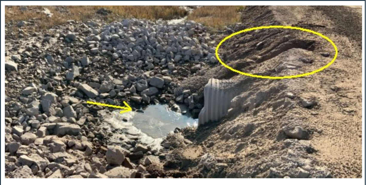
Figure 101: Culvert 202 inlet (looking south). Note the slope erosion at the edge of the road, adjacent to the culvert (yellow circle).
