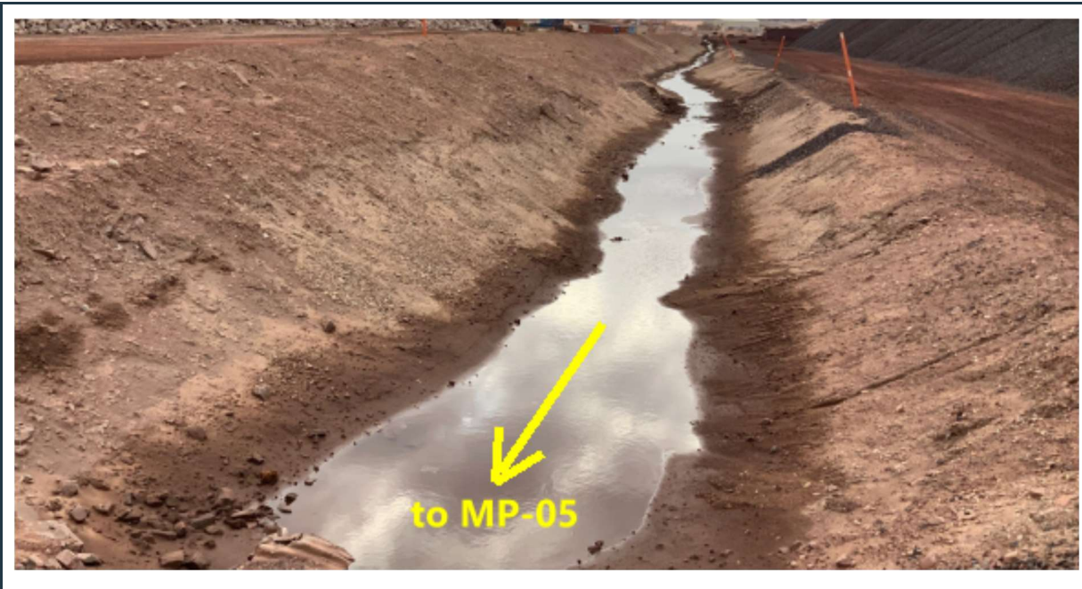
Figure 55: Surface water collection ditch adjacent to the crushed ore storage, draining to MP-05 pond.
