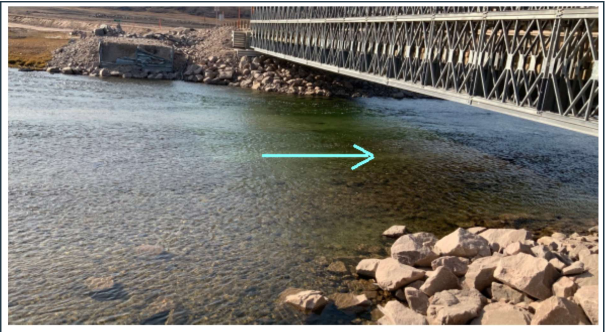
Figure 74: View of the south side of "bridge 17". Note the rip-rap scour protection at the abutments.
