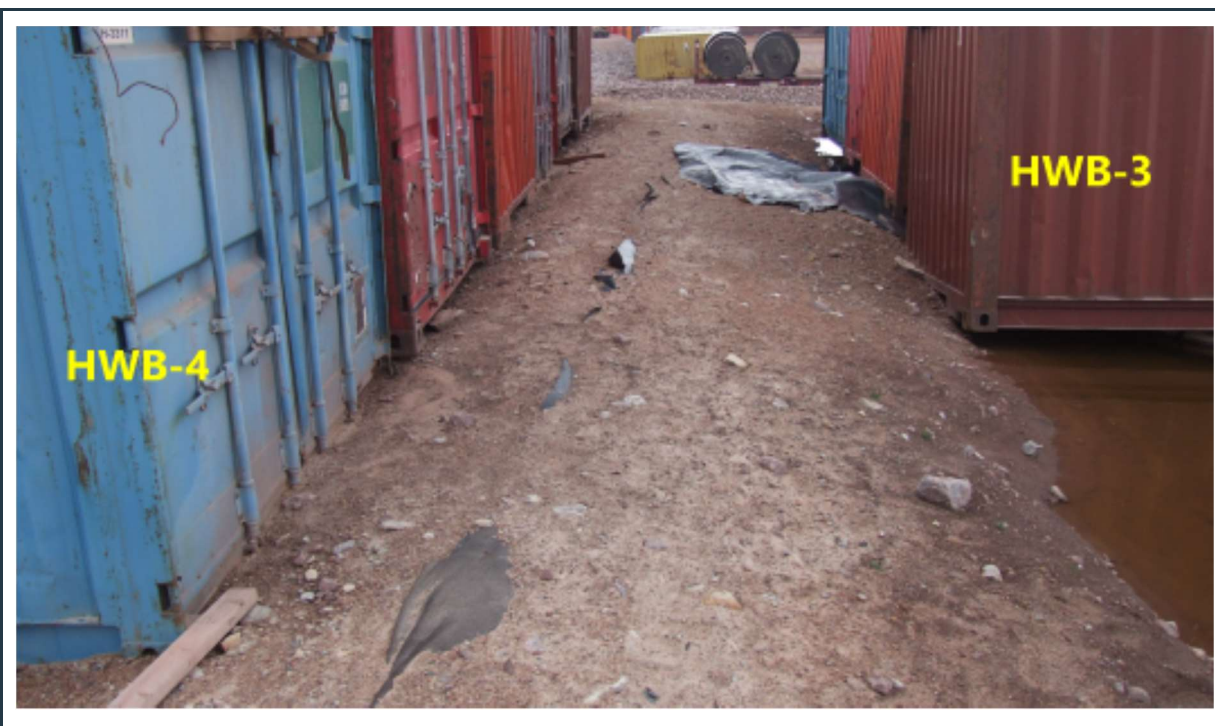
Figure 58: Exposed geotextile and liner on the internal berm between the HWB-3 and HWB-4 cells.
