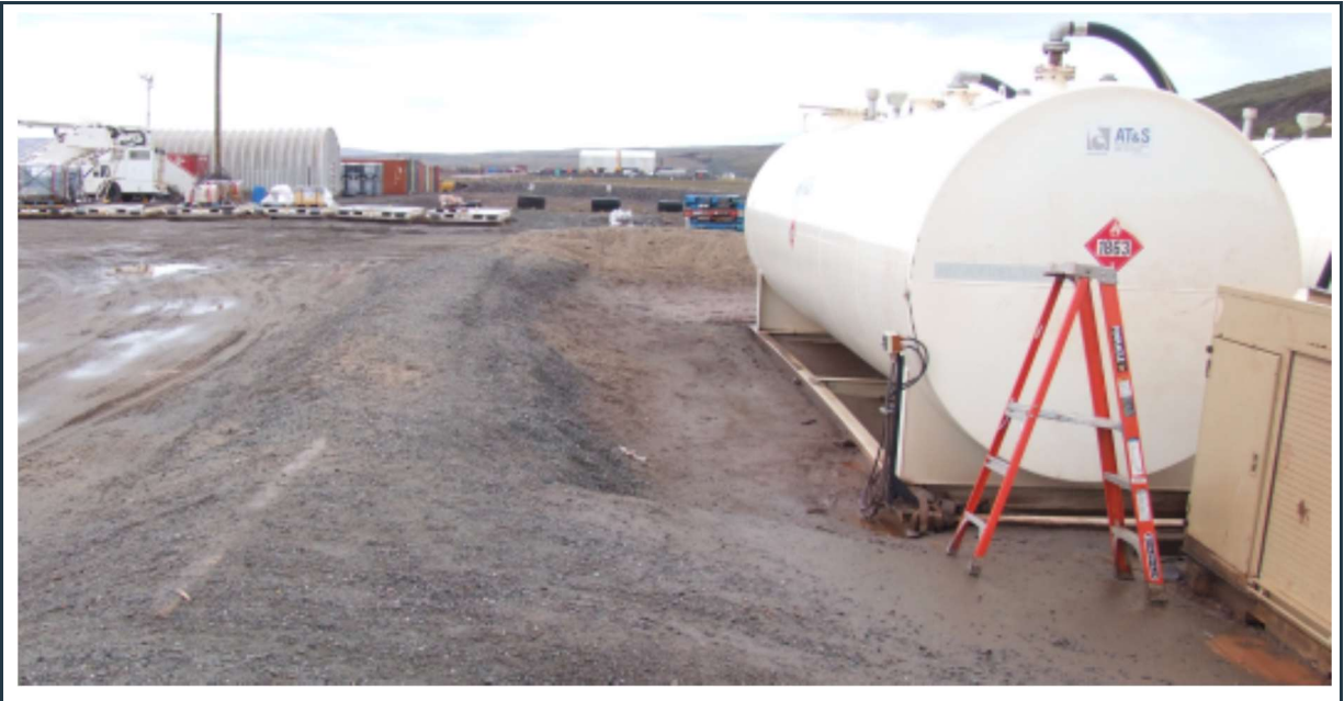
Figure 35: View of the well-maintained berm at the jetfuel storage cell.
