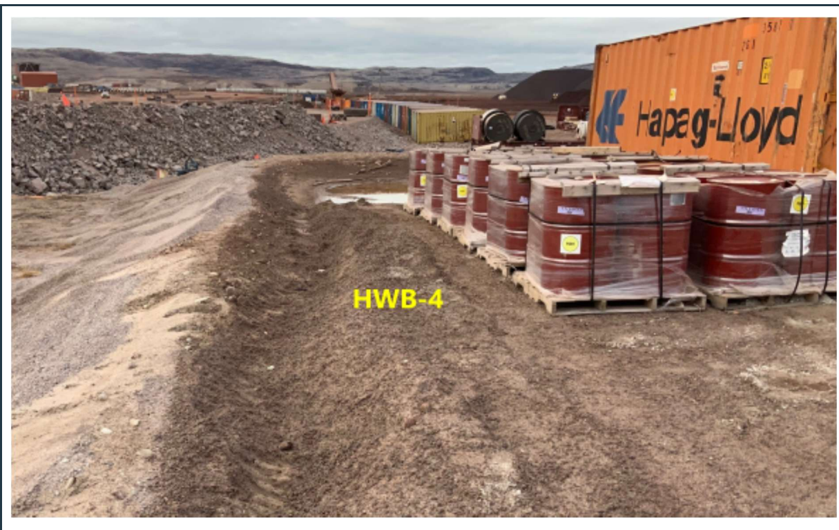
Figure 46: Upgraded stable berm and ponding water within the reconstructed HWB-4 cell.
