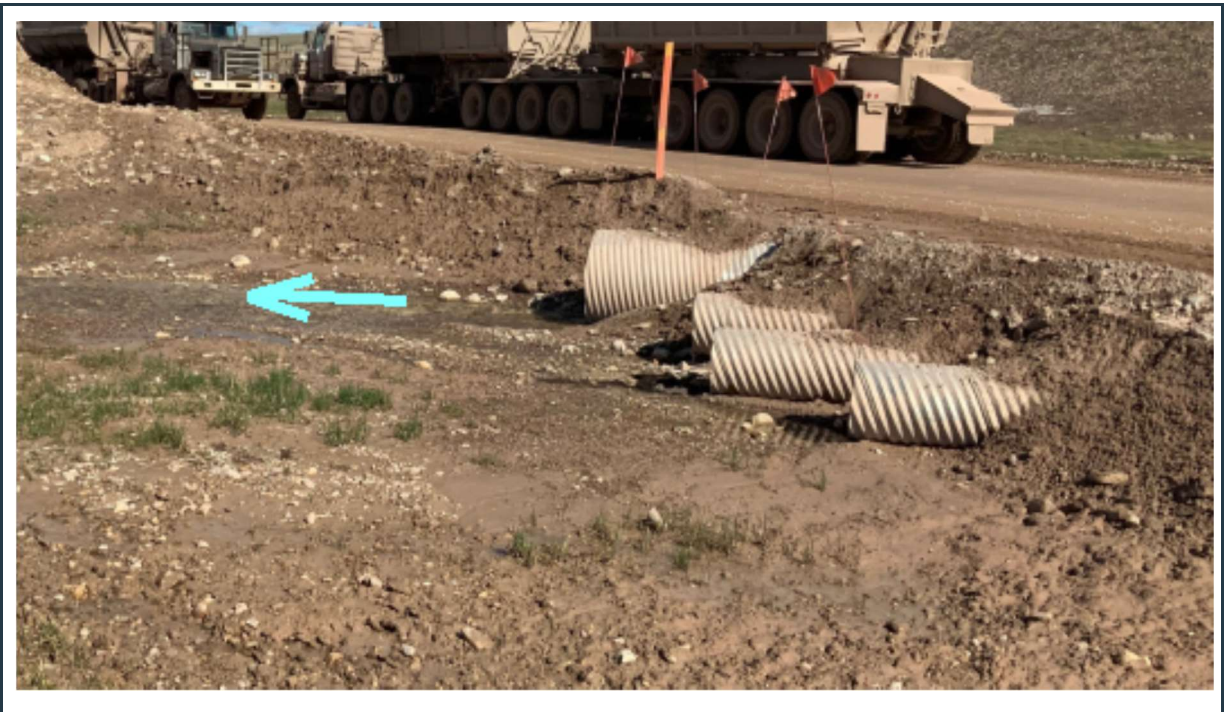
Figure 106: View of culvert(s) 102 (outlet) in good conditions.
