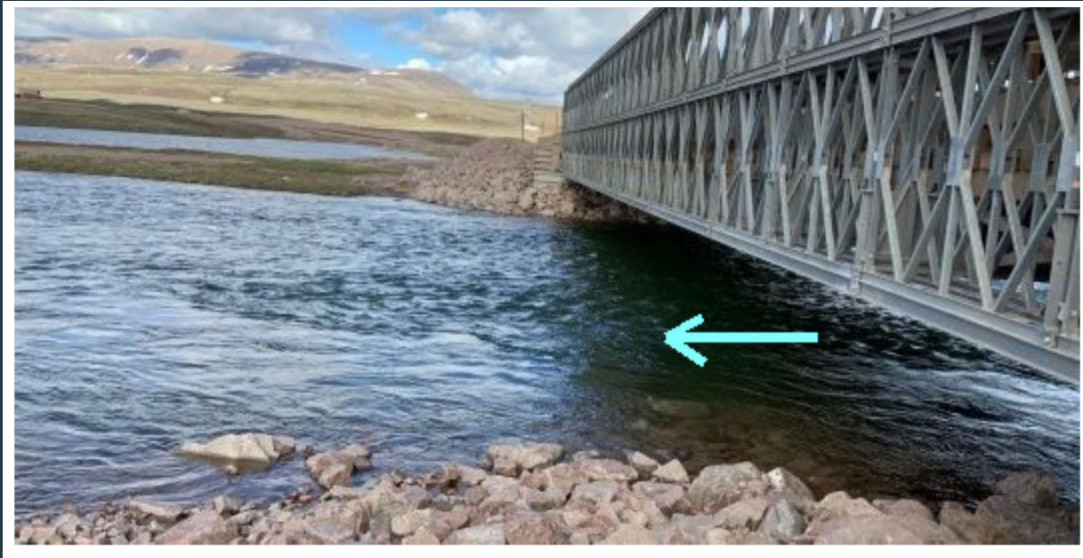
Figure 89: View of "bridge 17", looking north-east. Note the rip-rap scour protection.
