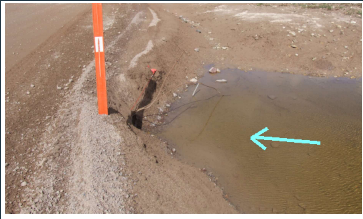
Figure 107: View of culvert 107 (inlet). Extension of the culvert and placement of riprap are required.
