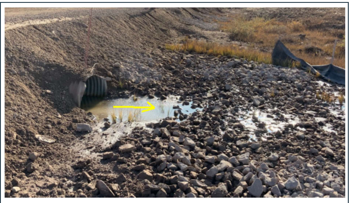
Figure 102: View of culvert 202 outlet (looking south). Flow of water is blocked by the crushed rock fill.
