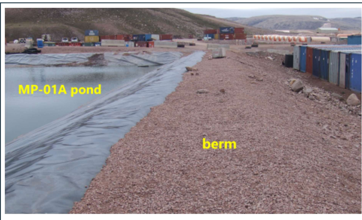
Figure 60: Berms in excellent condition with stable slopes around the MP-01A pond.
