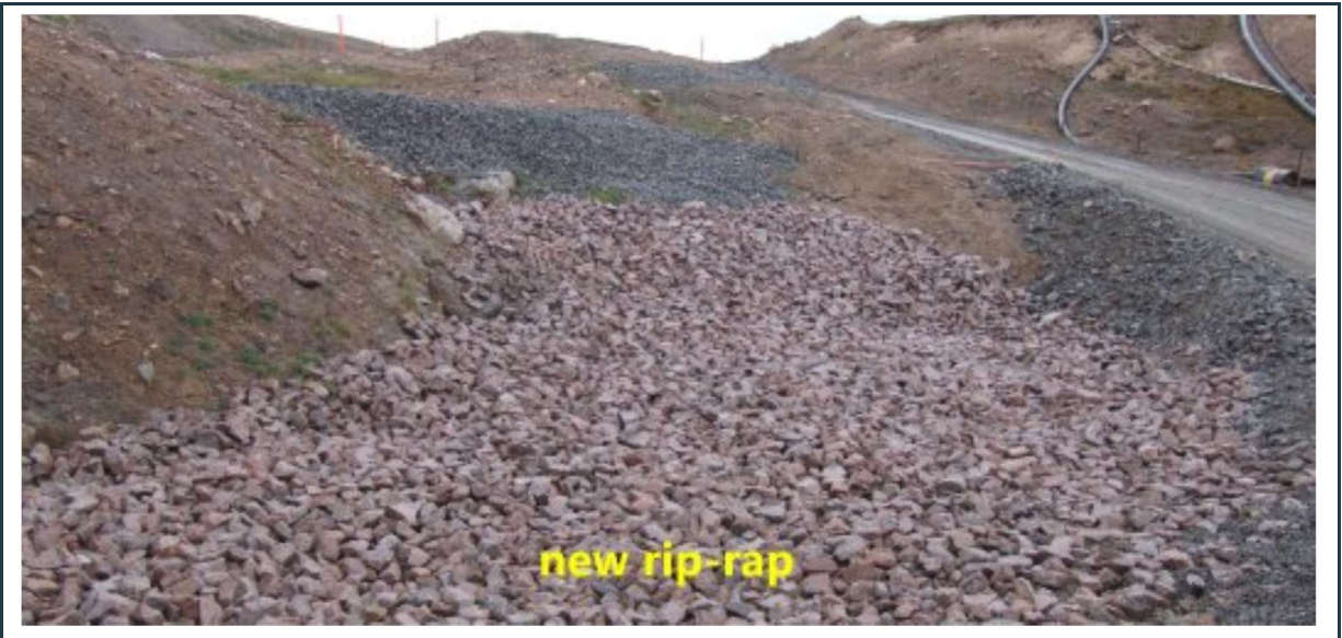
Figure 41: Recently placed rip-rap in one of the cells to prevent erosion of the channel floor at the critical vertical drop in elevation along the chain of sedimentation cells.
