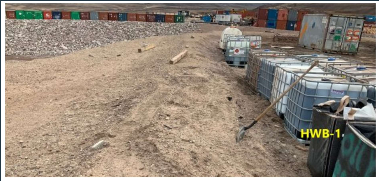
Figure 43: View of the, stable berm around the HWB-1 cell.
