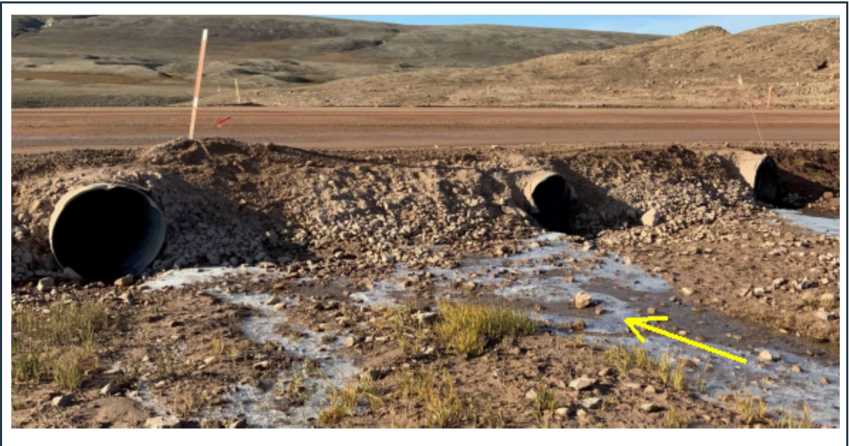
Figure 97: View of culvert(s) 112D inlets (looking west). Thin ice was already visible in the creek during the first week of September.
