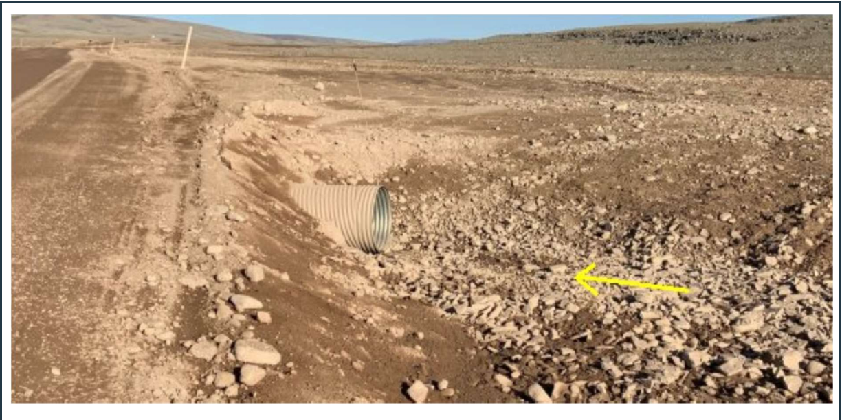
Figure 85: View of culvert 083 inlet (looking north). No flow was noted at the time of the inspection.
