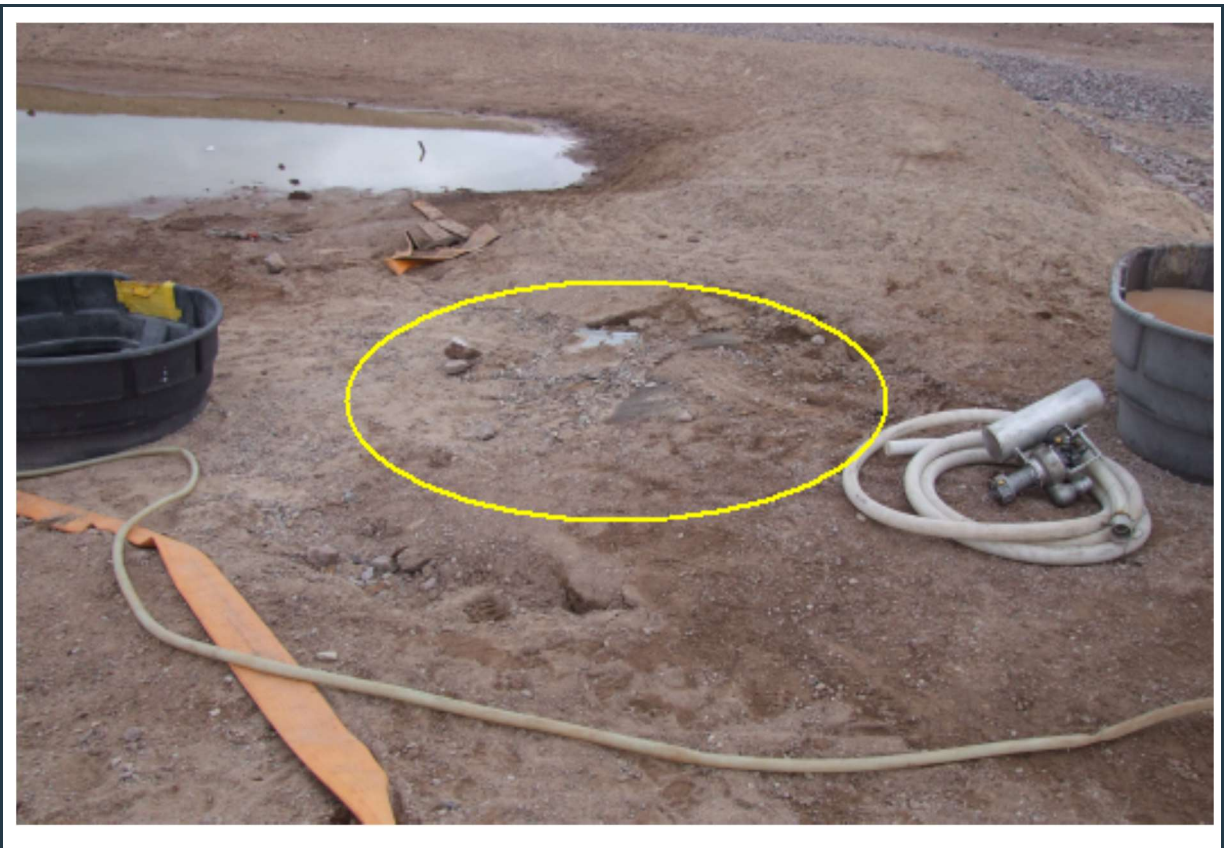
Figure 66: Condition of the ramp to the MP-04A snow dump, with exposed liner (yellow circle).
