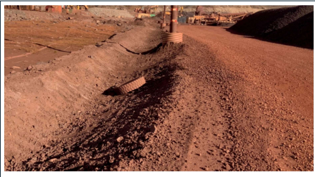
Figure 22: Well maintained surface-water collection ditch next to the crusher plant, leading to MS-06.
