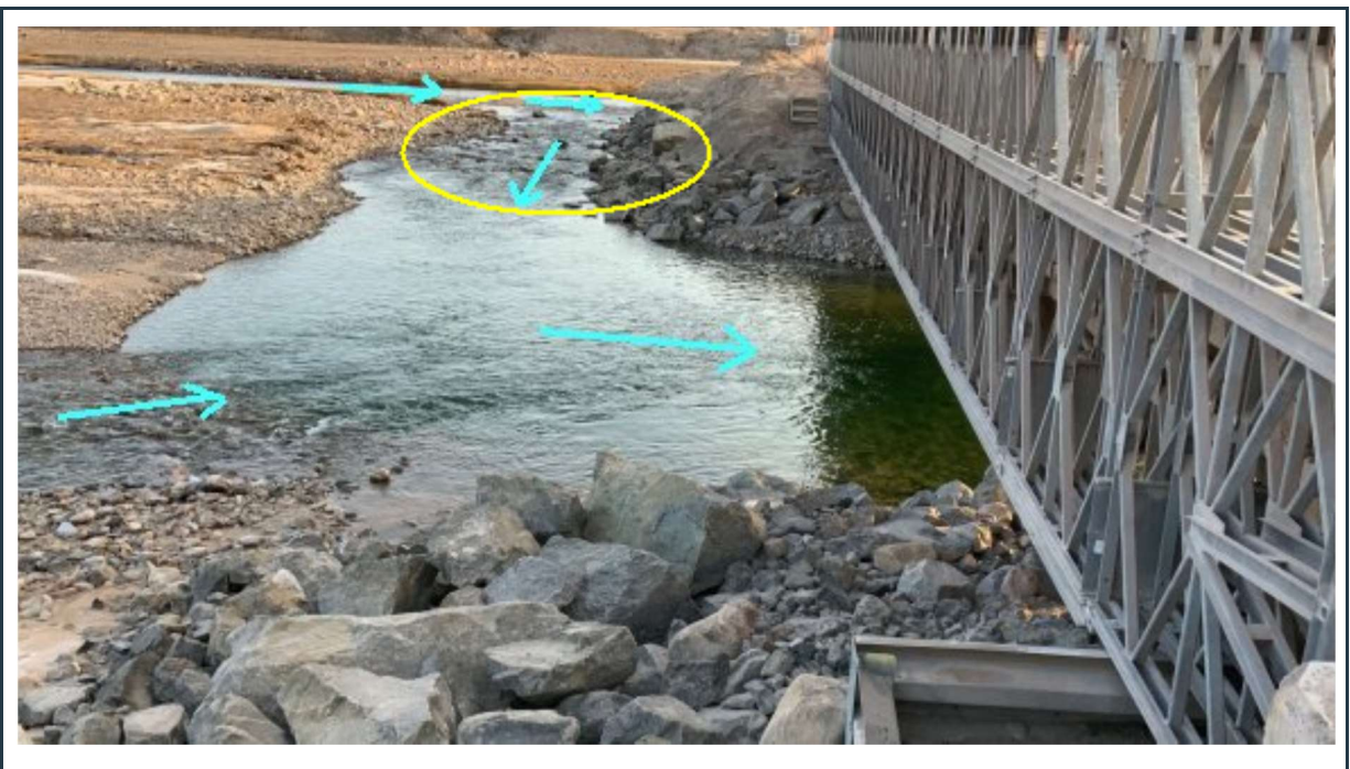
Figure 80: View of two abutments and the east side of bridge 97. Note the flow of water at the toe of the south abutment between the side-culverts and the bridge (yellow circle and also in Figure 8).
