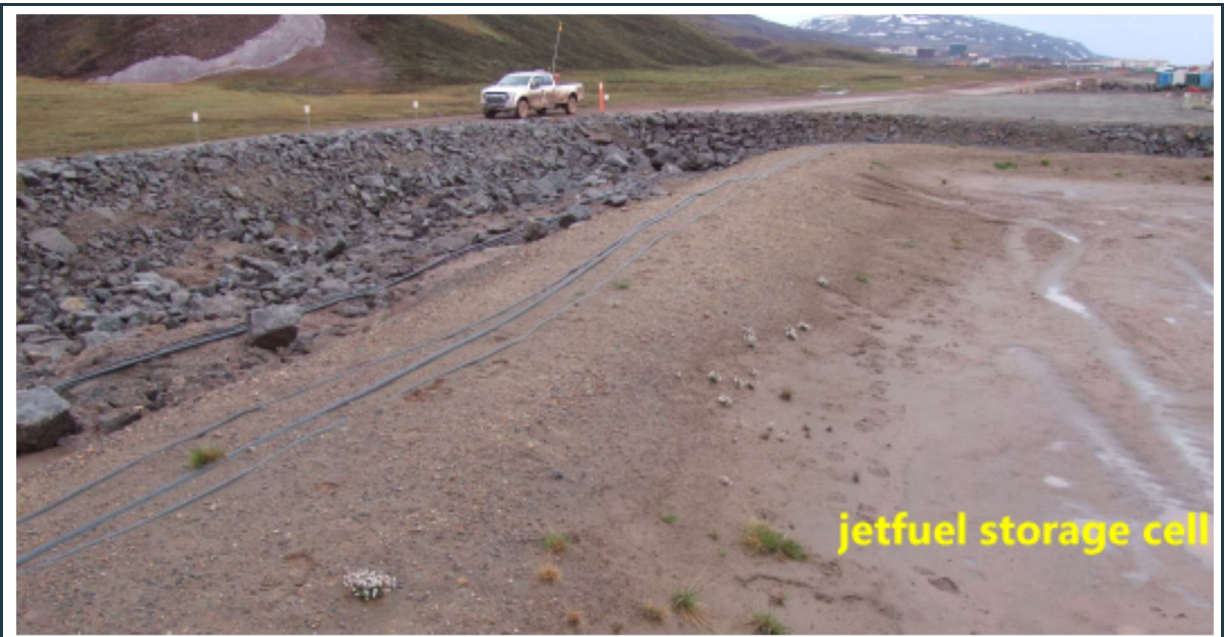
Figure 36: View of the jetfuel farm's double berm system (note the additional crushed rock berm between the cell's perimeter berm and the tote road/parking lot).
