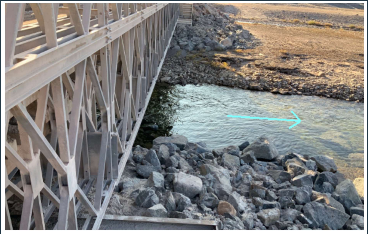
Figure 75: View of the west side of bridge 63, looking south. Note the low flow and stable abutments.
