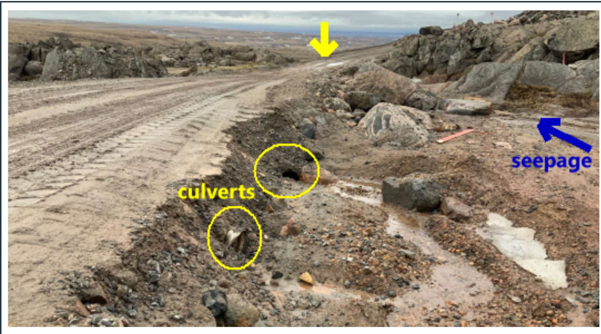
Figure 51: Existing culverts installed at the wrong place (yellow circles). New culvert required at the yellow arrow to prevent serious road problems in the future. Blue arrow indicates below grade seepage.
