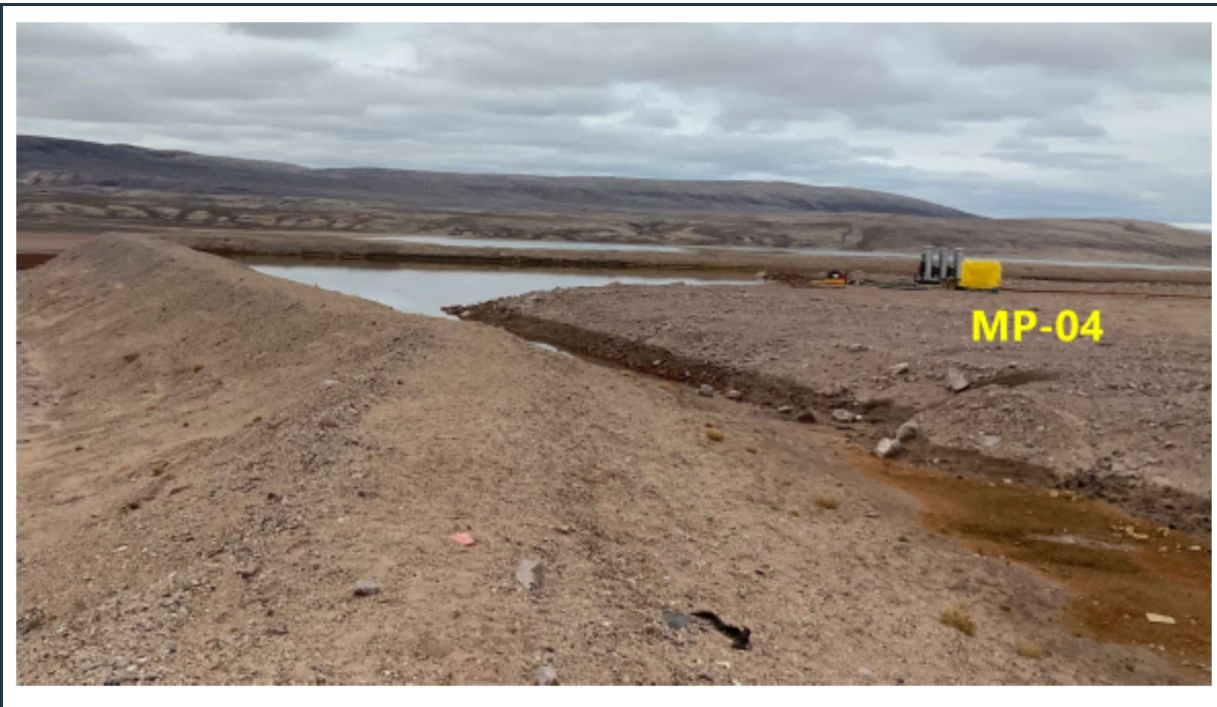
Figure 50: View of stable berm at the MP-04 landfarm, with covered waste and ponding water within the cell.
