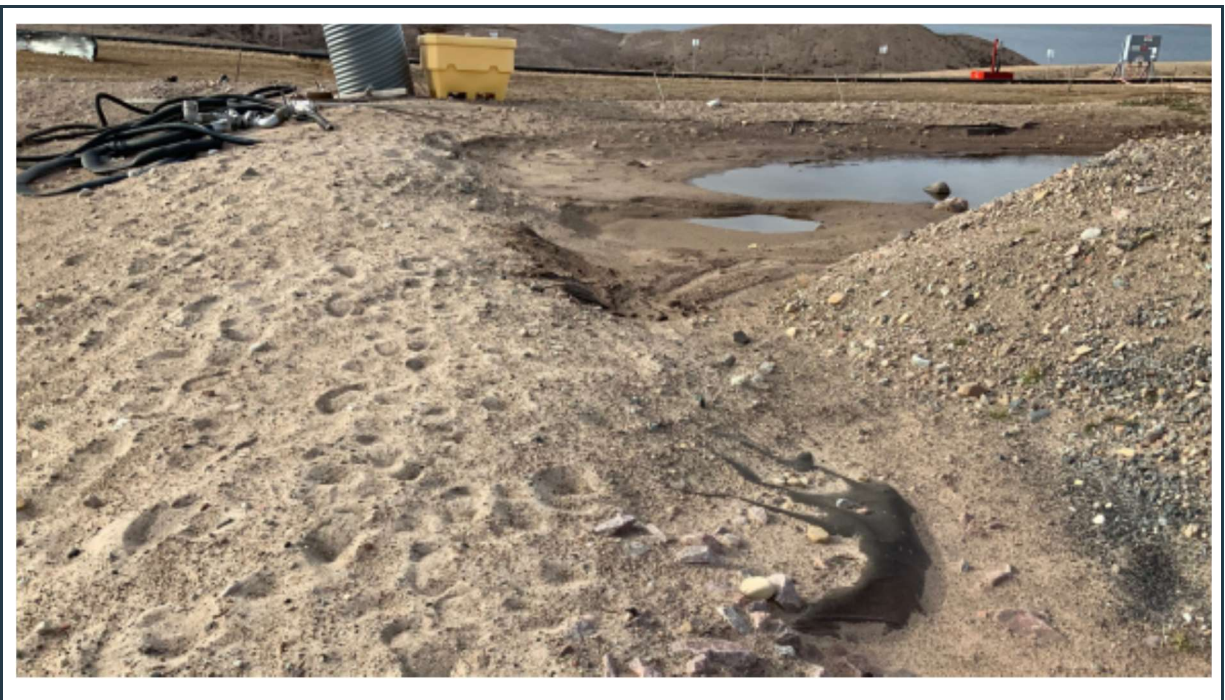
Figure 28: View of the generator fuel berm with exposed geotextile at a few locations.
