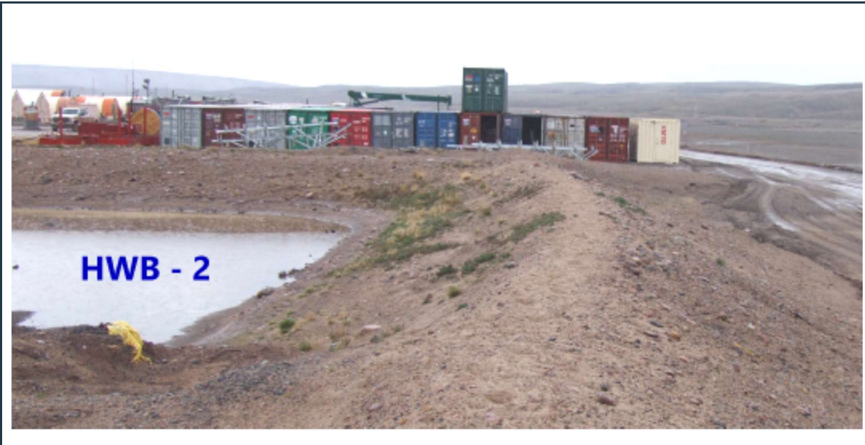
Figure 13: View of the stable berm at HWB-2. Other than some plastic, the cell is currently empty.
