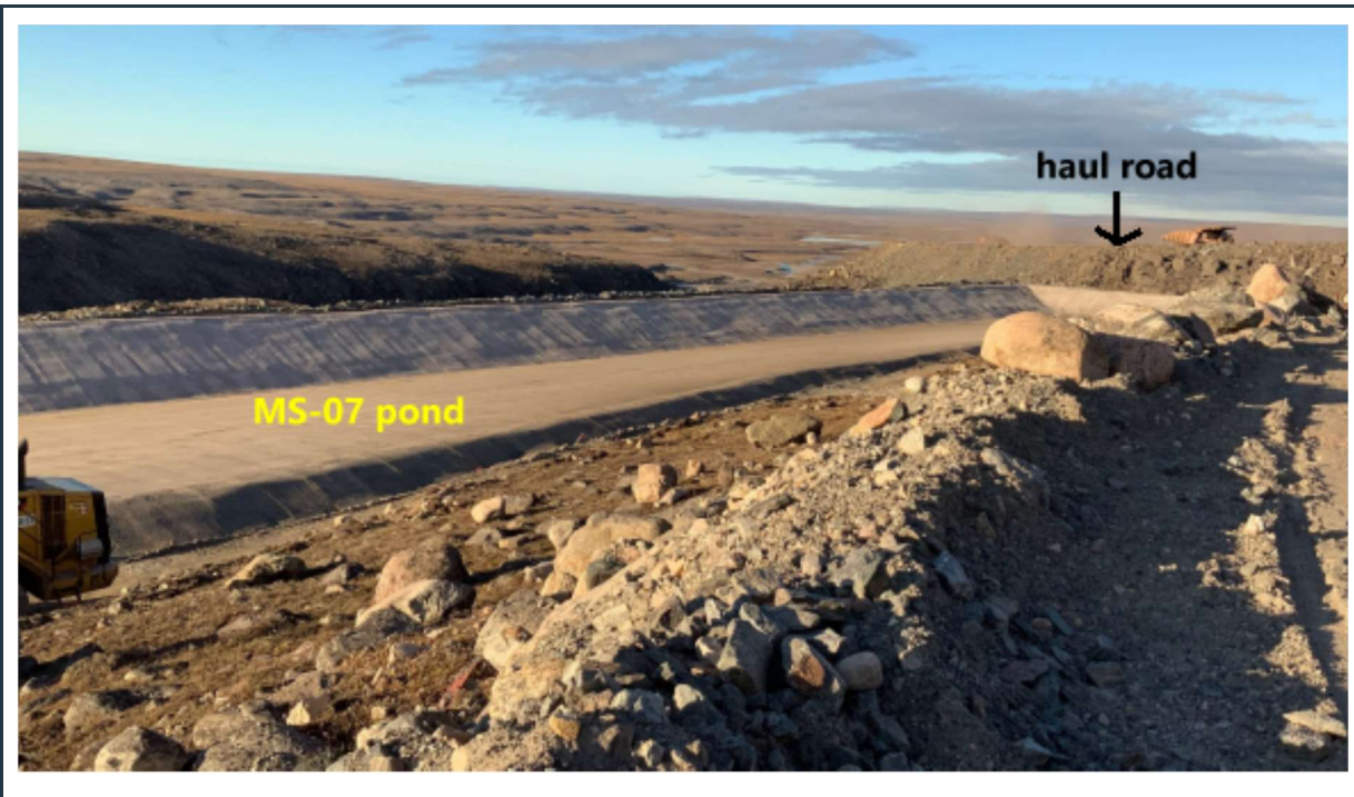
Figure 41: Construction of the MS-07 pond is in progress south of the proposed ore stockpile area.
