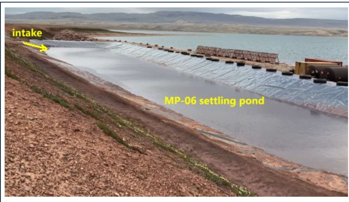
Figure 70: View of the lined MP-06 pond with stable berms (north-west corner of the ore stockpile).
