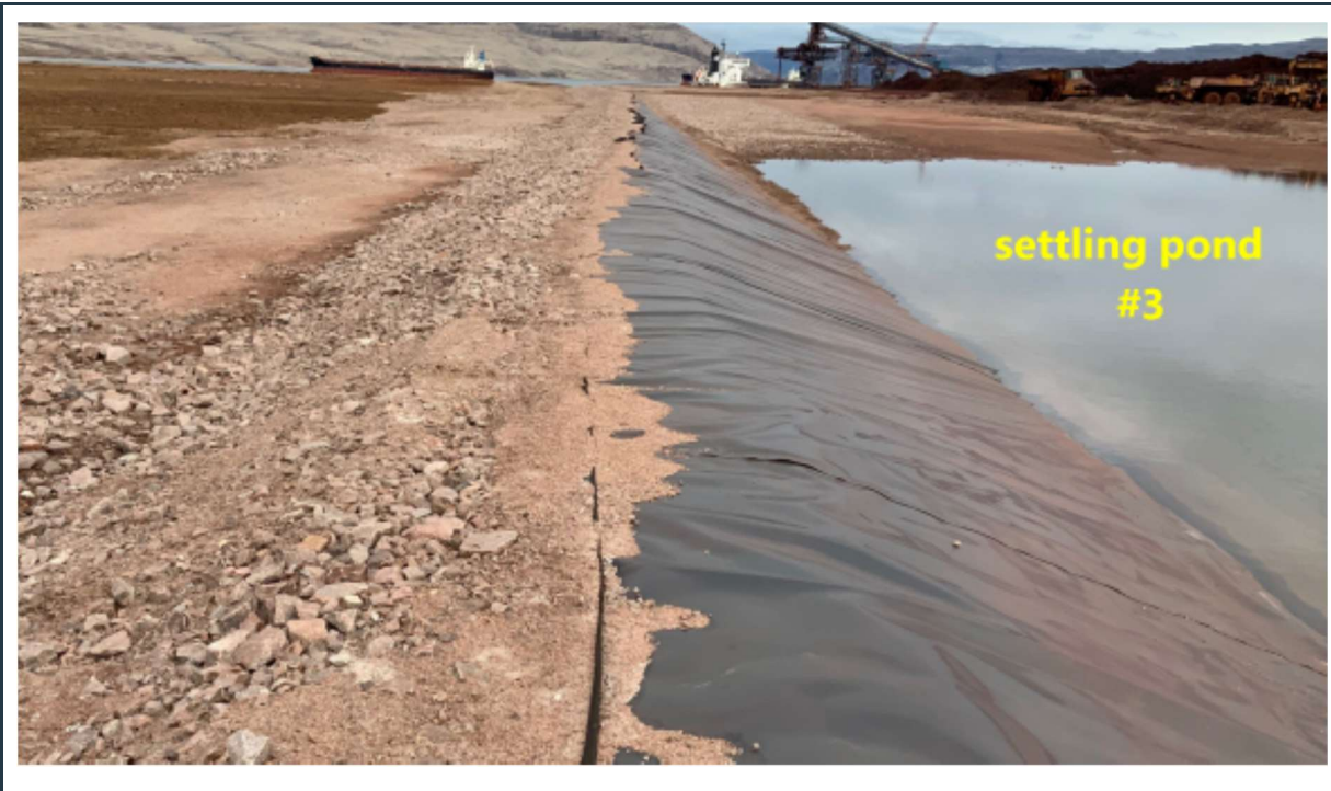
Figure 59: View of the lined, stable berm along the west side of settling pond #3.
