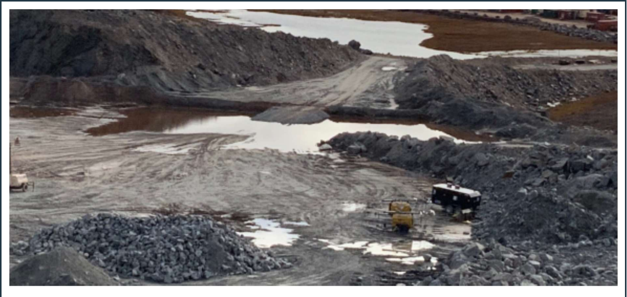
Figure 37: View part of the QMR2 quarry with area that still requires a more efficient surface water control. Rainwater should be properly drained from the traveled areas of the quarry.
