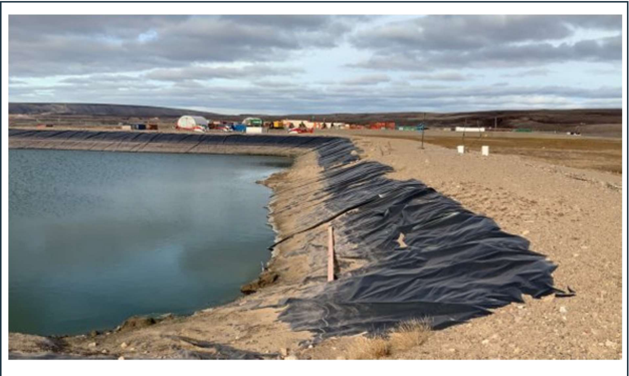
Figure 11: PWS pond #2 – Stable berm around the pond. The water was lowered in the summer.
