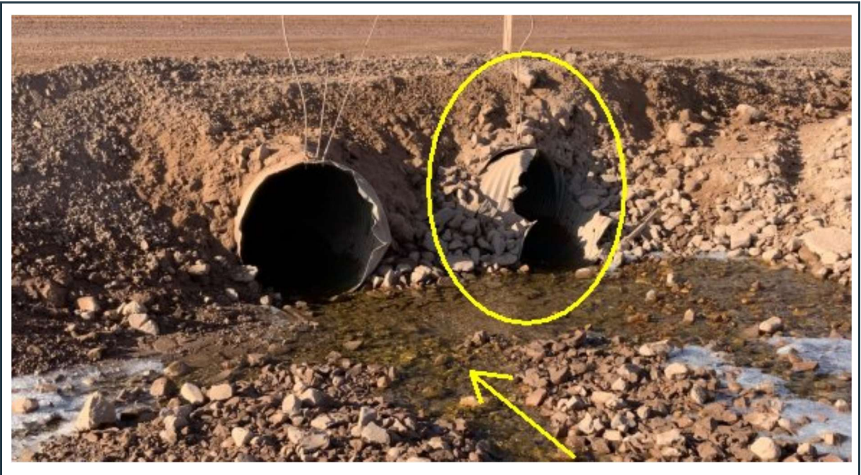
Figure 99: View of culvert(s) 114D inlets (looking west). Repair of the northern pipe is required (yellow circle).
