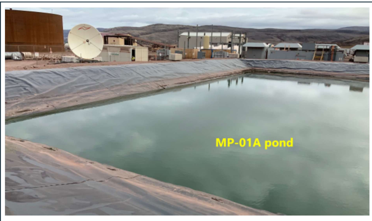
Figure 48: Berms and liner in excellent condition with stable slopes around the MP-01A pond.
