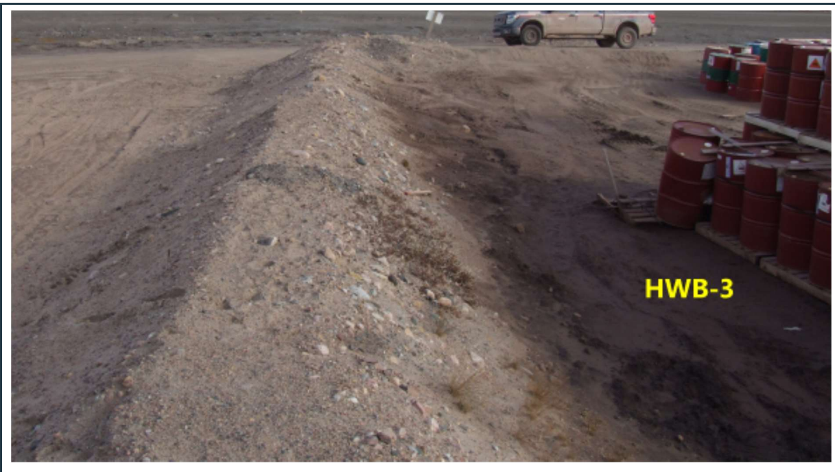
Figure 15: View of stable berms and the stored fuel barrels in HWB-3.
