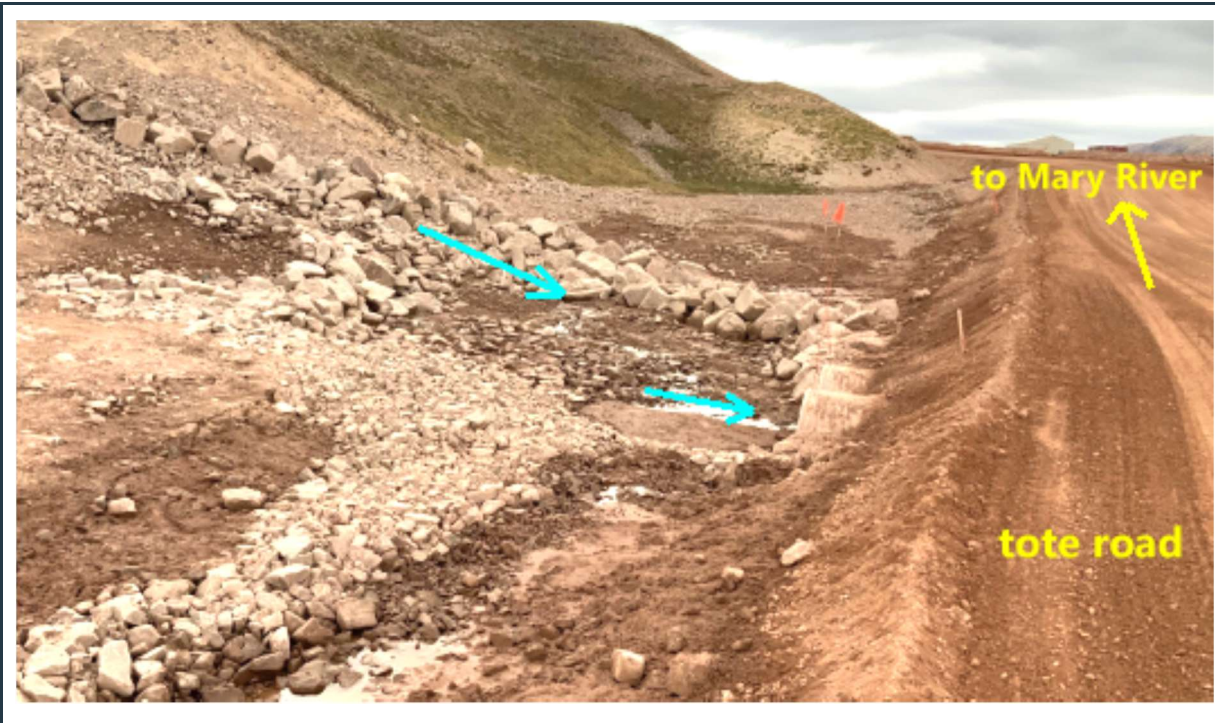
Figure 87: View of twin culverts, draining surface water under the tote road (inlet).
