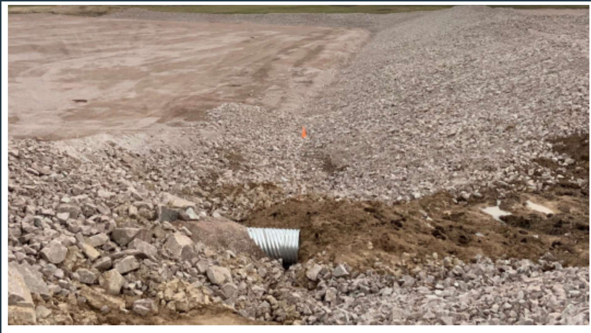
Figure 85: View of the P-SC surface water collection ditch and culvert (still under construction).
