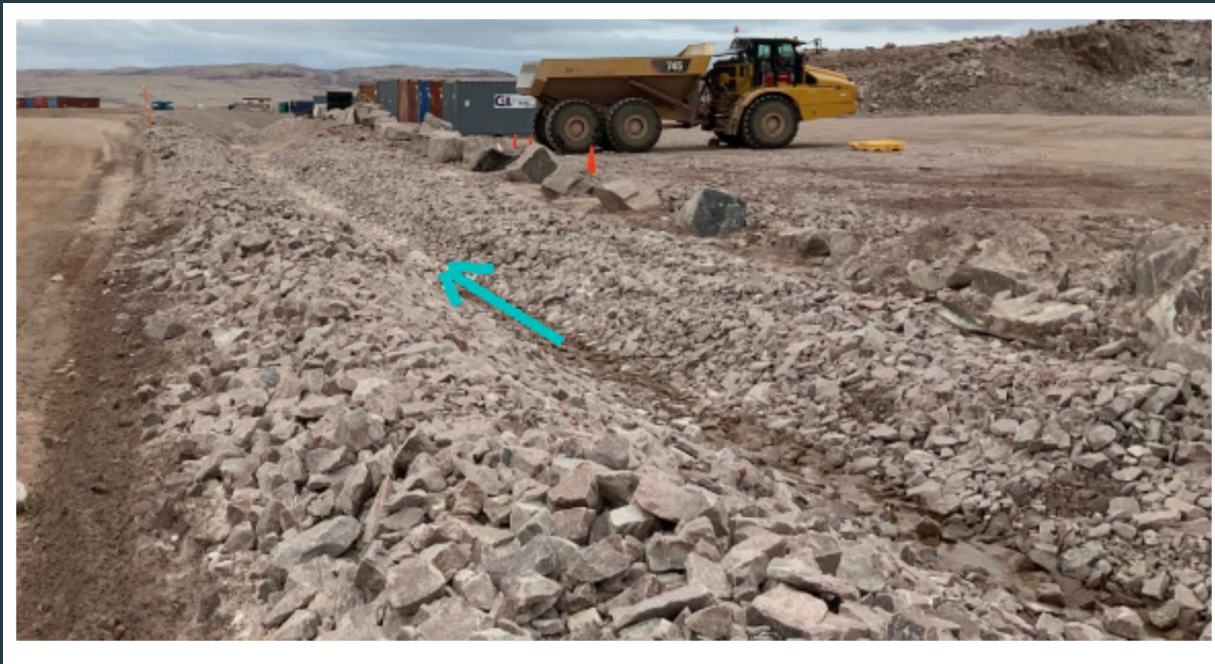
Figure 63: P-SWD-5 – "Q01-North" surface water collection ditch.
