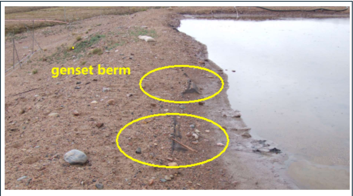
Figure 32: View of the berm near the generator, with exposed geotextile and liner at a few locations.
