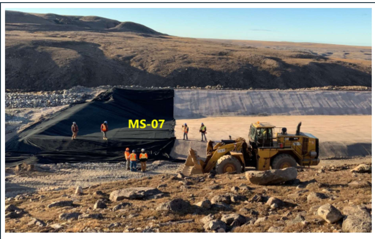
Figure 42: Construction of the MS-07 pond is in progress south of the proposed ore stockpile area.
