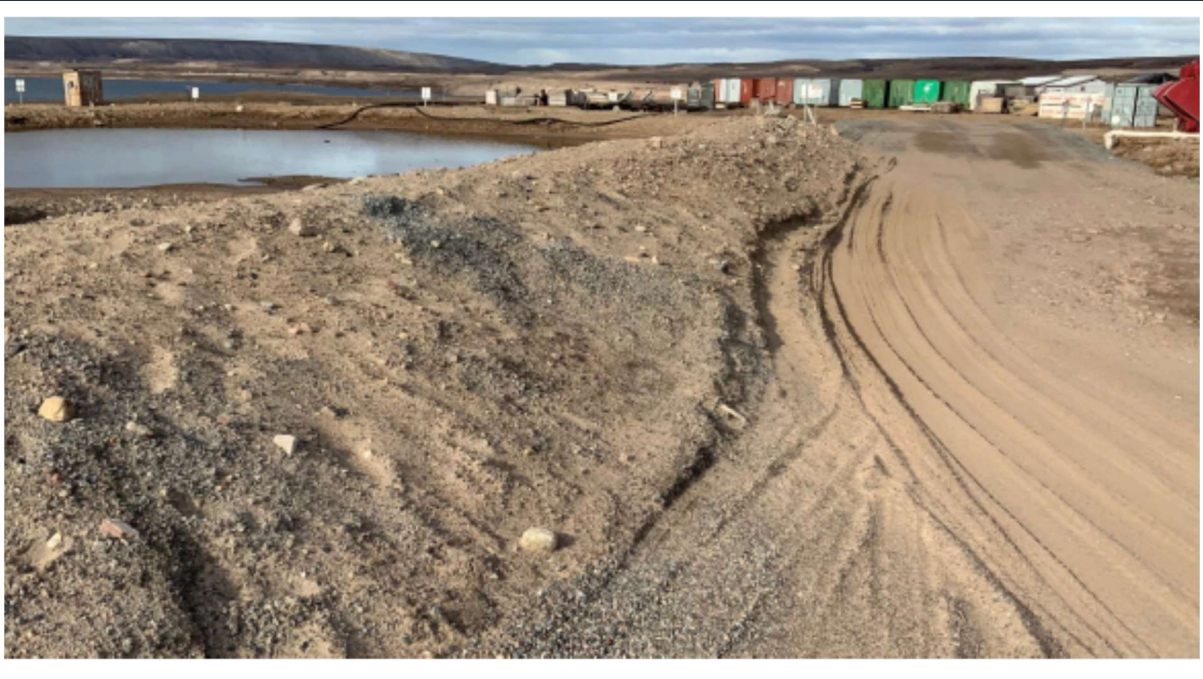
Figure 29: View of slope deterioration at a section of the generator fuel berm. Trucks bypassing occasional ponding surface water on the road are “cutting” into the toe of the berm.
