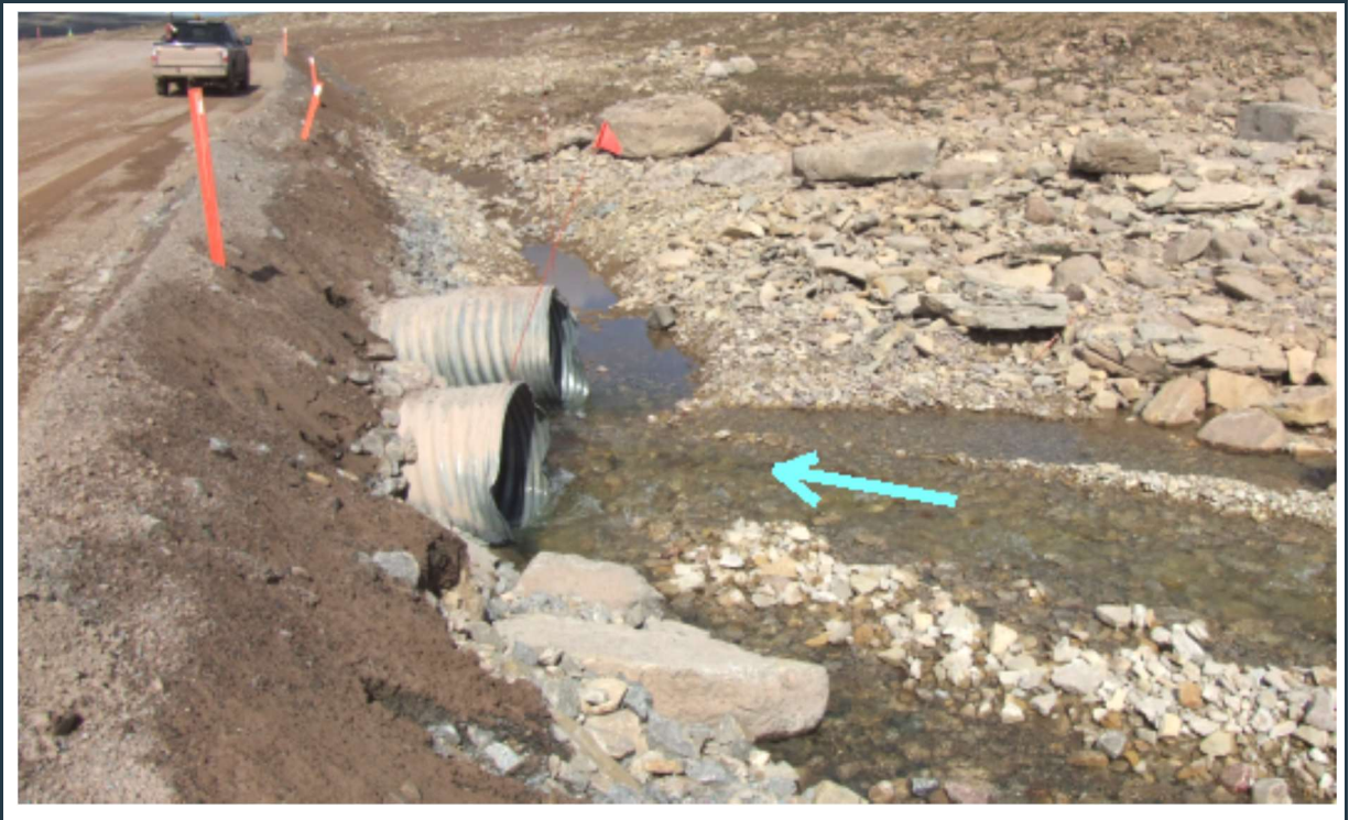
Figure 103: View of culvert(s) 094 (inlet) in good condition.
