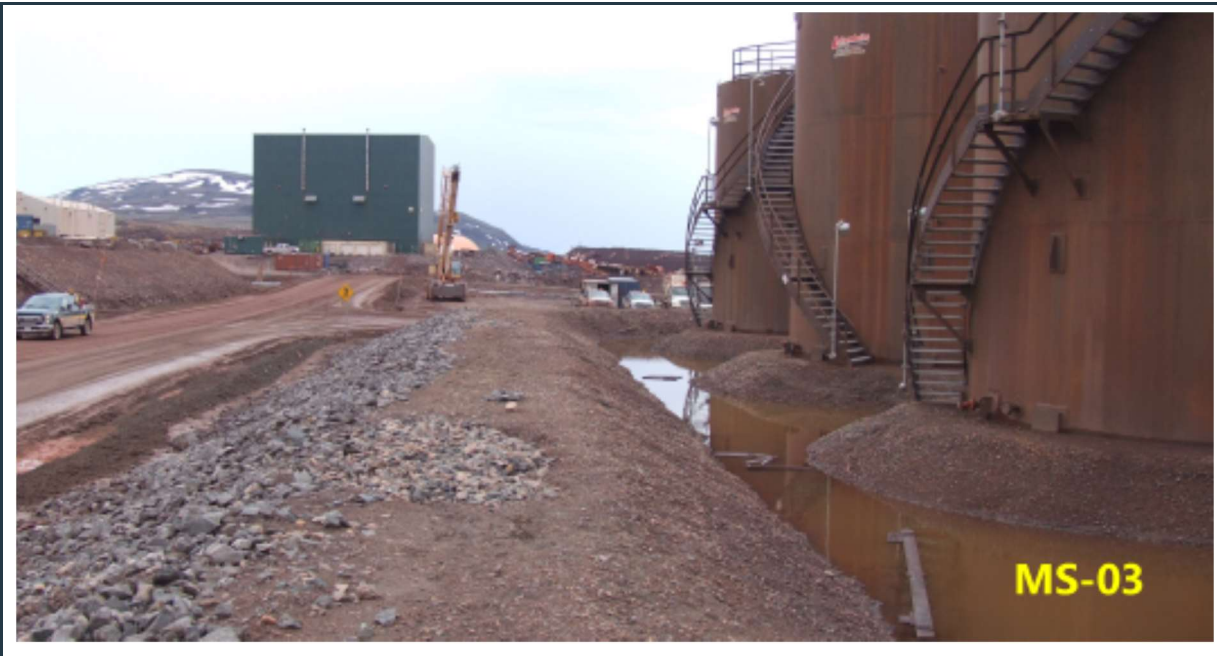
Figure 37: View of the MS-03 diesel fuel farm. Note some floating debris that should be removed.
