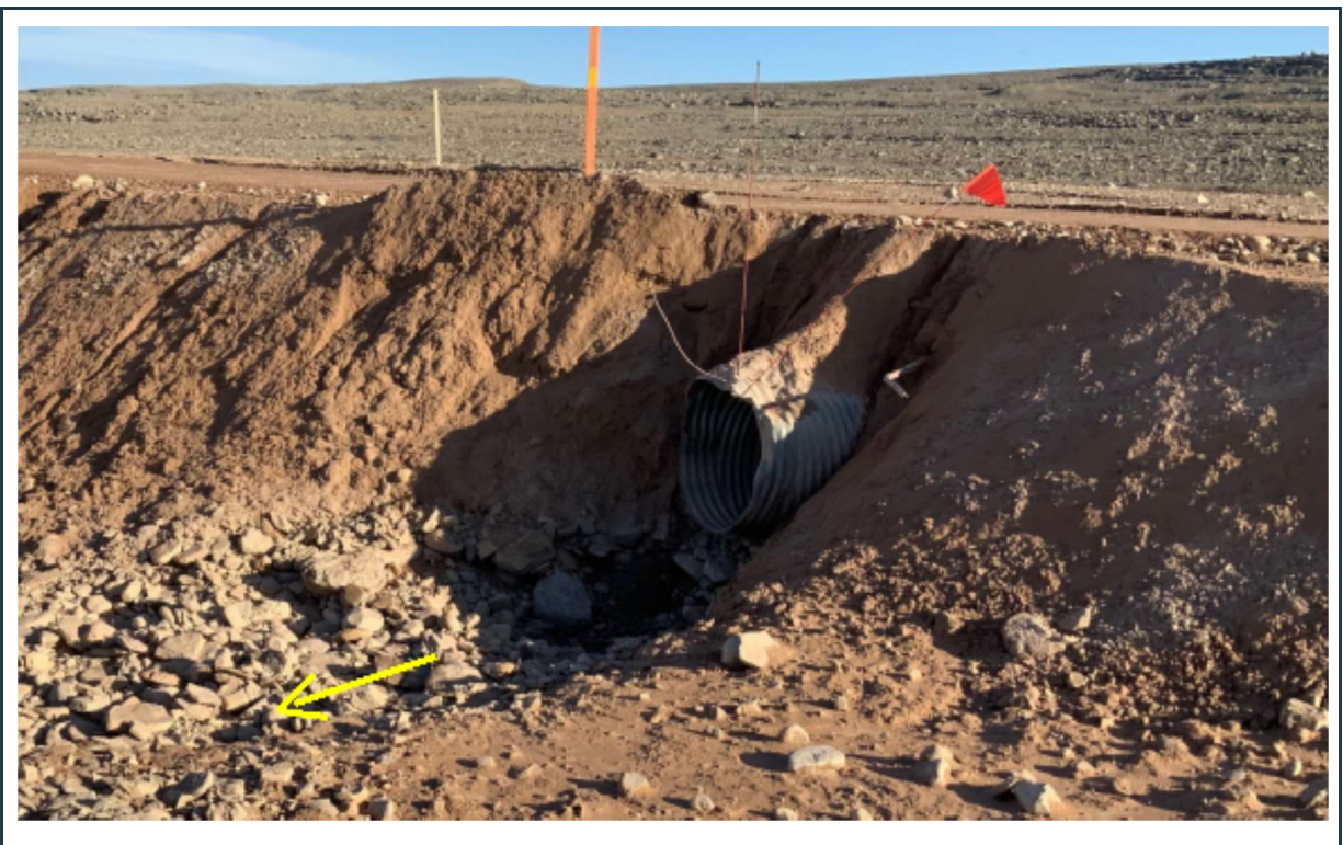
Figure 86: View of culvert 083 outlet (looking north-east), with slope erosion of the embankment around the culvert.
