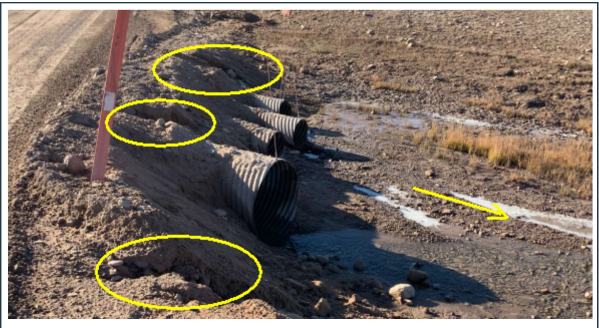
Figure 90: View of culvert(s) 102 outlets in good condition (looking south). Note some erosion on the slopes of the road embankment around the culverts (yellow circles).
