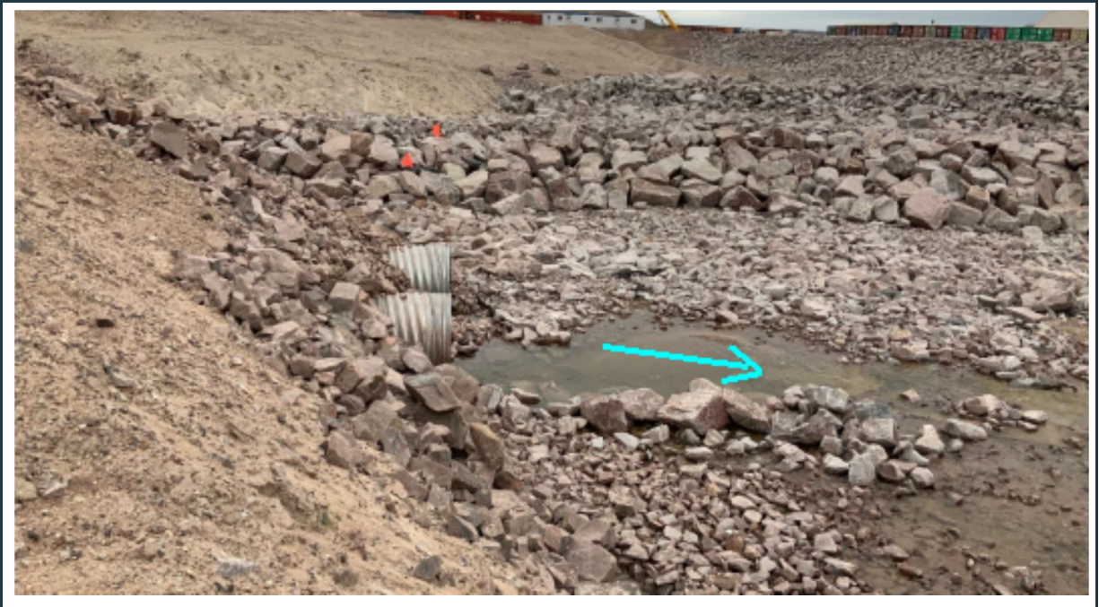
Figure 81: View of the P-SWD-7 surface water collection ditch and culverts (outlet).
