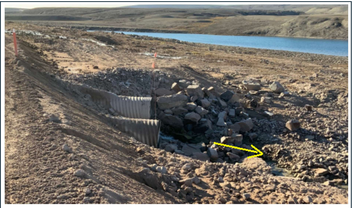
Figure 88: View of culvert(s) 094 outlet, in good condition (looking south).
