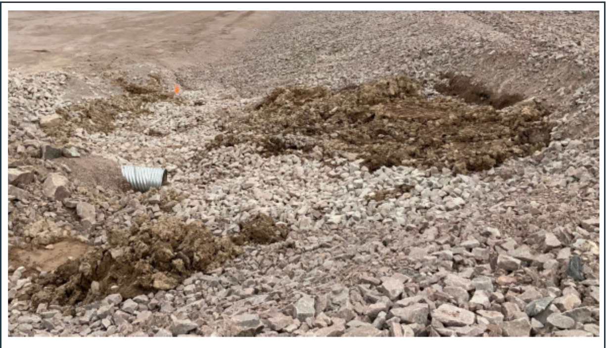
Figure 70: View of the PSC surface water collection ditch and culvert (still under construction). The culvert will need to be shortened and the slope with rip-rap regraded.
