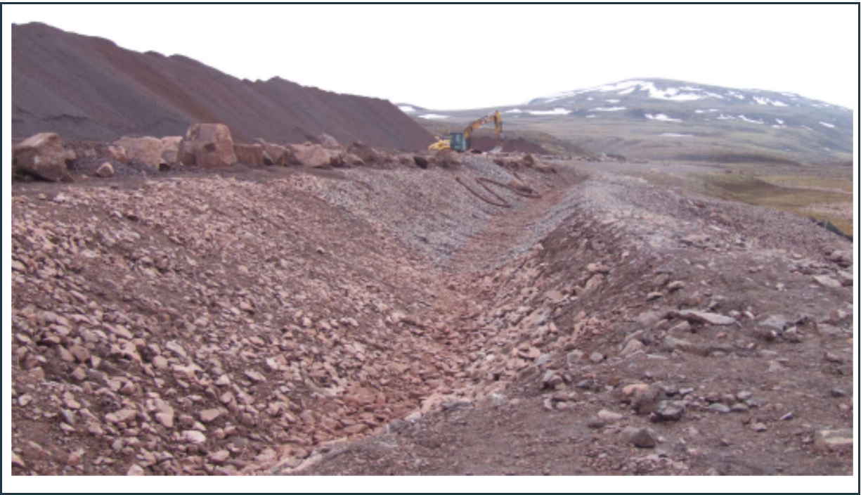
Figure 22: Well maintained surface-water collection ditch around the crusher plant, leading to MS-06.
