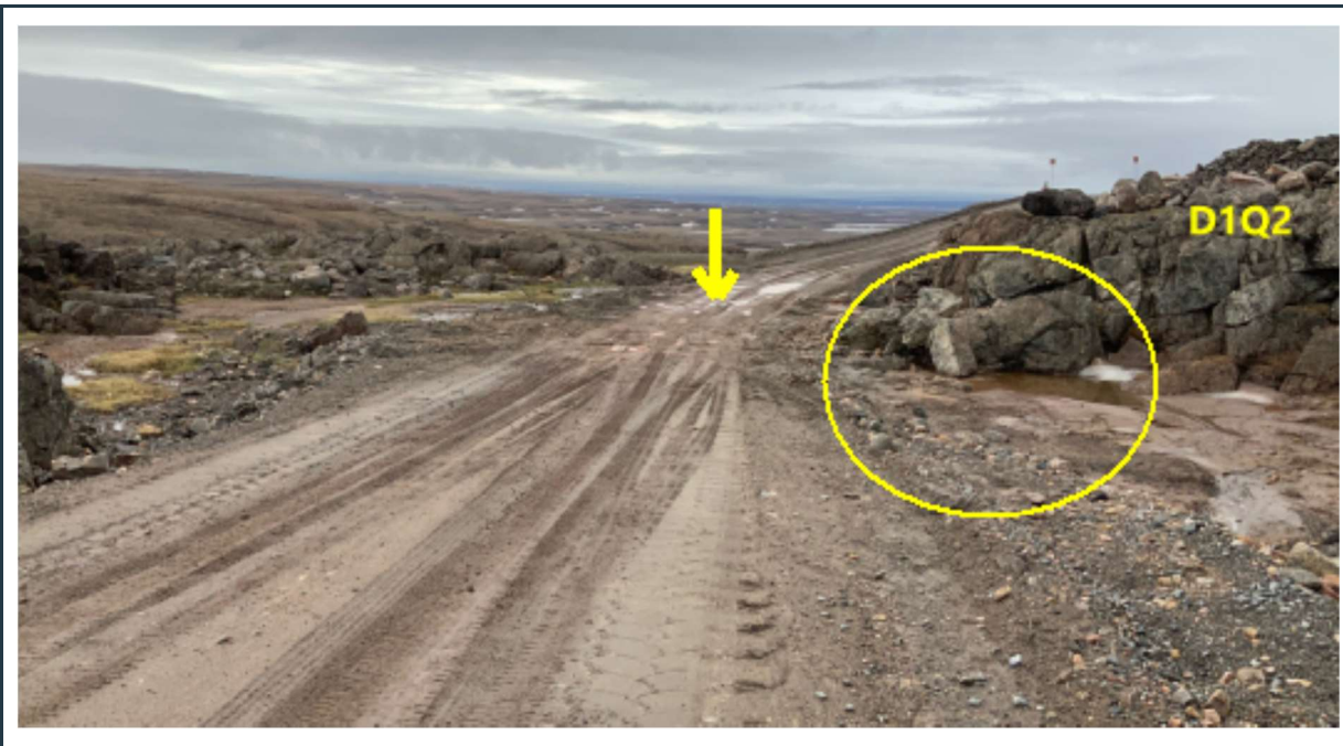
Figure 52: Ponding water at the edge of the future D1Q2 quarry. Culvert is required at the low point of the road and the road grade should be raised in the area above the culvert.
