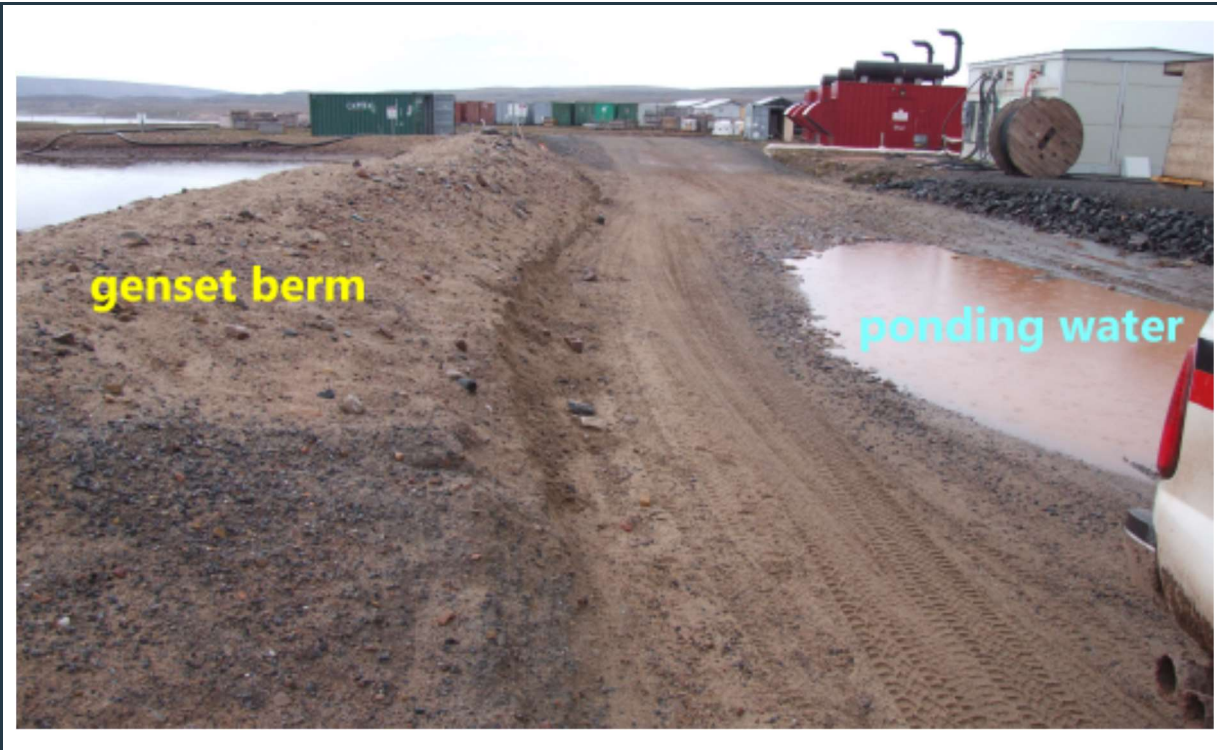
Figure 33: View of slope deterioration at a section of the berm near the generators. Trucks bypassing ponding surface water on the road are “cutting” into the toe of the berm.
