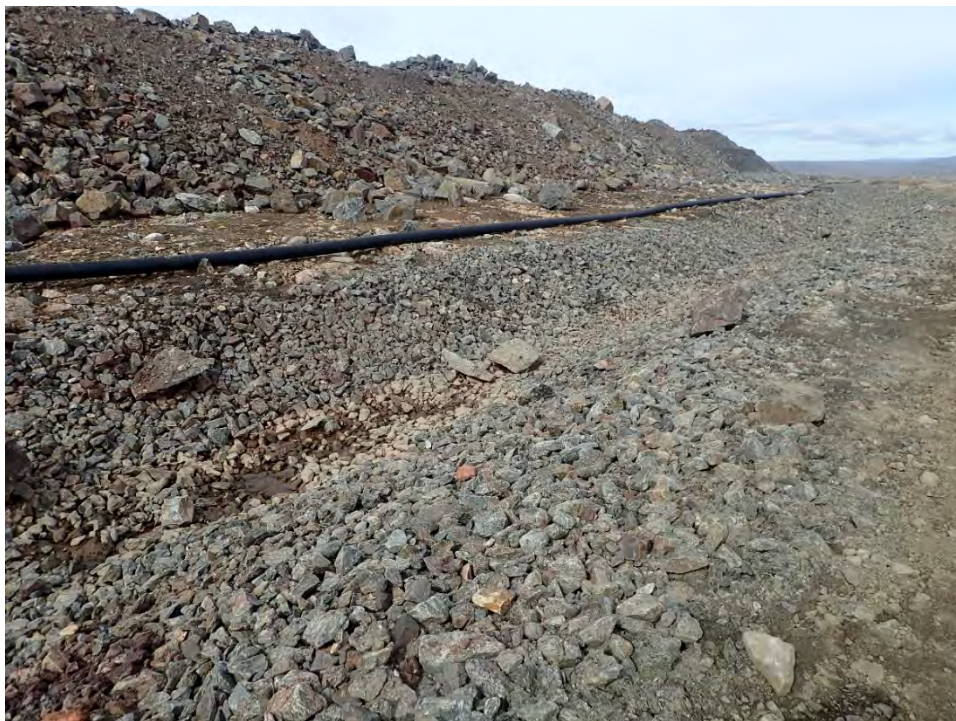
Photo 8 – New Pit Dewatering Line at Waste Rock Facility
