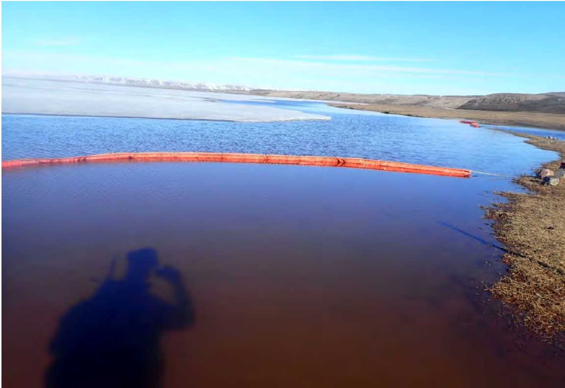
Photo 9: CLSP Outfall into Silt Curtain on June 11, 2020
