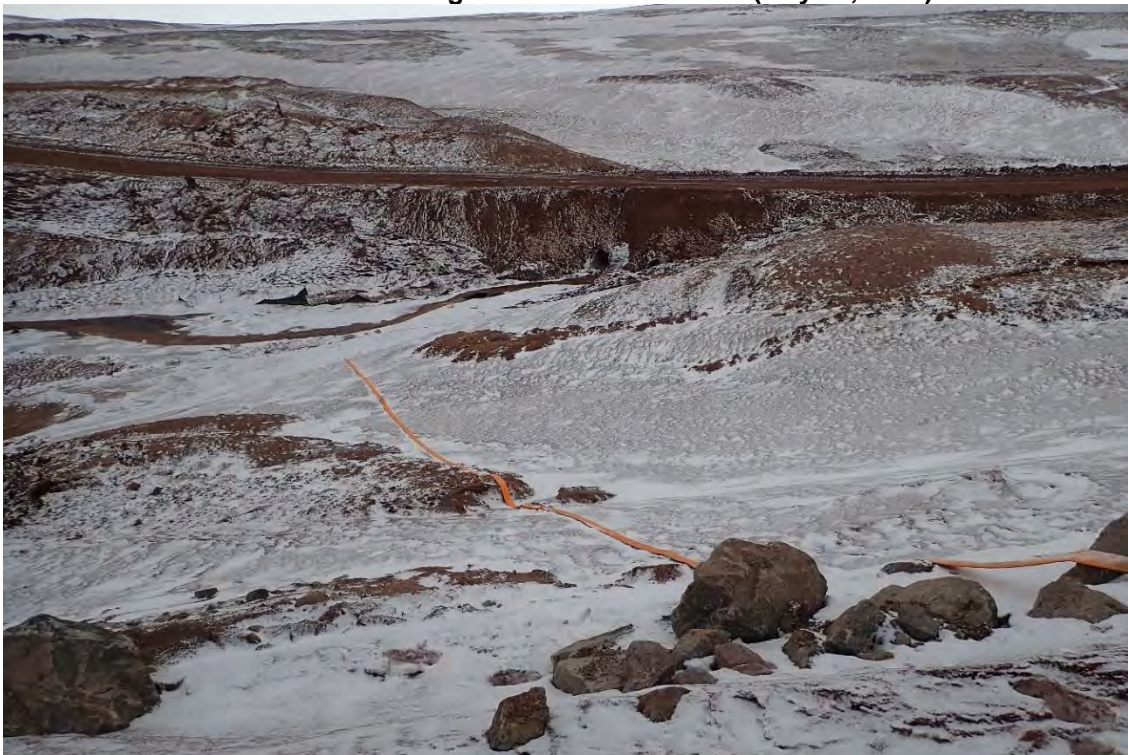
Photo 6. Pumping Diversion from Unstable Sandy Slope at the Outlet of BG-01 (May 18, 2020)
