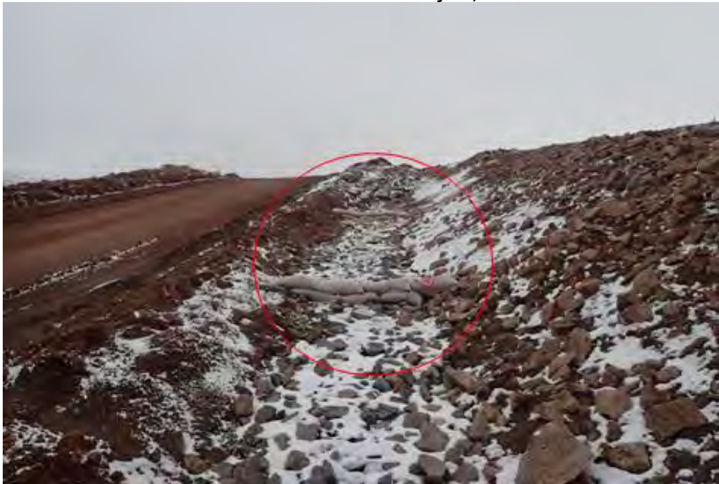
Photo 4: BG-01 Downstream Ditch with Sand Bags (May 18, 2020)
