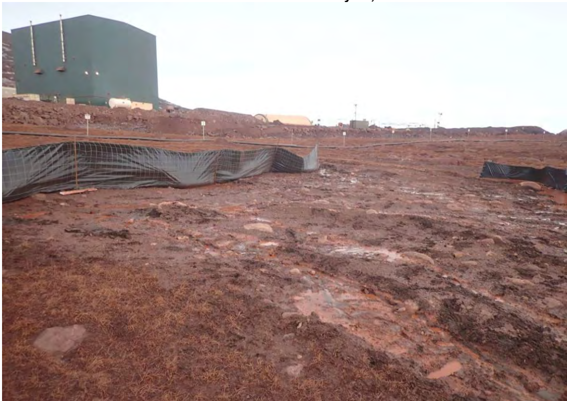
Photo 4. Erosion and Sediment Control Down Slope of Power Generation Building Minimizing Sediment Entering CV-187 (May 22, 2020)
