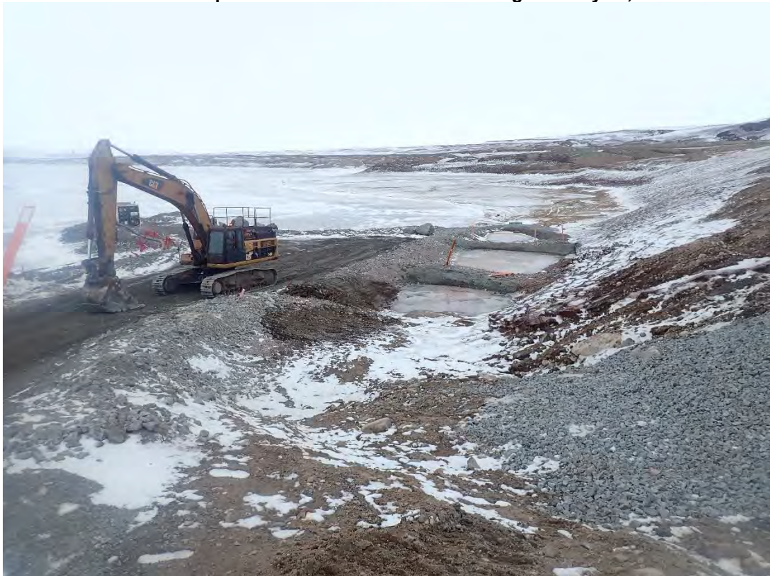
Photo 6: Camp Lake Settling Improvements on May 21, 2020
