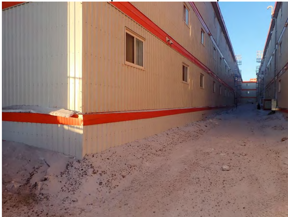
Photo 2. Spill location following clean-up
