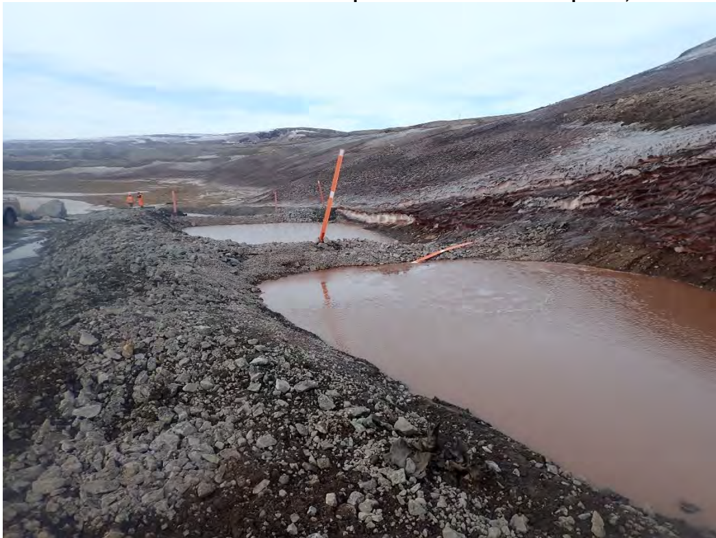
Photo 2. Camp Lake Check Dams on May 16, 2020
