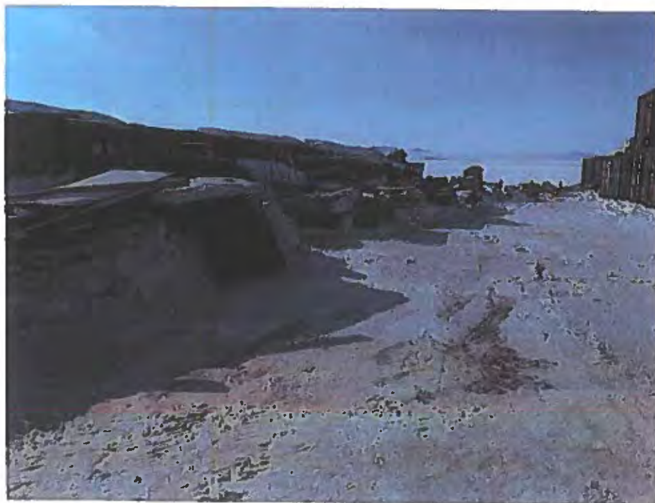
Photo 2. Remediated area at R3 Laydown
