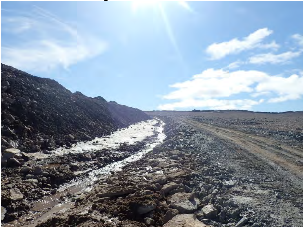
Photo 2. Ring Road Ditch Swale after Enhancement
