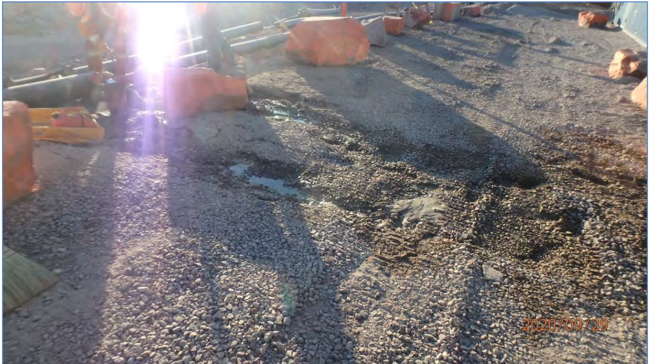
Photo 1. Sewage Spill Location before Clean Up on Sept 29, 2020
