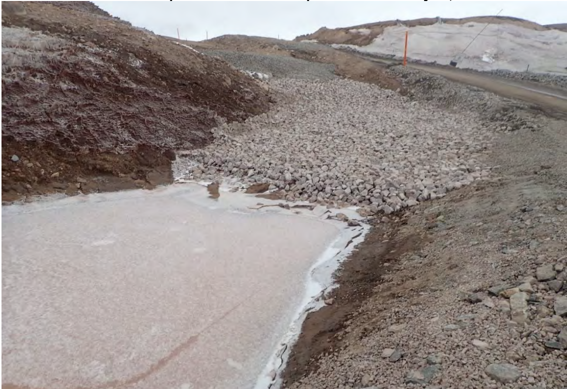
Photo 8: Camp Lake Slope Rip Rapping on May 23, 2020
