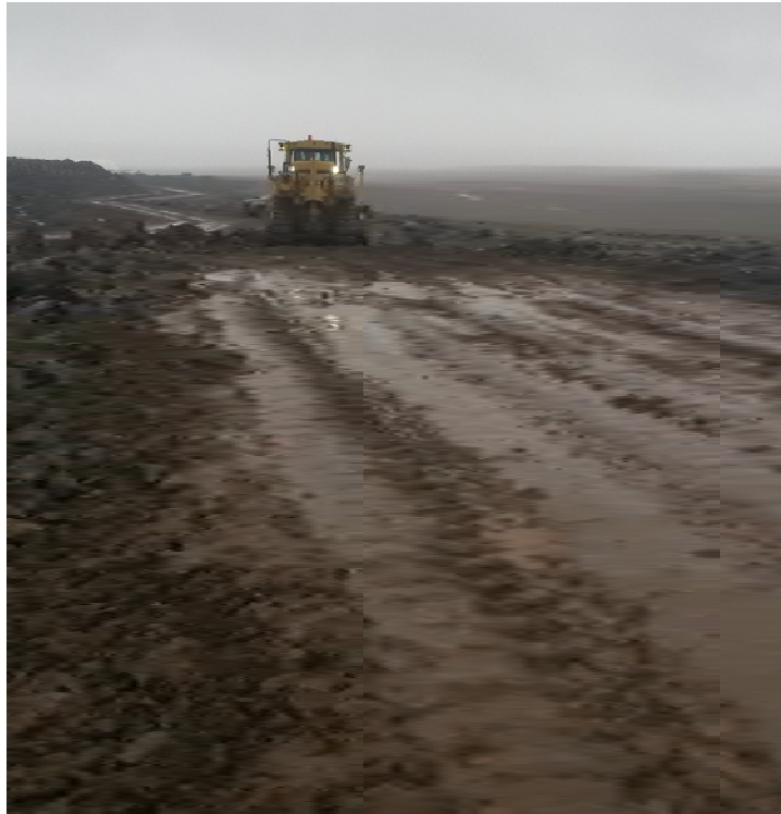
Photograph 20- East Ditch placement of rockfill for Diversion Berm August 14, 2021.
