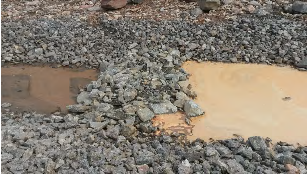
Photograph 6- West Ditch construction of check dam, June 28, 2021.
