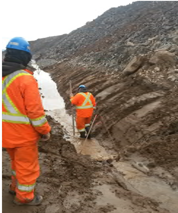
Photograph 10- West Ditch bottom elevation check, July 2, 2021.
