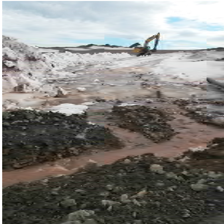
Photograph 8- East Ditch snow removal and temporary ditch construction, June 29, 2021.
