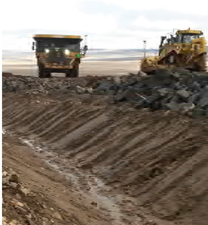
Photograph 18- East Ditch excavation in soft soil, August 10, 2021.
