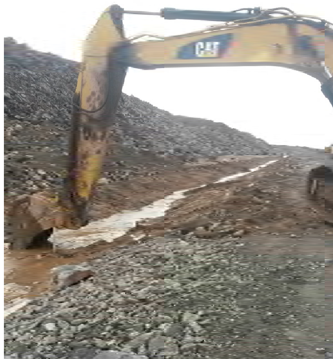
Photograph 9- West Ditch excavation in soft soil, July 1, 2021.
