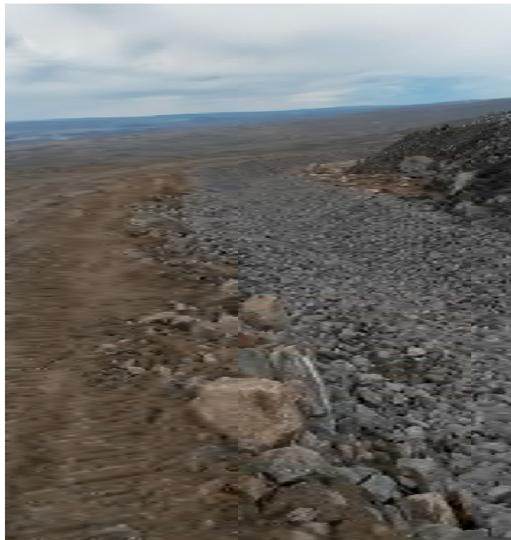
Photograph 13- West Ditch riprap layer for erosion protection, July 28, 2021.
