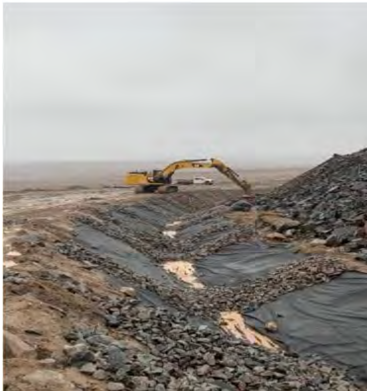
Photograph 11- West Ditch geotextile installation, July 26, 2021.
