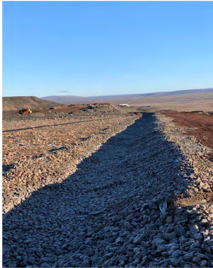
Photograph 24- East Ditch riprap cover of 280 mm thickness, August 27, 2021.
