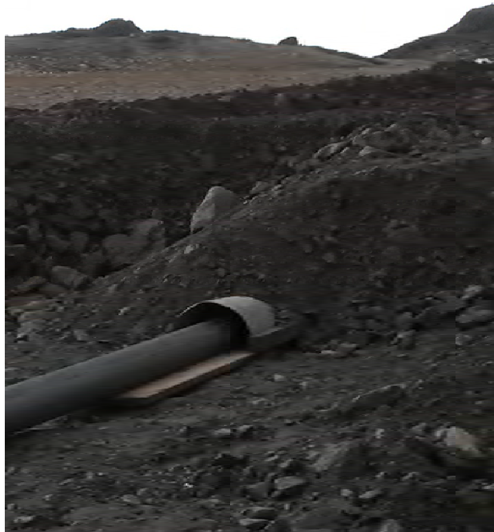
Photograph 16- East Ditch pipe culvert installation for protection of existing HDPE pipeline, August 8, 2021.
