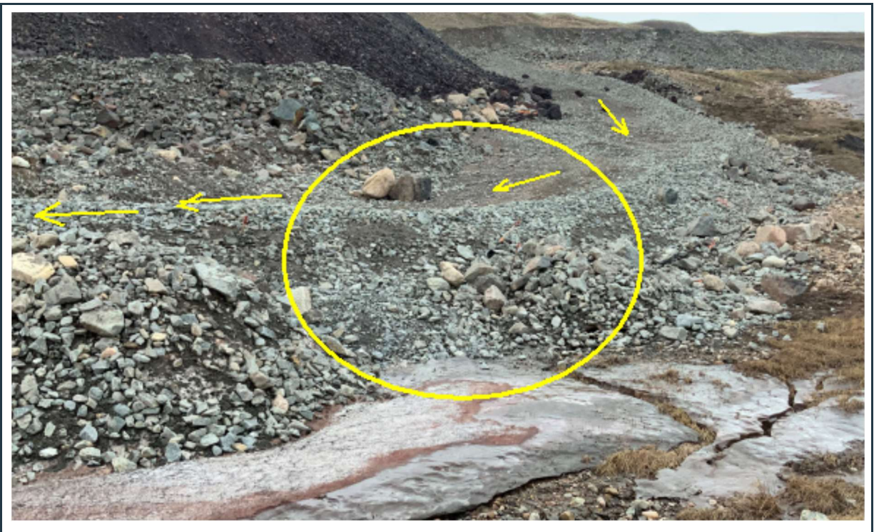
Figure 40: View of the surface water diversion berm at the new KM-106 ore stockpile area.
