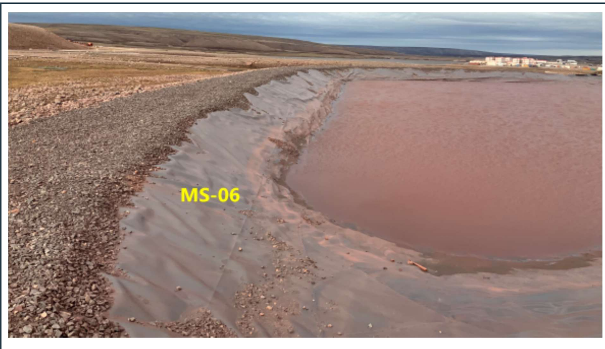
Figure 20: MS-06 surface-water collection and settling pond with robust, stable berms and intact liner.
