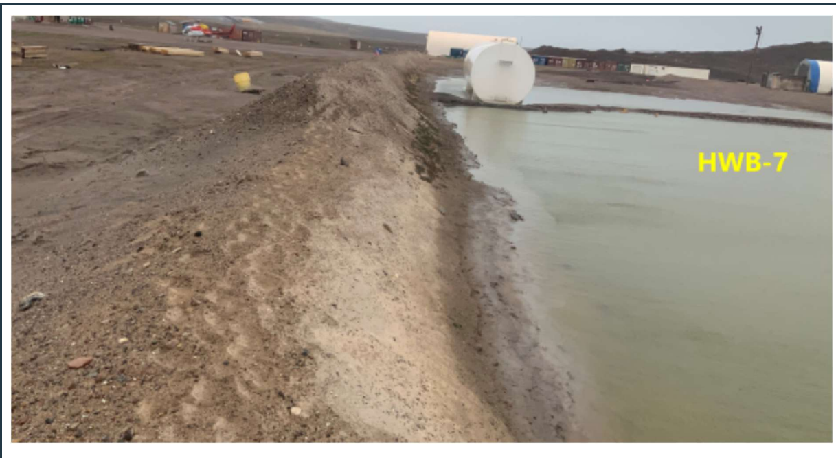
Figure 19: View of the large, flooded HWB-7 cell, with only one fuel tank stored.
