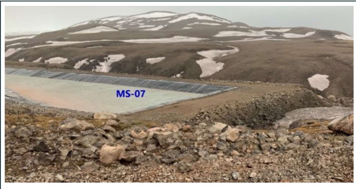
Figure 23: View of the recently completed MS-07 surface-water collection pond with robust, stable berms and intact liner.
