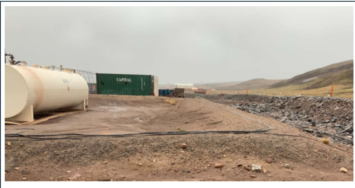
Figure 30: View of the well-maintained sand and gravel berm at the lined jet-fuel storage facility, with the additional rock fill protective berm, constructed between the cell and the tote road.
