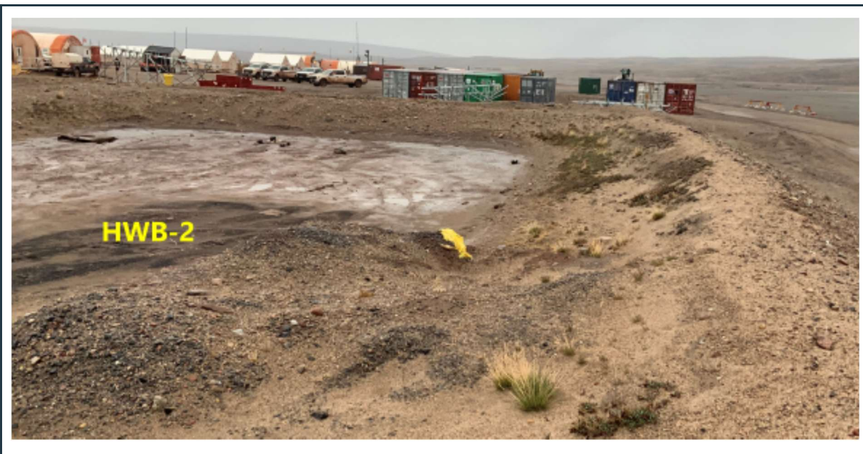
Figure 14: View of stable berms around HWB-2. The cell is currently empty.
