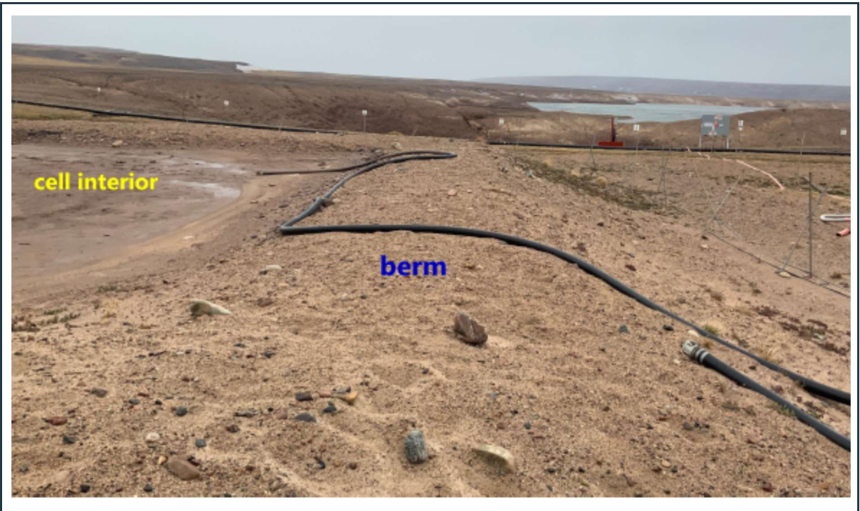
Figure 28: View of the stable berm around the "generator fuel bladder" cell. The cell is currently empty.
