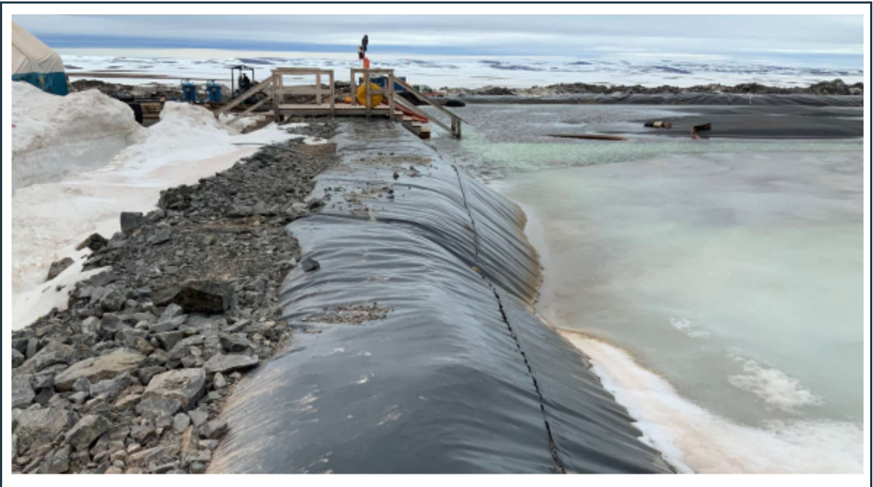
Figure 27: Stable rock fill berm at the water treatment pond, adjacent to the waste rock facility.
