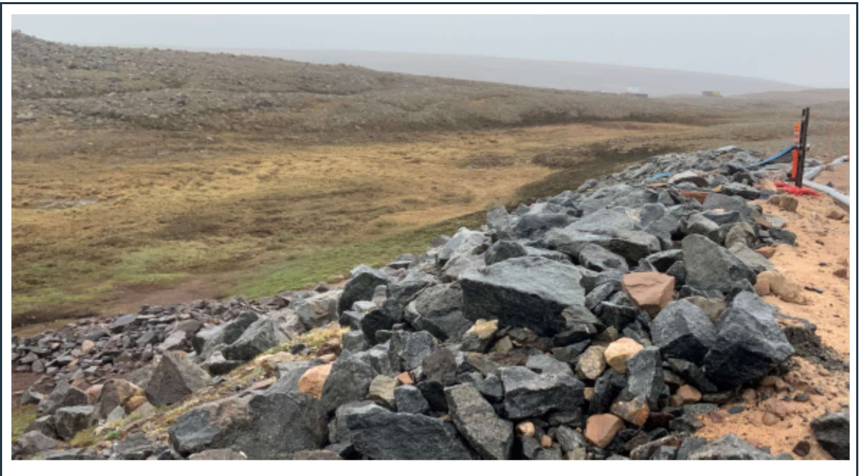
Figure 35: Stable rock fill riprap slope protection at the water discharge area.
