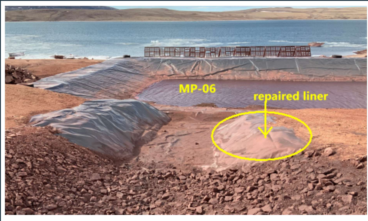
Figure 55: View of the lined MP-06 pond with robust, stable berms (north-west corner of the ore stockpile). Note the repaired liner on the slope of the intake to the pond (yellow circle).
