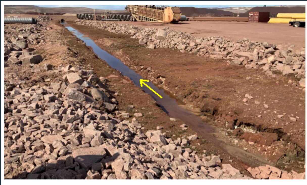
Figure 65: View of the W3/W14 uncompleted surface water collection ditch with some erosion.
