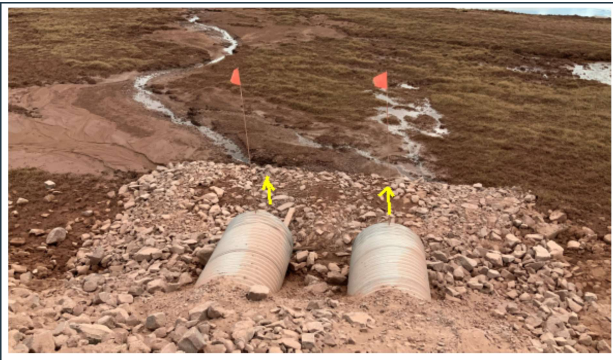
Figure 70: View of twin culverts, draining surface water from the quarry area (outlet).
