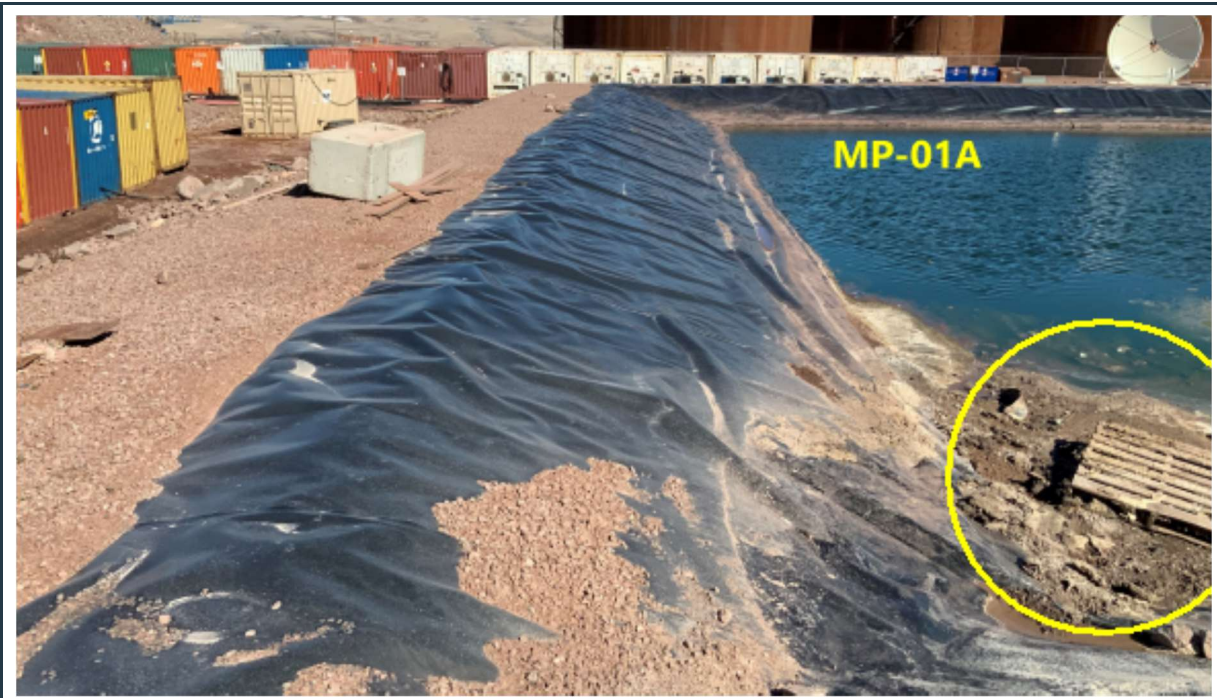
Figure 46: Berms and liner in good condition with stable slopes around the MP-01A pond. The waste (soil and wood), shown in one corner of the pond, should be removed (yellow circle).
