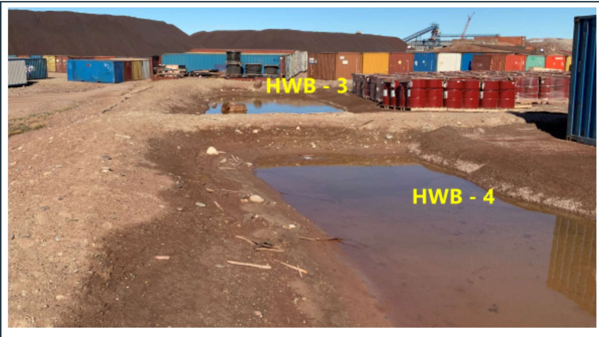
Figure 45: Stable berms around and ponding water within the HWB-3 and HWB-4 cells.
