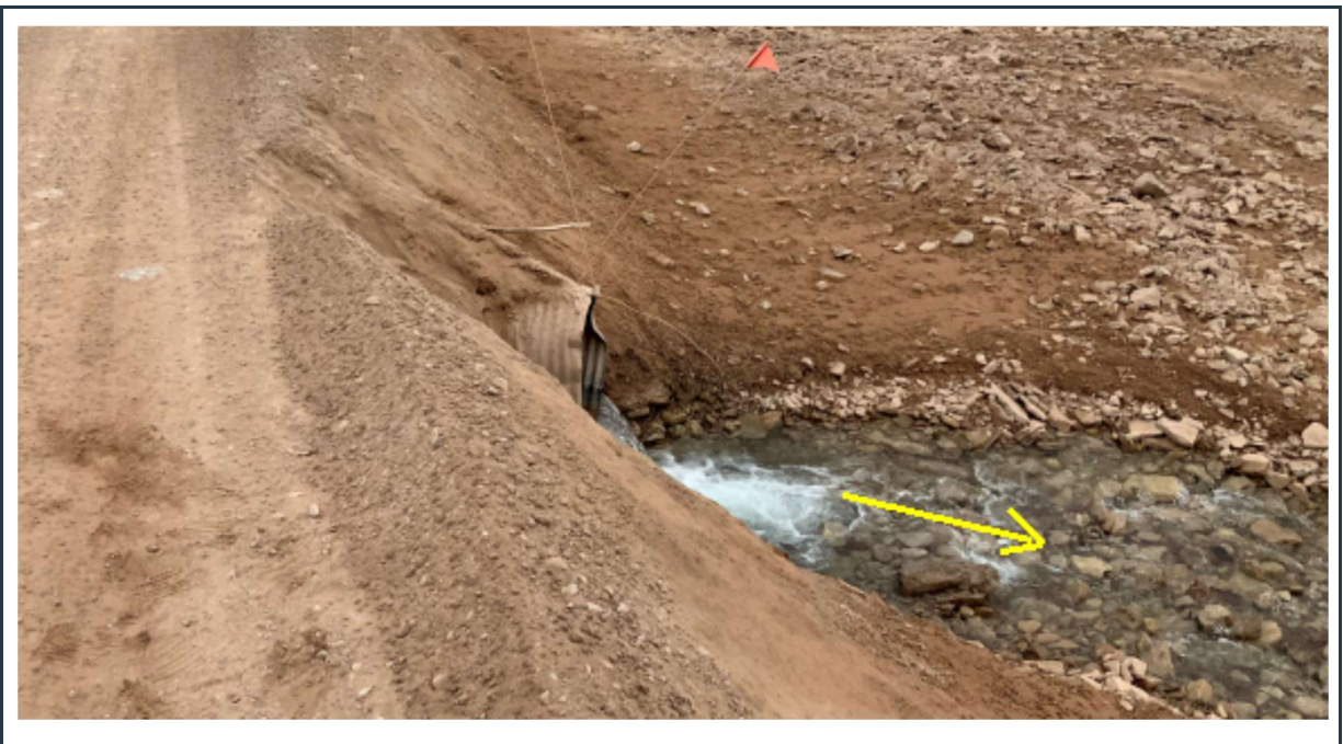
Figure 90: View of culvert 083 outlet, with erosion on the slope of the embankment around the culvert.
