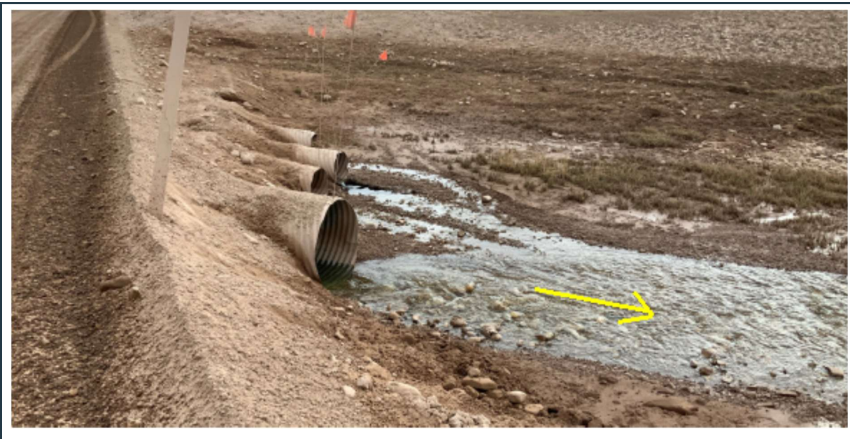
Figure 94: View of culvert(s) 102 outlets in good condition.
