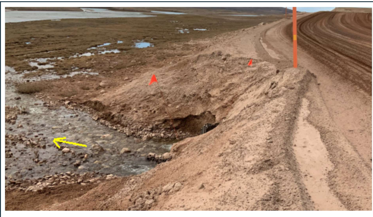
Figure 104: View of culvert(s) 114D damaged outlets. Repair (extension) of both pipes is required.
