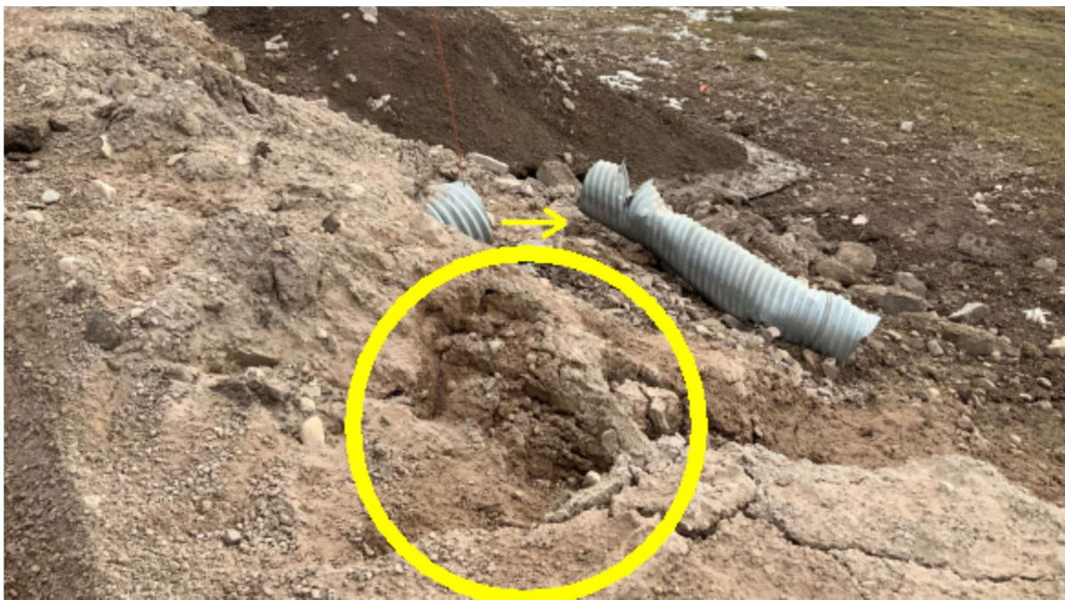
Figure 98: View of culvert 110A outlet. Note that a section of the pipe was cut off, and the erosion of the road embankment adjacent to the culvert (yellow circle).
