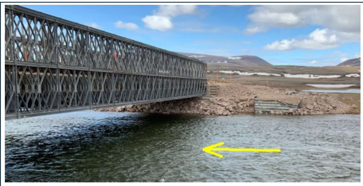
Figure 72: View of the south side of "bridge 17", with stable abutment and riprap scour protection.
