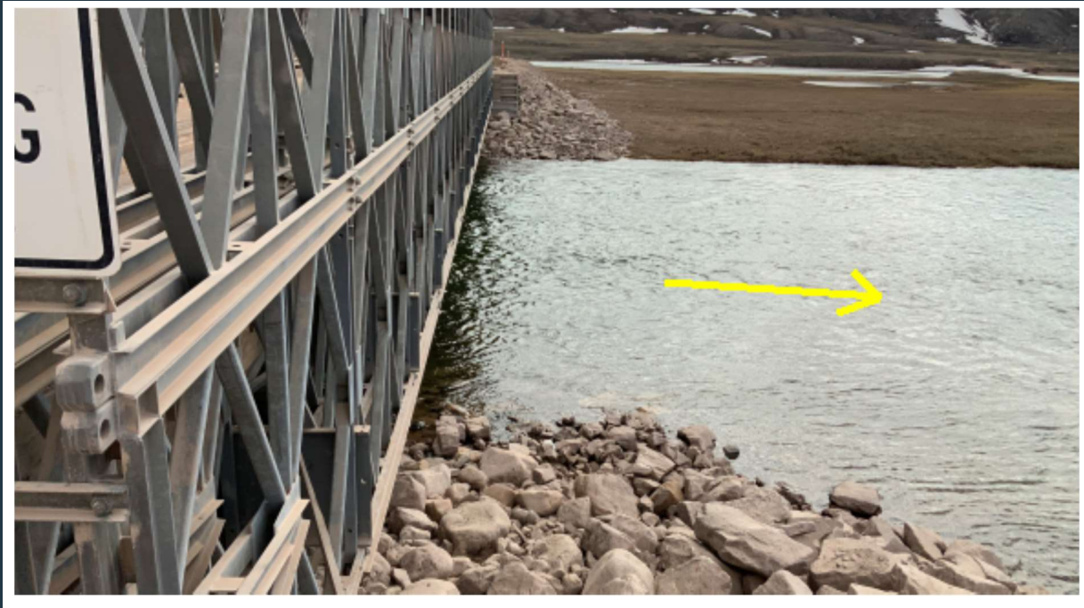
Figure 71: View of the north side of "bridge 17". Note the rip-rap scour protection at the abutments.
