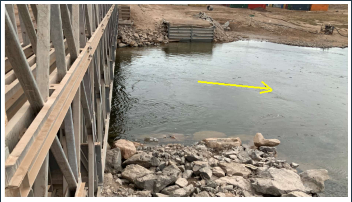
Figure 75: View of the west side of bridge 80, with the “old” abutment providing additional support.
