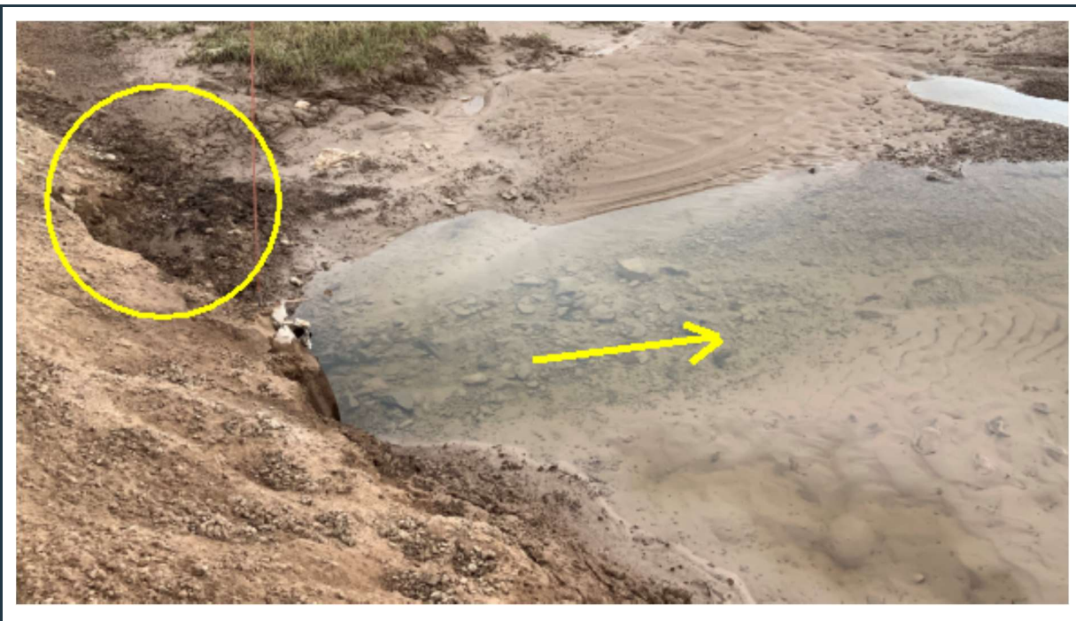
Figure 82: View of the outlet end of culverts 030A and B. Note that one of the pipes is clogged with soil.
