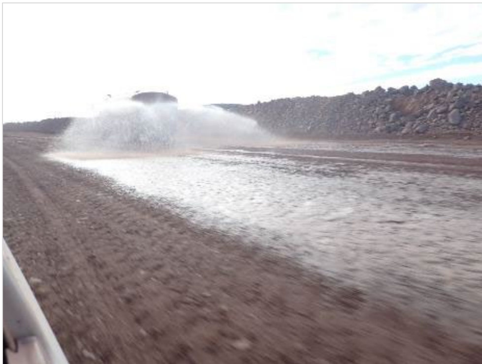
Photo 40 – Mine Site Haul Road Dust Suppression – July 2021
