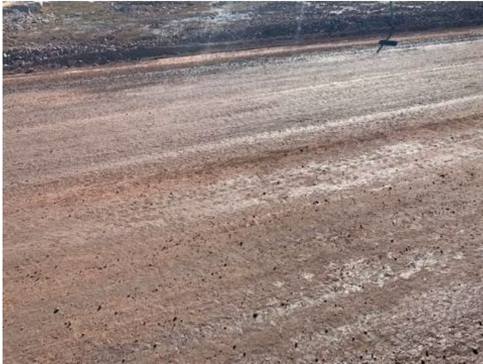
Photo 17 – Road Stabilization after DustBlok® Application
