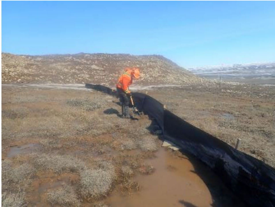
Photo 35 – Silt Fence Installation at Snow Stockpile Site (TR-SN-03) – June 2021
