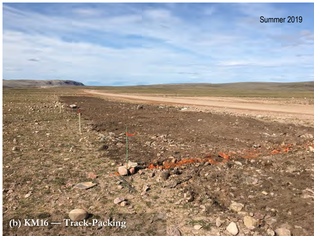
Photo 11. KM16 — Rough and loose (a) and Track-Packing (b).
