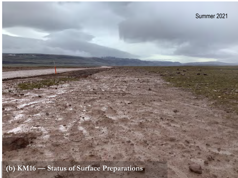
Photo 13. KM16 — Status of Cover Vegetation (a) and Surface Preparations (b).
