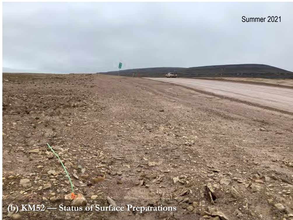
Photo 14. KM52 — Status of Cover Vegetation (a) and Surface Preparations (b).
