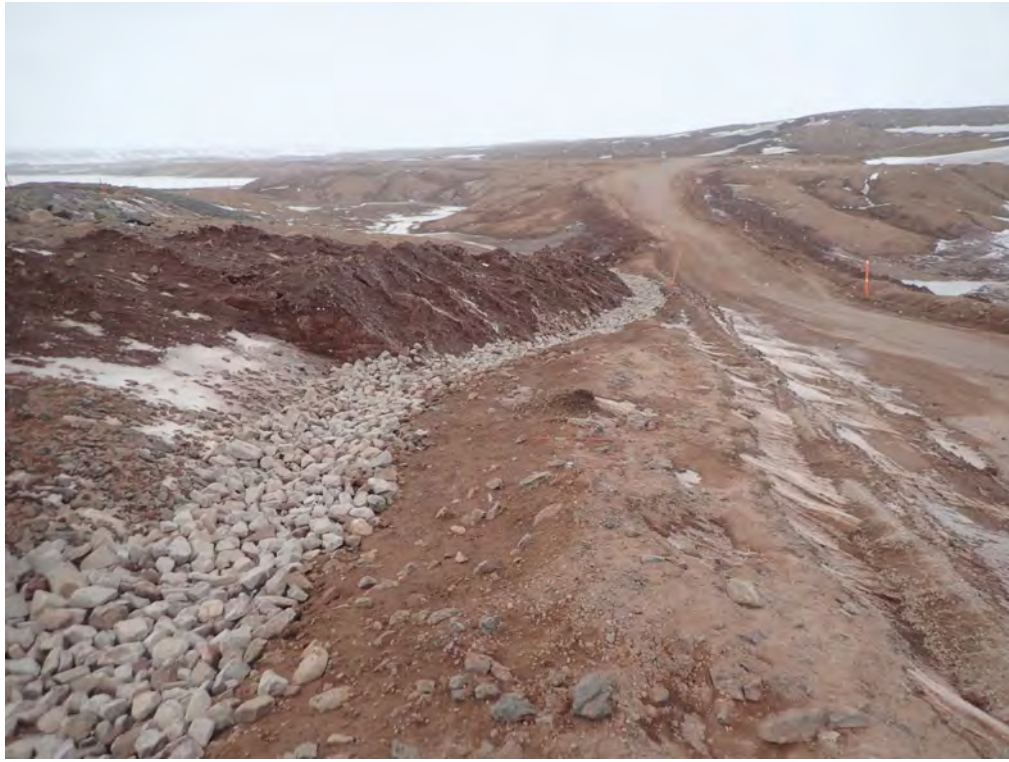
Photo 3. BG-01 Downstream Ditch Riprap Armouring (May 13, 2021)
