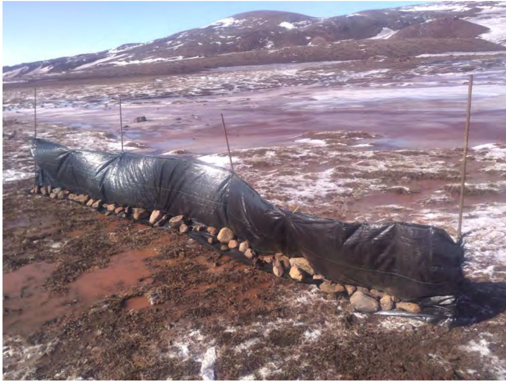
Photo 3. Erosion and Sediment Control at CV-186 Upstream of SDLT-OUT (May 12, 2021)
