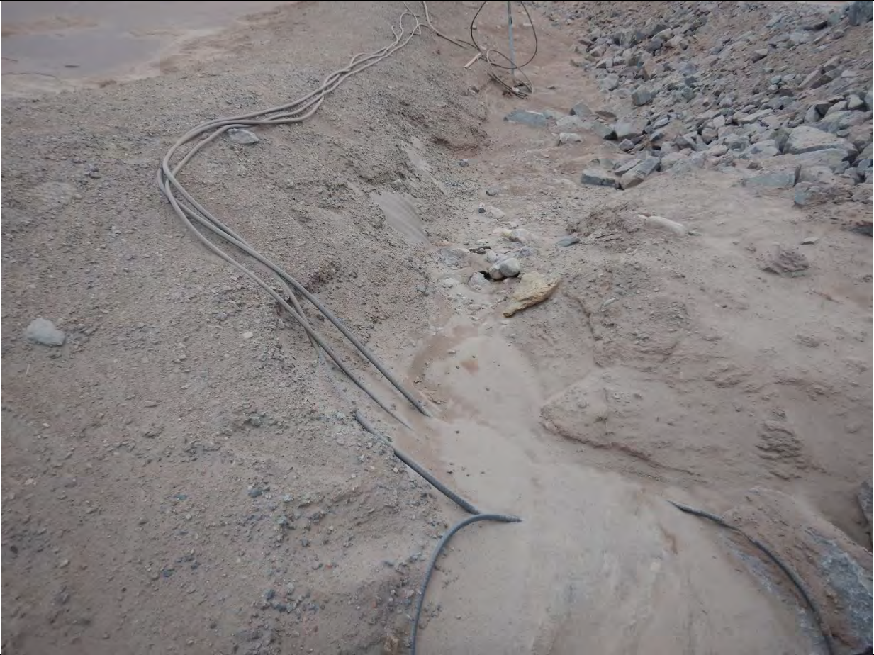
Description: Erosion on outside of aircraft fuel berm.
