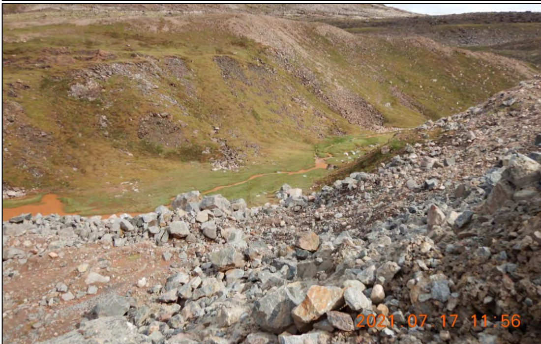
Photo 31. Site of the KM105 proposed sedimentation pond. Currently large quantity of pooling water with discoloration. No clear drainage path.
