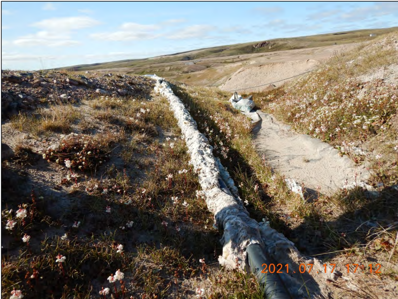
Photo 12. Old pipeline to Camp Lake Jetty. Insulation deteriorating and blowing on tundra.
