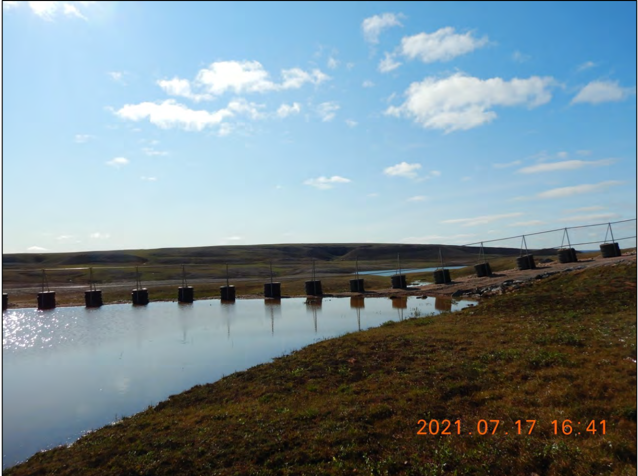
Photo 11. Landfill ponding water. Edge of ponding water appears to flow past barriers towards Sheardown Lake.
