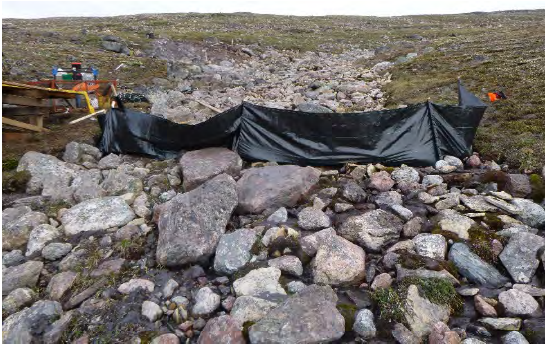
Photo 12 – Silt Fence at MR3-20-283 & 287 Location - 26 JULY 2021
