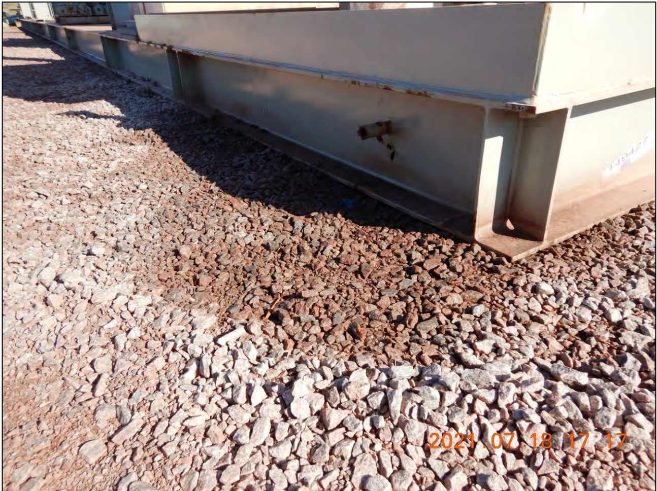
Photo 23. Potential oil spill at northwest corner of power generation station under construction.
