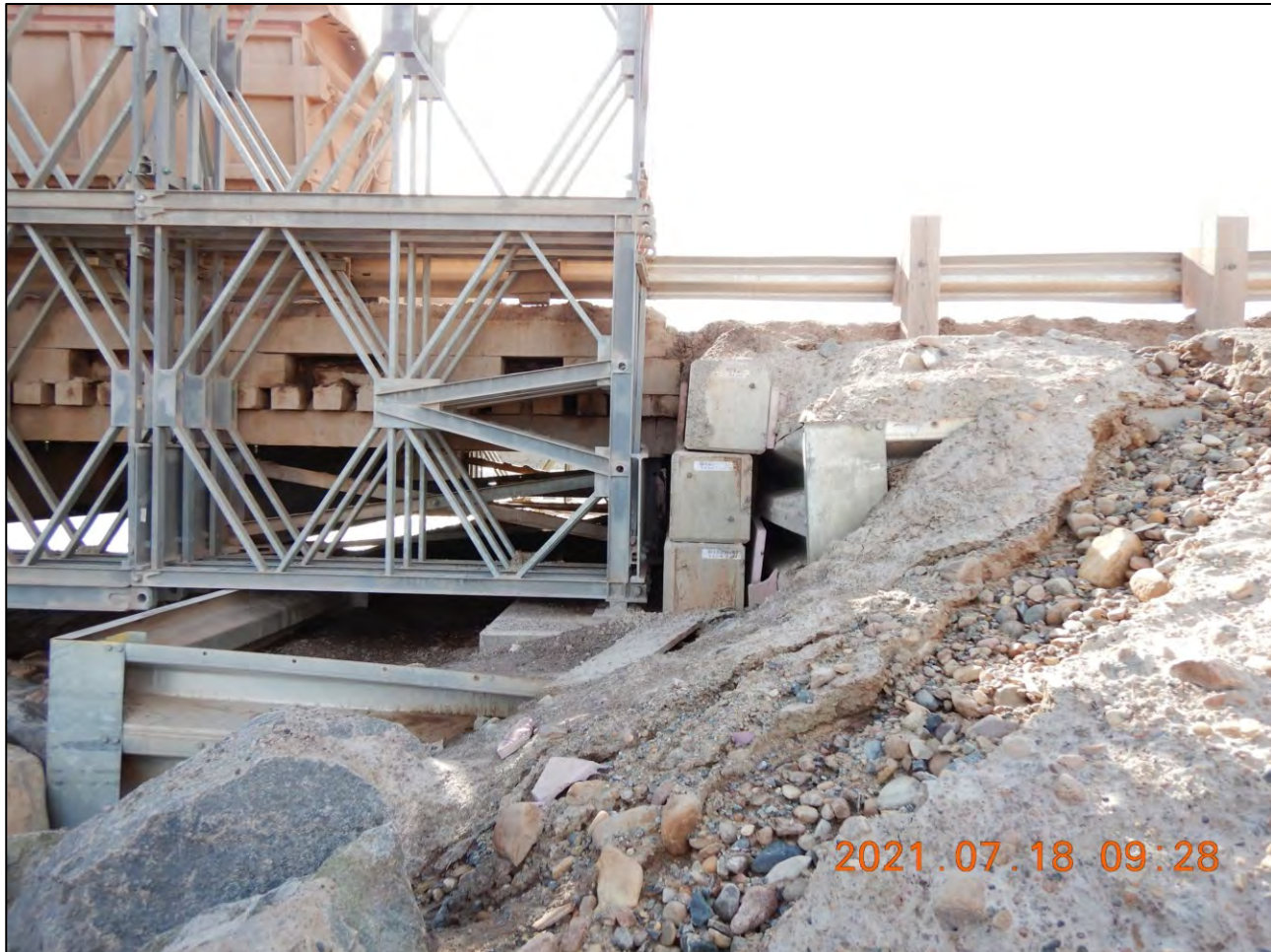
Photo 17. West bank foundation of KM97 bridge. Concrete blocks appear misaligned.
