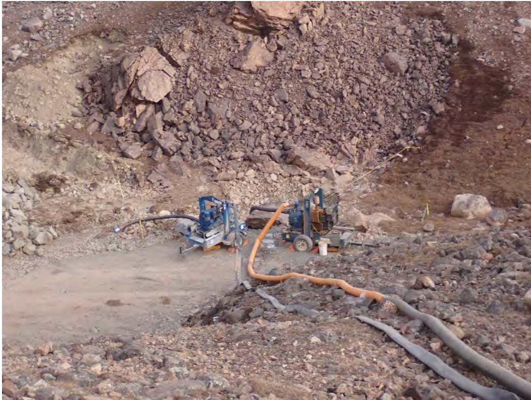
Photo 19 – Pumps at KM105 Dam Construction diverting water around active area
