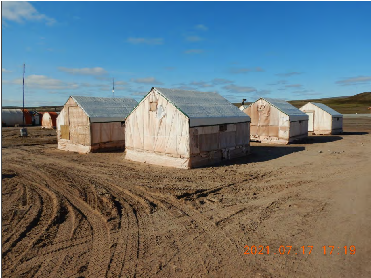
Photo 13. Deteriorating Weatherhaven facilities. Exposed insulation damaged by wind.
