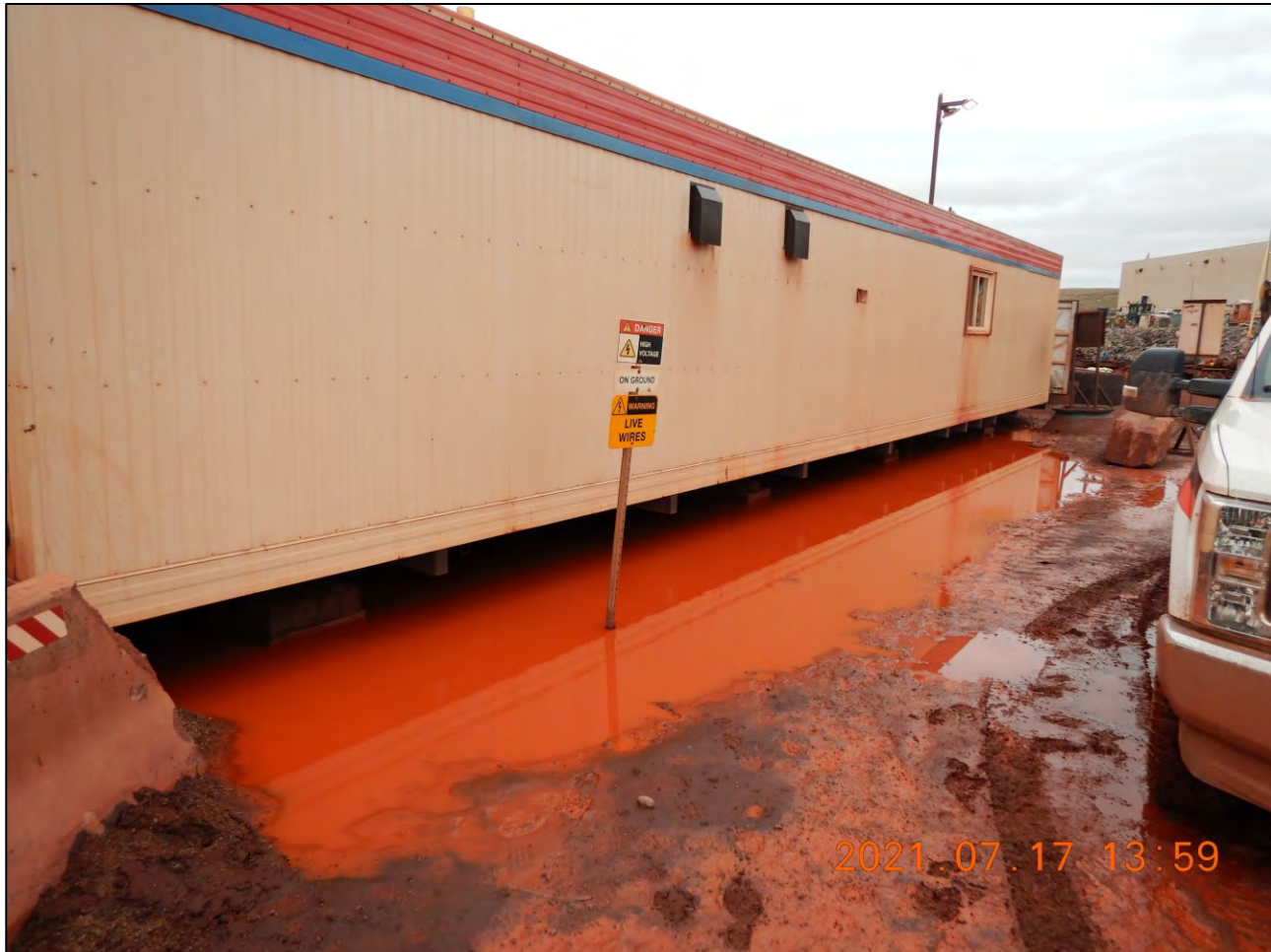
Photo 30. Muster station building inundated by contact water. Approximately 6in deep. Live wires running through contact water.
