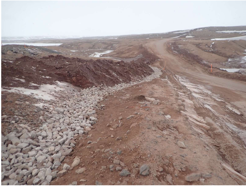
Photo 3. BG-01 Downstream Ditch Riprap Armouring (May 13, 2021)
