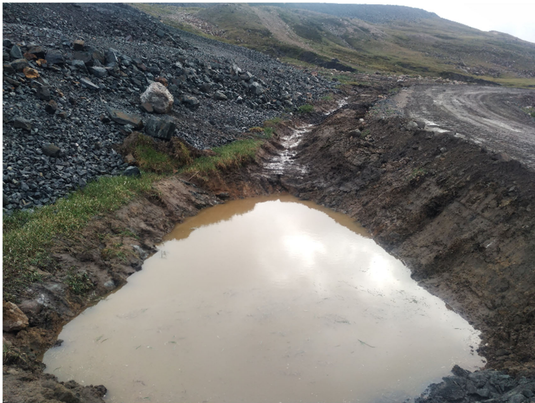
Photo 4. Enhanced sump at MS-106OS-02 spill location on July 27, 2021
