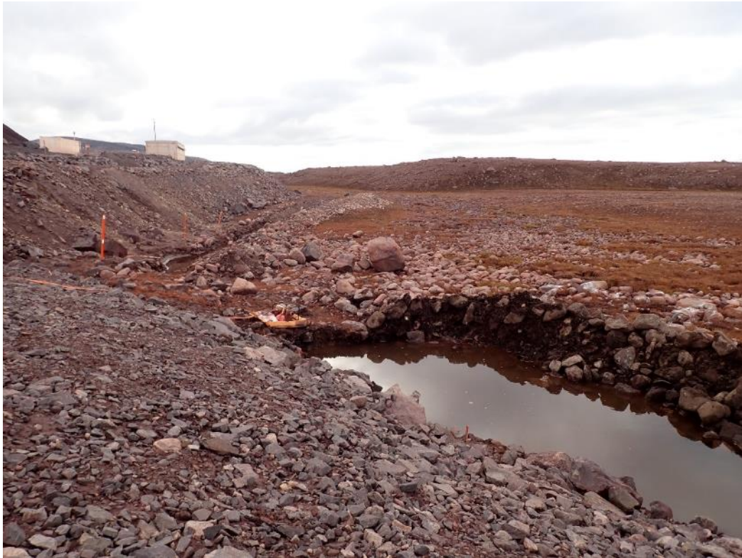
Photo 5. New sump pictured beside the existing emergency sump
