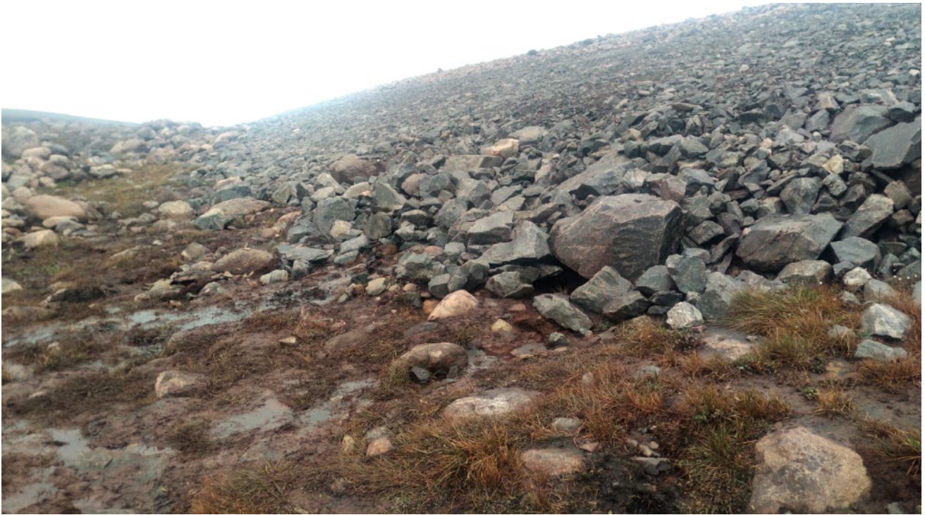
Photo 1. Seepage from toe of Crusher Facility Pond MS-06 on July 27, 2021
