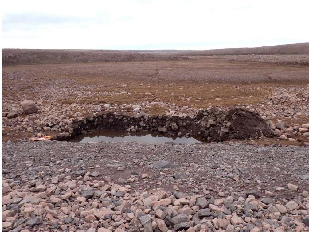
Photo 4. New emergency sump constructed down gradient of the seepage locations
