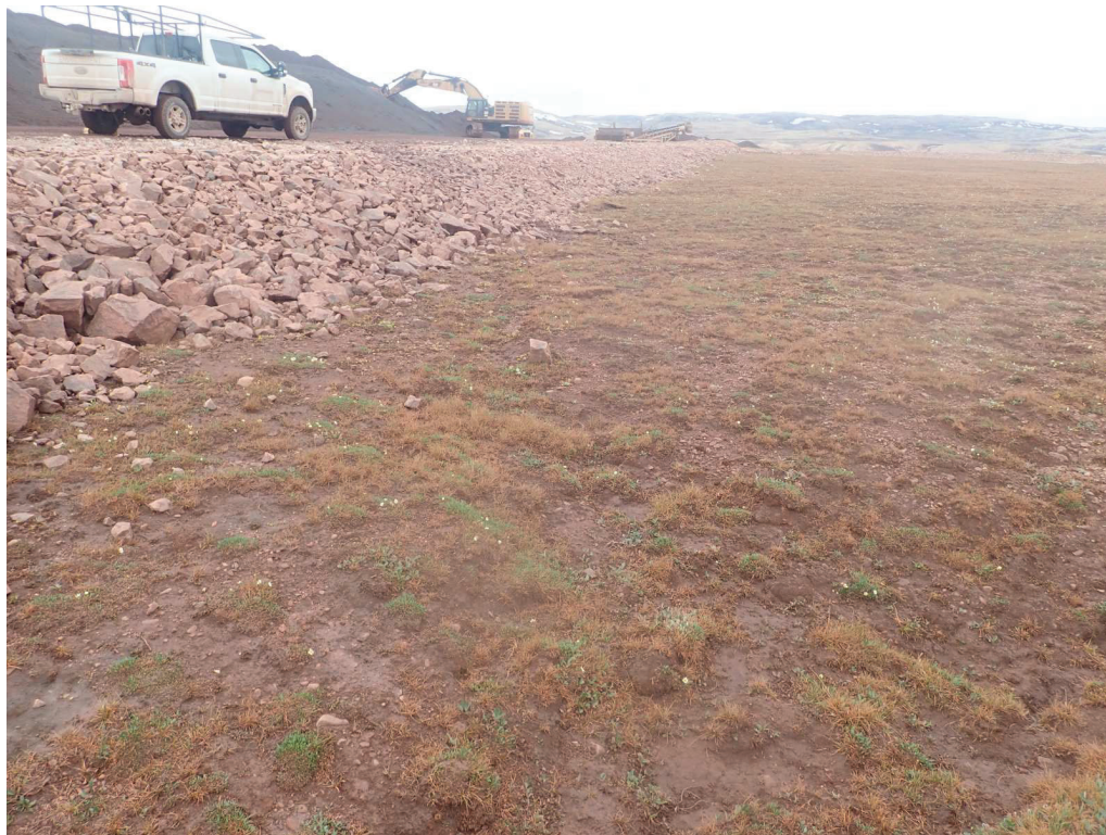
Photo 4. Tundra Down-Gradient of West Ore Pad Ditch Seepage Location (July 3, 2021)
