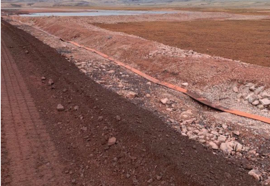
Photo 5. Modified Pond-to-Pond Transfer Process Configuration through Pipe, and Temporary Diversion Berm Preventing Ore Pad Runoff Water from Reporting to West Ore Pad Ditch (August 2, 2021)
