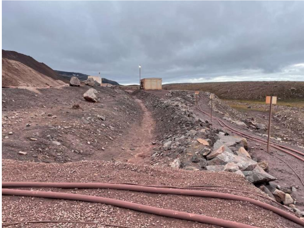
Photo 3. Crusher Facility Pond MS-06 south ditch showing dry conditions within ditch
