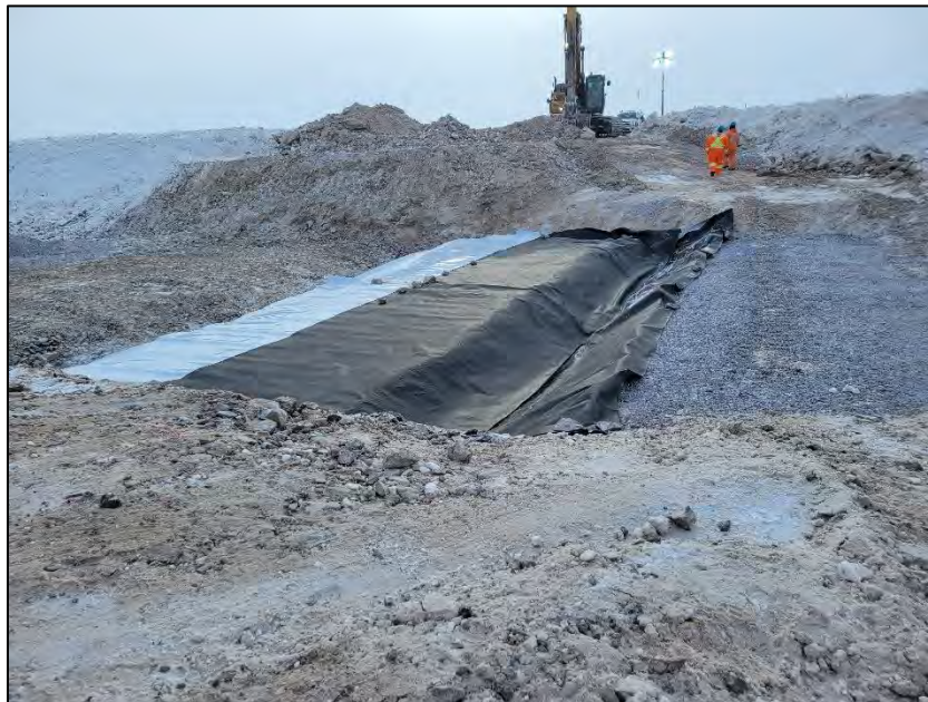
PHOTO 12. During Construction - Vantage Point 4 - Placement of Geomembrane and Geogrid Liner - Upstream Inlet - Looking Northeast (April 20, 2024).
