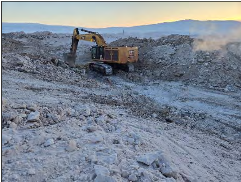
PHOTO 6. During Construction - Vantage Point 4 - Excavation of Blasted Material on Road Crossing - Looking Northeast (March 25, 2024).
