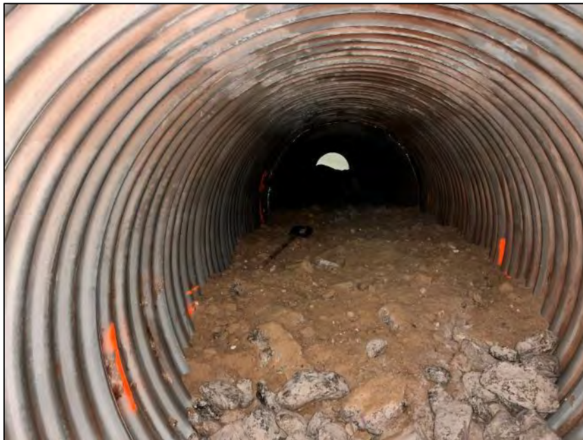
PHOTO 18. During Construction - Placement of Coarse Riprap and Stream Substrate Material in Low Flow Culverts - Looking North (April 06, 2024).
