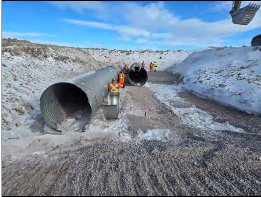
PHOTO 13. During Construction - Vantage Point 4 - Compaction of Culvert Backfill Under Road Crossing Around Low Flow Culverts - Looking North (March 31, 2024).
