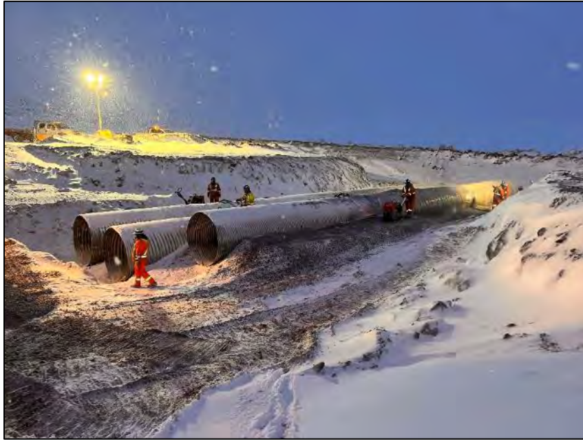
PHOTO 15. During Construction - Vantage Point 3 - Compaction of Culvert Backfill Material Around High Flow Culvert - Looking Northwest (April 01, 2024).
