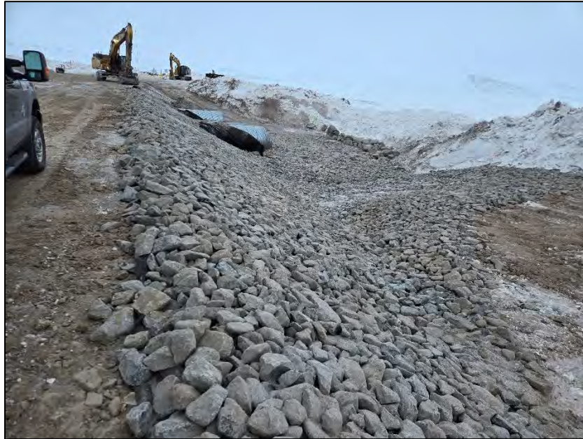
PHOTO 23. After Vantage Point 2 - Completed Downstream Outlet Apron and Slope Stabilization - Downstream Outlet Area - Looking North (May 03, 2024).
