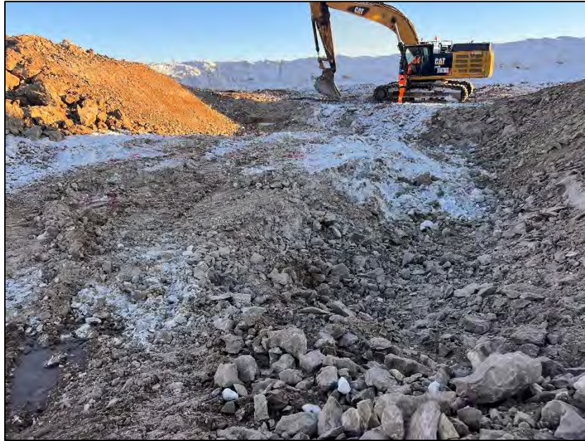
PHOTO 7. During Construction - Vantage Point 3 - Blast Excavation - Road Crossing and Downstream Outlet - Looking North (April 17, 2024).
