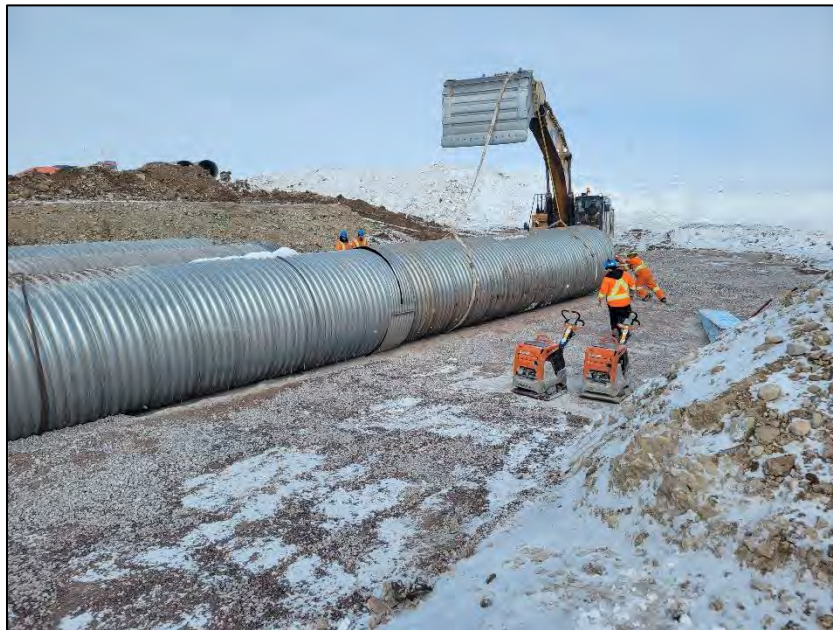
PHOTO 14. During Construction - Vantage Point 3 - Installation of 2.0 m diameter corrugated steel pipe low flow culvert - Looking North (April 23, 2024).
