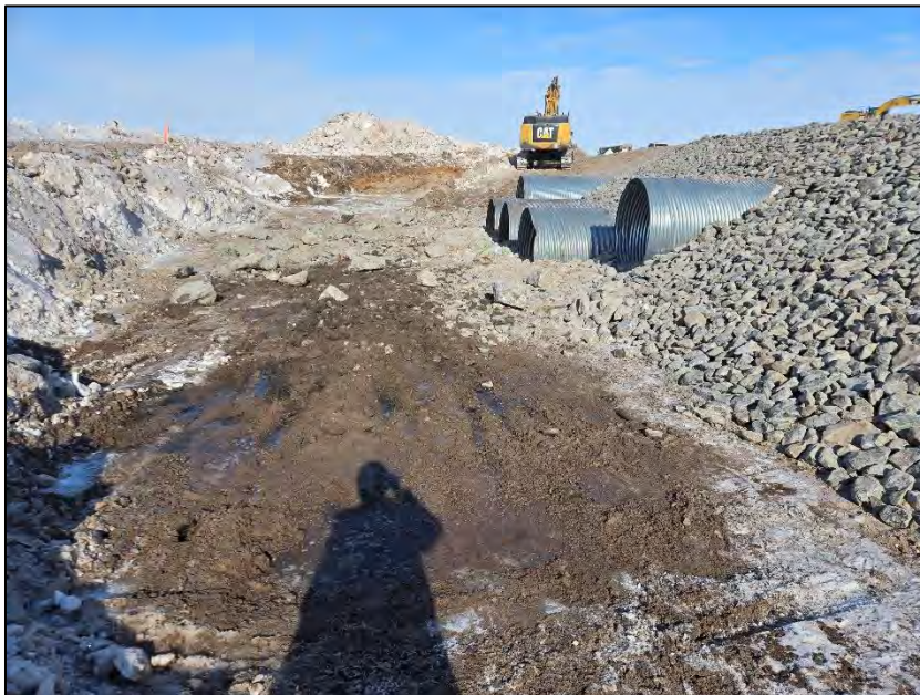
PHOTO 22. Following Construction - Vantage Point 3 - Completed south (inlet) apron with Coarse Riprap and Stream Substrate Material - Looking Northwest (May 04, 2024).
