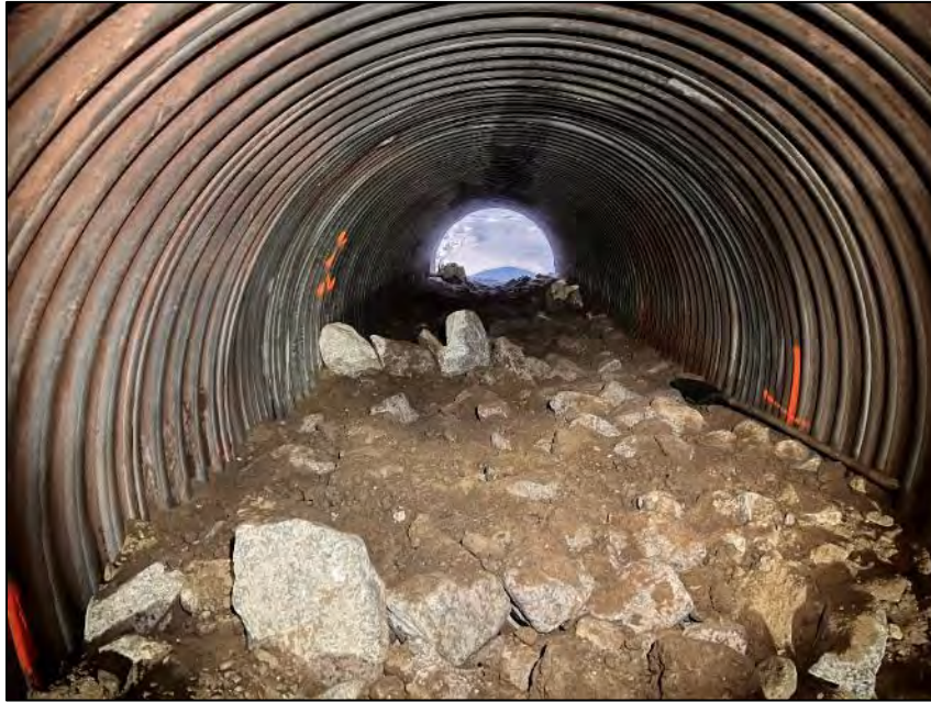
PHOTO 17. During Construction - Placement of Boulder Clusters in Low Flow Culverts - Looking North (April 03, 2024).
