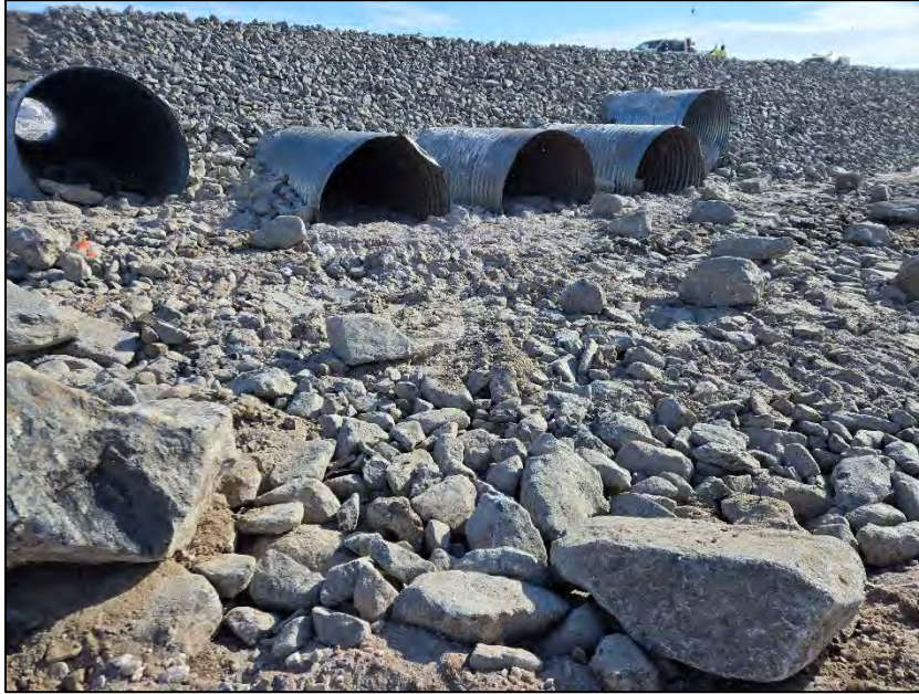
PHOTO 21. Following Construction - Vantage Point 2 - Completed north (outlet) apron with Coarse Riprap and Stream Substrate Material - Looking Northwest (May 04, 2024).
