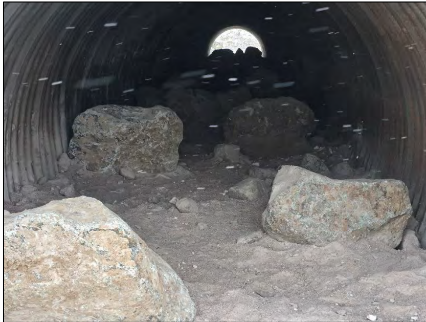
PHOTO 25. Following Construction - Completed placement of boulder clusters and coarse riprap and stream substrate material within the interior of the low flow culvert (May 03, 2024).
