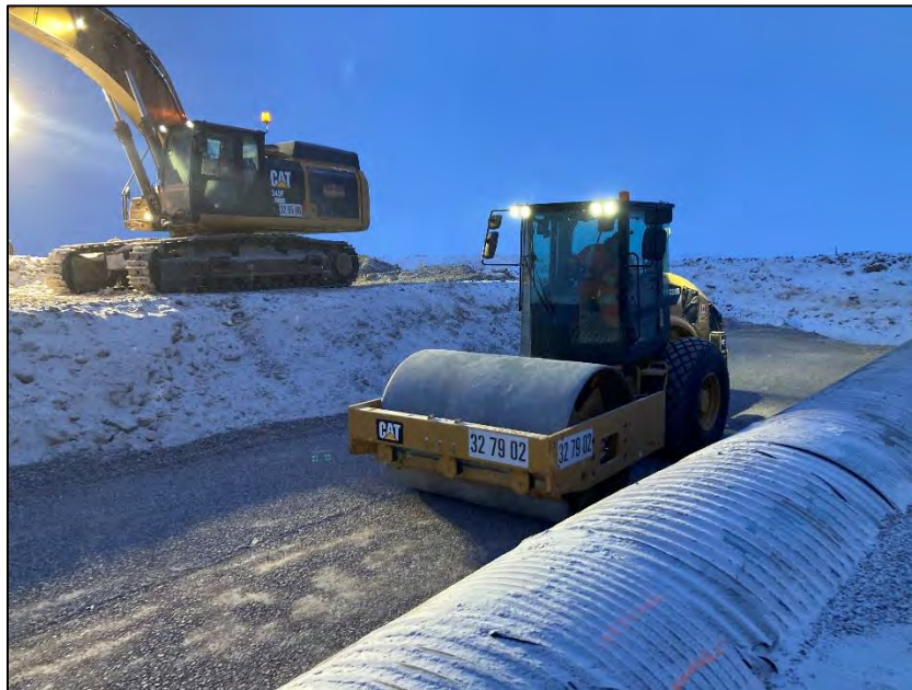
PHOTO 16. During Construction - Vantage Point 3 - Compaction of Culvert Backfill Material - Looking North (April 25, 2024).
