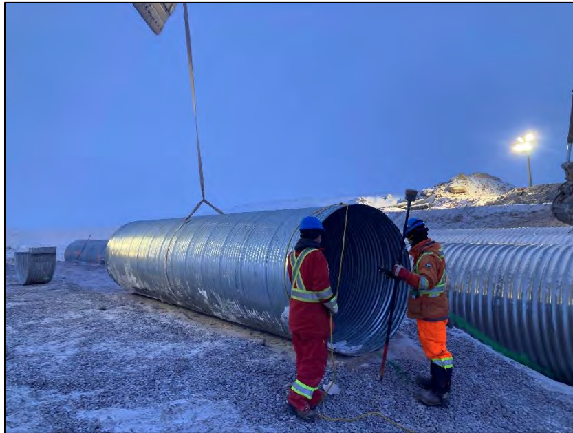
PHOTO 17. During Construction - Vantage Point 3 - Placement of segment of 1.8 m diameter corrugated steel pipe high flow culvert - Looking Northeast (April 25, 2024).
