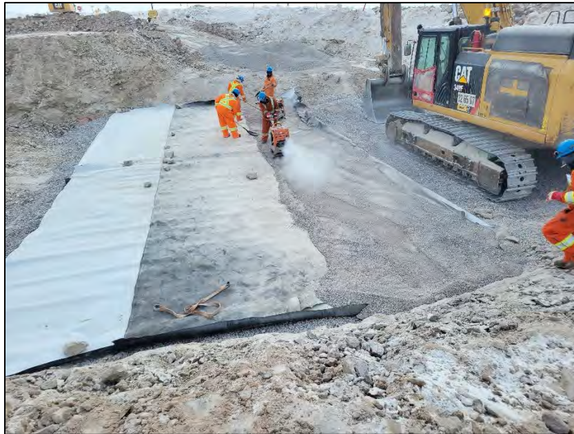
PHOTO 13. During Construction - Vantage Point 3 - Compaction of 3/4 inch Material in Plug Trench - Looking West (April 20, 2024).
