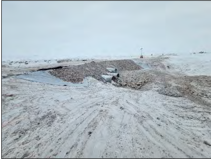
PHOTO 21. During Construction - Vantage Point 2 - Placement of Coarse Riprap and Stream Substrate Material in Upstream Inlet - Looking West (April 11, 2024).
