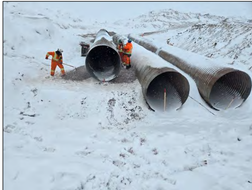
PHOTO 14. During Construction - Vantage Point 4 - Placement of 1.8 m Diameter Corrugated Steel High Flow Culvert - Looking South (April 01, 2024).
