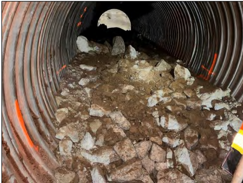
PHOTO 16. During Construction - Placement of Coarse Riprap and Stream Substrate Material in Low Flow Culverts - Looking North (April 03, 2024).
