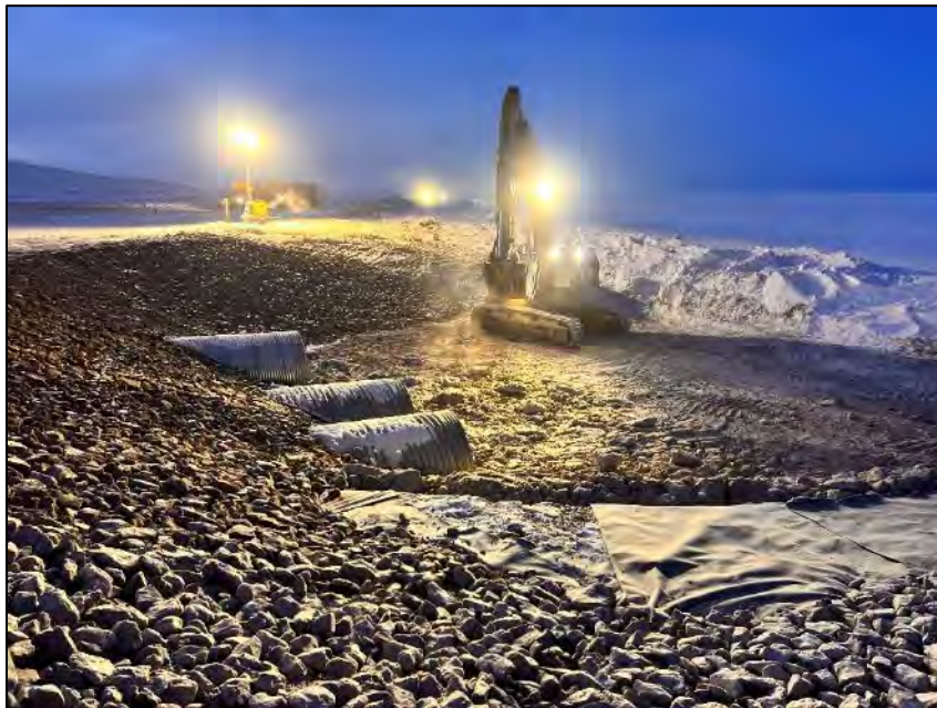
PHOTO 20. During Construction - Vantage Point 4 - Completed Downstream Outlet and Slope Stabilization - Looking Southeast (April 11, 2024).
