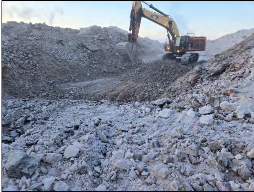
PHOTO 7. During Construction - Vantage Point 3 - Excavation of Blasted Material in Upstream Inlet and Road Crossing - Looking South (March 25, 2024).
