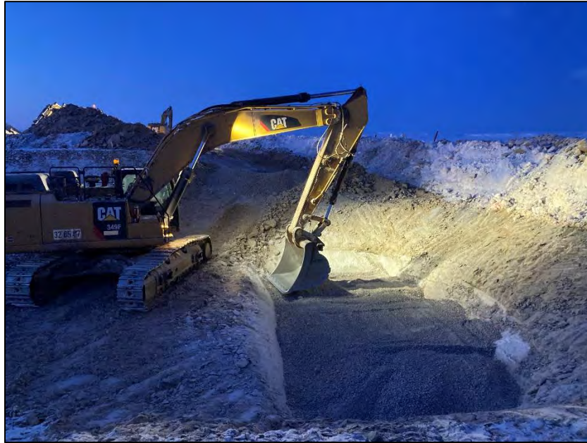
PHOTO 9. During Construction - Vantage Point 4 - Compaction of Culvert Backfill Material - Upstream inlet - Looking East (April 18, 2024).
