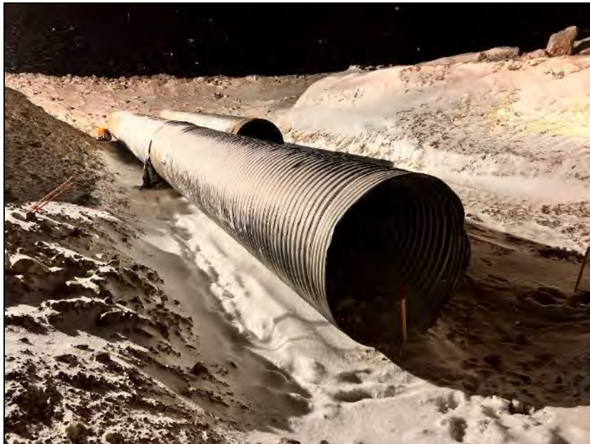
PHOTO 12. During Construction - Vantage Point 4 - Placement of 2.0 m Diameter Corrugated Steel Low Flow Culverts - Looking Northeast (March 30, 2024).
