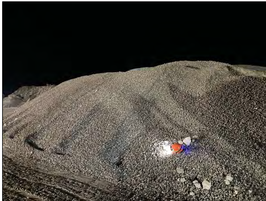
PHOTO 26. Material Stockpile - 32 mm minus Culvert Backfill Material - km 60 Laydown - Looking Northeast (March 10, 2024).
