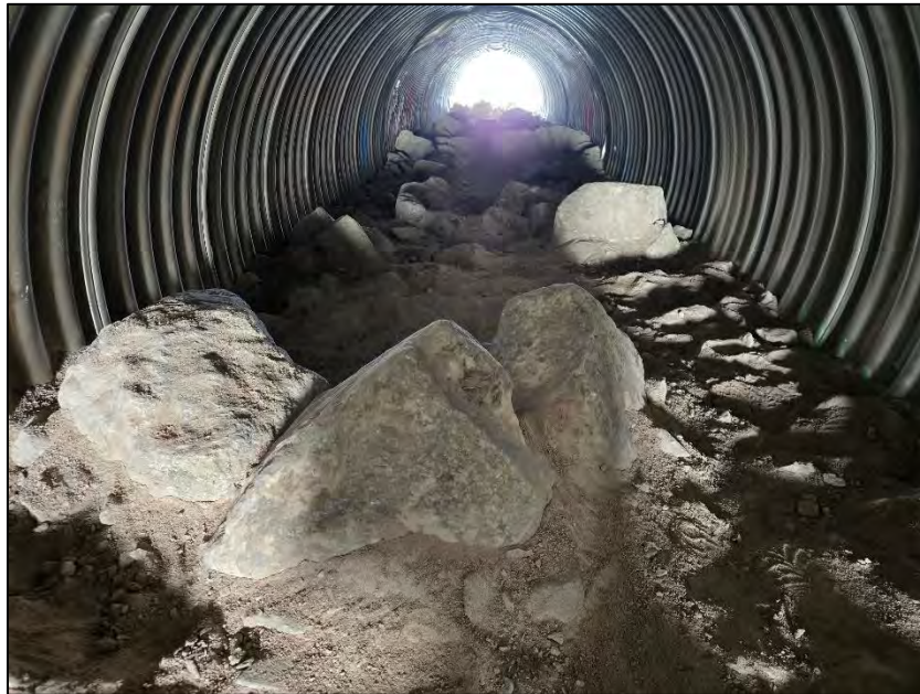
PHOTO 19. During Construction - Placement of Boulder Clusters in Low Flow Culvert - Looking North (May 01, 2024).
