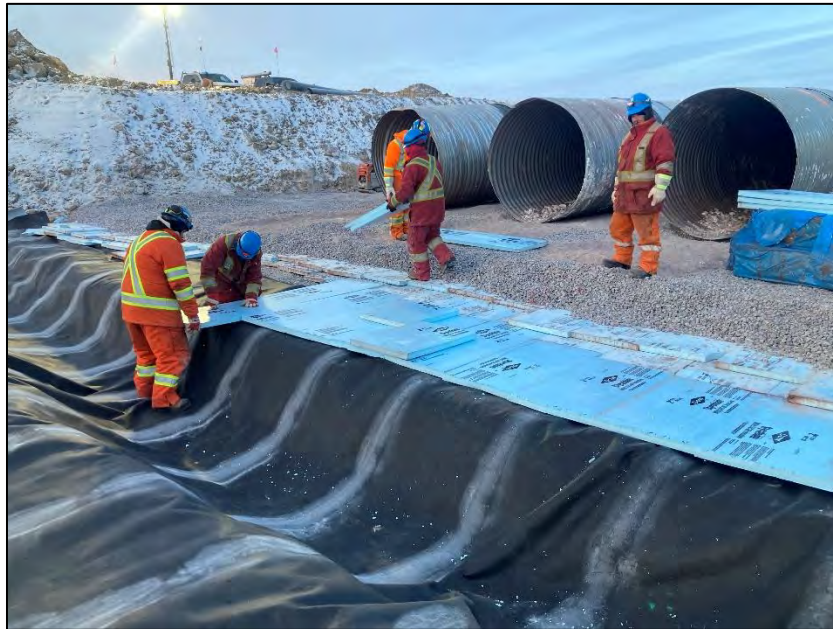
PHOTO 15. During Construction - Vantage Point 1 - Placement of Insulation - Road Crossing - Looking Northeast (April 23, 2024).
