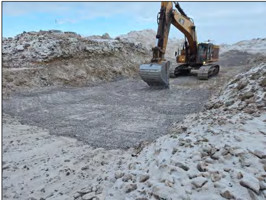
PHOTO 10. During Construction - Vantage Point 3 - Placement of Culvert Backfill Material Under Road Crossing and Downstream Outlet - Looking Northwest (March 28, 2024).
