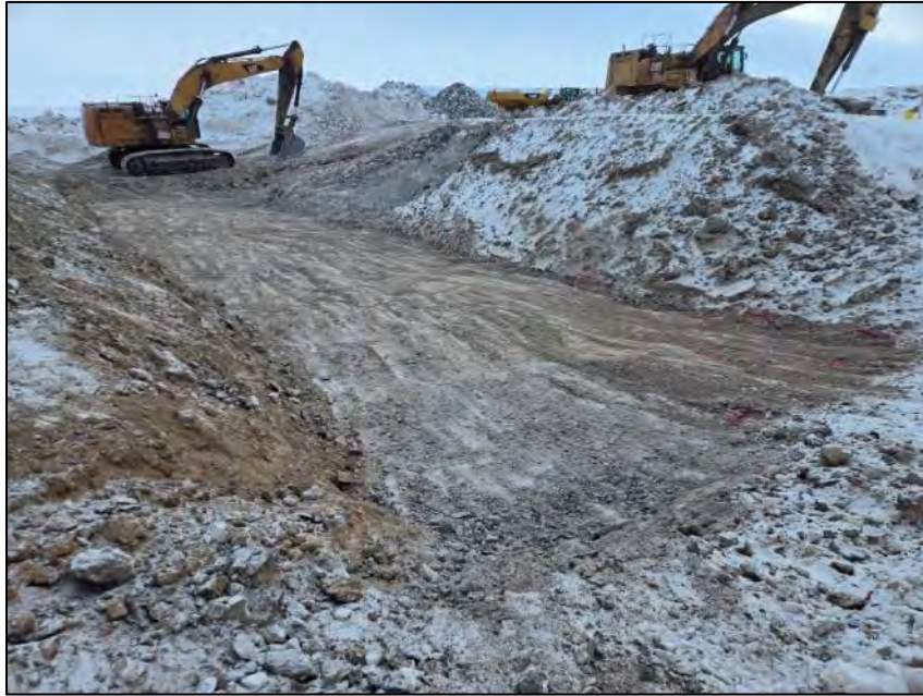
PHOTO 9. During Construction - Vantage Point 2 - Preparation of Foundation Surface Under Road Crossing and Inlet and Outlet - Looking Southwest (March 28, 2024).
