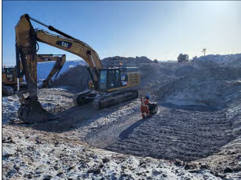
PHOTO 10. During Construction - Vantage Point 4 - Placement and Compaction of Culvert Backfill Material - Upstream inlet - Looking Northeast (April 19, 2024).
