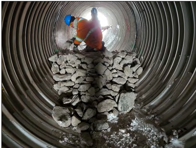
PHOTO 20. During Construction - Placement of Coarse Riprap and Stream Substrate Material in Low Flow Culvert - Looking South (May 02, 2024).
