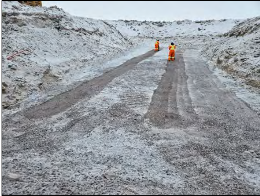
PHOTO 11. During Construction - Vantage Point 3 - Compaction of Culvert Backfill Material Under Road Crossing and Upstream Inlet - Looking North (March 29, 2024).
