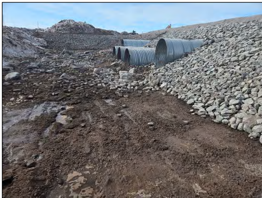
PHOTO 24. Following Construction - Vantage Point 3 - Completed Upstream Inlet Apron and Slope Stabilization -Upstream Inlet Area - Looking North (April 5, 2024).
