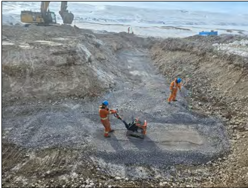
PHOTO 11. During Construction - Vantage Point 2 - Compaction of Culvert Backfill Material - Looking Northwest (May 05, 2024).
