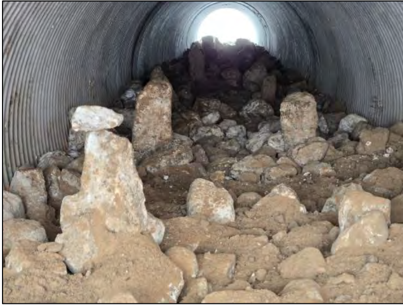
PHOTO 19. Following Construction - Completed placement of coarse riprap and stream substrate material within the interior of the low flow CSP culvert at CV-001 (April 1, 2024).
