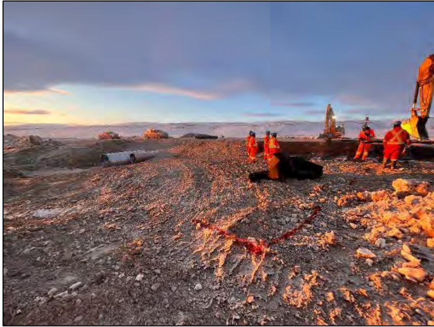
PHOTO 25. During Construction - Vantage Point 3 - Installation of Geotextile for Slope Stabilization - Looking Northeast (May 09, 2024).
