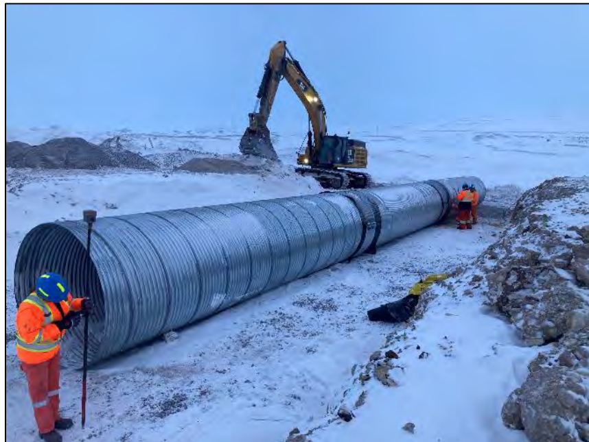
PHOTO 18. During Construction- Vantage Point 3 - Installation of 2.0 m diameter low flow culvert - Looking Northeast (April 29, 2024).
