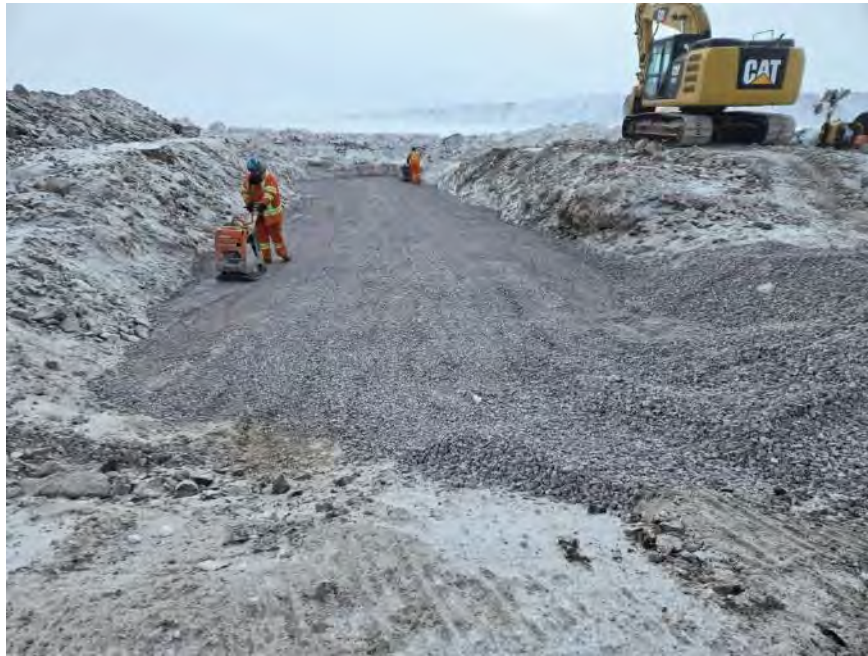
PHOTO 7. During Construction - Vantage Point 1 - Compaction of culvert backfill material - Road crossing and upstream inlet - Looking South (March 27, 2024).
