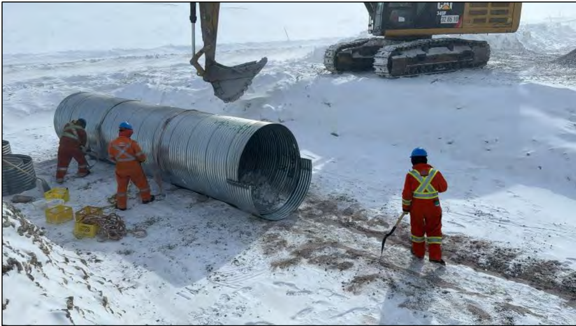
PHOTO 17. During Construction - Vantage Point 4 - Installation of 2.0 m diameter low flow culvert - Looking Southeast (April 29, 2024).
