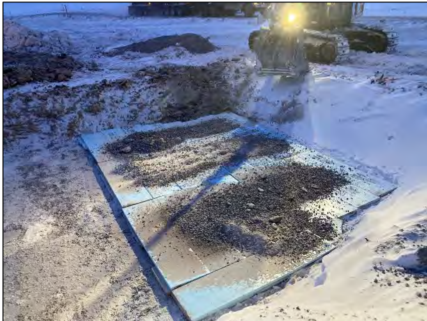
PHOTO 14. During Construction - Vantage Point 1 - Placement of Styrofoam Insulation in downstream end of crossing - Looking Southwest (April 26, 2024).
