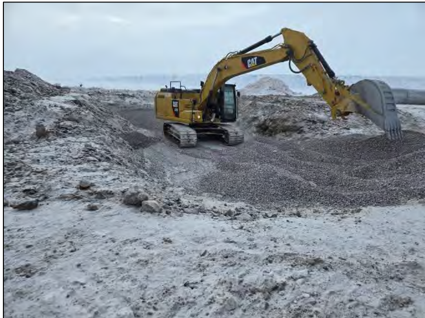
PHOTO 6. During Construction - Vantage Point 2 - Placement of culvert backfill - Road crossing and upstream inlet - Looking South (March 27, 2024).
