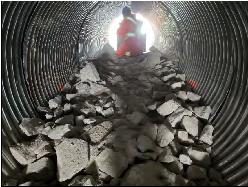
PHOTO 27. During Construction - Riprap and Stream Substrate Material placement in low flow culvert - Looking East (May 12, 2024).
