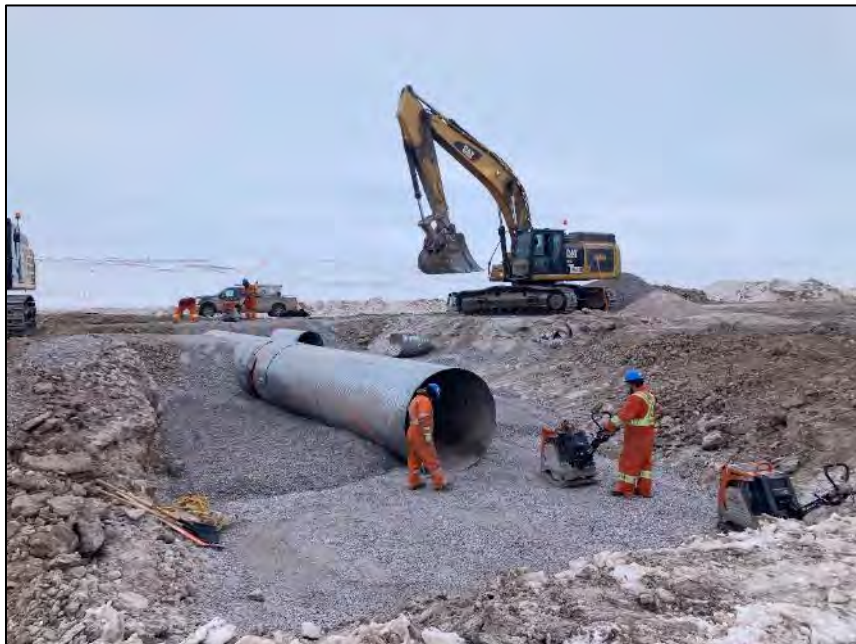
PHOTO 24. During Construction - Vantage Point 4 - Compaction of Culvert Backfill Material around Culverts - Looking Southeast (May 06, 2024).
