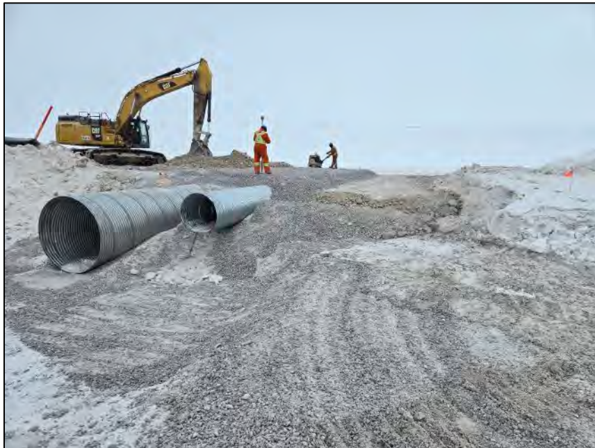
PHOTO 22. During Construction - Vantage Point 3 - Compaction of Culvert Backfill Material above high and low flow culverts - Looking Northeast (April 31, 2024).
