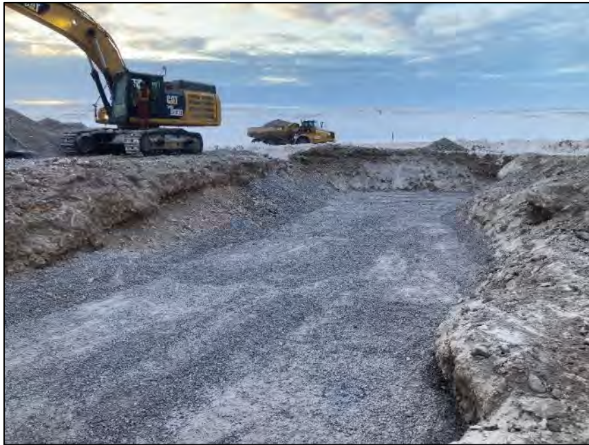
PHOTO 13. During Construction - Vantage Point 3 - Compacted Culvert Backfill Material - Looking Northeast (May 05, 2024).
