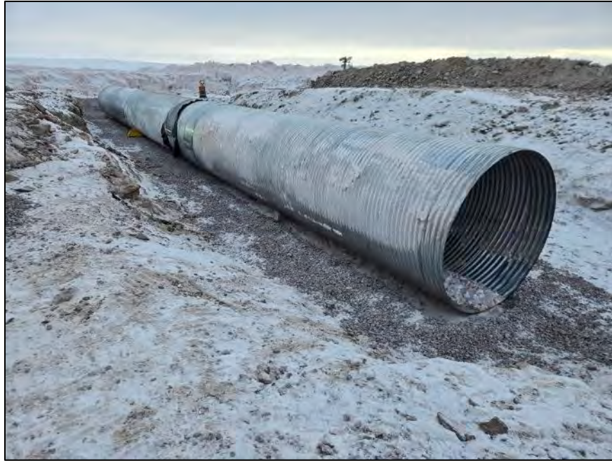
PHOTO 9. During Construction - Vantage Point 4 - Installation of 1.8 m diameter corrugated steel pipe low flow culvert - Road crossing and downstream outlet - Looking Northeast (March 28, 2024).
