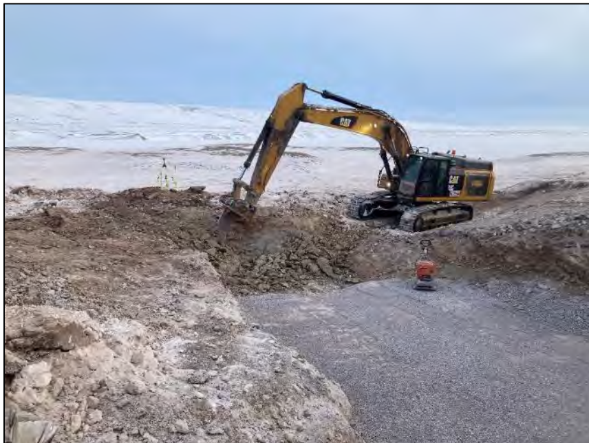
PHOTO 14. During Construction - Vantage Point 2 - Ripping of Outlet Apron - Looking Northeast (May 05, 2024).
