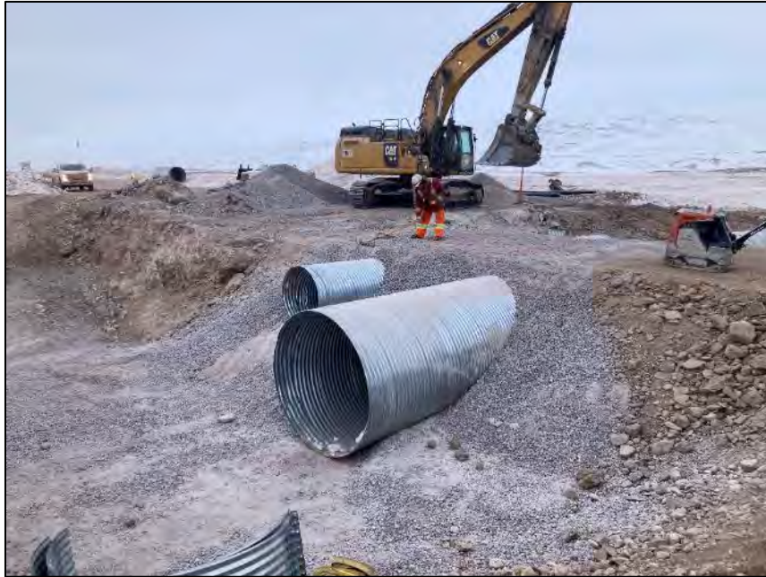
PHOTO 23. During Construction - Vantage Point 1 - Compaction of Culvert Backfill Material around Culverts - Looking Southwest (May 06, 2024).
