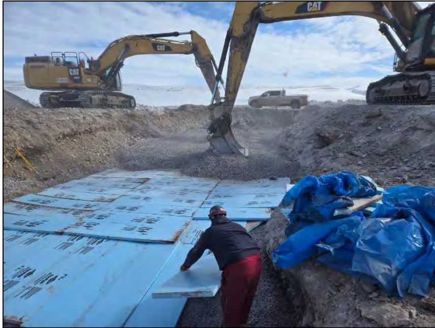
PHOTO 17. During Construction - Vantage Point 3 - Placement of Culvert Backfill Material and Installation of Styrofoam Insulation - Looking Northeast (May 06, 2024).
