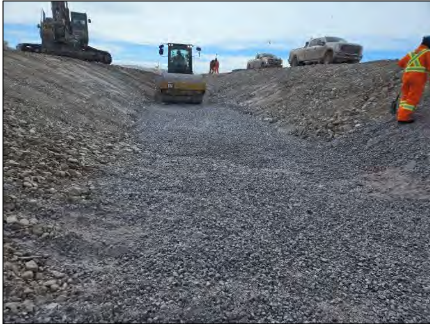
PHOTO 29. During Construction - Vantage Point 1 - Compaction of Culvert Backfill Material in Inlet Apron - Looking South (May 10, 2024).
