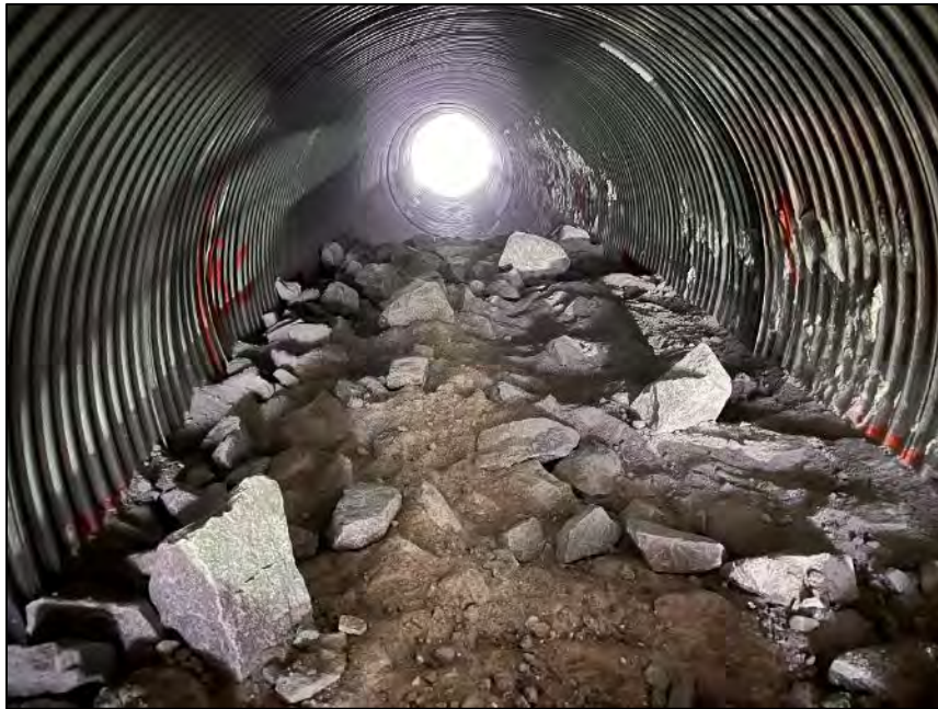
PHOTO 27. During Construction - Culvert Infill in Low Flow Culvert - Looking West (May 10, 2024).
