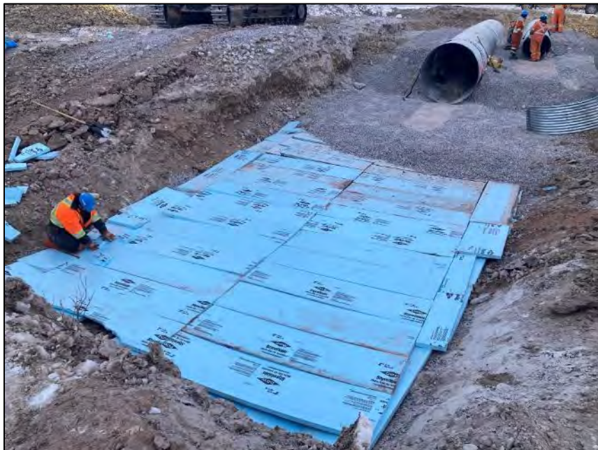
PHOTO 22. During Construction - Vantage Point 3 - Installation of Styrofoam Insulation - Looking Northeast (May 06, 2024).
