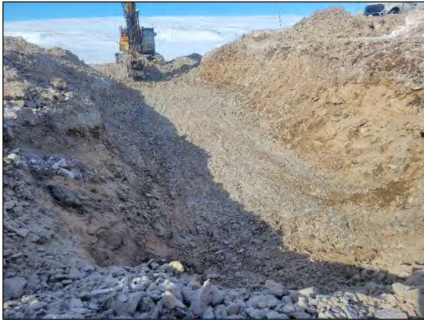
PHOTO 7. During Construction - Vantage Point 4 - Blast Excavation - Road Crossing and Upstream Inlet - Looking Northwest (April 24, 2024).
