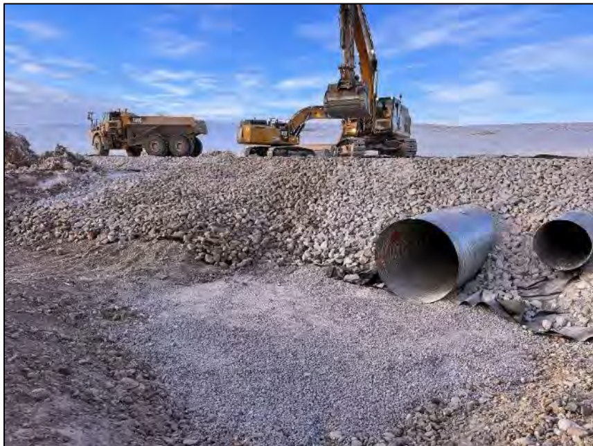
PHOTO 30. During Construction - Vantage Point 3 - Placement of Riprap for Slope Stabilization - Looking Northeast (May 10, 2024).
