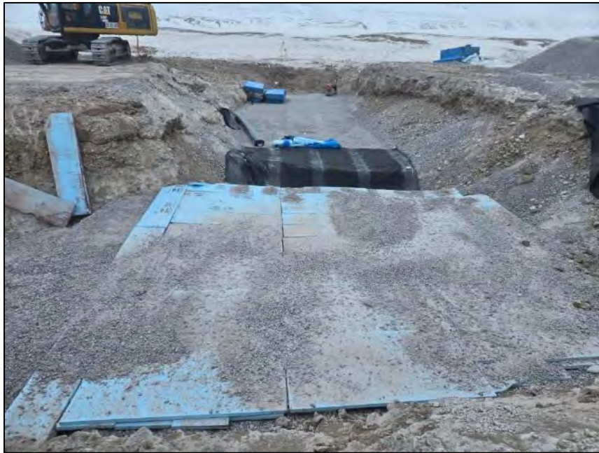
PHOTO 15. During Construction - Vantage Point 2 - Installation of Geotextile and Geomembrane Anchor Trench and Styrofoam - Looking Northwest (May 06, 2024).
