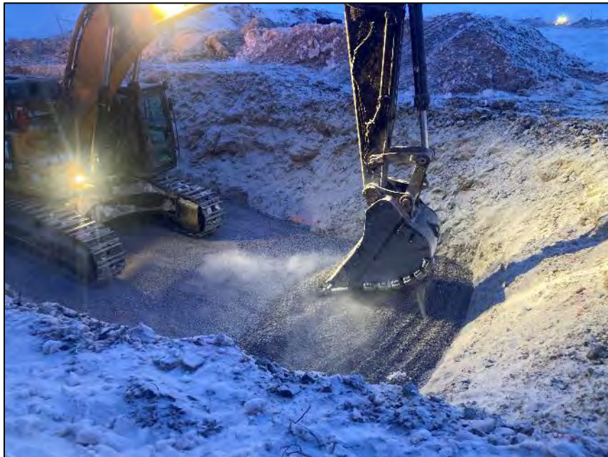
PHOTO 10. During Construction - Vantage Point 4 - Placement of Culvert Backfill Material - Road Crossing and downstream outlet - Looking Southeast (April 24, 2024).
