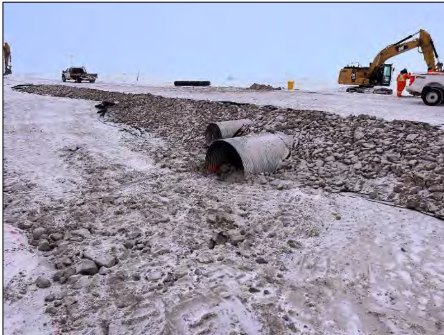
PHOTO 14. During Construction - Vantage Point 1 - Placement of geotextile and riprap on the north side slope at CV-001 - Road crossing and upstream inlet - Looking South (March 30, 2024).
