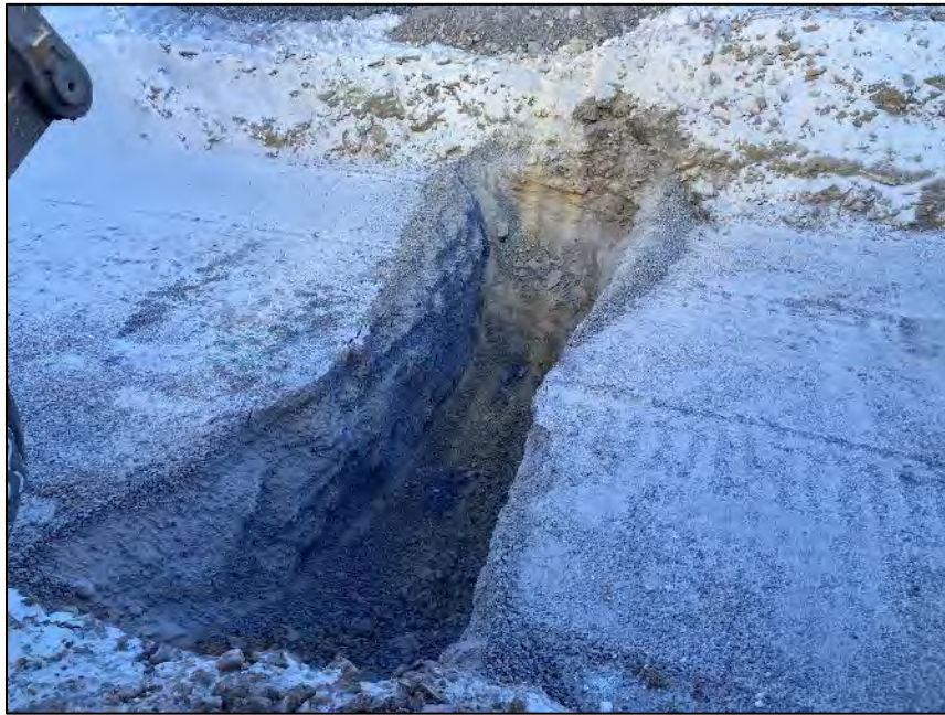
PHOTO 11. During Construction - Vantage Point 4 - Excavation of key-in trench in downstream end of crossing - Looking Southeast (April 25, 2024).
