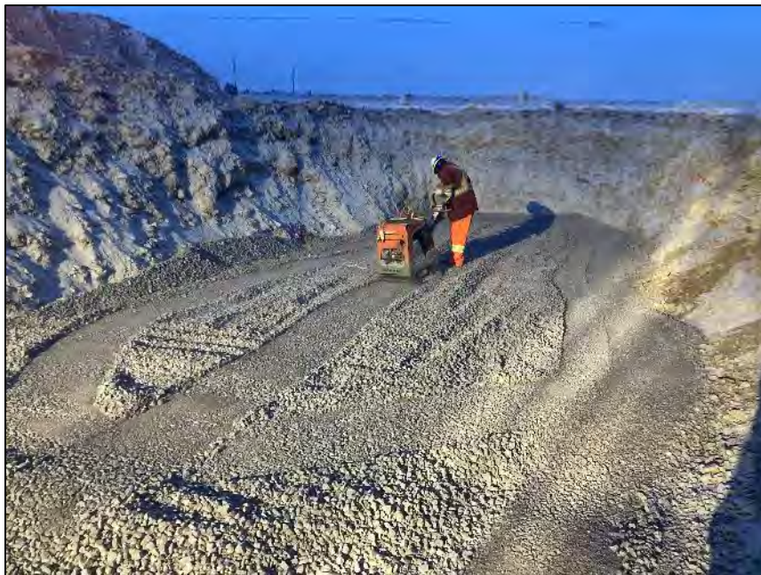
PHOTO 8. During Construction- Vantage Point 1 - Compaction of Culvert Backfill Material - Upstream inlet - Looking Southwest (April 24, 2024).
