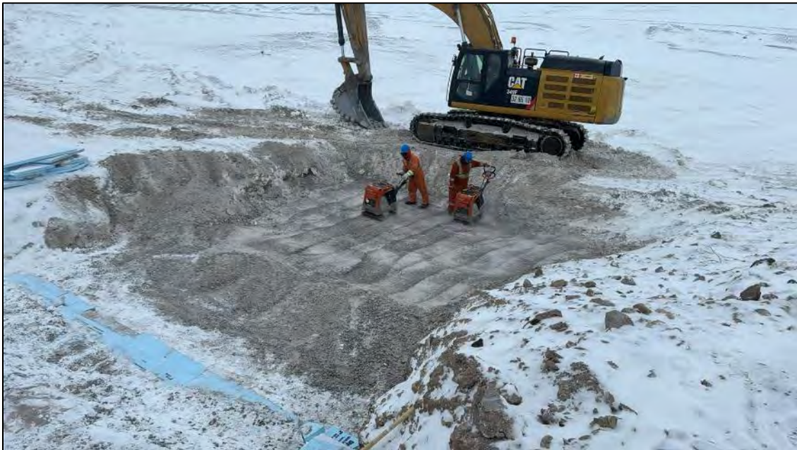
PHOTO 16. During Construction - Vantage Point 3 - Compaction of Culvert Backfill Material in upstream inlet area - Looking Northeast (April 29, 2024).
