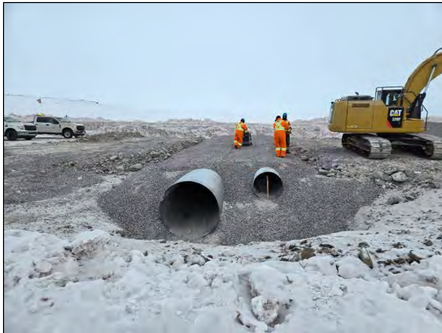
PHOTO 12. During Construction - Vantage Point 1 - Placement of culvert backfill material above the low and high flow CSP culverts - Road crossing and upstream inlet - Looking South (March 30, 2024).
