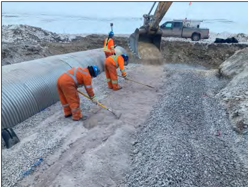
PHOTO 20. During Construction - Vantage Point 3 - Placement and Grading of Culvert Bedding Material - Looking Northeast (May 06, 2024).
