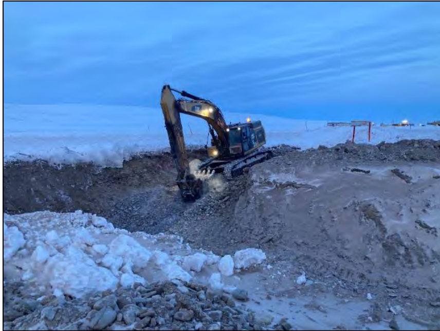
PHOTO 9. During Construction - Vantage Point 1 - Excavation of Unsuitable Material from Inlet Apron - Looking South (May 04, 2024).
