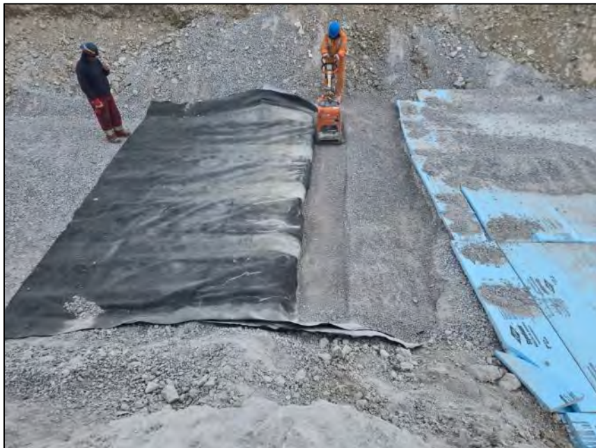
PHOTO 16. During Construction - Vantage Point 2 - Compaction of Culvert Backfill Material in Anchor Trench - Looking North (May 06, 2024).
