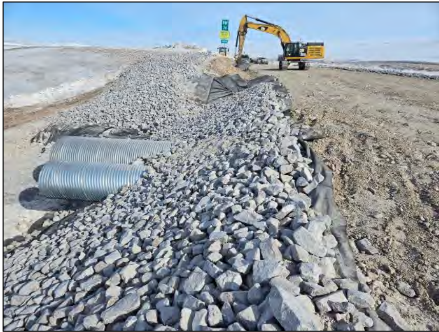
PHOTO 25. During Construction - Vantage Point 3 - Installation of geotextile and riprap placement on outlet side of crossing - Looking Northeast (May 05, 2024).
