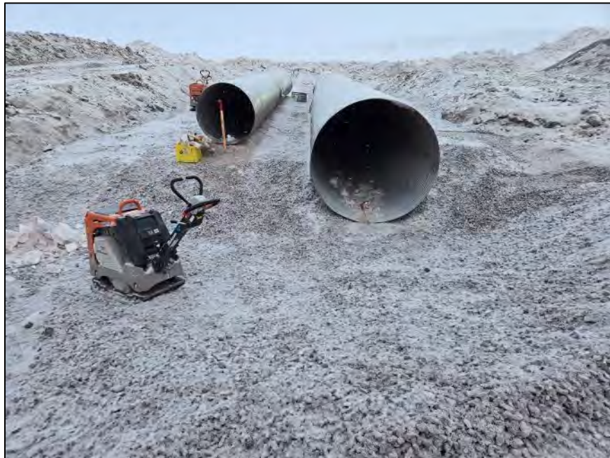
PHOTO 10. During Construction - Vantage Point 1 - Installation of 1.0 m diameter corrugated steel pipe high flow culvert - Road crossing and upstream inlet - Looking South (March 29, 2024).
