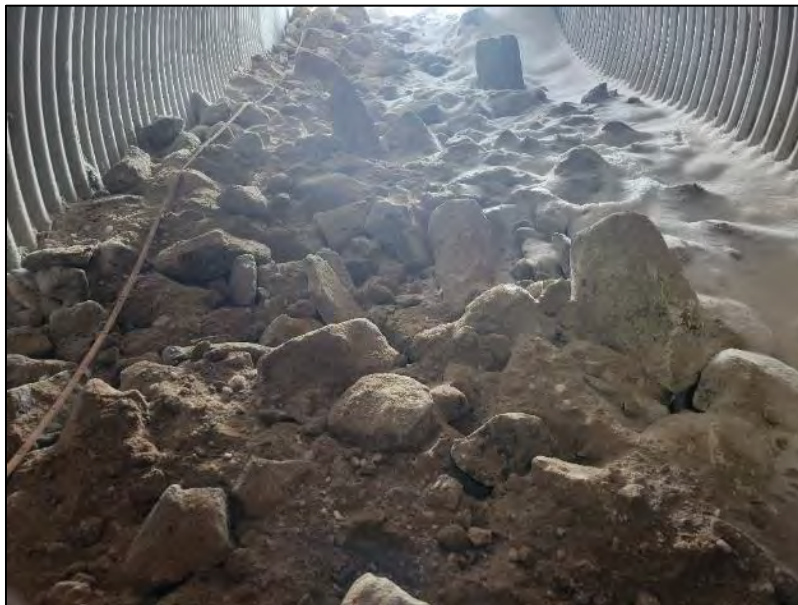
PHOTO 20. Following Construction - Completed placement of coarse riprap and stream substrate material within the interior of the low flow CSP culvert at CV-001 (April 16, 2024).
