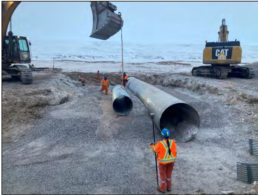
PHOTO 21. During Construction - Vantage Point 2 - Installation of High Flow Culvert - Looking Northeast (May 06, 2024).
