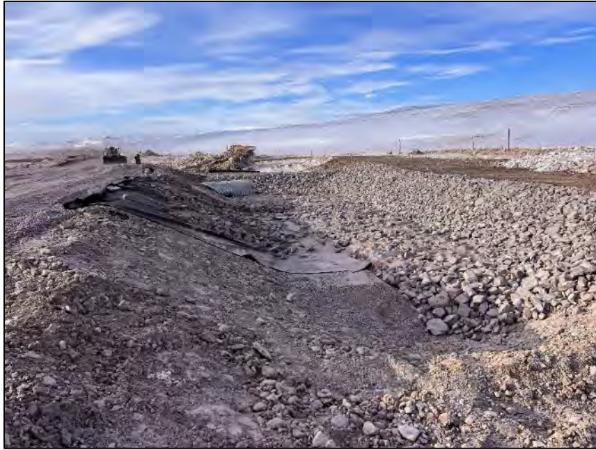
PHOTO 31. During Construction - Vantage Point 2 - Placement of Coarse Riprap and Stream Substrate Material in Inlet Apron - Looking North (May 11, 2024).
