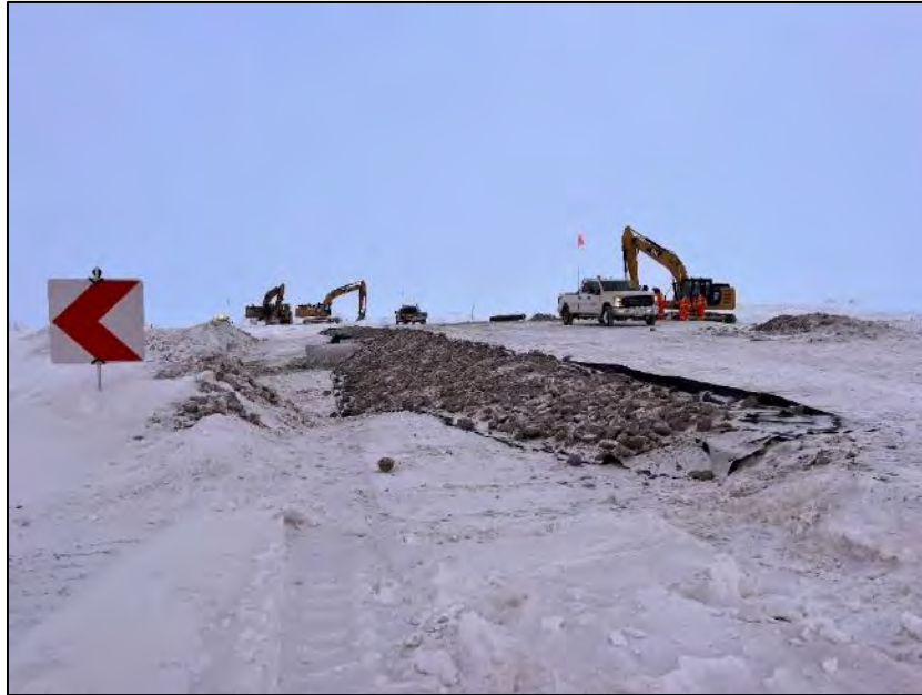
PHOTO 13. During Construction - Vantage Point 1 - Placement of geotextile on the north slope at CV-001 - Road crossing and upstream inlet - Looking South (April 5, 2024).
