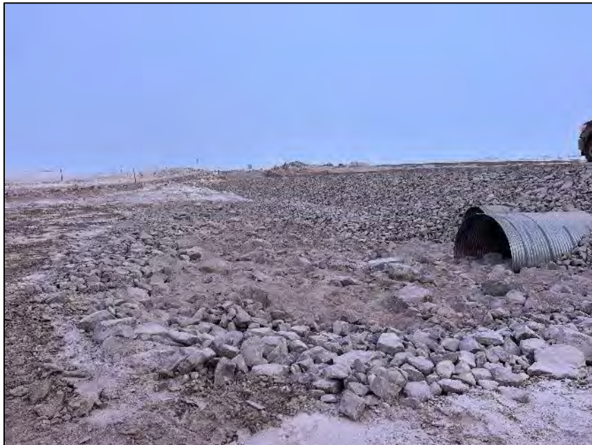
PHOTO 28. After Construction - Vantage Point 1 - Final arrangement of inlet apron - Looking Southeast (May 13, 2024).
