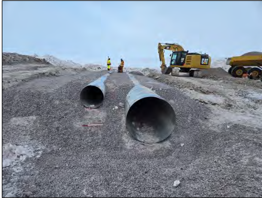
PHOTO 11. During Construction - Vantage Point 1 - Installation of 1.8 m diameter corrugated steel pipe low flow culvert and 1.0 m diameter corrugated steel pipe high flow culvert - Road crossing and upstream inlet - Looking South (March 30, 2024).
