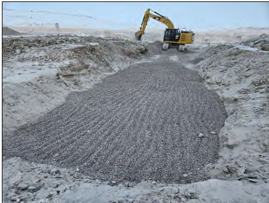
PHOTO 8. During Construction - Vantage Point 3 - Compaction of culvert backfill material - Road crossing and upstream inlet - Looking North (March 27, 2024).
