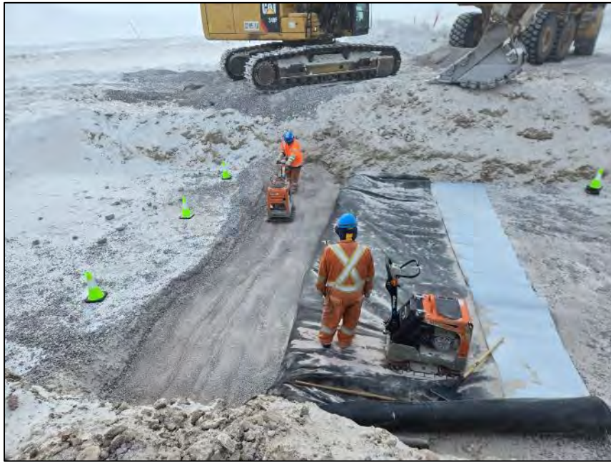
PHOTO 13. During Construction - Vantage Point 2 - Compaction of 3/4 inch minus Material in key-in trench in downstream end of crossing - Looking Northwest (April 26, 2024).
