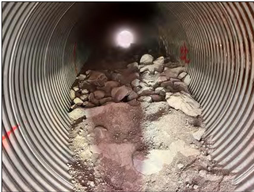
PHOTO 28. During Construction - Culvert Infill in Low Flow Culvert - Looking East (May 10, 2024).
