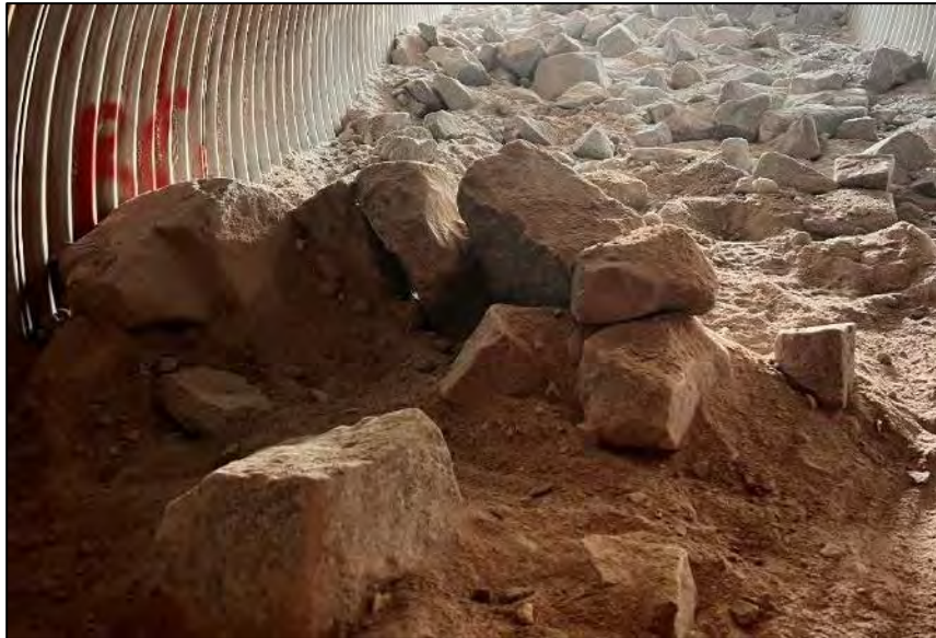
PHOTO 32. During Construction - Completed Boulder Cluster in Low Flow Culvert - Looking West (May 11, 2024).
