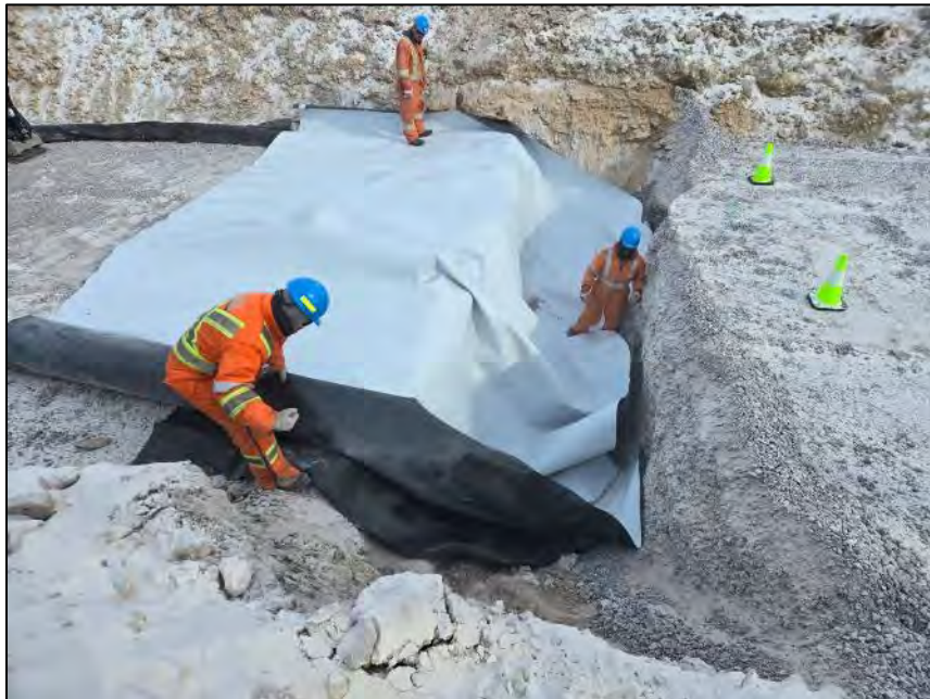
PHOTO 12. During Construction - Vantage Point 4 - Installation of geotextile and geomembrane in key-in trench in downstream end of crossing - Looking Southeast (April 26, 2024).
