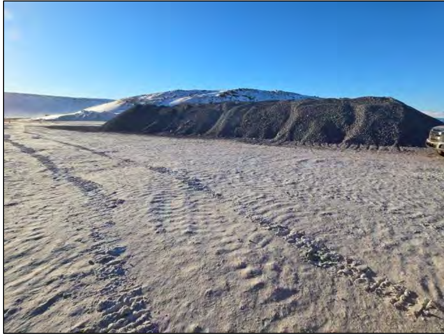
PHOTO 21. Material Stockpile - 32 mm minus culvert backfill material - km 94 laydown - Looking South (March 24, 2024).
