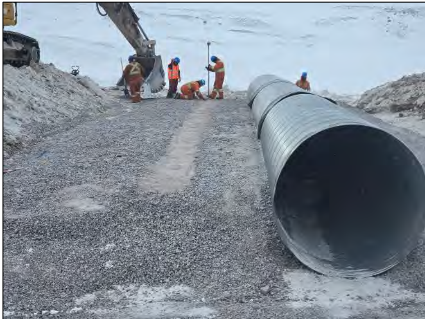
PHOTO 20. During Construction - Vantage Point 1 - Placement of Culvert Bedding Material under high flow culvert - Looking Southwest (April 30, 2024).
