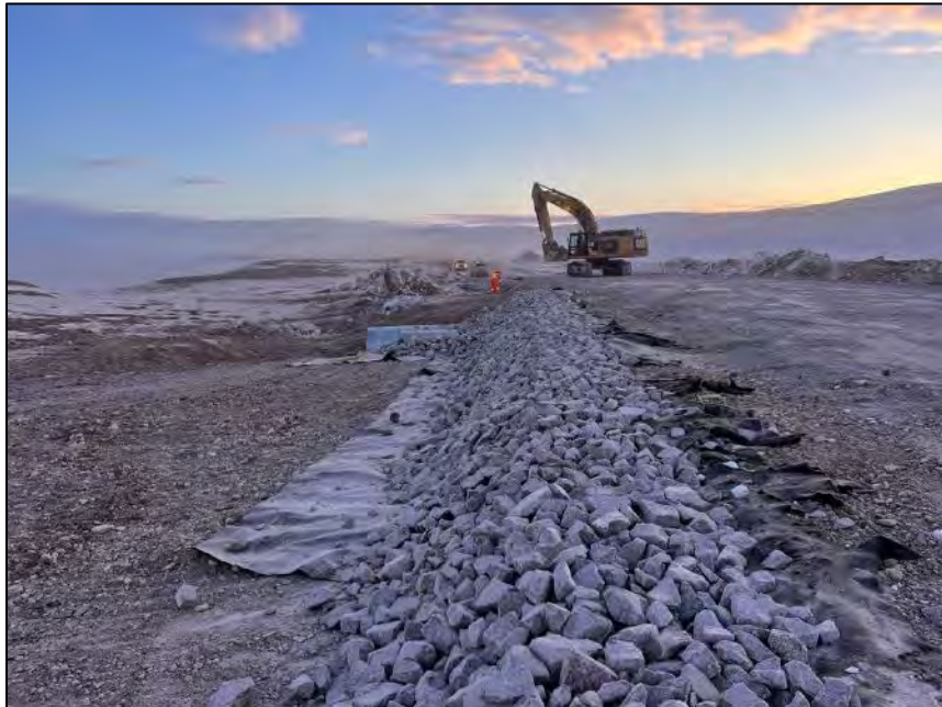
PHOTO 26. During Construction - Vantage Point 3 - Placement of Riprap for Slope Stabilization - Looking North (May 09, 2024).
