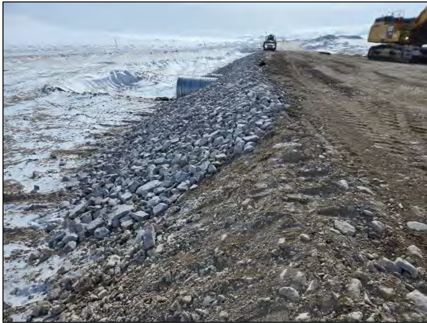
PHOTO 23. During Construction - Vantage Point 3 - Slope stabilization and riprap placement on inlet side of crossing - Looking South (May 04, 2024).
