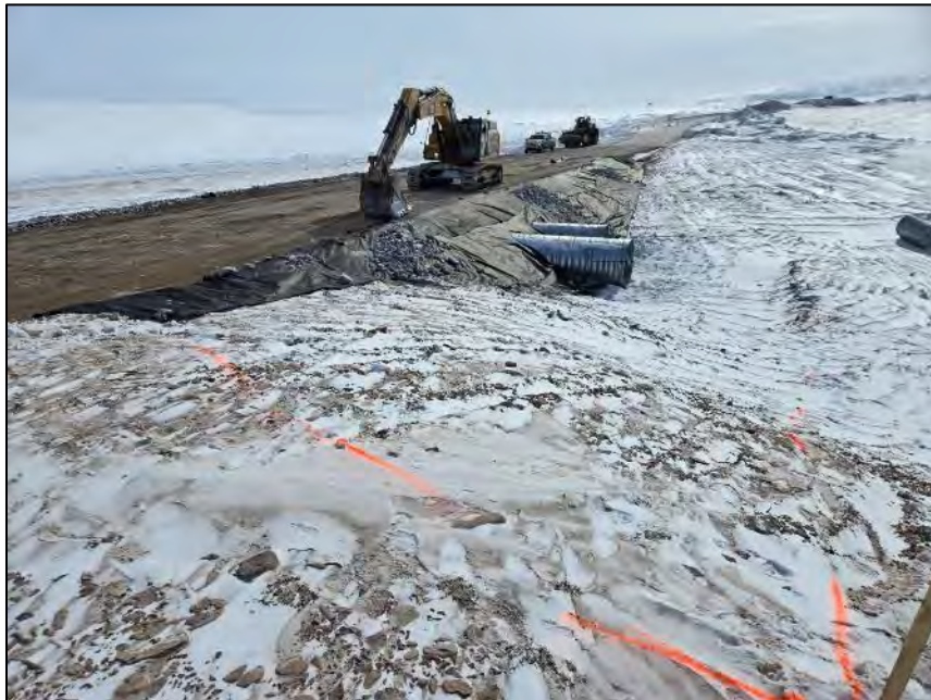
PHOTO 24. During Construction - Vantage Point 4 - Installation of geotextile on outlet side of crossing - Looking Southeast (May 04, 2024).
