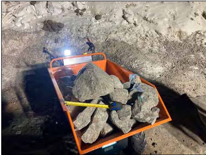
PHOTO 37. Equipment - Ducar Motorized Wheel Barrow loaded with Coarse Riprap - CV-059 (March 26, 2024).
