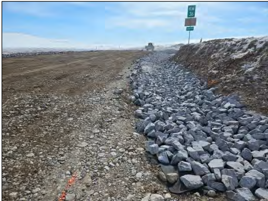
PHOTO 26. During Construction - Vantage Point 4 Riprap and geotextile placement in ditches on west side of crossing - Looking Southeast (May 05, 2024).
