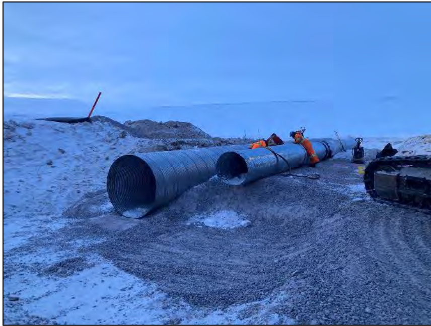
PHOTO 21. During Construction - Vantage Point 3 - Installation of high flow culvert - Looking Northeast (April 30, 2024).
