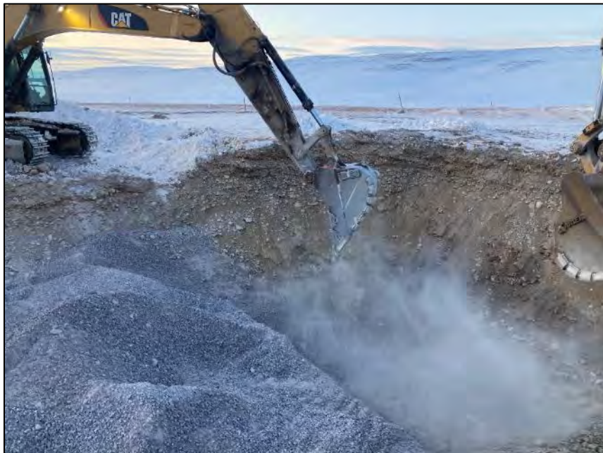
PHOTO 12. During Construction - Vantage Point 3 - Placement of Culvert Backfill Material in Inlet Apron - Looking North (May 05, 2024).
