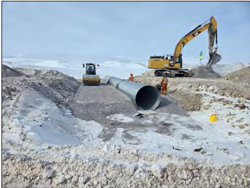
PHOTO 19. During Construction - Vantage Point 4 - Compaction of Culvert Backfill Material around low flow culvert - Looking Southeast (April 30, 2024).
