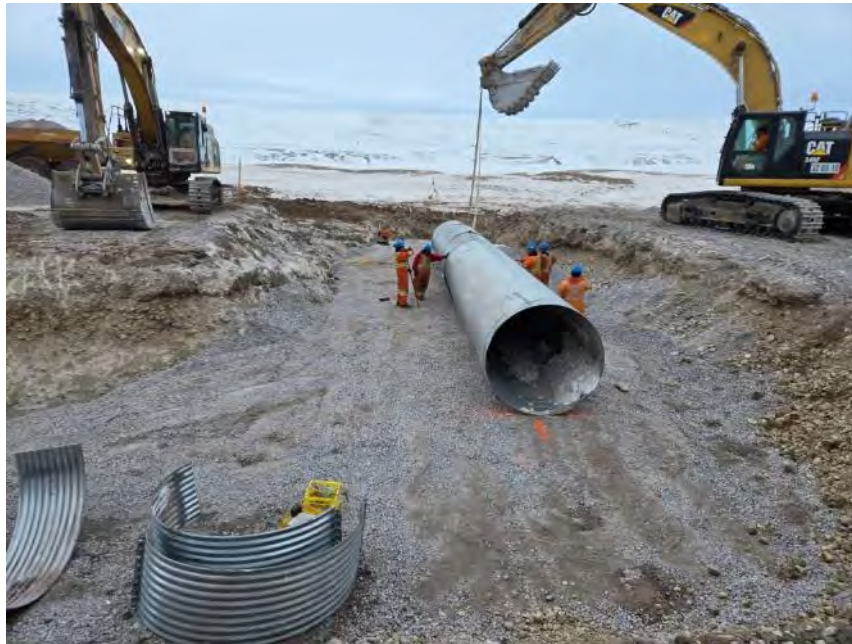
PHOTO 19. During Construction - Vantage Point 2 - Installation of Low Flow Culvert - Looking Northwest (May 06, 2024).
