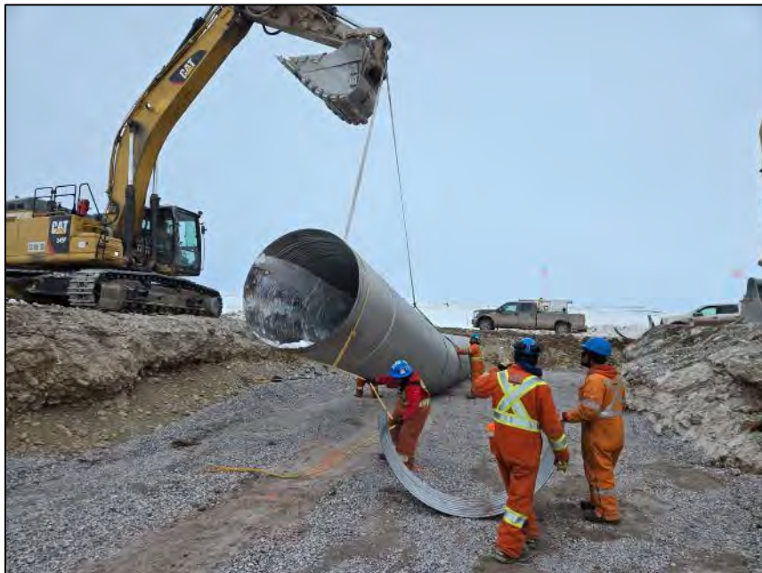
PHOTO 18. During Construction - Vantage Point 3 - Installation of Low Flow Culvert - Looking Northeast (May 06, 2024).
