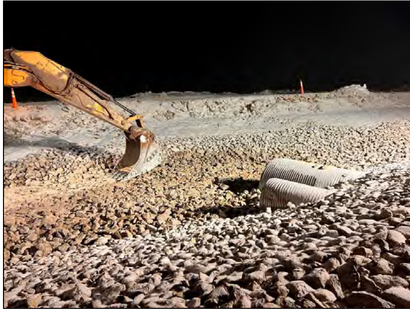
PHOTO 19. Following Construction - Vantage Point 3 - Completed CV-059 west (outlet) apron with coarse riprap and stream substrate material - looking northwest (March 29, 2024).
