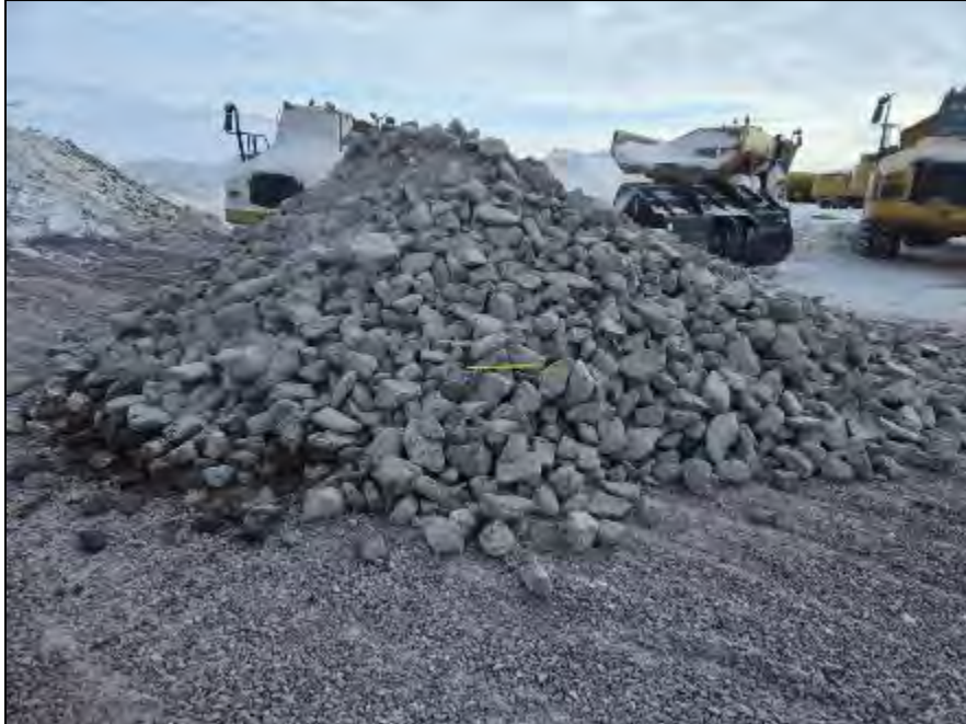
PHOTO 22. Material stockpile - Fine riprap - km 60 Laydown - looking southeast (March 22, 2024).
