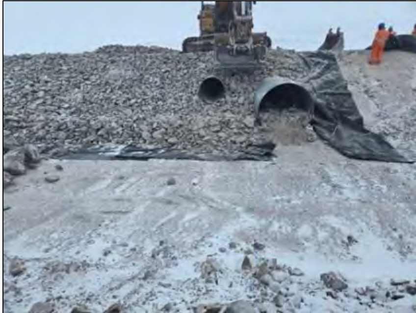
PHOTO 14. During - Vantage Point 2 - Placement of geotextile and riprap on west side slope at CV-057 - Upstream inlet - looking west (March 30, 2024).
