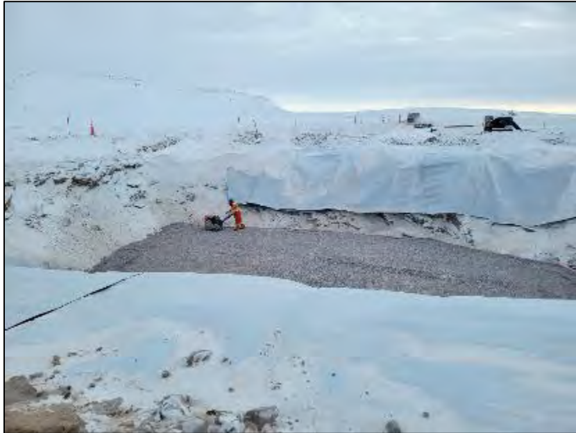
PHOTO 7. During - Vantage Point 3 - Compaction of culvert backfill material - Road crossing and downstream outlet - looking north (March 13, 2024).
