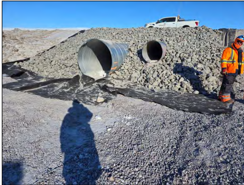
PHOTO 17. During Construction - Vantage Point 3 - Placing geotextile and riprap on west side slope at CV-059 - looking north (March 25, 2024).
