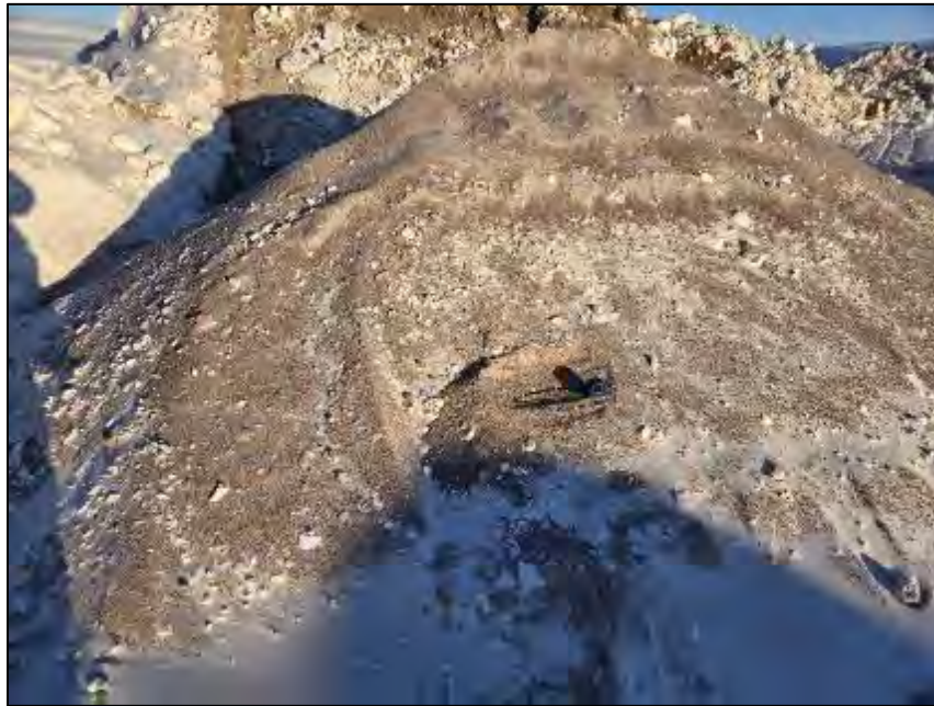
PHOTO 21. Material stockpile - 32 mm minus culvert backfill material - km 60 laydown - looking northeast (March 10, 2024).
