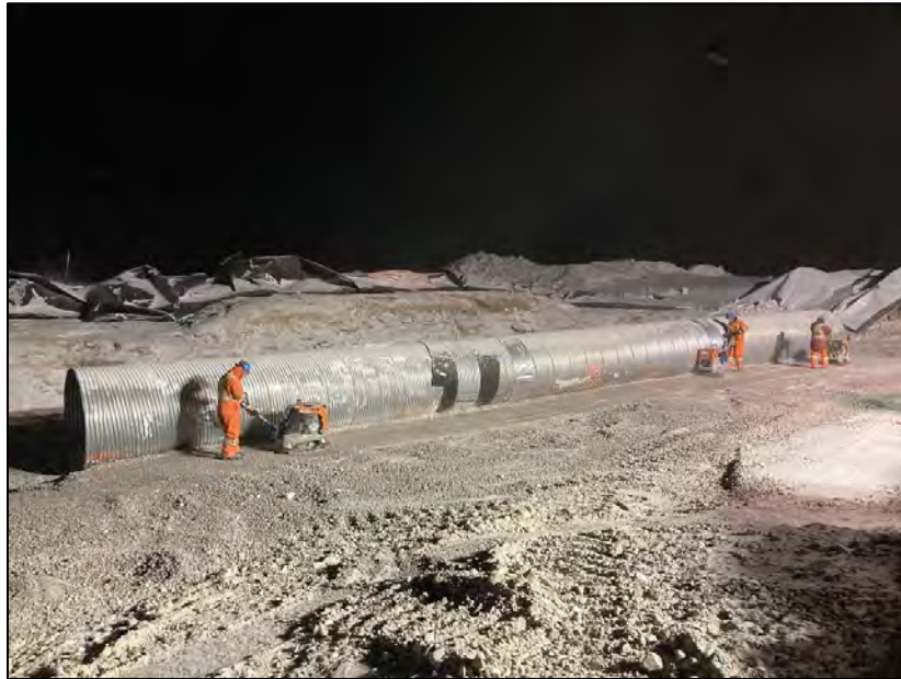
PHOTO 13. During Construction - Vantage Point 3 - Installation of 1.8 m diameter corrugated steel pipe low flow culvert - looking north (March 17, 2024).
