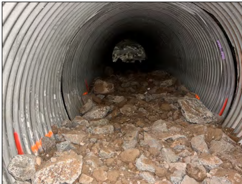
PHOTO 24. Following Construction - Completed placement of coarse riprap and stream substrate material within the interior of the low flow CSP culvert at CV-059 (March 28, 2024).
