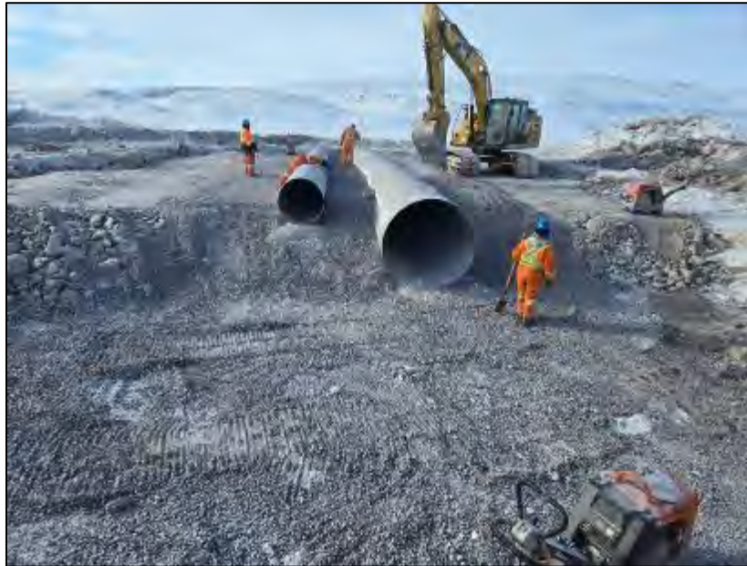
PHOTO 11. During - Vantage Point 2 - Installation of 1.8 m diameter corrugated steel pipe low flow culvert and 1.0 m diameter corrugated steel pipe high flow culvert - Upstream inlet - looking southwest (March 22, 2024).
