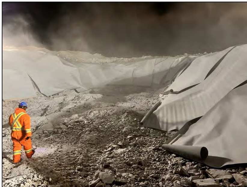
PHOTO 8. During Construction - Vantage Point 3 - Completed blast excavation with slope stabilization - road crossing and upstream inlet - looking northeast (March 4, 2024).
