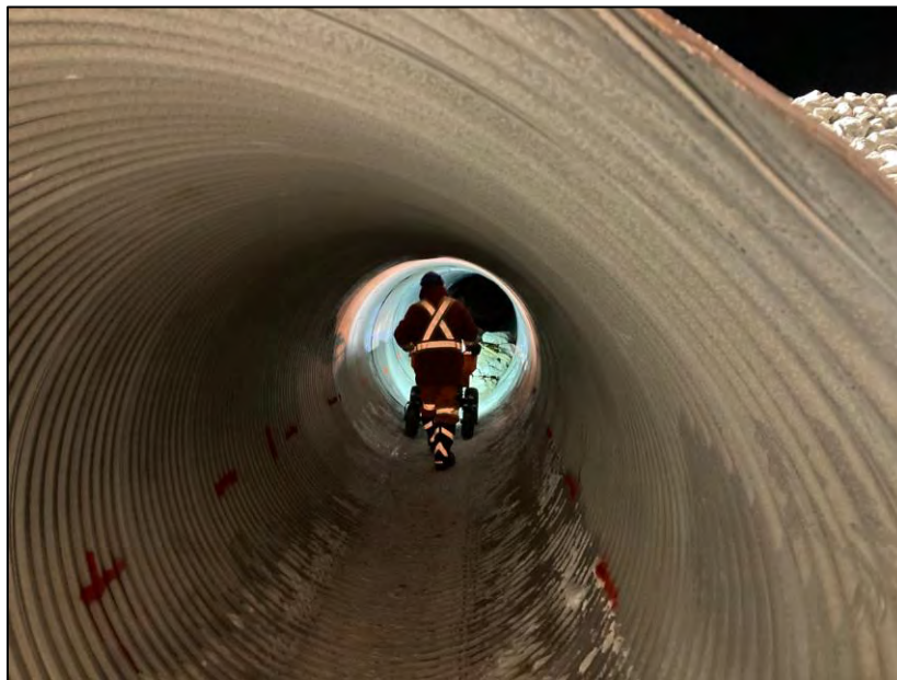
PHOTO 18. During Construction - Placement of coarse riprap and stream substrate material using electric wheelbarrow within the interior of the low flow CSP culvert at CV-059 - west (outlet) - looking northeast (March 27, 2024).
