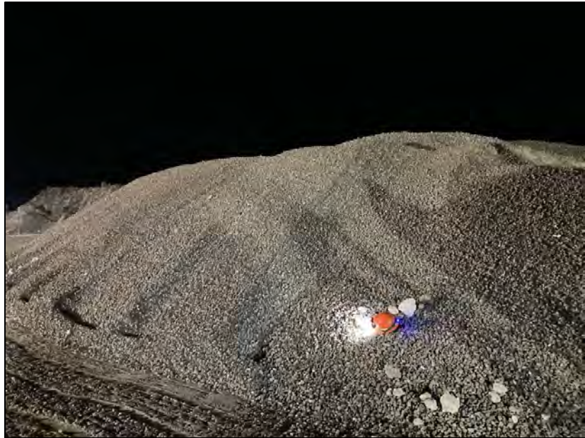
PHOTO 25. Material stockpile - 32 mm minus culvert backfill material - km 60 laydown - looking northeast (March 10, 2024).
