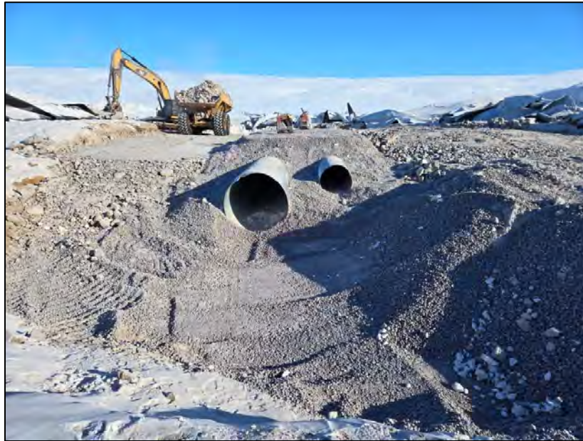
PHOTO 15. During Construction - Vantage Point 4 - Installation of high flow and low flow culverts - downstream outlet area - looking northeast (March 21, 2024).
