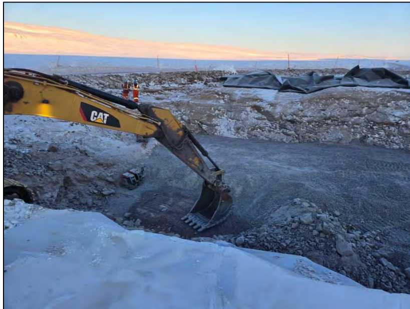
PHOTO 10. During Construction - Vantage Point 2 - Placement of culvert backfill material - upstream inlet - looking west (March 14, 2024).
