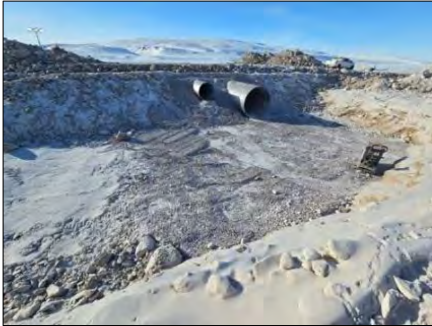
PHOTO 13. During - Vantage Point 2 - Placement of culvert backfill material above the low and high flow CSP culverts - Upstream inlet - looking west (March 26, 2024).
