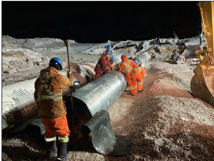
PHOTO 14. During Construction - Vantage Point 3 - Installation of 1.0 m diameter corrugated steel pipe high flow culvert - looking northeast (March 19, 2024).
