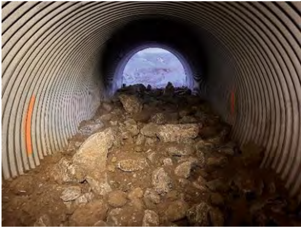
PHOTO 19. After - Completed placement of coarse riprap and stream substrate material within the interior of the low flow CSP culvert at CV-057 (March 29, 2024).
