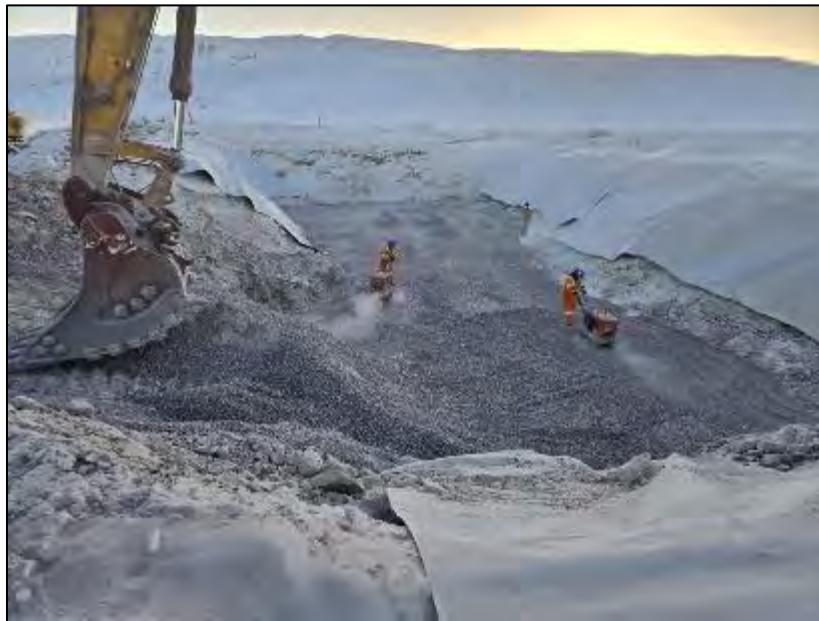
PHOTO 8. During - Vantage Point 2 - Compaction of culvert backfill material - Road crossing and upstream inlet - looking west (March 15, 2024).
