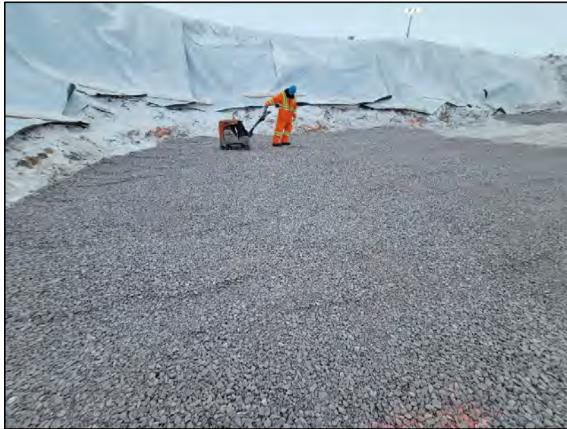
PHOTO 9. During Construction- Vantage Point 1 - Compaction of culvert backfill material - upstream inlet - looking south (March 12, 2024).
