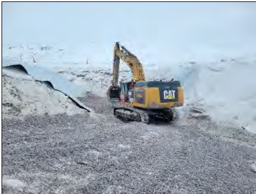
PHOTO 6. During - Vantage Point 2 - Placement of culvert backfill material - Road crossing and downstream outlet - looking west (March 12, 2024).
