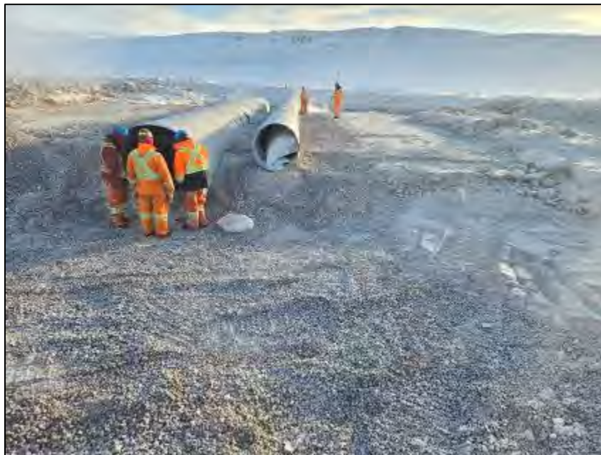
PHOTO 12. During - Vantage Point 3 - Installation of 1.8 m diameter corrugated steel pipe low flow culvert and 1.0 m diameter corrugated steel pipe high flow culvert - Downstream outlet - looking northeast (March 22, 2024).
