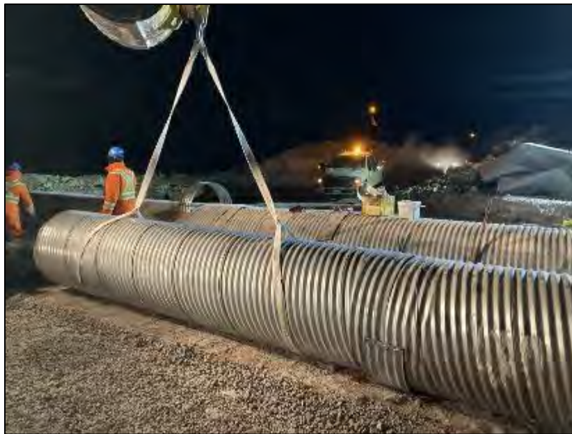
PHOTO 10. During - Vantage Point 2 - Installation of 1.0 m diameter corrugated steel pipe high flow culvert - looking northwest (March 19, 2024).
