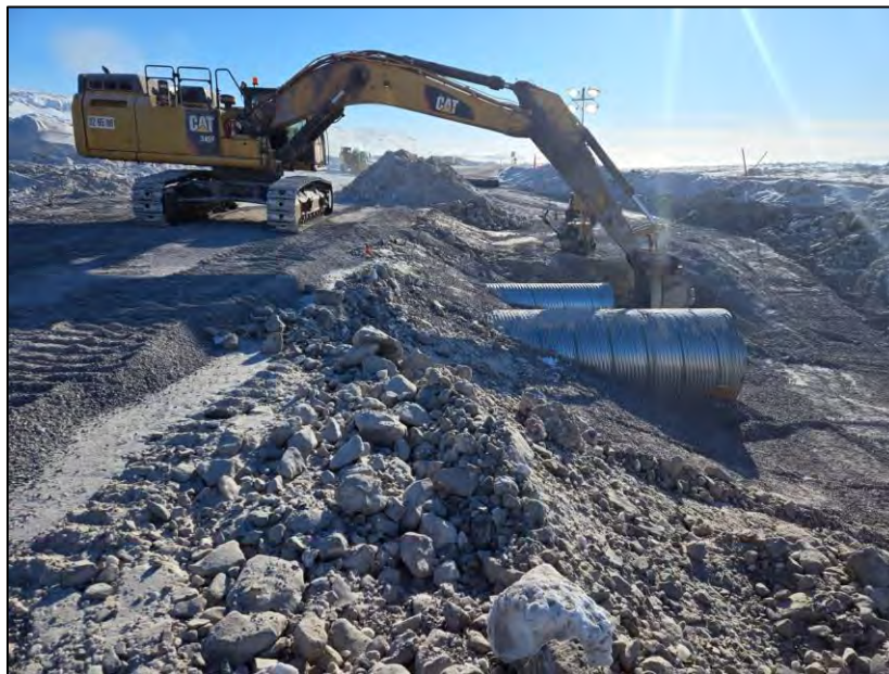
PHOTO 16. During Construction - Vantage Point 4 - Grading 2H:1V west side slope at CV-059 - looking southwest (March 24, 2024).
