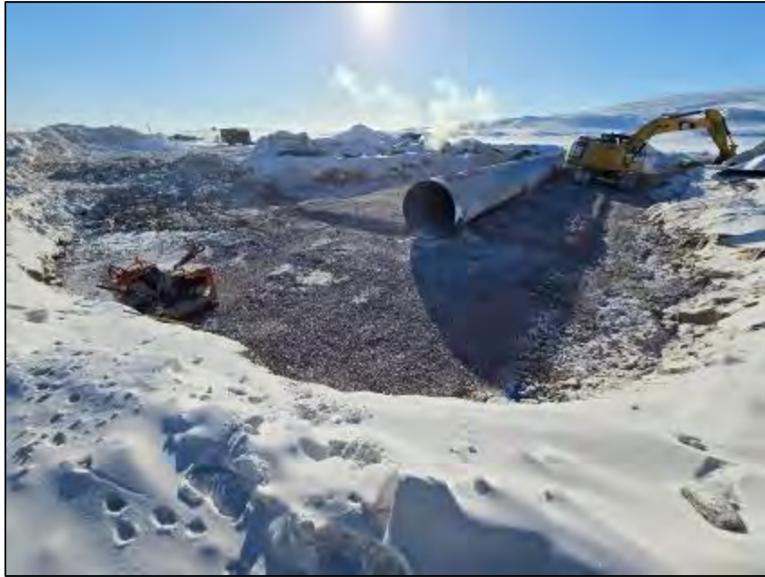
PHOTO 9. During - Vantage Point 3 - Installation of 1.8 m diameter corrugated steel pipe low flow culvert - Road crossing and downstream outlet - looking northeast (March 20, 2024).
