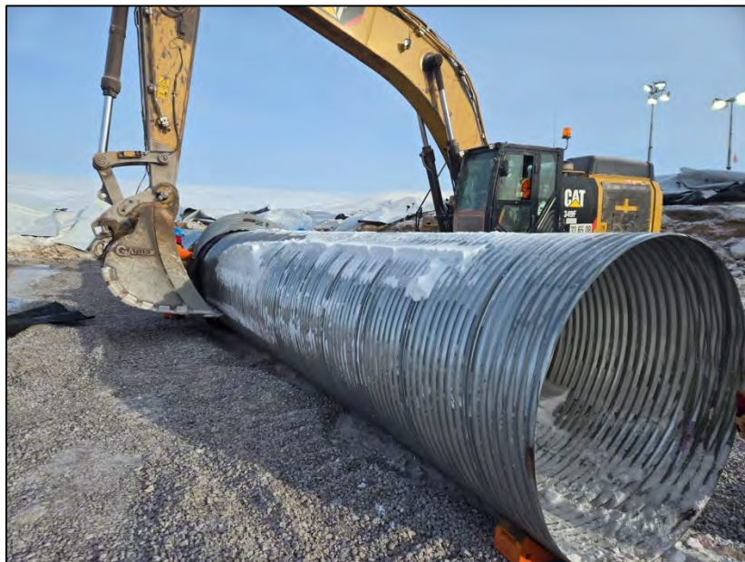
PHOTO 12. During Construction - Vantage Point 4 - Installation of 1.8 m diameter corrugated steel pipe low flow culvert - looking southeast (March 17, 2024).
