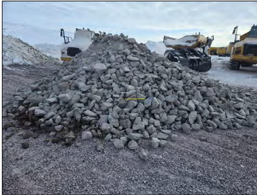
PHOTO 27. Material Stockpile - Fine Riprap - km 60 laydown - looking southeast (March 22, 2024).
