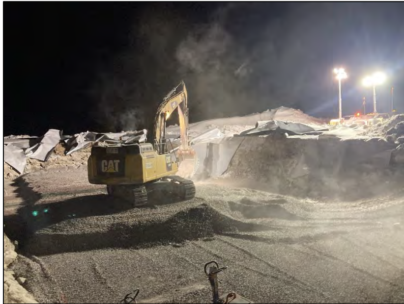
PHOTO 11. During Construction - Vantage Point 4 - Placement of culvert backfill material - road crossing and downstream outlet - looking southeast (March 15, 2024).
