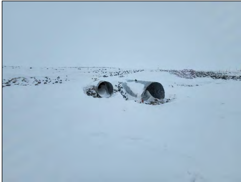
PHOTO 21. Following Construction - Vantage Point 2 - Completed installation of high flow and low flow culverts - upstream inlet area - looking northwest (April 5, 2024).
