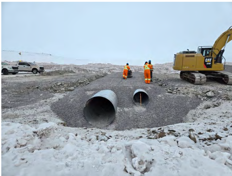
Photo 9 Compacted 32 mm minus material above low and high flow culverts at CV-001. Photo taken March 30, 2024, facing northeast.
