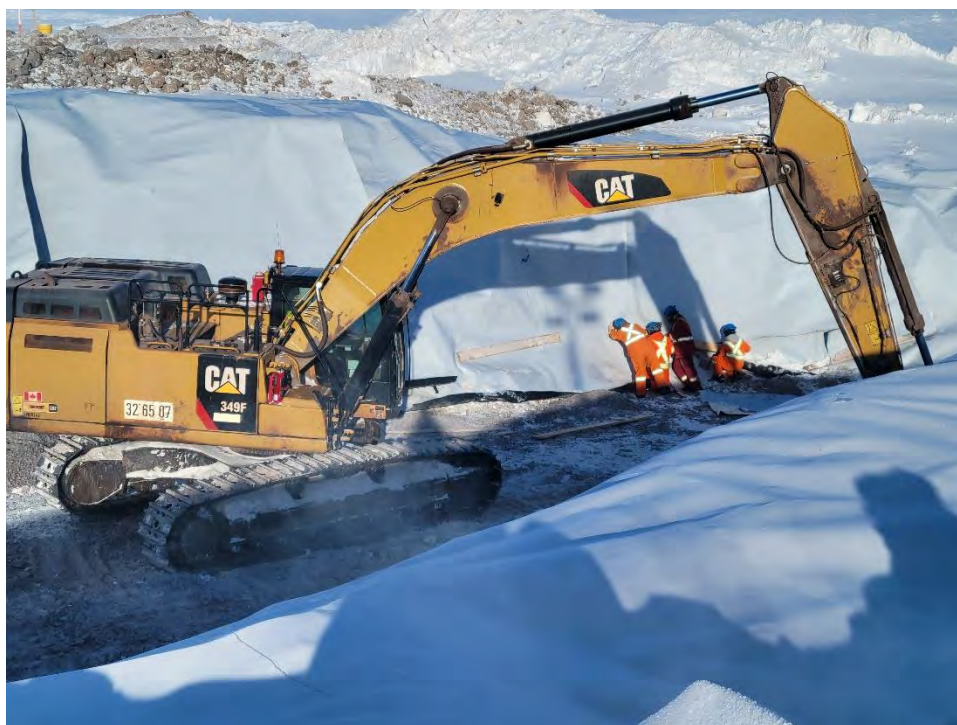
Photo 5 Shortening of geomembrane at CV-059. Photo Taken March 08, 2024, looking north.
