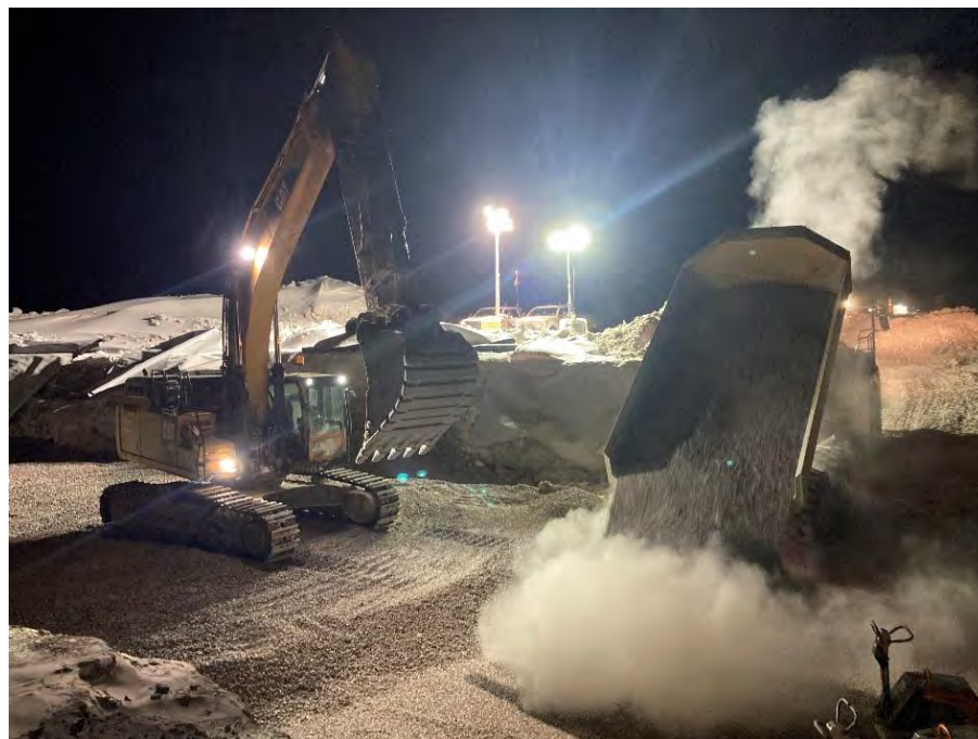
Photo 9 Placement of 300 mm lift of 32 mm minus material at CV-059. Photo taken March 15, 2024.
