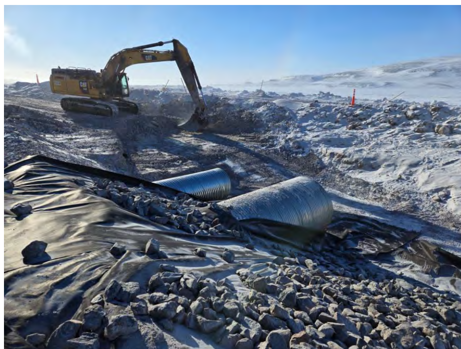
Photo 2 Excavating the western apron (outlet) area at CV-059. Photo taken March 25, 2024.
