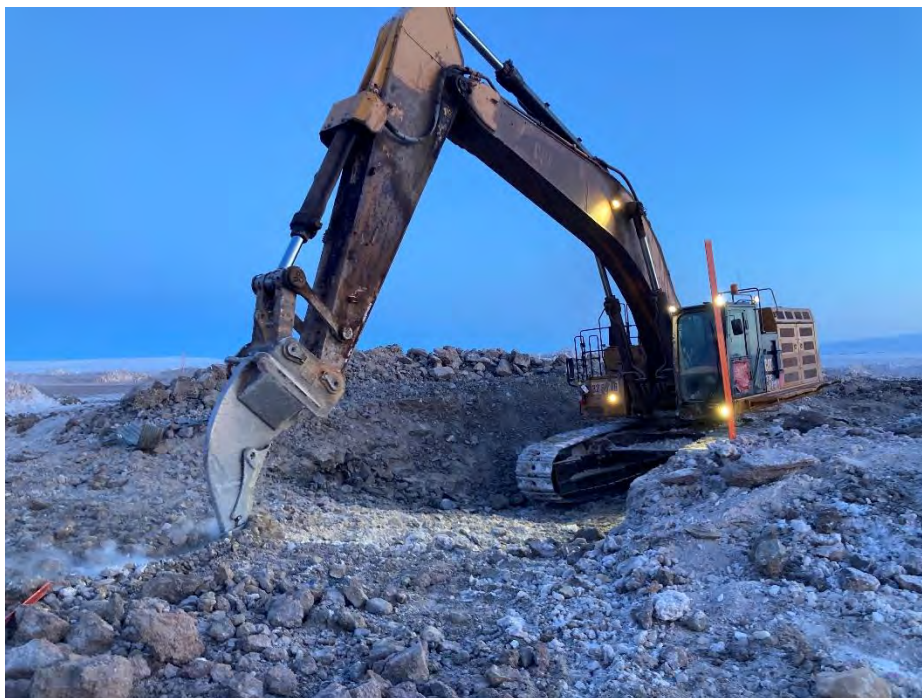
Photo 3 Ripping the excavation surface for foundation preparation at CV-001. Photo taken March 25 2024.
