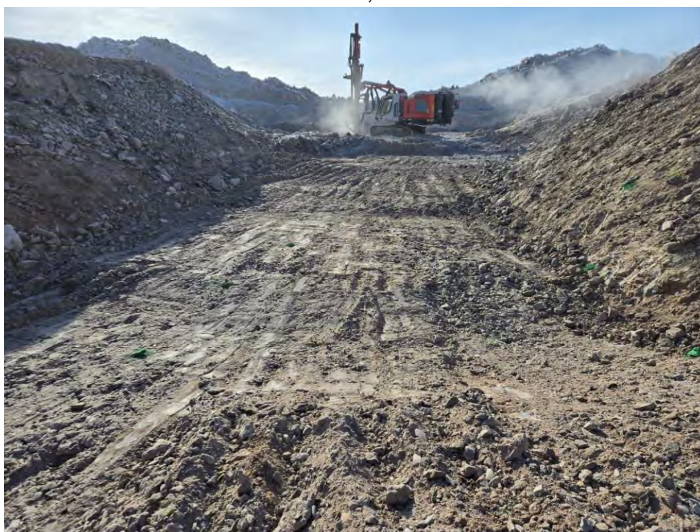
Photo 6 Additional "honeycomb" drilling at base of BG-04 to assist with further ripping and excavation. Photo taken March 26, 2024, facing southwest.
