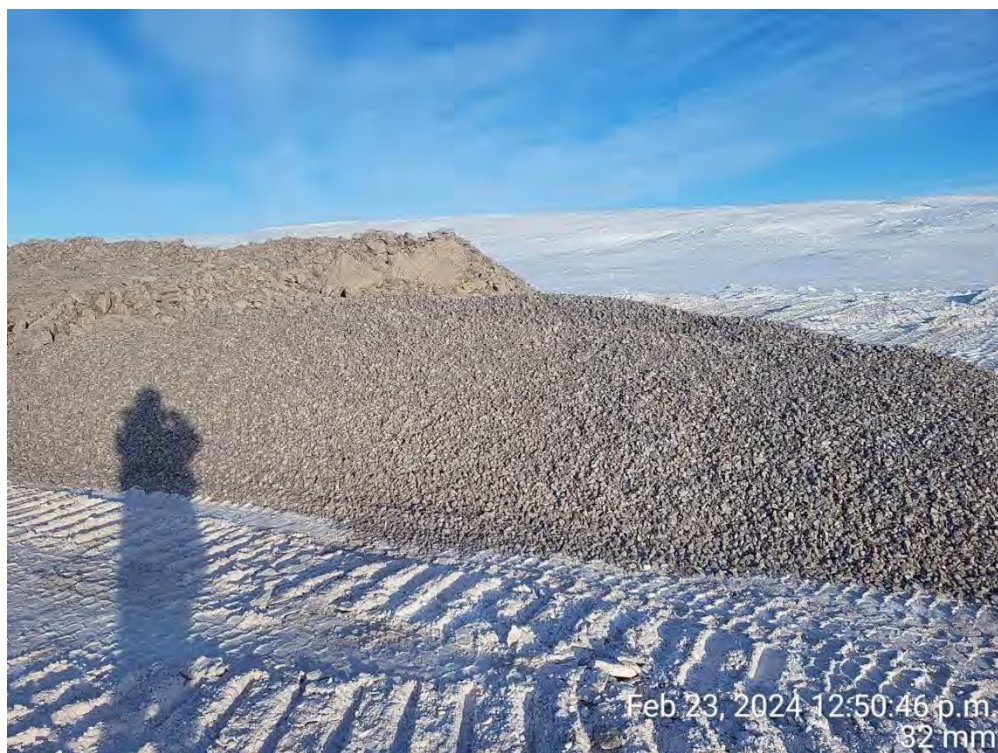
Photo 15: Looking at the 32 mm minus stockpile at km 60 (February 23, 2024)
