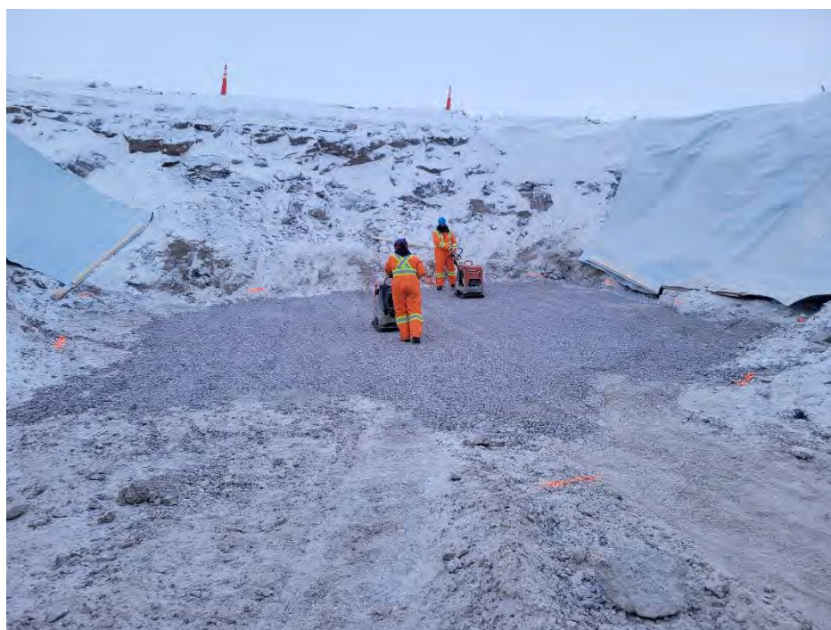
Photo 4 Compaction of a 200 mm lift of 32 mm minus material at CV-057. Photo taken March 12, 2024.
