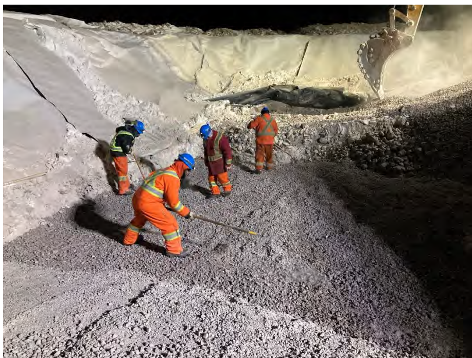
Photo 6 Labourers manually spreading 32 mm minus material for a 200 mm lift at CV-057. Photo taken March 13, 2024.
