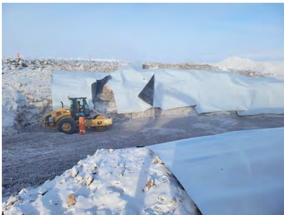
Photo 3 Smooth Drum Roller Compactor being used for the 32 mm minus Culvert Backfill at CV-059. Photo taken March 05, 2024.
