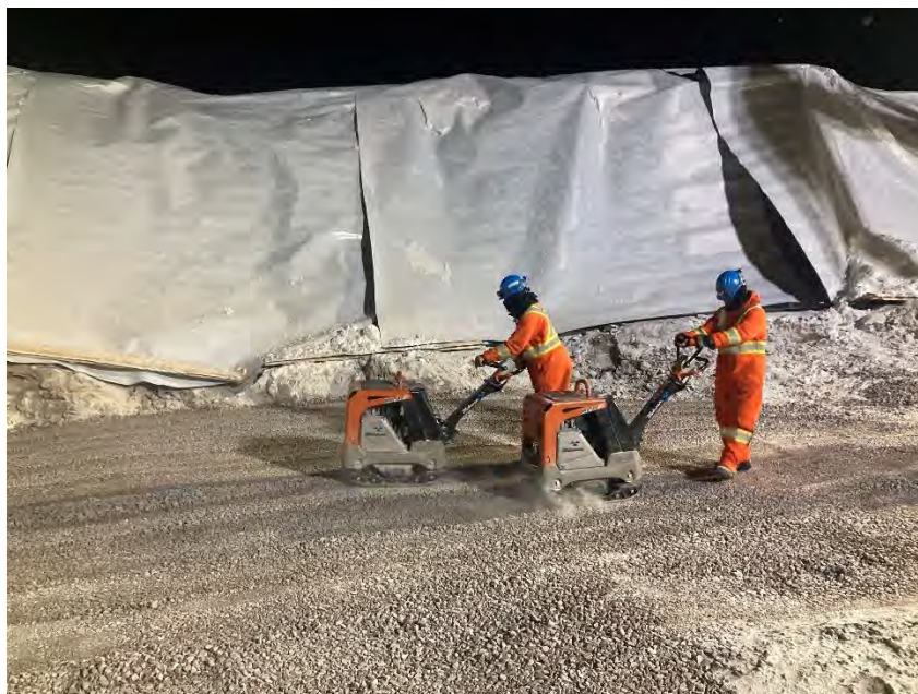
Photo 3 Compaction of a 200 mm thick Culvert Backfill material lift at CV-057 using the hand guided plate compactors. Photo taken March 11, 2024.
