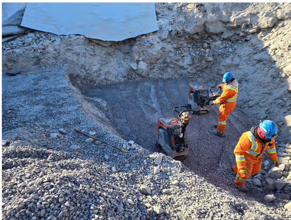
Photo 8 Compaction of 200 mm lift of 32 mm minus material at CV-057 ramp area. Photo taken March 15, 2024.
