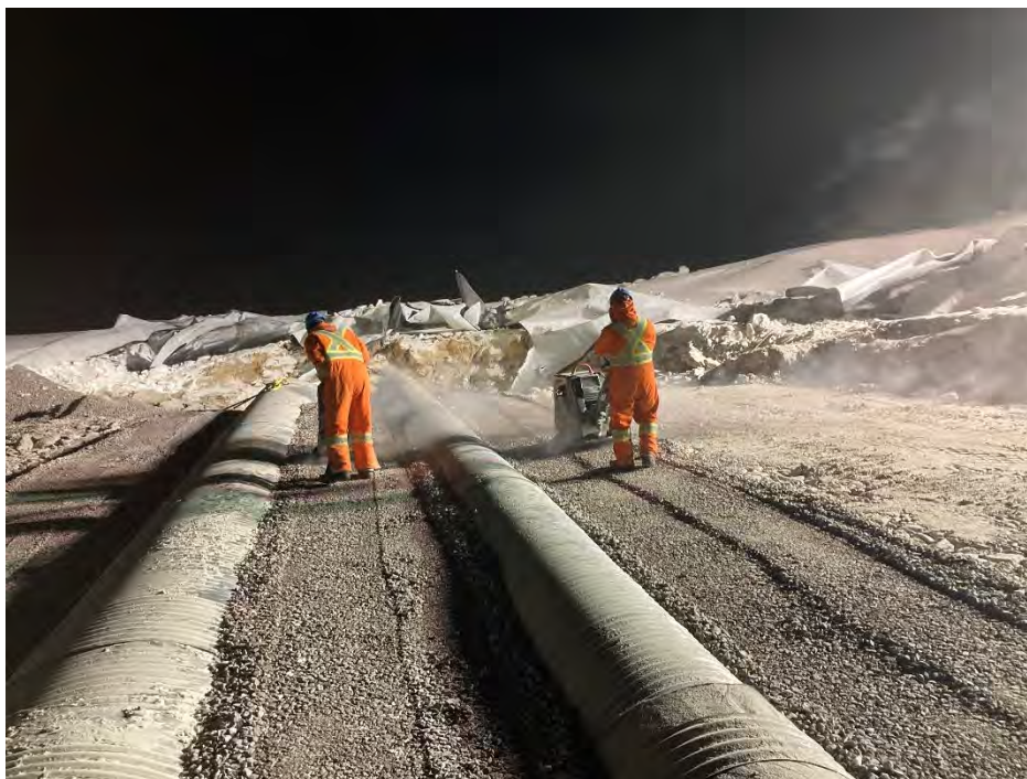
Photo 5 Compaction of 32 mm minus material around the culverts at CV-059. Photo taken March 20, 2024.
