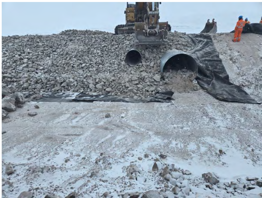
Photo 14 Placing geotextile and fine riprap on 2H:1V east side slope at CV-057. Photo taken March 30, 2024, facing west.
