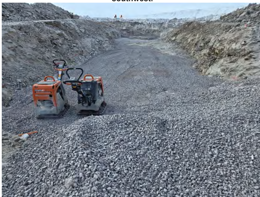
Photo 7 Prepared and approved foundation surface at CV-001. Photo taken March 26, 2024, facing southwest.
