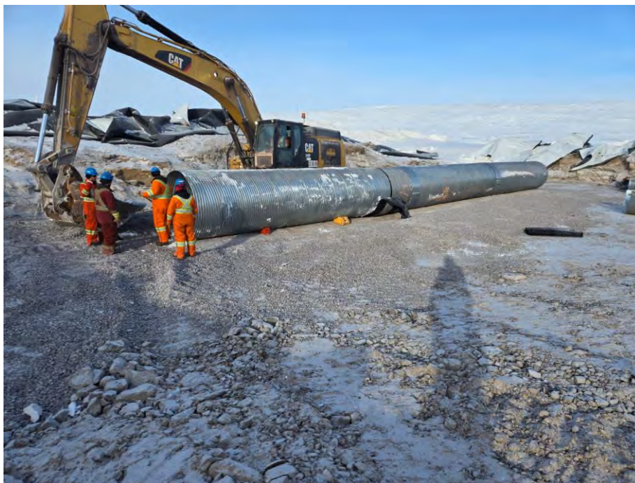
Photo 1 Full length (25.66 m) of the low flow culvert in place at CV-059. Photo taken March 17, 2024.
