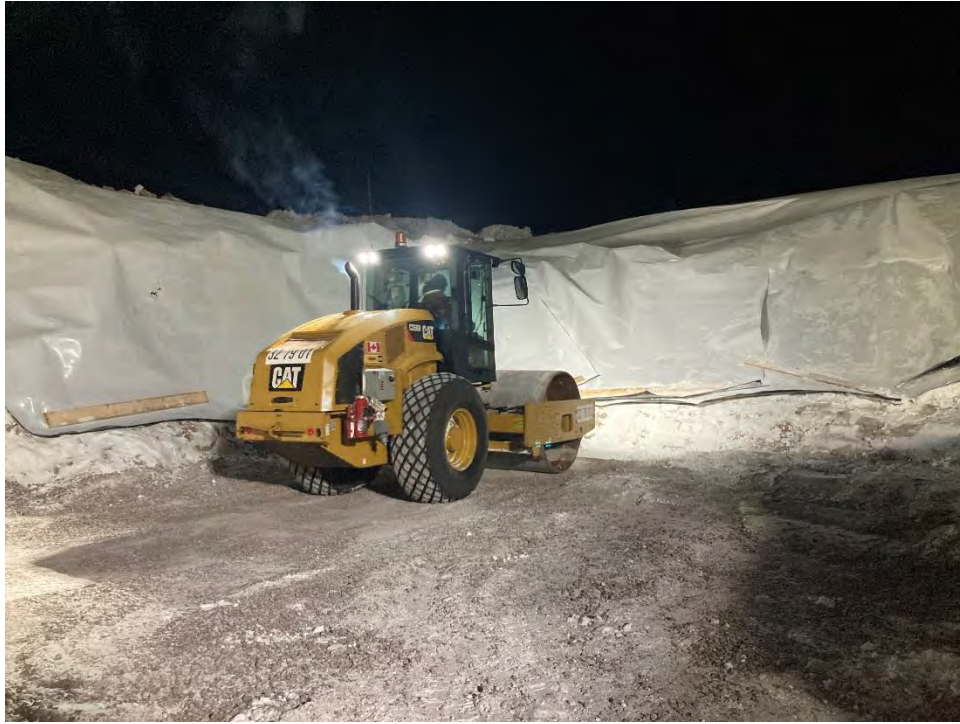
Photo 7 Compacting the base of the excavation at CV-059. Photo taken March 09, 2024, looking north.
