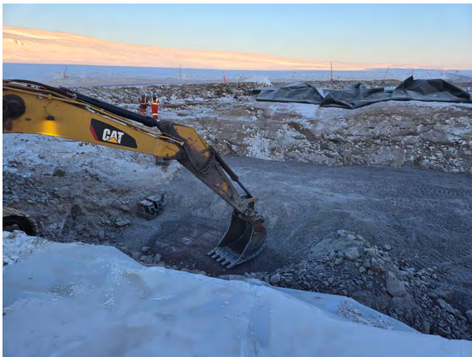
Photo 7 Placing of 200 mm lift of 32 mm minus material at CV-59. Photo taken March 14, 2024.
