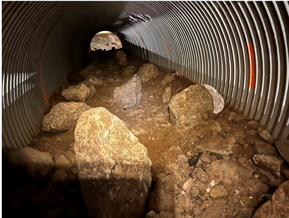
Photo 13 In progress low flow culvert infilling with coarse riprap and stream substrate material at CV-057. Photo taken March 29, 2024.
