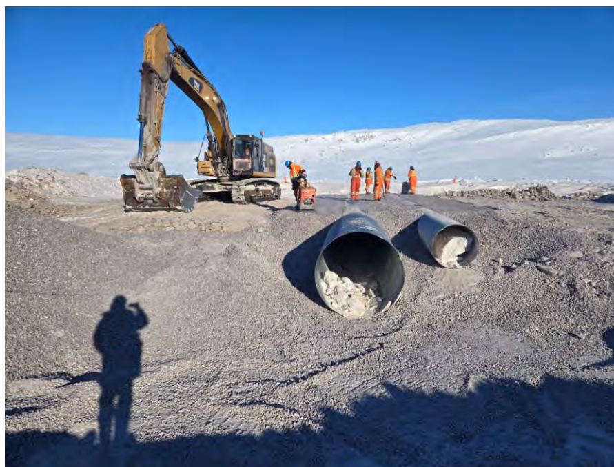
Photo 8 Compaction of 32 mm minus material adjacent to the installed culverts at CV-057. Photo taken March 23, 2024.
