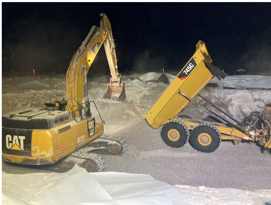
Photo 11 Placement of 300 mm lift of 32 mm minus material at CV-057. Photo taken March 16, 2024.
