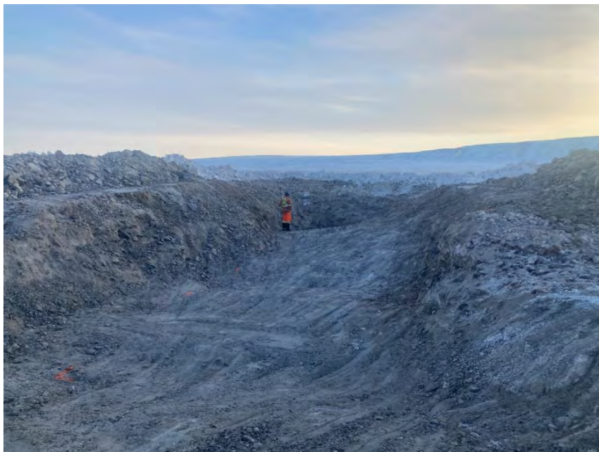
Photo 7 Prepared and approved foundation surface at CV-001. Photo taken March 26, 2024, facing southwest.
