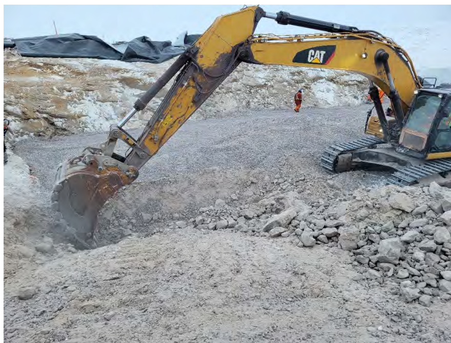
Photo 5 Excavation of blast material from access ramp for foundation preparation at CV-059. Photo taken March 13, 2024.
