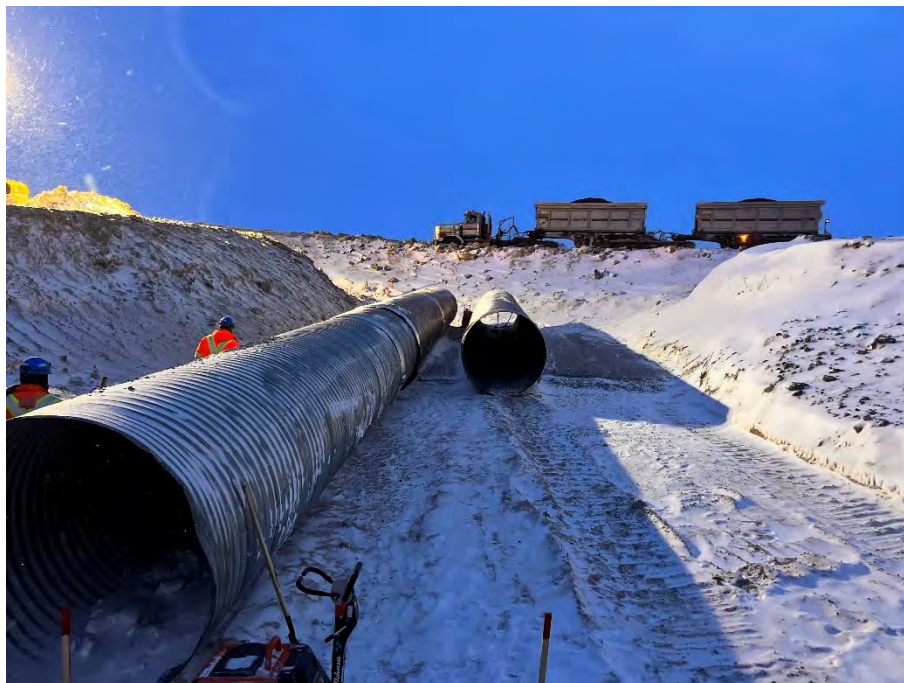
Photo 11 Compacted 32 mm minus material and uncompacted 3/16" culvert bedding material below the placed low flow culverts at BG-04. Photo taken March 30, 2024, facing north.
