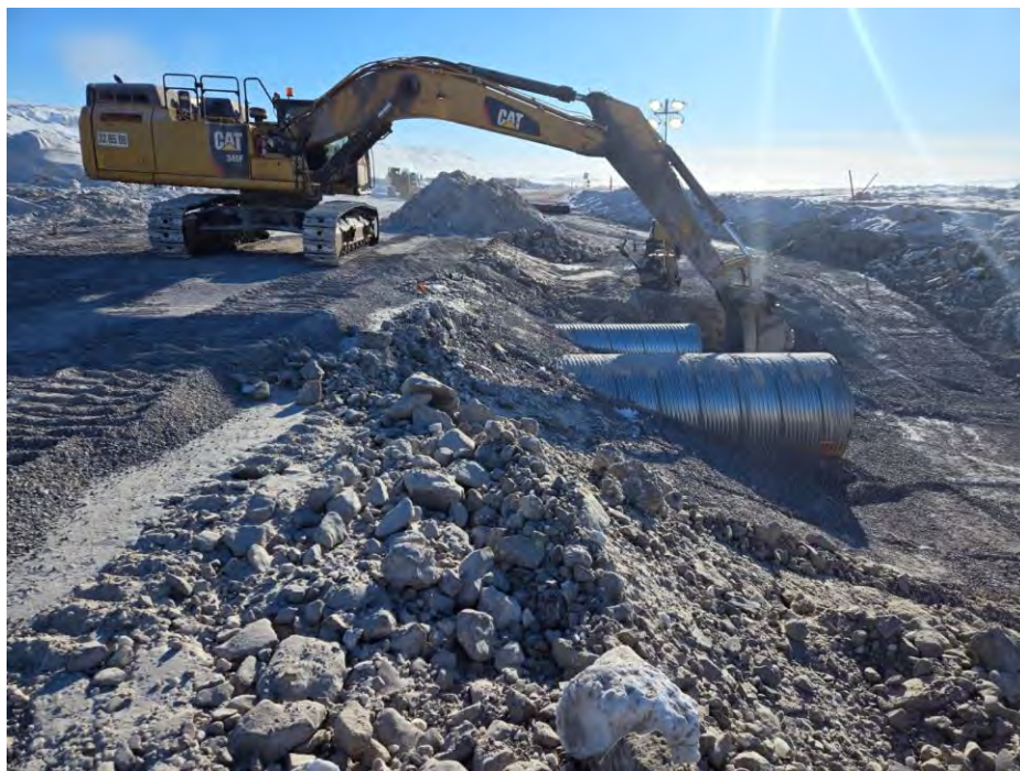
Photo 1 Grading 2H:1V west side slope at CV-059. Photo taken March 24, 2024.
