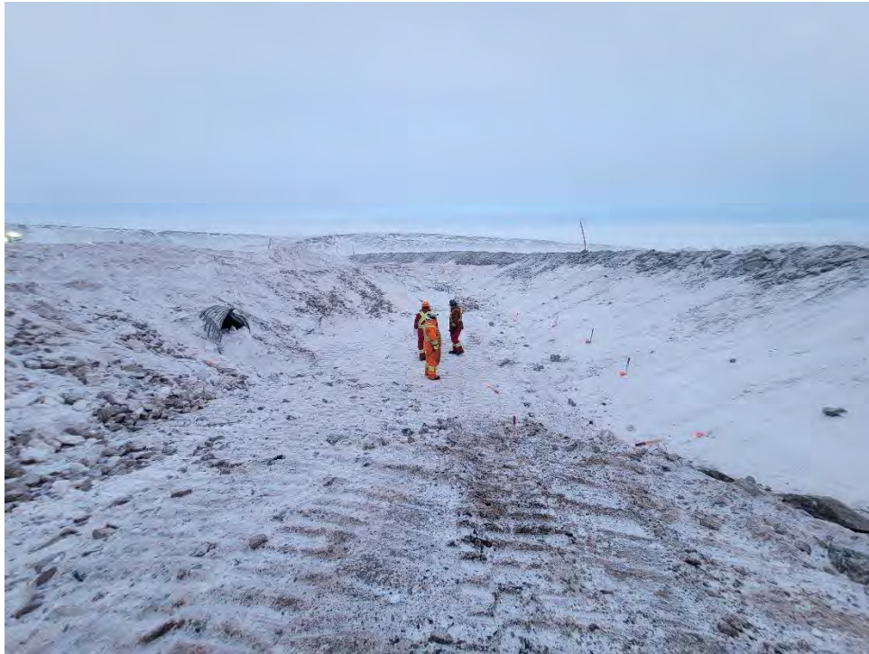
Photo 7: Inspection of blast layout markers for BG-04
