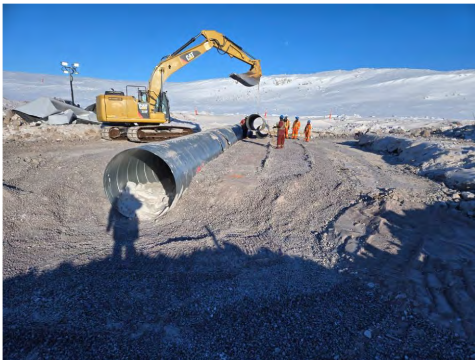
Photo 6 Placement of second 6 m segment of 1.0 m diameter high flow CSP culvert at CV-057. Photo taken March 21, 2024, looking northeast.
