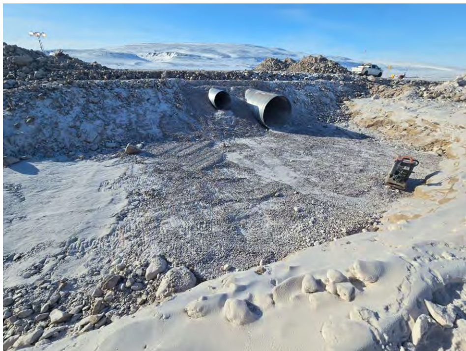
Photo 5 Placed local fill material above the low and high flow CSP culverts at CV-057. Photo taken March 26, 2024.
