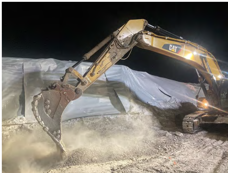
Photo 2 Placement of a 200 mm thick Culvert Backfill material lift at CV-057. Photo taken March 11, 2024.
