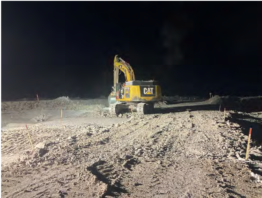
Photo 9 Placement of blast material overtop of 32 mm minus 1H:1V slope trapezoid at CV-059. Photo taken March 23, 2024.
