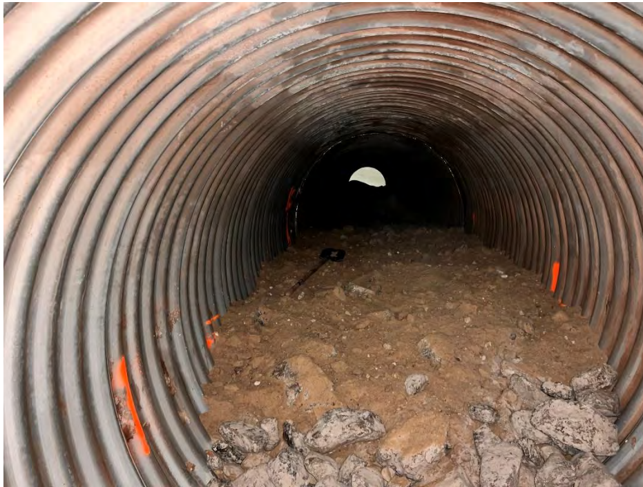
Photo 31 Culvert Infill Material progress during nightshift at BG-04 East low flow culvert. Photo taken April 5, 2024.
