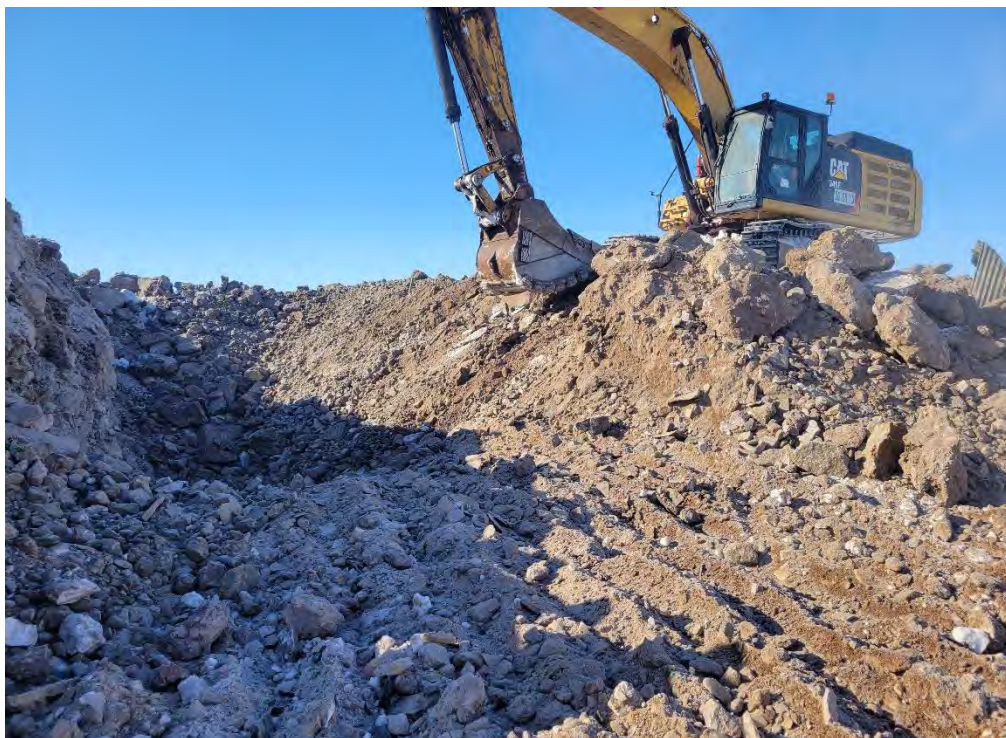
Photo 21 Frozen blasted material being excavated by Nuna at CV-216. Photo taken April 12, 2024, facing southwest.
