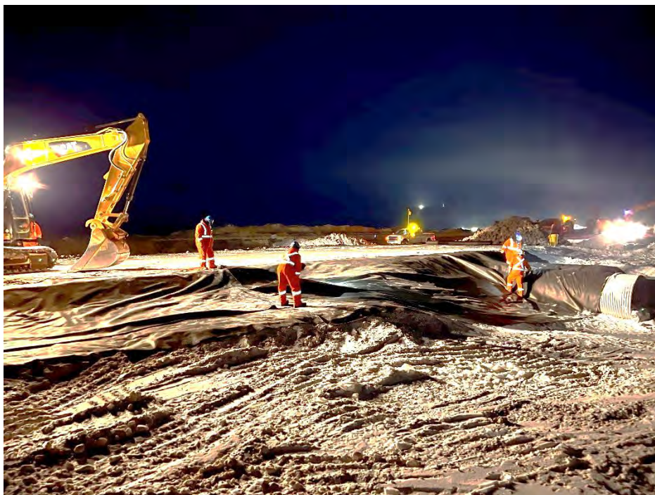
Photo 29 Geotextile placement on the outlet road slope at CV-001. Photo taken April 5, 2024, facing east.
