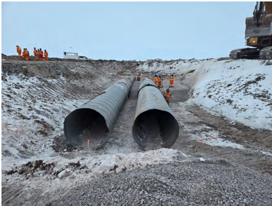
Photo 4 2.0 m diameter low flow CSP culverts fully installed at BG-04. Photo taken March 31, 2024, facing north.
