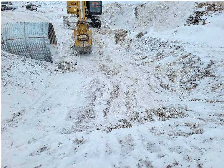
Photo 28 Snow removal from the inlet of CV-001. Photo taken April 5, 2024, facing north.
