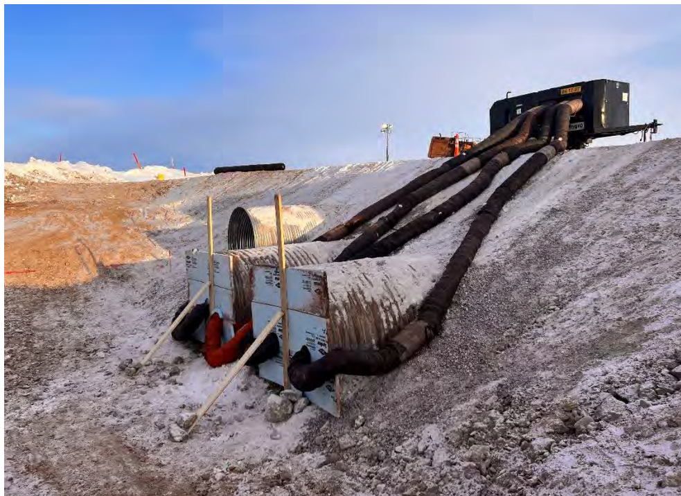
Photo 18 Frost fighters installed in the inlet end of the low flow culverts at BG-04. Photo taken April 11, 2024, facing east.
