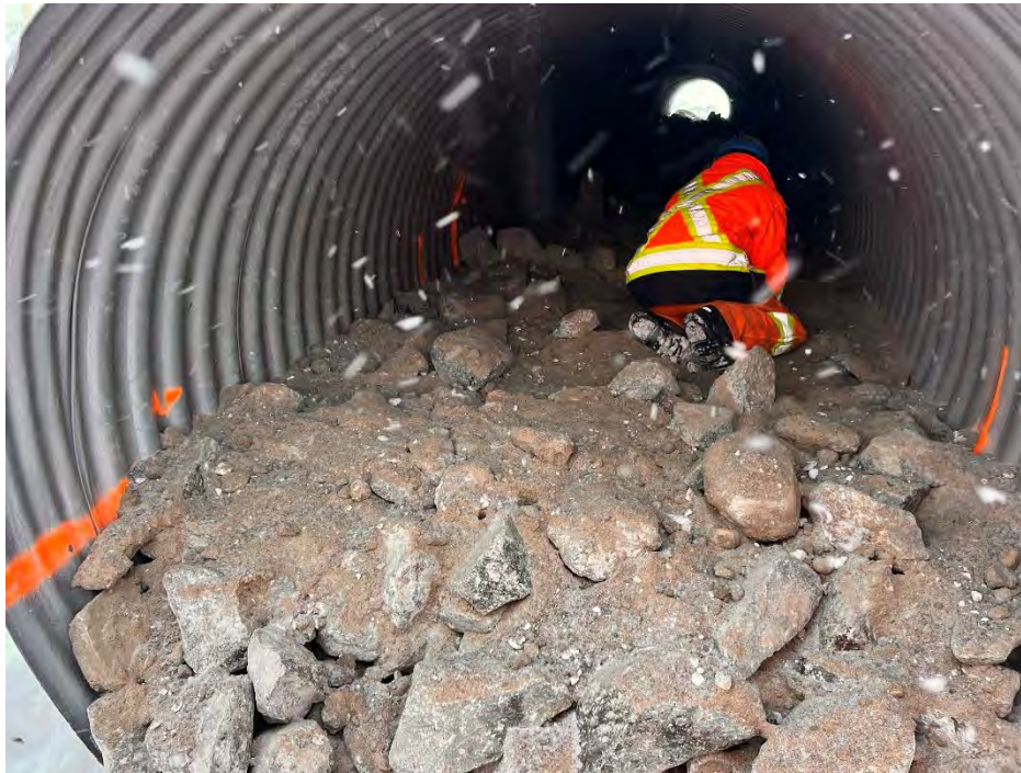
Photo 27 Stream substrate material being added to Riprap fill in voids throughout the 0.80 of riprap in West low flow culvert at the outlet side. Photo taken April 4, 2024, facing inlet.
