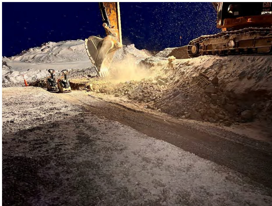
Photo 8 Local borrow area fill placement beside compacted 32 mm minus Culvert Backfill material at BG-04. Photo taken April 7, 2024, facing southwest.
