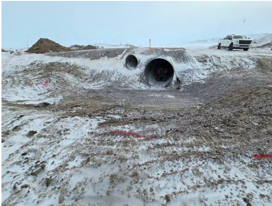
Photo 5 North apron area and prepared coarse riprap and stream substrate material for low flow CSP culvert infilling at CV-001. Photo taken March 31, 2024, facing south.
