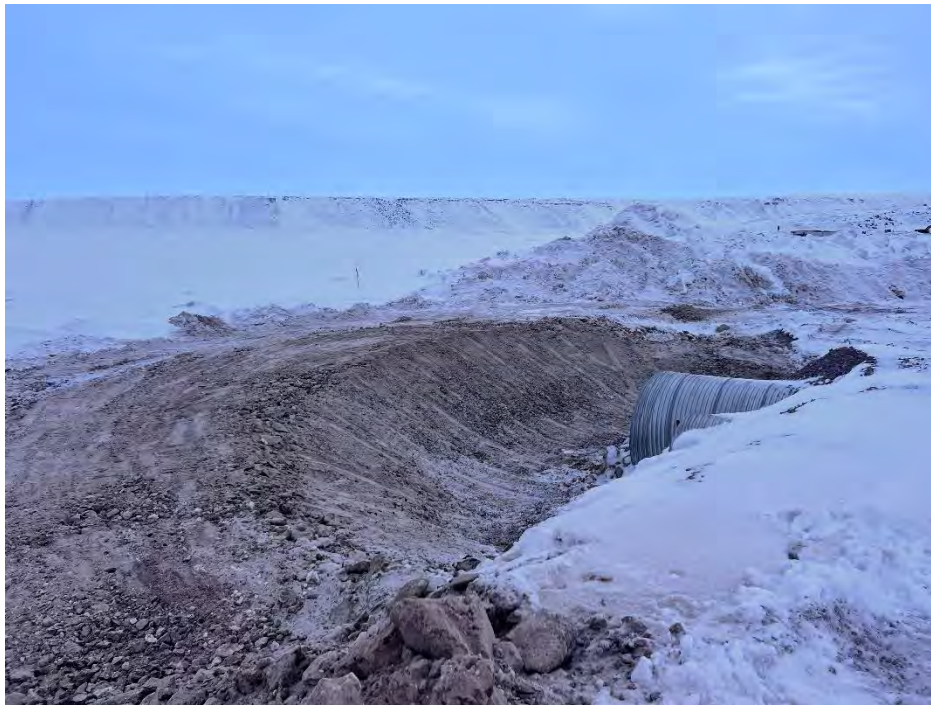
Photo 25 CV-001 excavated outlet apron. Photo taken April 3, 2024, facing northwest.
