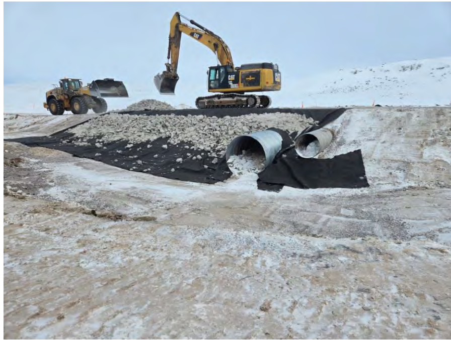
Photo 1 Placing geotextile and fine riprap on the west 2H:1V side slope at CV-057. Photo taken March 31, 2024, facing east.
