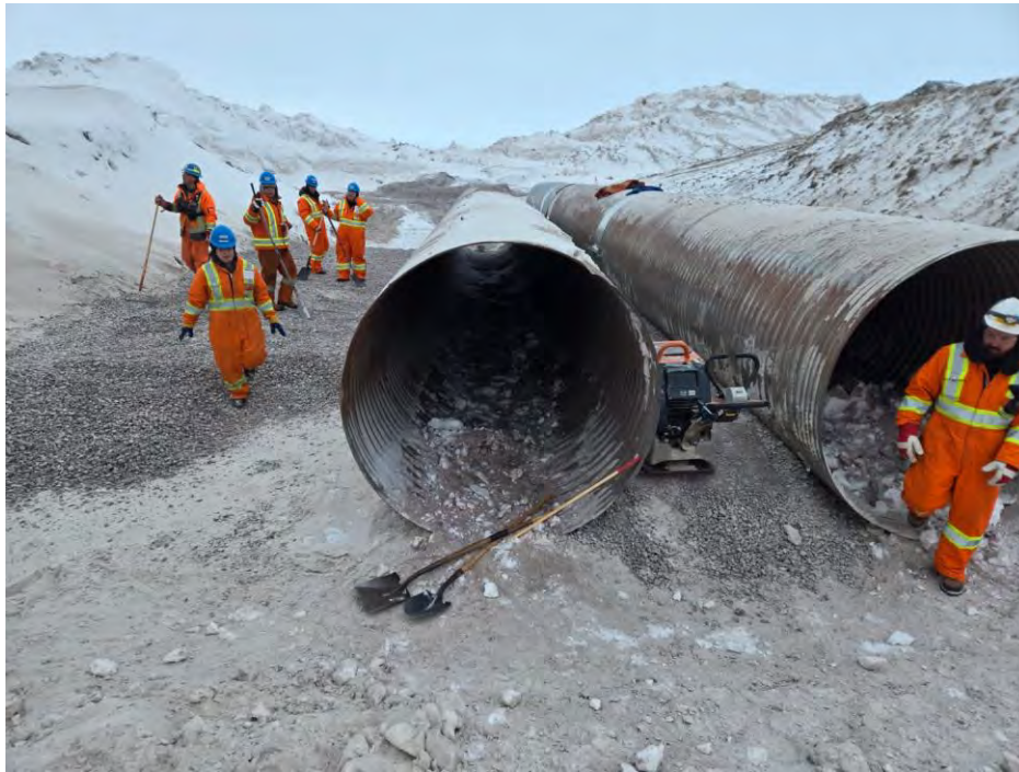
Photo 3 Placing and compacting 32 mm minus culvert backfill material at BG-04. Photo taken March 31, 2024, facing south.
