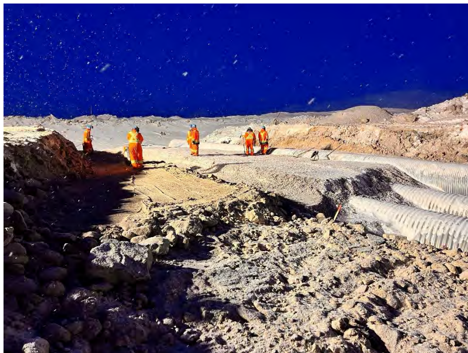
Photo 7 Local borrow area fill placement and compaction against the 32 mm minus Culvert Backfill Material on the west side of the low flow culverts at BG-04. Photo taken April 7, 2024, facing northeast.
