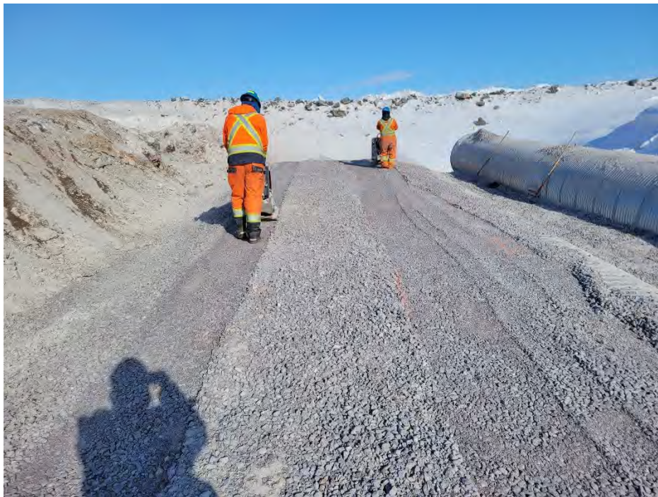
Photo 4 Uncompacted 15 cm (6 inch) layer of 32 mm minus material above the low flow culverts. Photo taken April 7, 2024, facing east.
