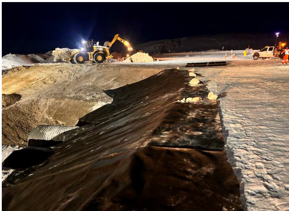
Photo 15 Non-woven geotextile installed on the outlet apron side slopes in preparation of Fine Riprap placement at BG-04. Photo taken April 12, 2024, facing west.
