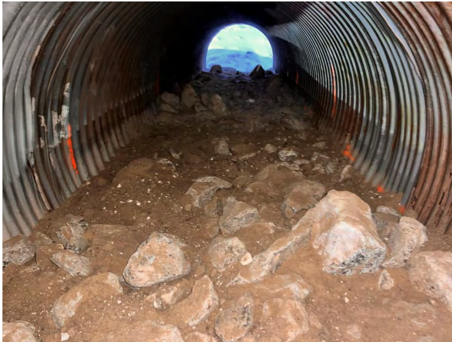
Photo 23 Boulder cluster placement in west low flow culvert at BG-04. Photo taken April 3, 2024, facing inlet.
