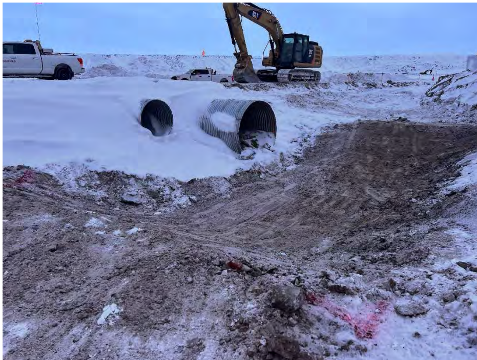
Photo 24 CV-001 excavated inlet apron. Photo taken April 3, 2024, facing northwest.
