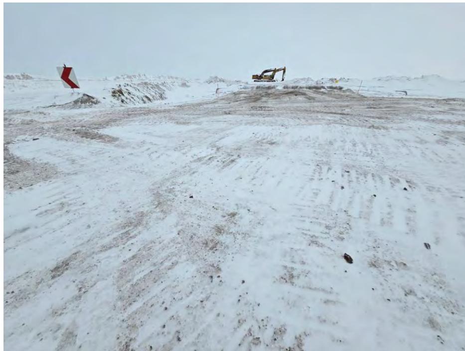
Photo 16 Cleaned approach ramp and above top of 32 mm minus material areas at CV-001 for placing local fill. Photo taken April 2, 2024, facing southeast.
