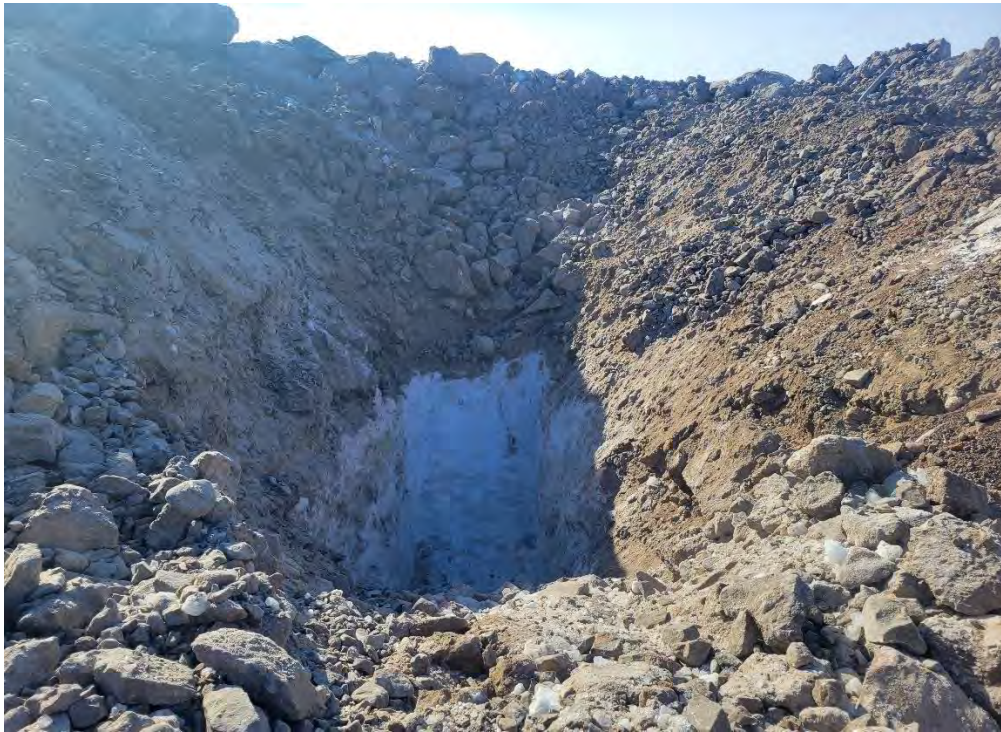
Photo 19 Ice found below the blasted material at CV-216. Photo taken April 12, 2024.
