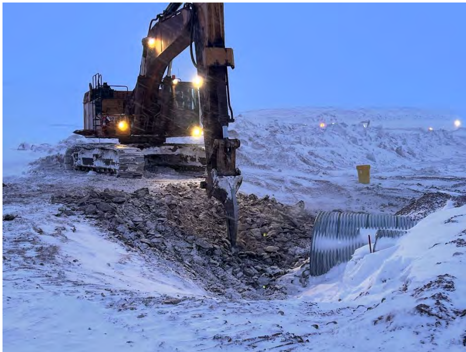
Photo 18 Ripping of outlet culvert apron at CV-001 culvert. Photo taken April 2, 2024, facing west.
