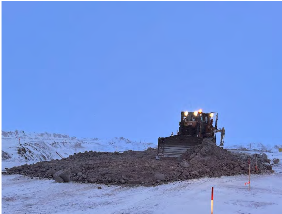
Photo 17 Local fill material placed by dozer over CV-001 culvert. Photo taken April 2, 2024, facing west.
