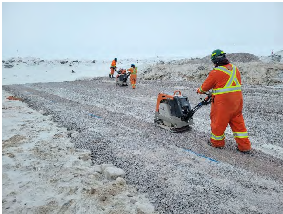
Photo 10 Compaction of 20 cm lift of 32 mm minus material at BG-04. Photo taken April 8, 2024, facing east.
