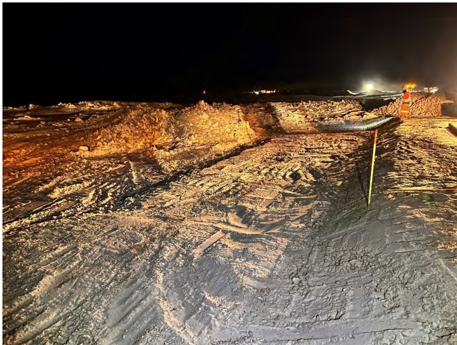
Photo 32 Side slope stabilization surface before Non-Woven Geotextile. Photo taken April 5, 2024, facing northwest.
