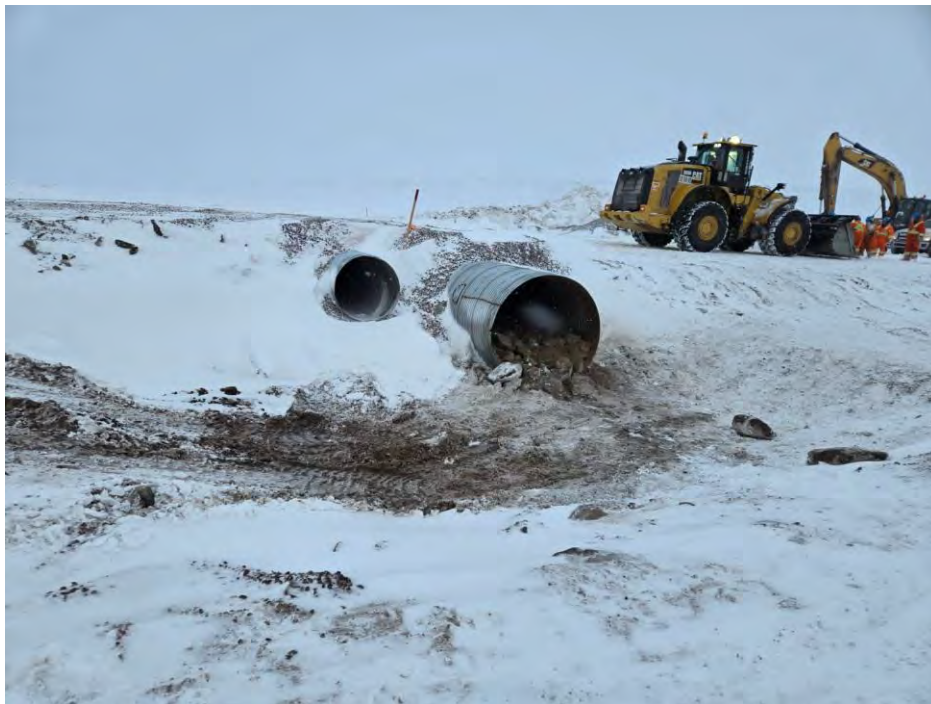
Photo 12 Low flow culvert at CV-001 completely infilled to 0.72 m above the base of the low flow culvert. Photo taken April 1, 2024, facing south.
