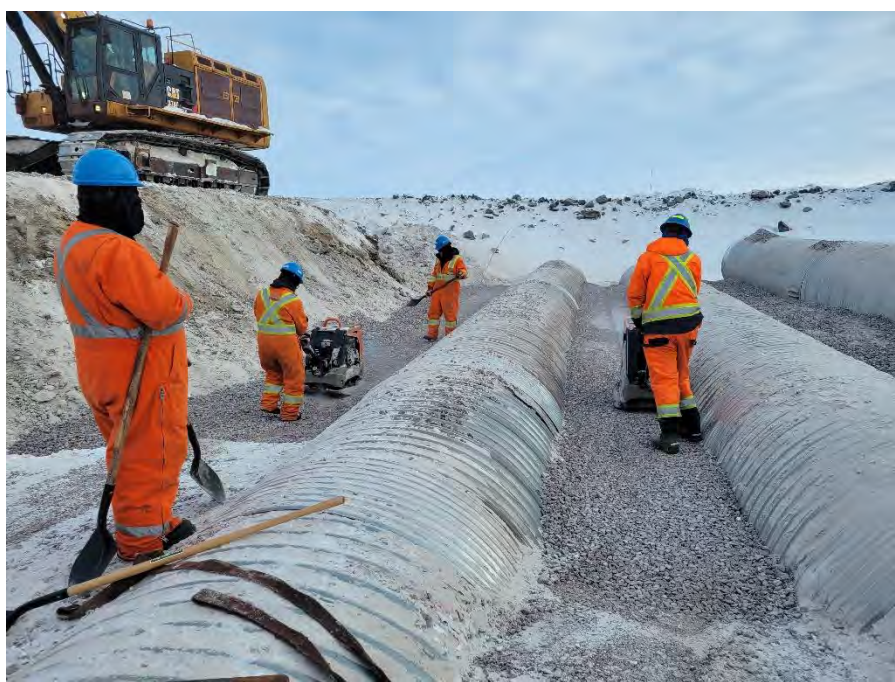
Photo 2 Compaction of 20 cm lift of 32 mm minus material at BG-04. Photo taken April 7, 2024, facing east.
