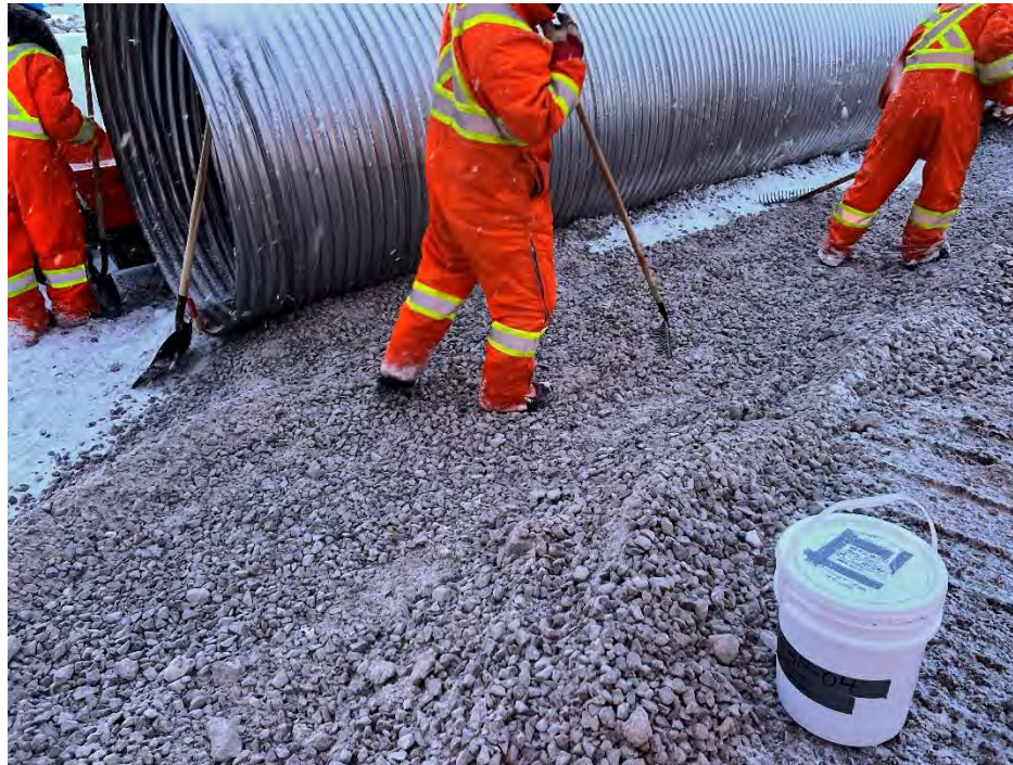
Photo 15 32 mm minus Culvert Backfill Material record sample R-CBF-04 collected from BG-04. Photo taken April 1, 2024, facing northwest behind high flow culvert.
