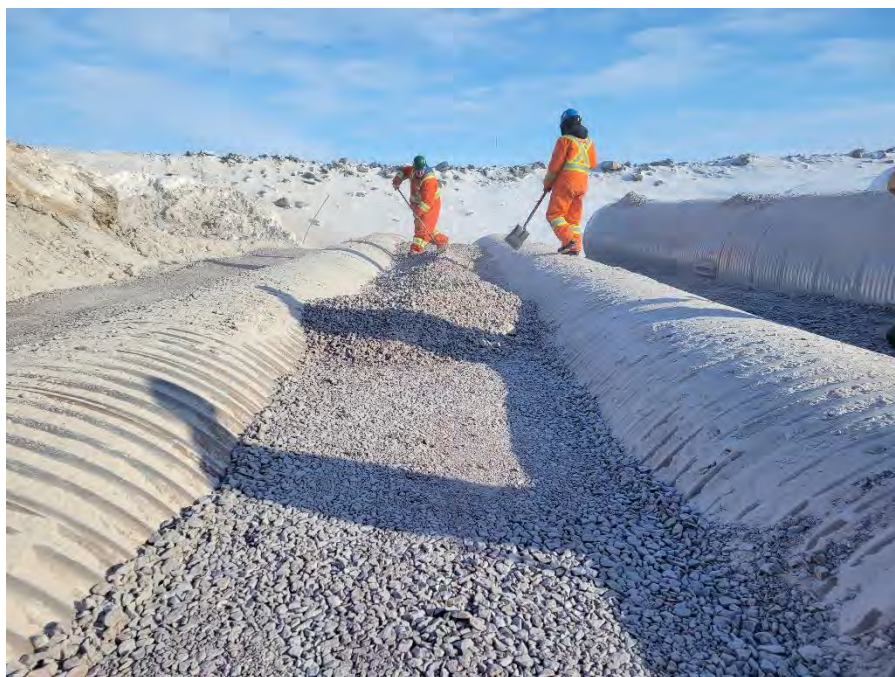
Photo 1 Placement and grading of 20 cm lift of 32 mm minus material at BG-04. Photo taken April 7, 2024, facing east.
