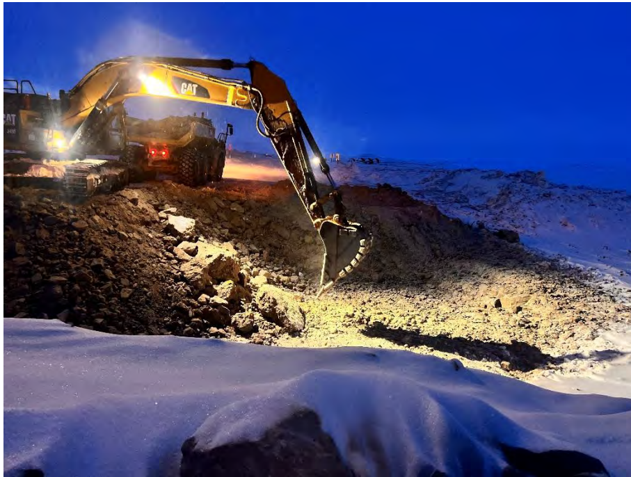
Photo 25 Ongoing excavation of blasted material at CV-216. Photo taken April 13, 2024, facing northbound on the tote road.
