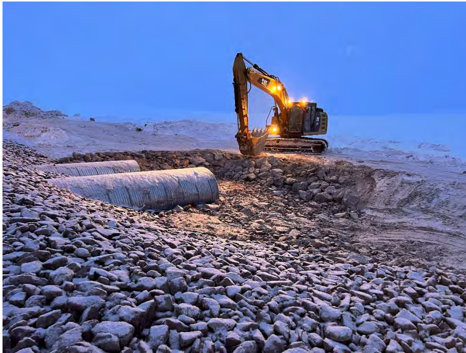
Photo 5 Coarse Riprap mixed with Stream Substrate Material placed for CV-001 outlet apron. Photo taken April 7, 2024, facing southeast.
