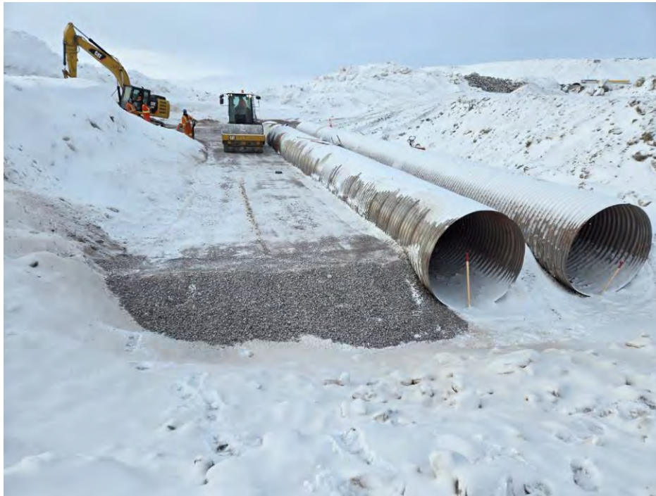
Photo 9 Compacting 32 mm minus material under the high flow CSP culvert location at BG-04. Photo taken April 1, 2024, facing south.
