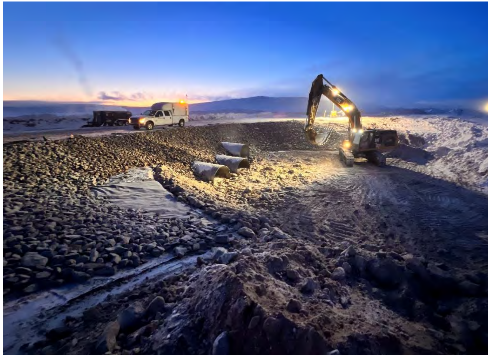
Photo 17 Outlet apron and side slopes at BG-04. Photo taken April 12, 2024, facing east.
