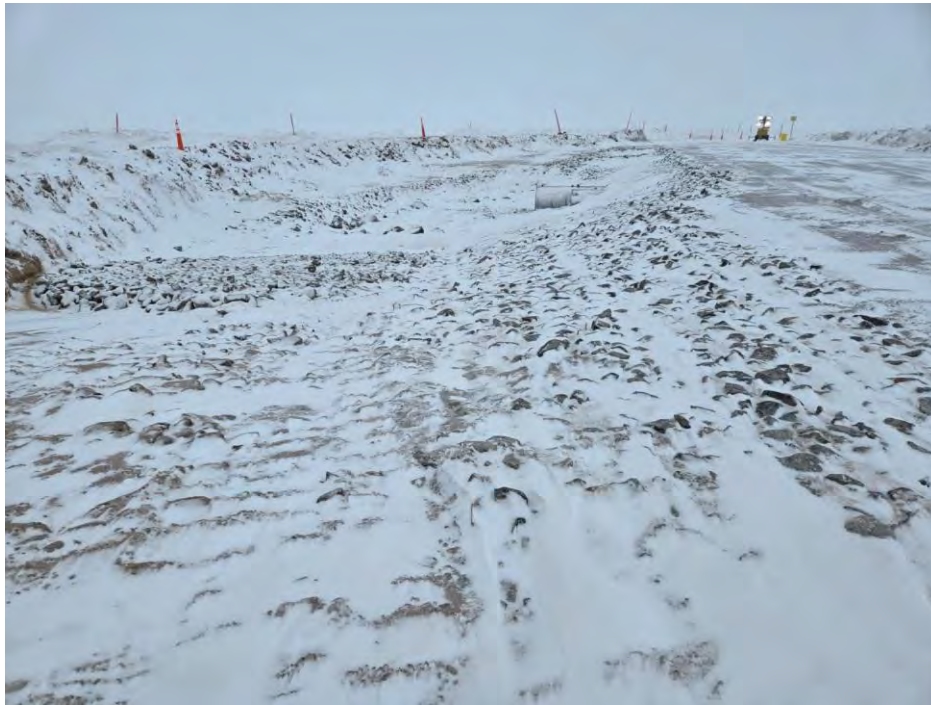
Photo 11 Completed riprap placement in the west apron at CV-059. Photo taken April 1, 2024, facing north.
