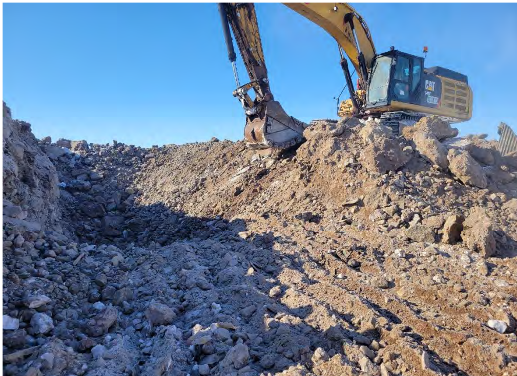
Photo 19 Frozen blasted material being excavated by Nuna at CV-216. Photo taken April 12, 2024, facing southwest.
