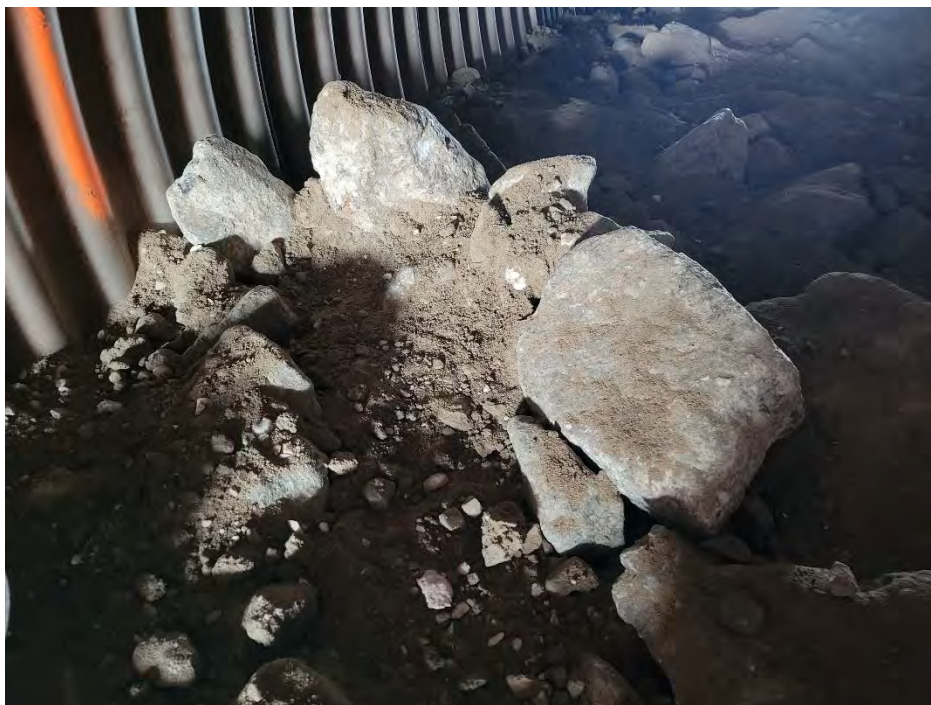
Photo 26 Boulder cluster placement at BG-04. Photo taken April 4, 2024.
