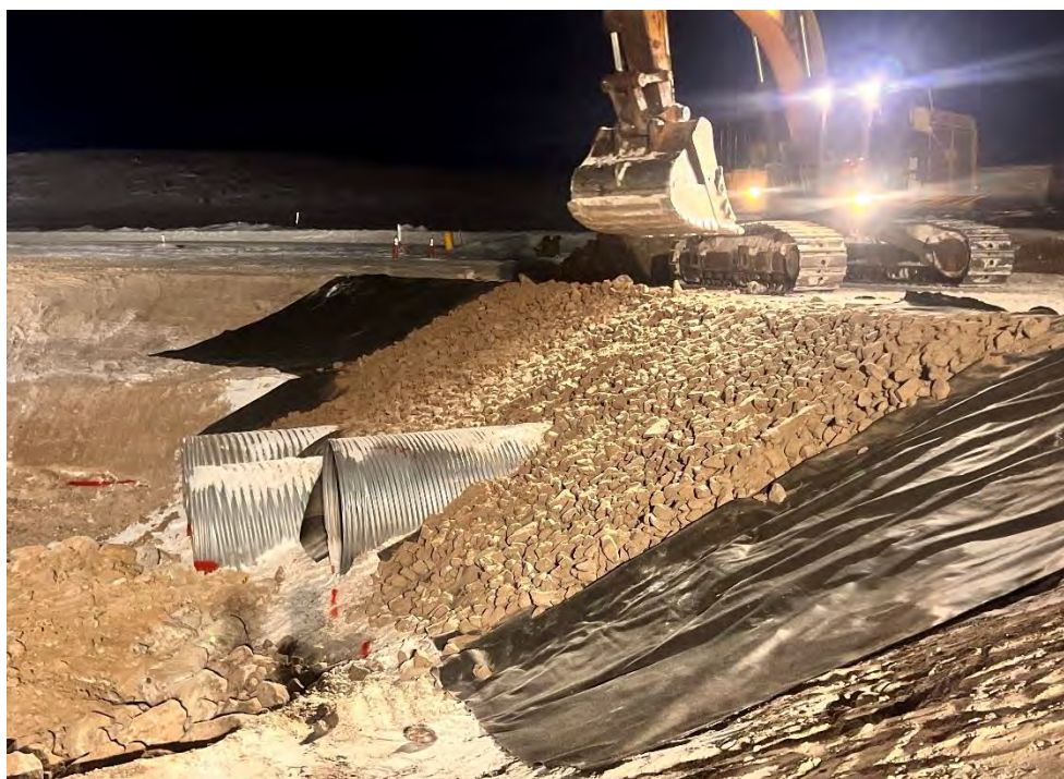
Photo 16 Fine Riprap placement on top of non-woven geotextile installed on the outlet apron side slopes at BG-04. Photo taken April 12, 2024, facing west.
