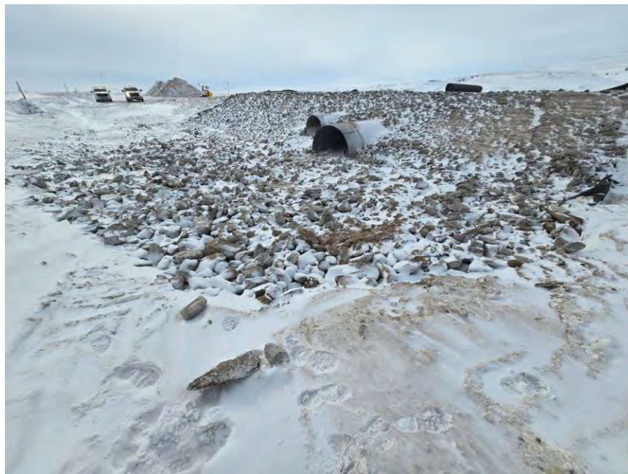
Photo 2 East apron area complete with coarse riprap mixed with stream substrate material at CV-057. Photo taken March 31, 2024, facing south.
