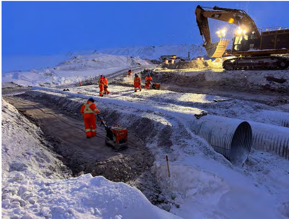
Photo 9 Local borrow area fill and 32 mm minus Culvert Backfill placement and compaction at BG-04. Photo taken April 7, 2024, facing southeast.
