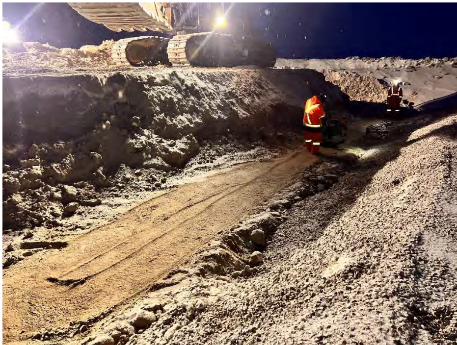
Photo 6 Local borrow area fill placement and compaction against the 32 mm minus Culvert Backfill Material on the west side of the low flow culverts at BG-04. Photo taken April 7, 2024, facing north.
