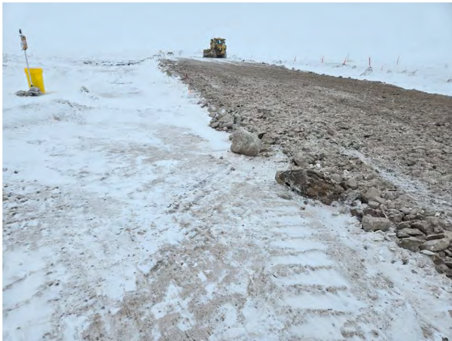
Photo 10 Placed and graded local fill material for the construction of the south approach ramp at CV057. Photo taken April 1, 2024, facing north.
