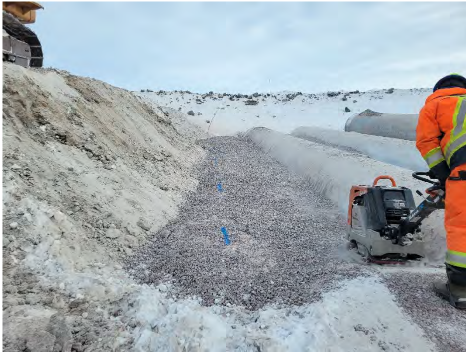
Photo 3 Edge of 32 mm minus material trapezoid marked out in blue paint. Photo taken April 7, 2024, facing east.
