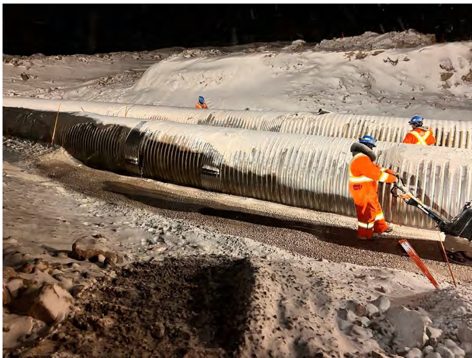
Photo 8 Compaction of 32 mm minus culvert backfill lift on south side at BG-04. Photo taken March 31, 2024, facing northeast.
