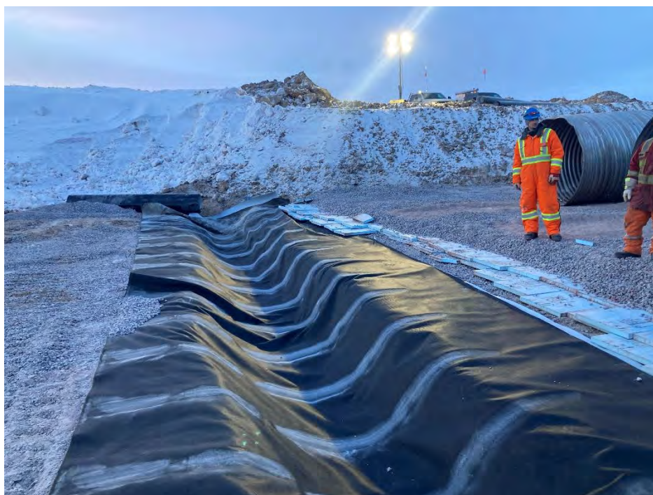
Photo 6 Second layer of plug (geotextile) placed atop the geomembrane in the outlet trench at CV-216. Photo taken April 23, 2024, facing east.
