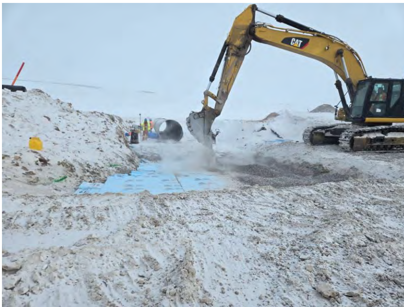
Photo 4 Placement of 32 mm minus material over installed insulation in the western apron area at CV-102. Photo taken April 29, 2024, facing east.
