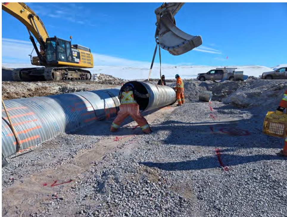
Photo 6 Installation of third segment of 1.0 m diameter high flow CSP culvert at CV-106. Photo taken May 7, 2024, facing east.
