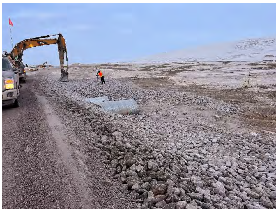
Photo 17 Outlet apron area infilled with Coarse Riprap and 3/16 inch material at CV-106. Photo taken May 11, 2024, facing south.
