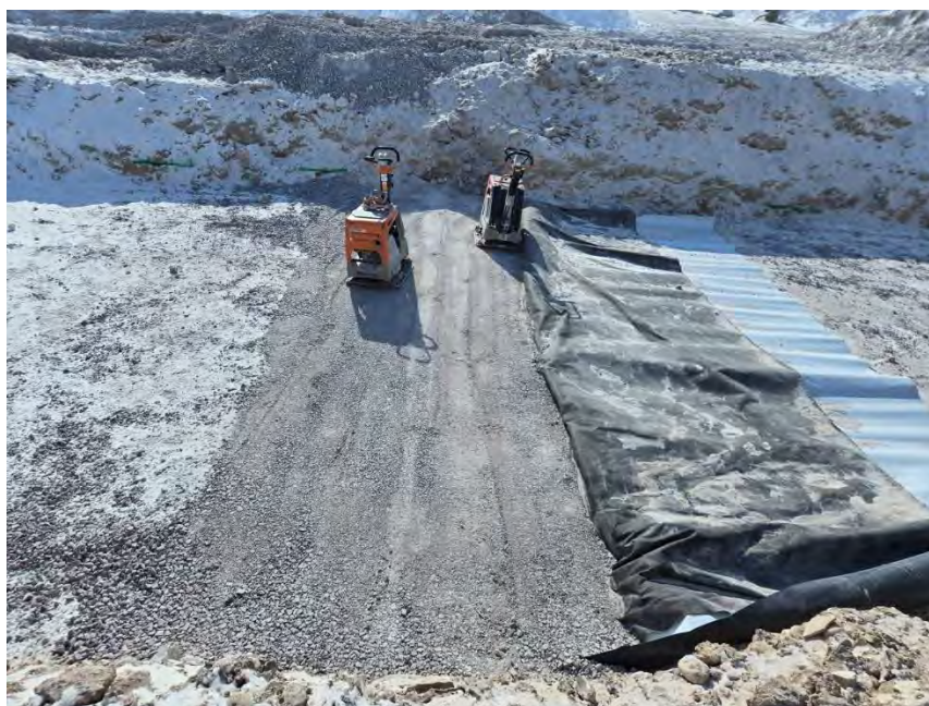
Photo 11 Backfilled and compacted anchor-trench with \frac{3}{4} inch minus material at CV-102. Photo taken April 26, 2024, facing south.
