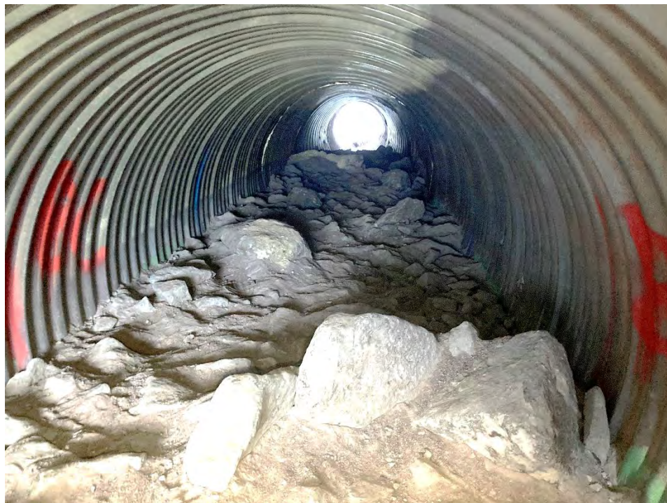
Photo 6 Boulder clusters installed at 6.5 m interval with embedded protruding boulders between clusters within the northern low flow culvert at CV-216. Photo taken April 30, 2024, facing upstream.
