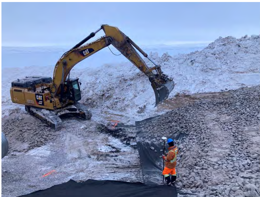
Photo 11 Placement of fine riprap on the northeastern apron side slopes at CV-216. Photo taken May 2, 2024, facing north.
