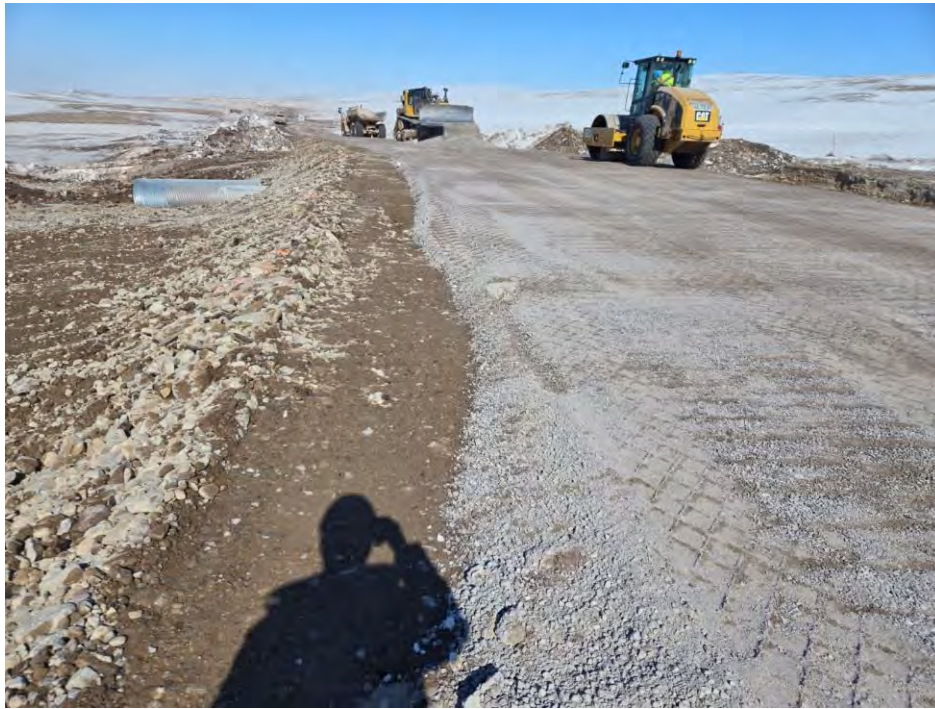
Photo 9 Placing and compacting 3/4 inch road topping material at CV-106. Photo taken May 8, 2024, facing north.
