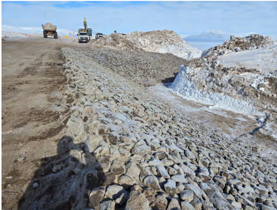
Photo 15 Northwest outlet apron side slopes stabilized with non-woven geotextile and fine riprap at CV-216. Photo taken May 4, 2024, facing northwest.
