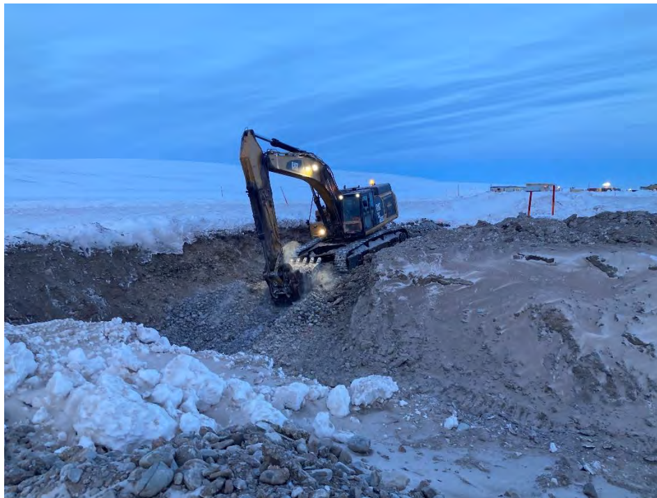
Photo 16 Excavation of unsuitable materials from the inlet apron area at CV-106. Photo taken May 4, 2024, facing southeast.
