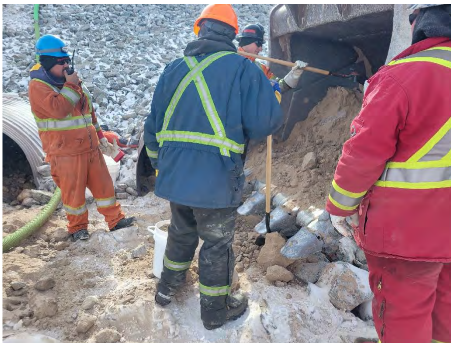
Photo 1 Placement of addition Stream Substrate Material in the low flow culverts at BG-04. Photo taken April 21, 2024, facing south.
