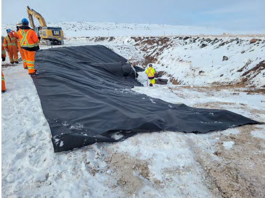
Photo 4 Placement of non-woven geotextile on the upstream slope of BG-04. Photo taken April 16, 2024, facing northwest.
