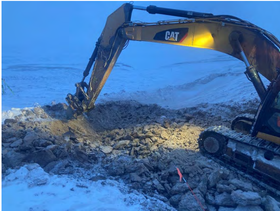
Photo 13 Ripping and excavation of the western outlet apron at CV-106. Photo taken May 3, 2024, facing northwest.
