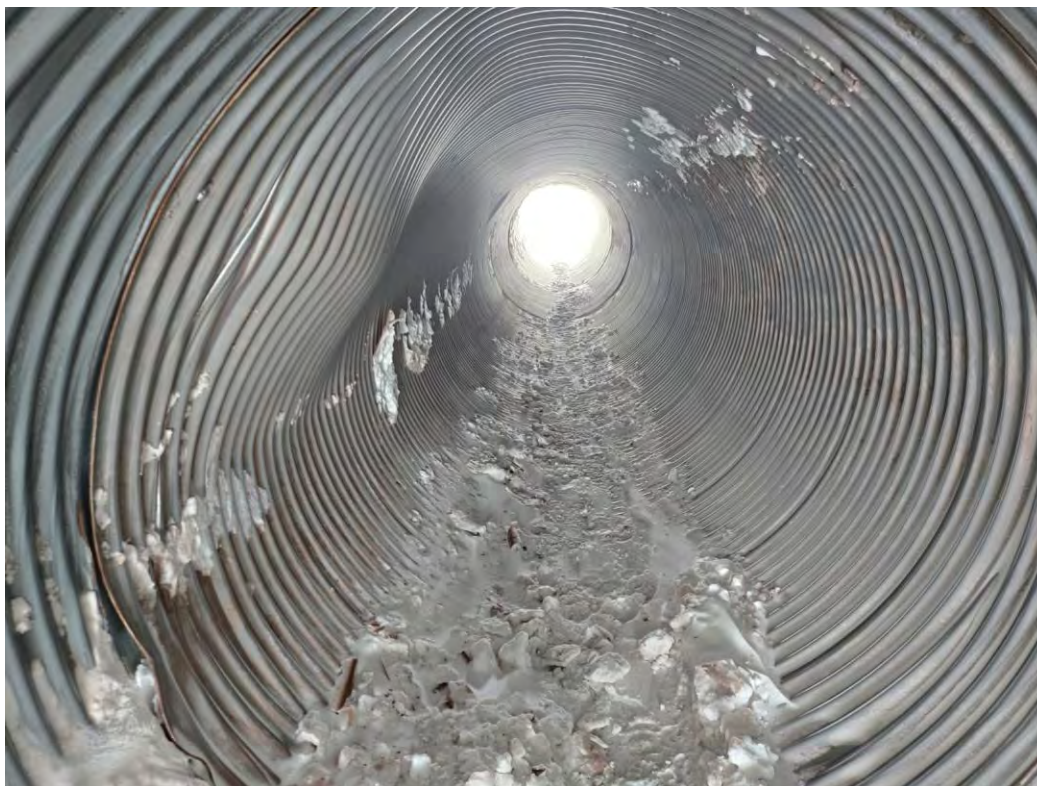
Photo 3 Dent in northern high flow CSP culvert at CV-216. Photo taken morning of April 29, 2024, facing northeast (outlet).
