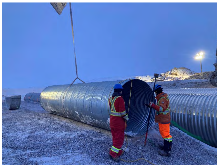
Photo 10 Installation of the first 8.0 m long segment of the eastern 1.8 m diameter high flow CSP culvert at CV-216. Photo taken April 25, 2024, facing northeast.
