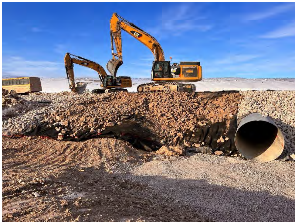
Photo 12 Placement of Fine Riprap on Non-Woven Geotextile on graded 2H:1V side slopes at CV-106. Photo taken May 10, 2024, facing east.
