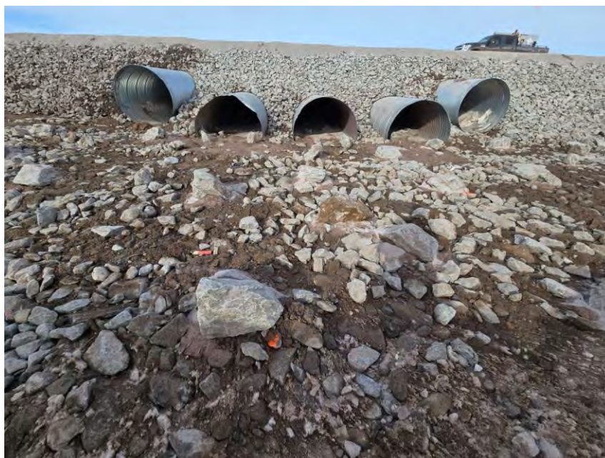
Photo 2 Completed inlet apron area and culvert inverts at CV-216. Photo taken May 5, 2024, facing east.
