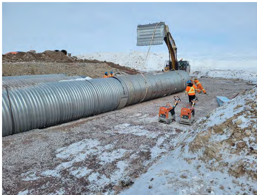
Photo 5 Installation of the second 9.0 m long segment of the 2.0 m diameter low flow CSP culverts at CV-216. Photo taken April 23, 2024, facing south.
