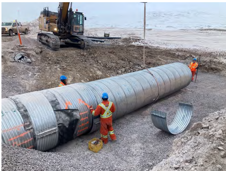
Photo 5 Installation of fourth and final 8.0 m long segment of the 1.8 m diameter low flow CSP culvert at CV-106. Photo taken May 6, 2024, facing southwest.
