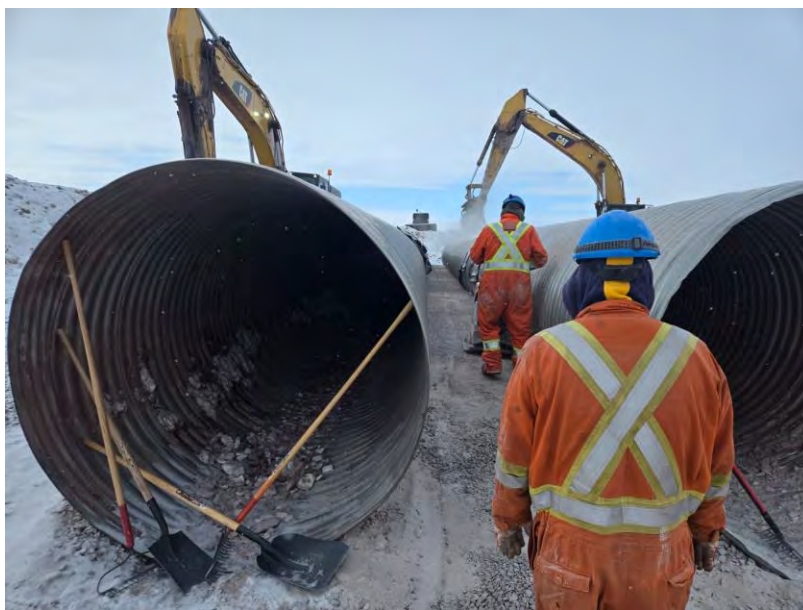
Photo 9 Compacting second lift of culvert backfill material between placed low flow CSP culverts at CV-216. Photo taken April 25, 2024, facing southwest.
