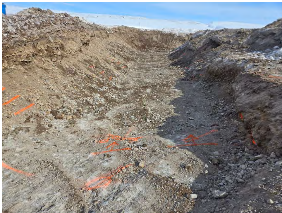
Photo 1 Approved foundation surface of the road crossing area at CV-106. Photo taken May 5, 2024, facing east.
