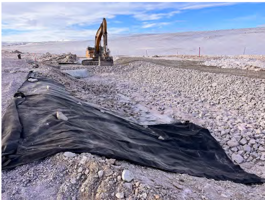
Photo 15 Non-Woven Geotextile placed on 2H:1V side slopes and thermal berm within the inlet apron area at CV-106. Photo taken May 11, 2024, facing north.
