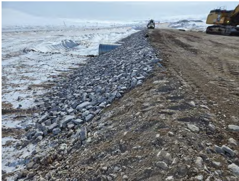
Photo 14 Eastern side slopes with geotextile and fine riprap placed at CV-102. Photo taken May 4, 2024, facing south.
