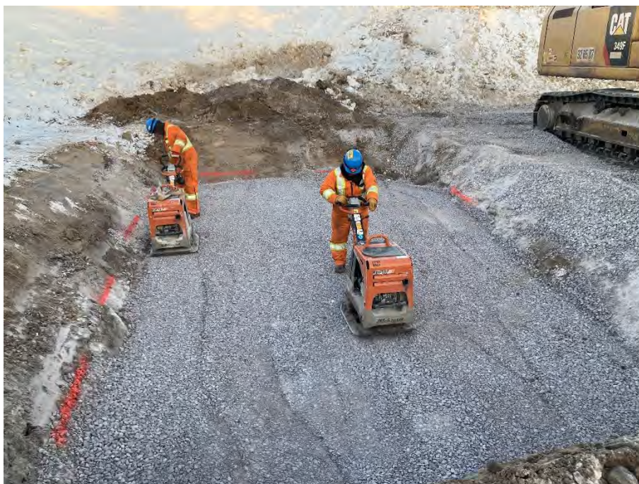
Photo 2 Compaction of 32 mm minus material at the outlet apron at CV-216. Photo taken April 21, 2024, facing east.
