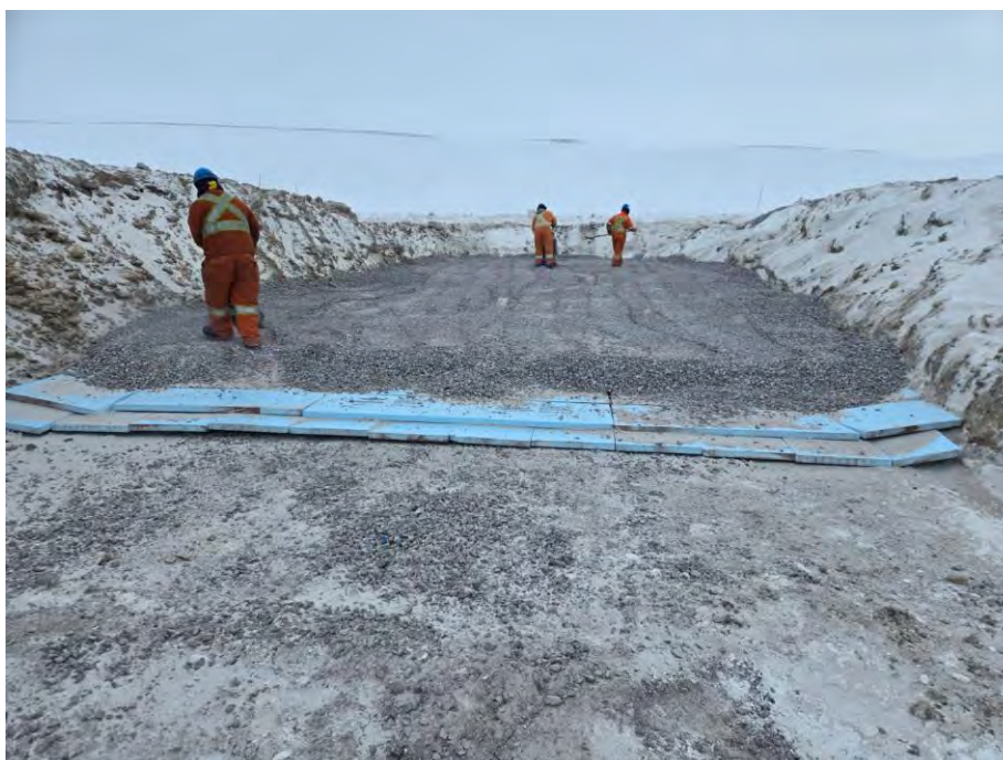
Photo 14 Compaction of the first 200 mm lift of 32 mm minus material above insulation at CV-102. Photo taken April 27, 2024, facing east.
