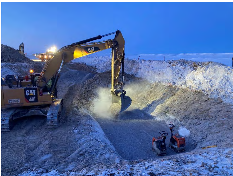
Photo 10 Placement of 32 mm minus material at the inlet apron at CV-216. Photo taken April 18, 2024, facing southeast.
