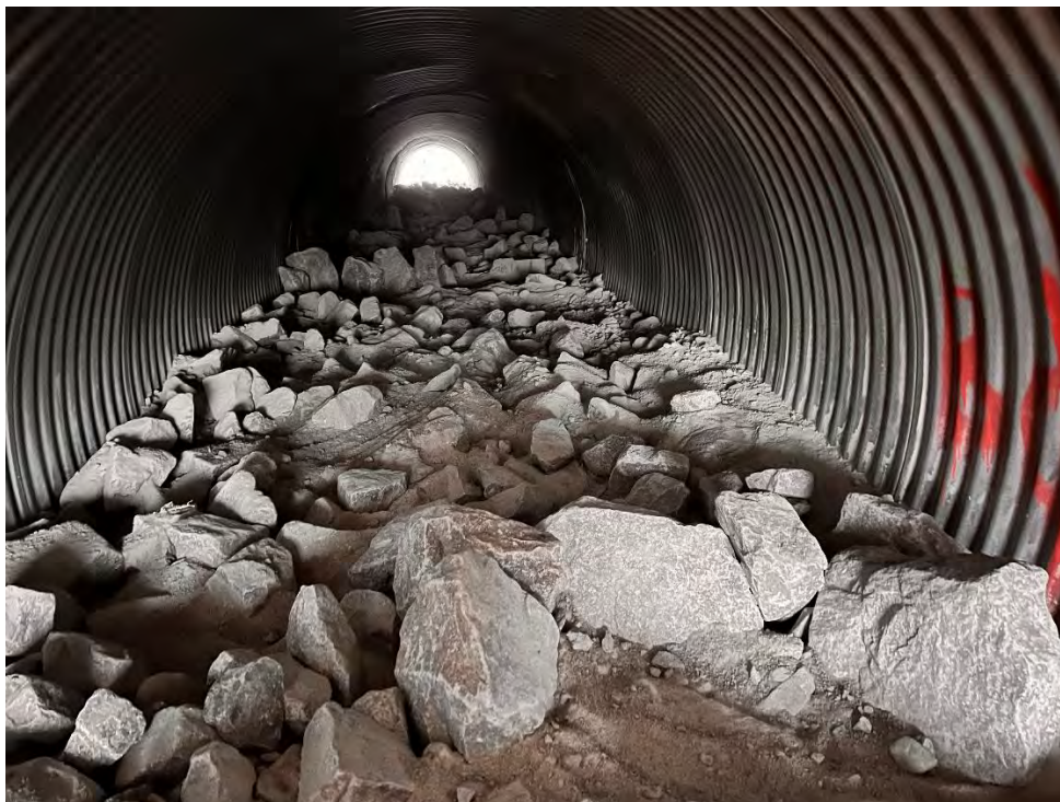
Photo 16 Infilled 1.8 m diameter low flow CSP culvert complete with boulder clusters at CV-106. Photo taken May 11, 2024, facing upstream.
