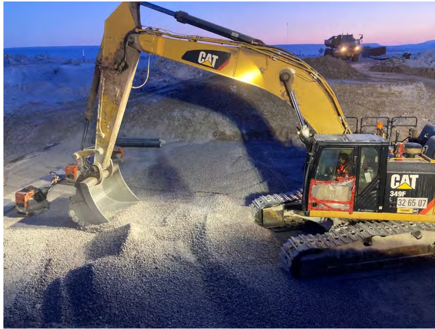
Photo 15 Placement of 32 mm minus material at the CV-216 road crossing area. Photo taken April 20, 2024, facing west.
