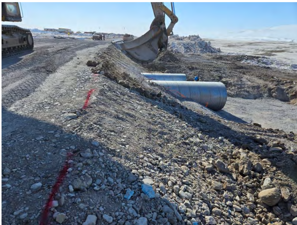
Photo 11 Grading 2H:1V side slopes at CV-106. Photo taken May 9, 2024, facing south.
