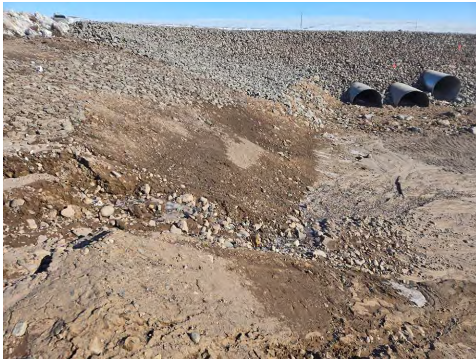
Photo 10 Rill erosion and sediment fan deposition in outflow environment on southwest side slopes at BG-04. Photo taken May 9, 2024, facing north.
