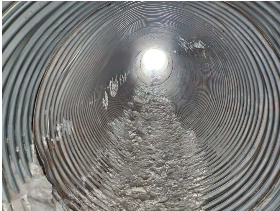
Photo 5 Pushed out dent in the northern high flow CSP culvert at CV-216. Photo taken April 30, 2024, facing downstream.
