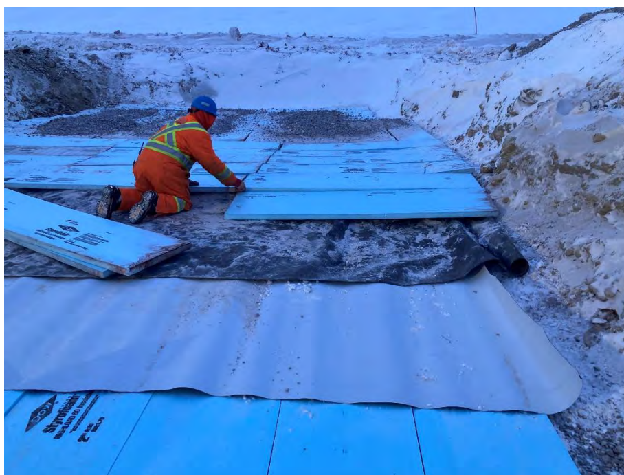
Photo 12 Installation of the insulation material layered with the excess geomembrane and geotextile material from the geomembrane anchor-trench at CV-102. Photo taken April 26, 2024, facing east.
