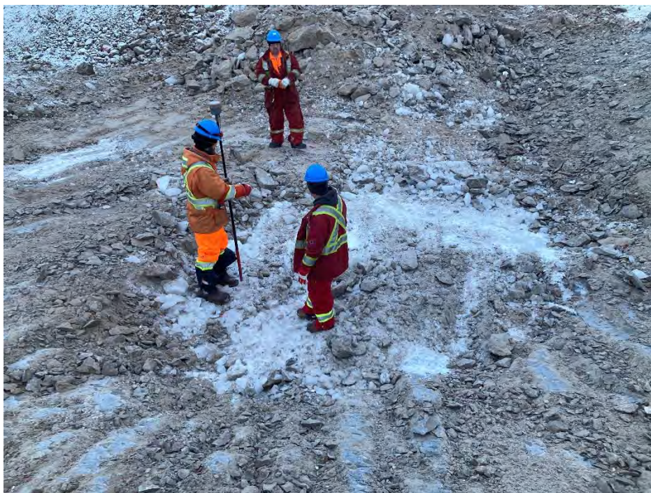
Photo 8 Ice encountered in the inlet excavation area at CV-216. Photo taken April 18, 2024, facing southeast.
