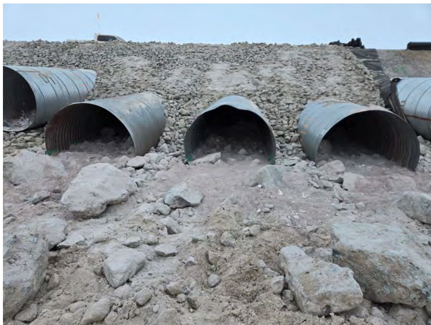
Photo 12 Outlet low flow CSP culverts and outlet apron area at CV-216. Photo taken May 3, 2024, facing southwest.
