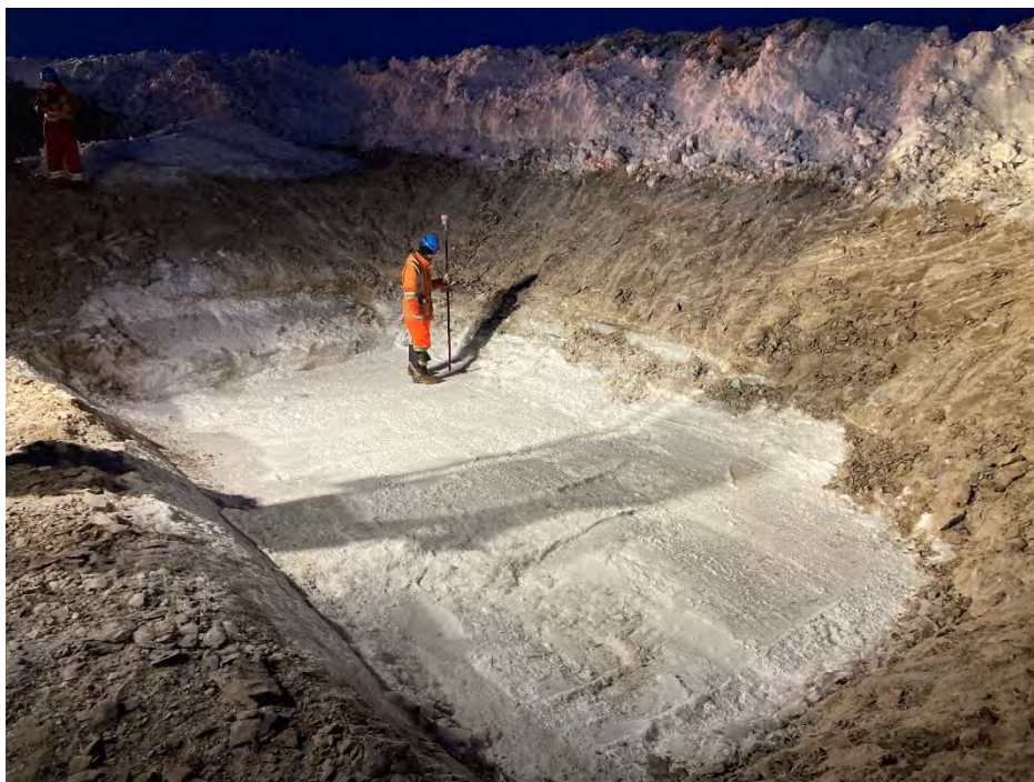
Photo 9 Approval foundation surface at the inlet apron at CV-216. Photo taken April 18, 2024, facing southeast.
