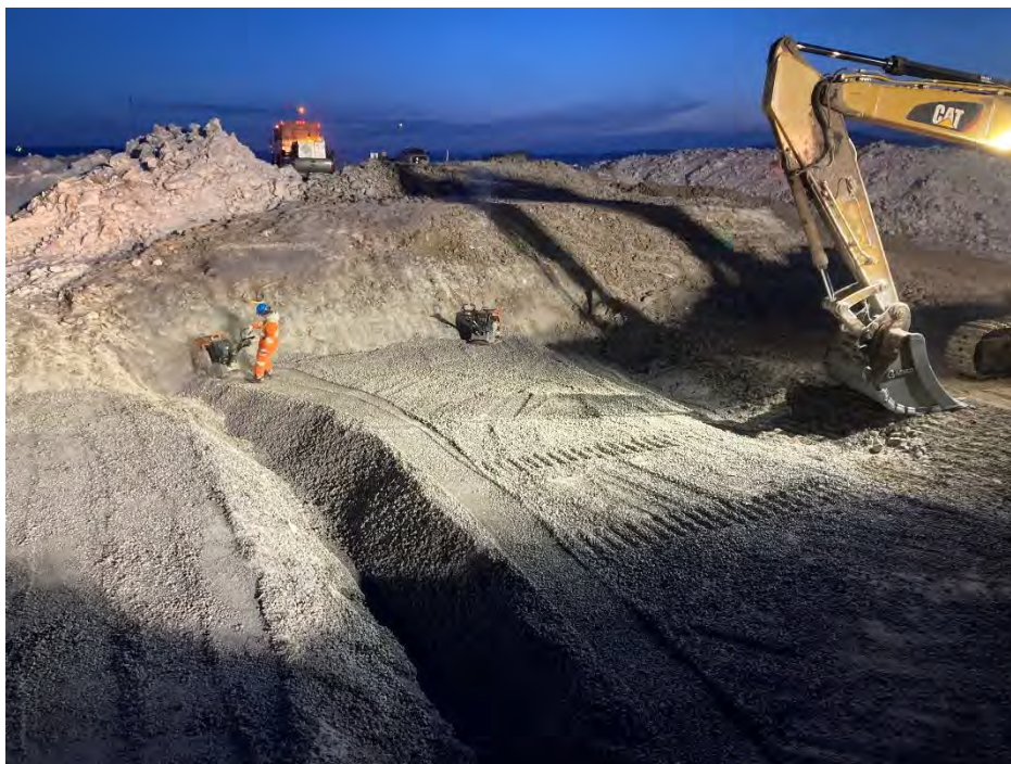
Photo 13 Compaction of 32 mm minus material and location of geomembrane/geotextile key in trench at the inlet of CV-216. Photo taken April 19, 2024, facing northwest.
