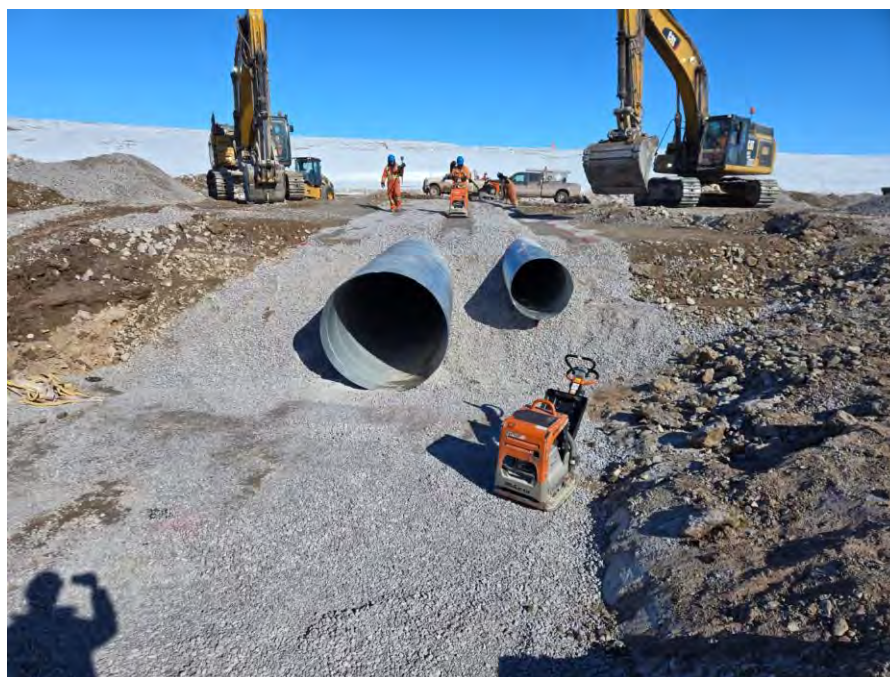
Photo 7 Compacting 32 mm minus material between low and high flow CSP culverts with uncompacted 150 mm zone above the culverts at CV-106. Photo taken May 7, 2024, facing east.
