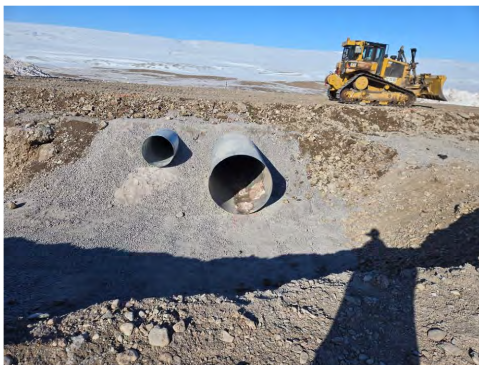
Photo 8 Placing local fill material above the compacted 32 mm minus material and constructing approach ramps at CV-106. Photo taken May 8, 2024, facing west.
