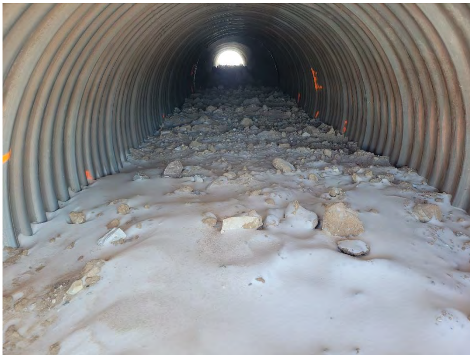
Photo 2 Lack of Boulder Clusters and Protruding Boulders in the southern half of the low flow culverts at BG-04.
