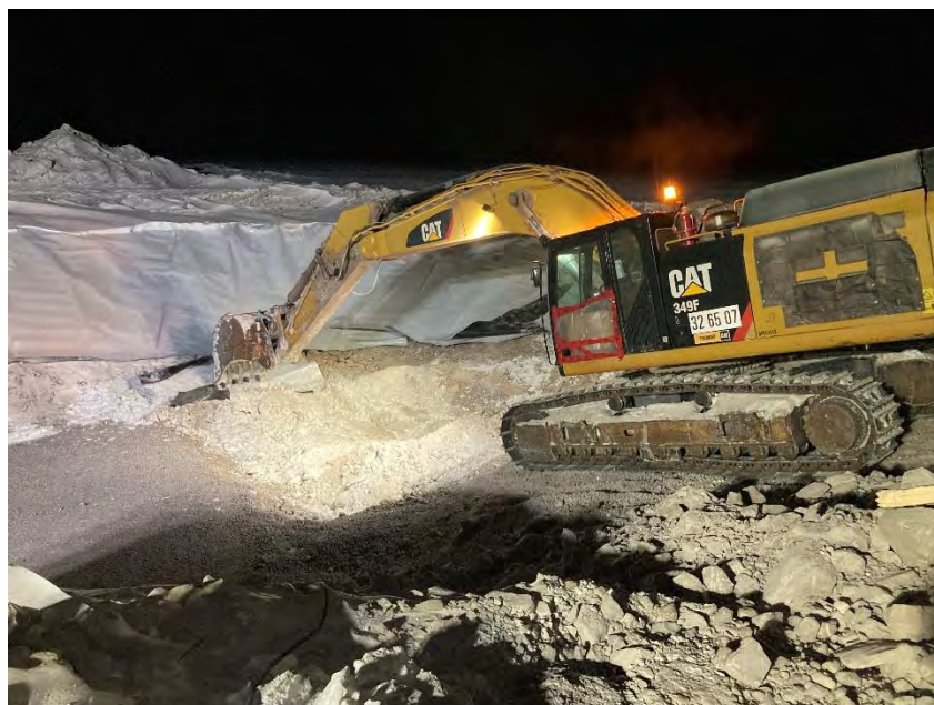
Photo 6: Excavating unsuitable materials within Section 3. Photo taken March 14, 2024.
