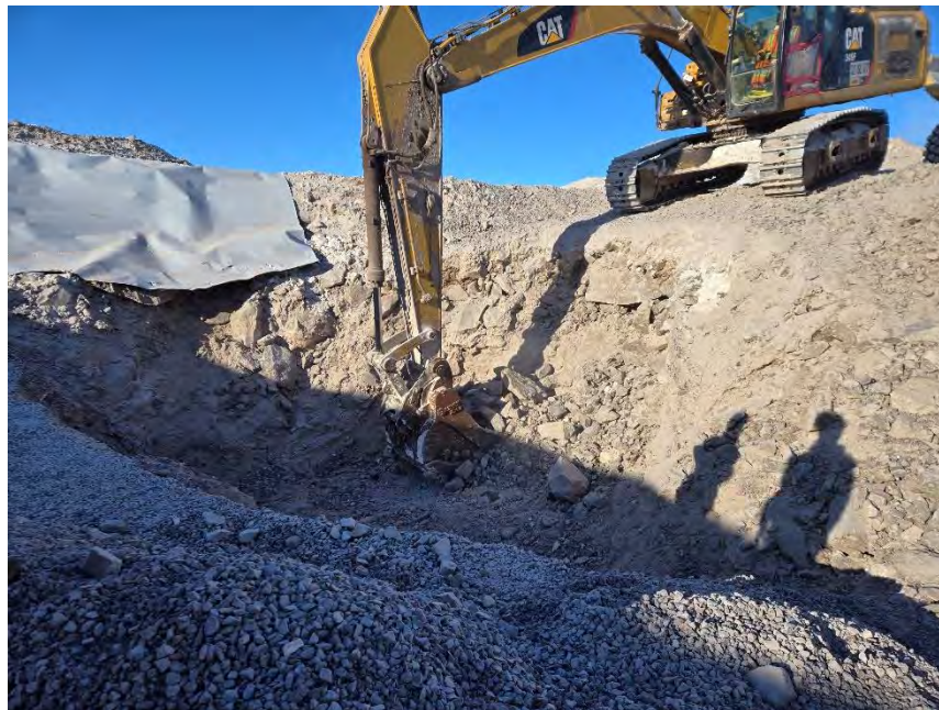
Photo 7: Excavating unsuitable materials within Section 4. Photo taken March 15, 2024.
