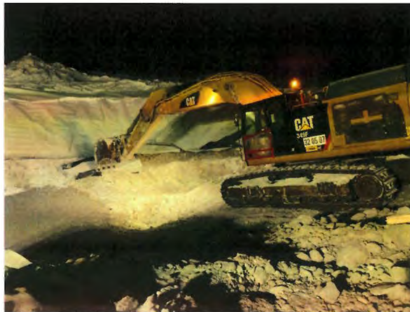
Photo 6: Excavating unsuitable materials within Section 3. Photo taken March 14, 2024.
