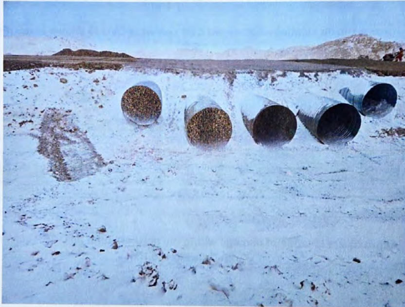
Photo 2 Northern high flow CSP culvert backfilled at CV-216. Photo taken April 29, 2024, facing northeast.
