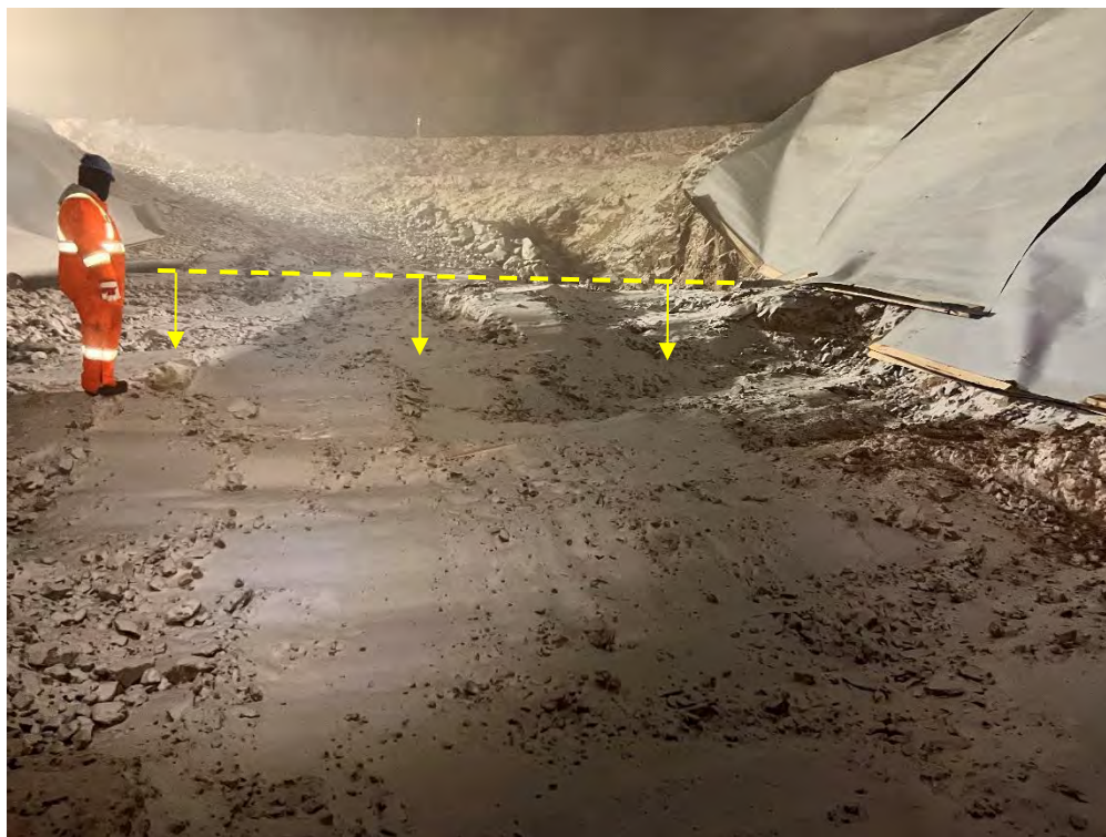
Photo 5 Approximate Subgrade Acceptance Area. Photo taken March 4, 2024.
