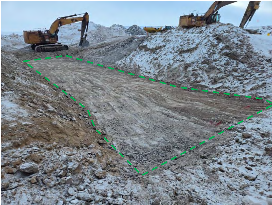
Photo 2 Prepared foundation surface at BG-04 highlighted in green. Photo taken March 28, 2024, looking south.
