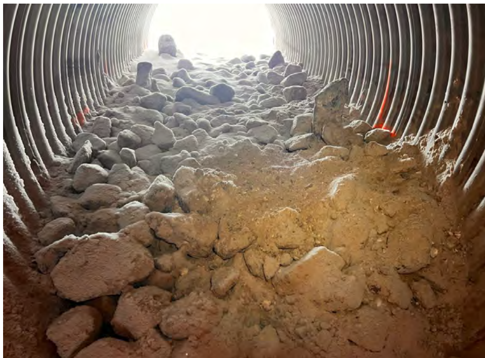
Photo 1 Placed Culvert Infill Material in the east low flow culvert at BG-04 (Facing Inlet)
