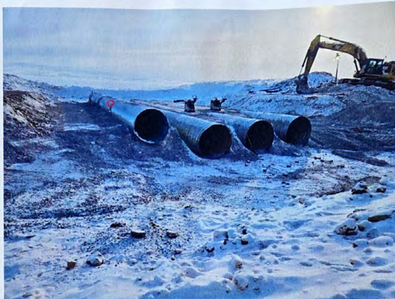
Photo 1 Northern high flow CSP culvert installed at CV-216, location of future damage approximated in red. Photo taken April 26, 2024, facing east.
