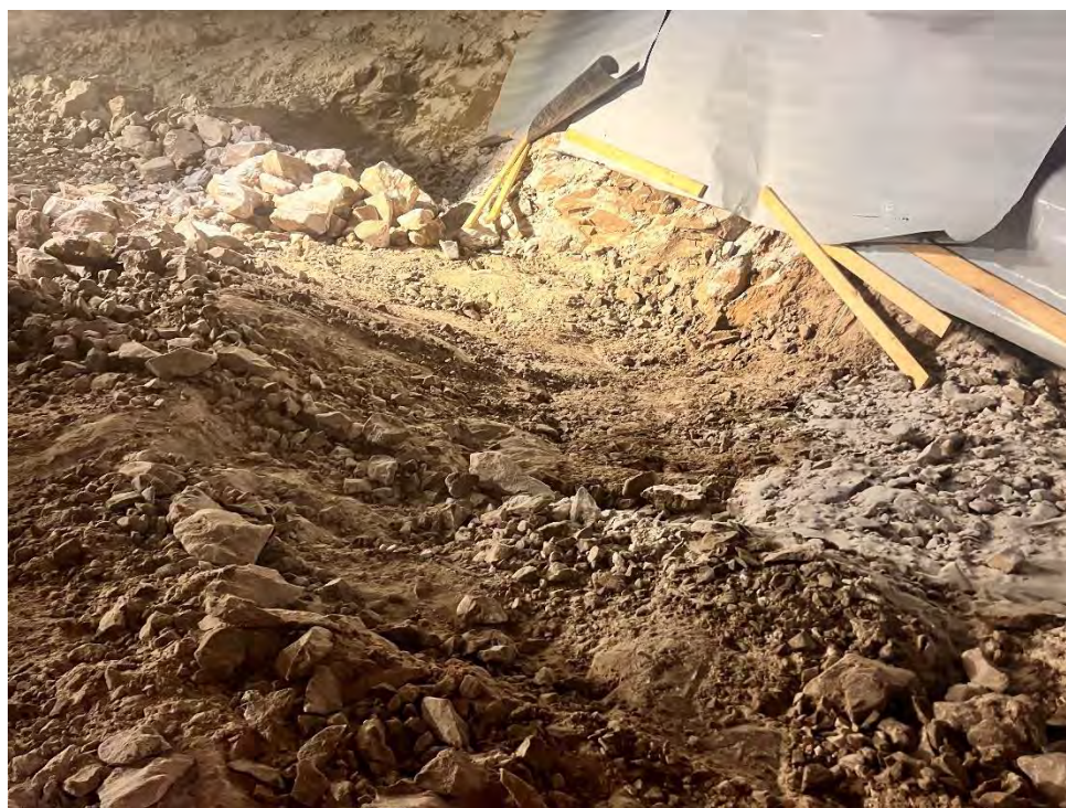
Photo 4 Cleared area with excavator prior to Foundation Acceptance. Photo taken March 4, 2024.
