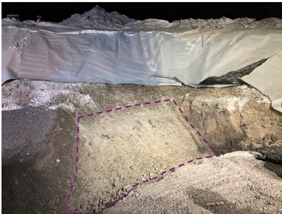
Photo 3: Approximate Foundation Acceptance Area - Section 3, outlined in purple. Photo taken March 14, 2024.
