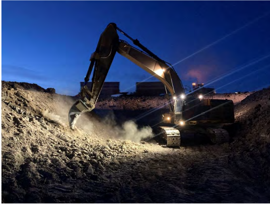
Photo 1 Ripping excavation surface for foundation preparation at BG-04. Photo taken March 26, 2024.
