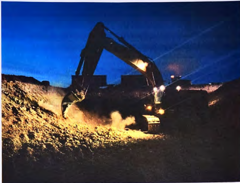
Photo 1 Ripping excavation surface for foundation preparation at BG-04. Photo taken March 26, 2024.
