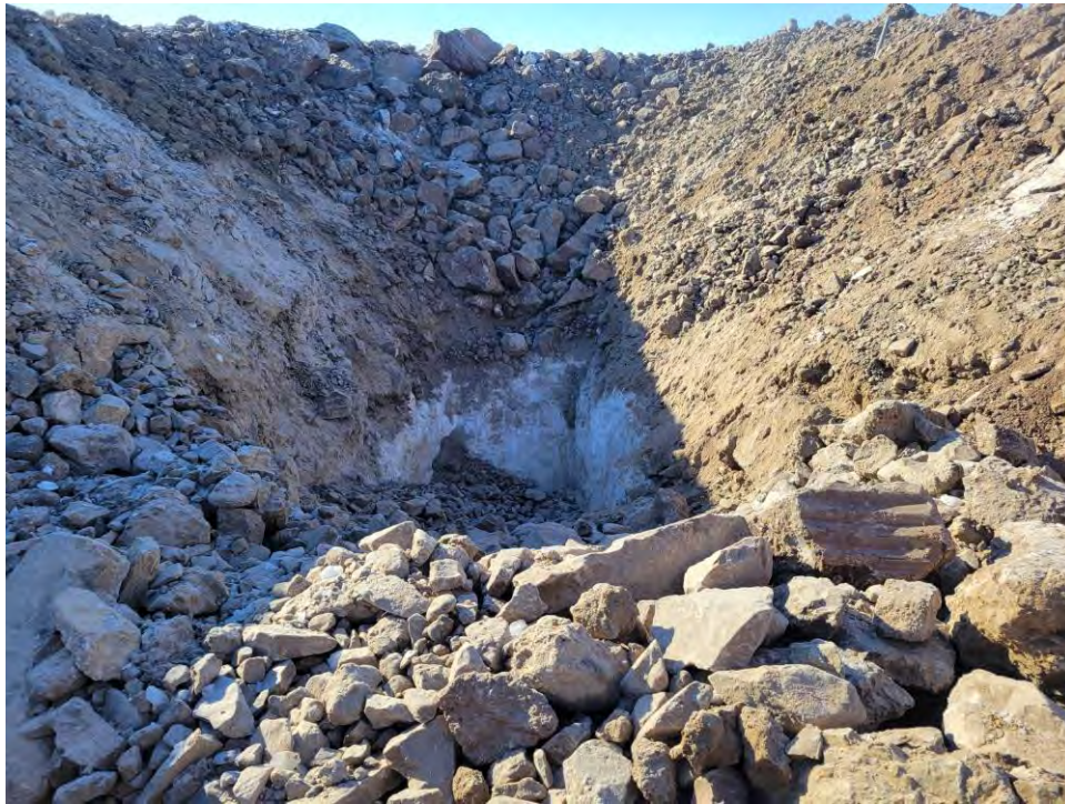
Photo 1 Looking at the Initial Discovery of Massive Ice at CV-216
