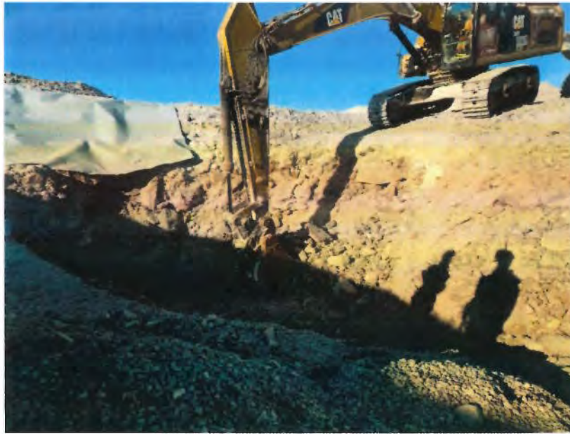
Photo 7: Excavating unsuitable materials within Section 4. Photo taken March 15, 2024.
