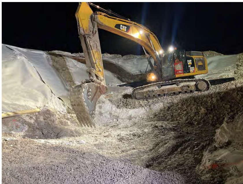
Photo 5: Excavating unsuitable materials within Section 2. Photo taken March 14, 2024.
