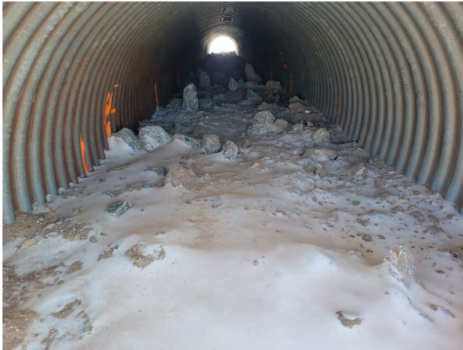
Photo 1 Boulder Clusters and Protruding Boulders (inadequately sized boulders) in the southern half of the low flow culverts at BG-04.
