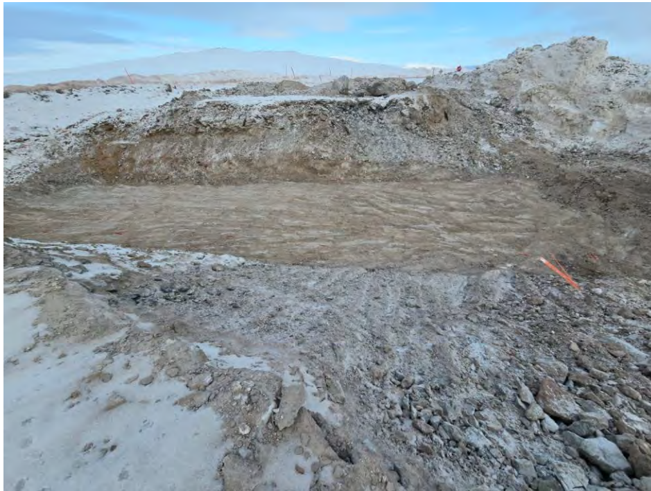
Photo 3 Prepared foundation surface at BG-04. Photo taken March 28, 2024, looking east.
