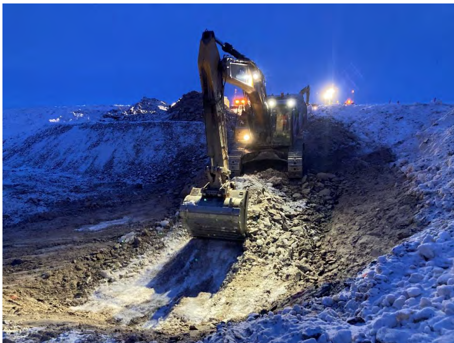
Photo 1 Excavating unsuitable materials within Section 1 at CV-216 inlet apron. Photo taken April 18, 2024, looking east.
