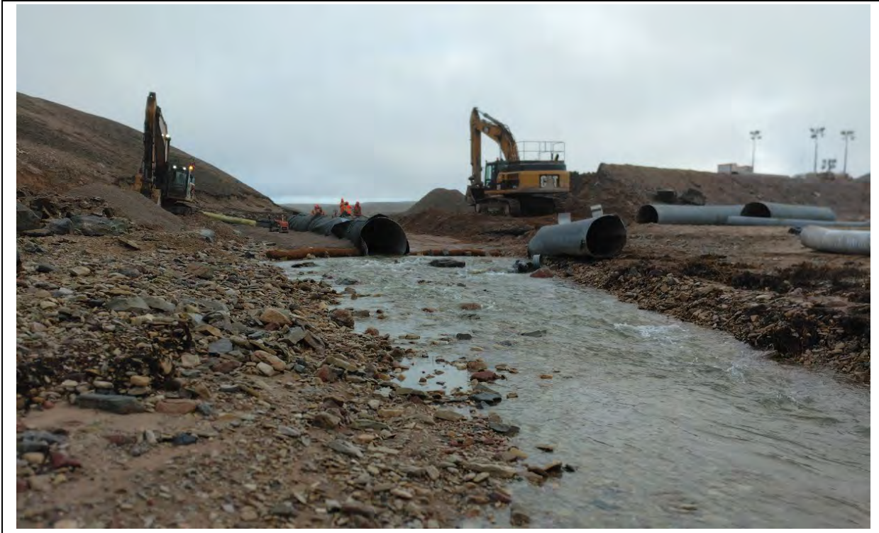
Photo 9. KM 63.5, looking west at crossing, 2024-09-27 1800mm culvert and ESC Installed.
