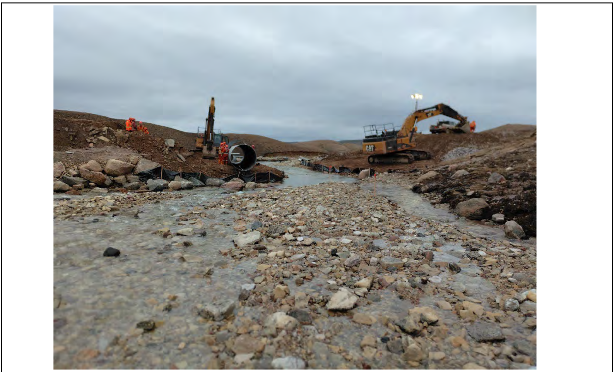
Photo 8. KM 63.5, east of crossing, 2024-09-26, 1800mm culvert staged for assembly.
