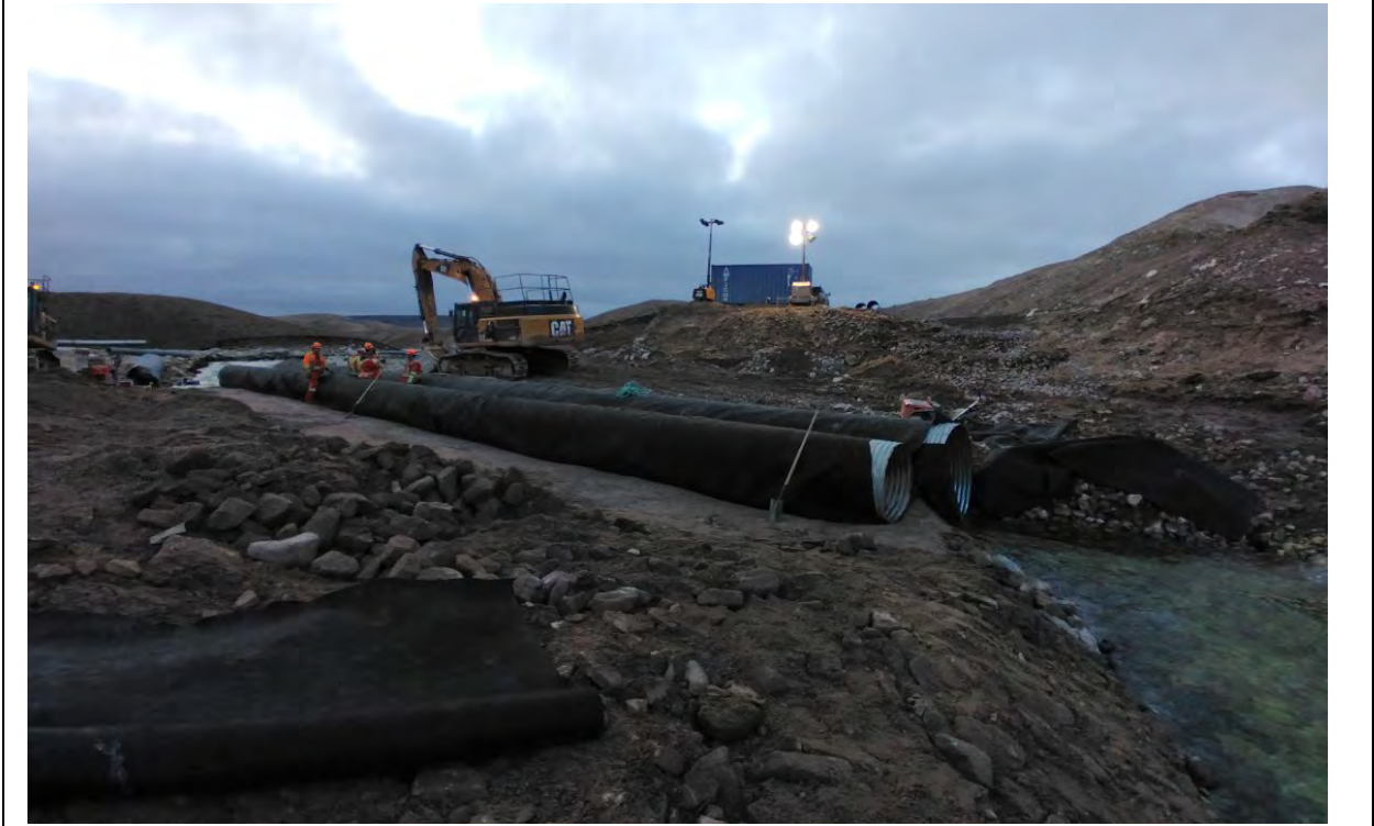
Photo 11. KM 63.5, looking northwest at crossing, 2024-09-27, high flow culvert installed.
