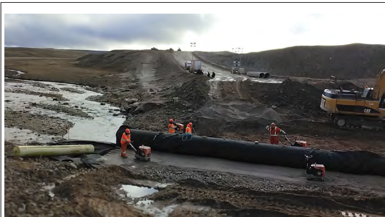
Photo 9. KM 63.5, looking west at crossing, 2024-09-27 1800mm culvert and ESC Installed.
