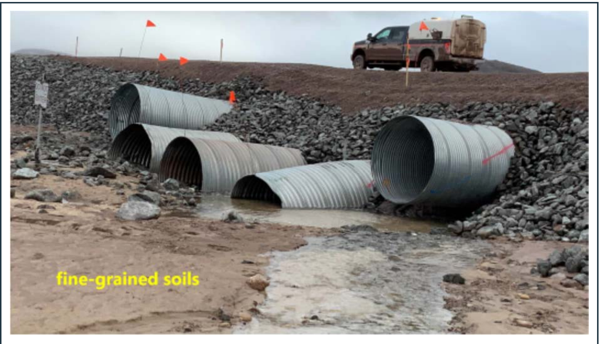
Figure 110: View of the inlet of five culverts at KM 80+500. All five culverts suffered serious differential settlements (sagging) and all of them will need to be replaced as soon as practically possible.
