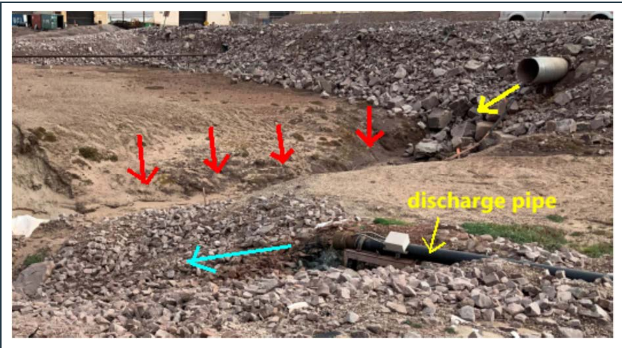
Figure 85: View of the end of the water discharge pipe (blue arrow) and a nearby culvert (yellow arrow) draining water to the same valley. More ripraps should be placed into the upper section of the valley, marked by red arrows, to prevent erosion of the valley floor and side-slopes.
