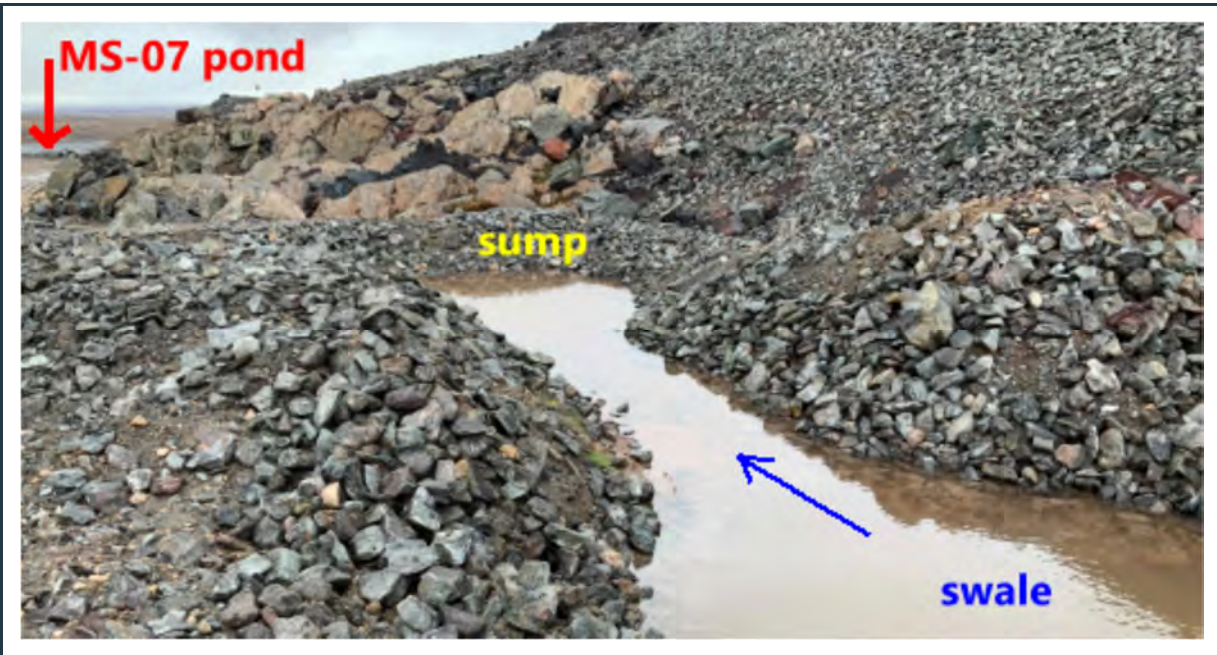
Figure 52: View of the new drainage ditch/swale and sump pit south of the KM-106 ore stockpile area, collecting local run-off. Note the recently completed riprap erosion protection along the sides of the swale and sump. Water from the sump is pumped into the nearby MS-07 pond.
