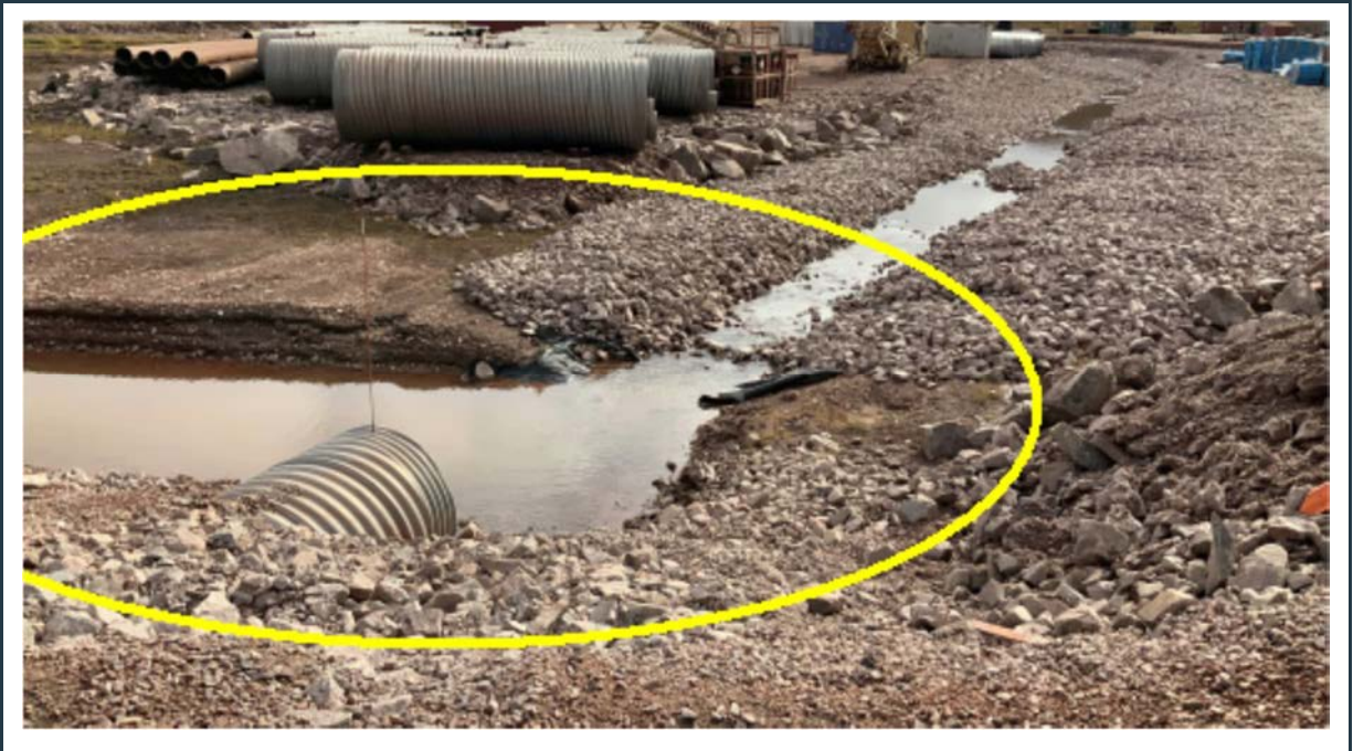
Figure 78: View of the partly completed W3/W14 surface water collection ditch with crushed rock riprap slope protection. The area around the culvert's inlet and the side-ditch from the left still require the placement of geotextile and riprap for erosion protection.
