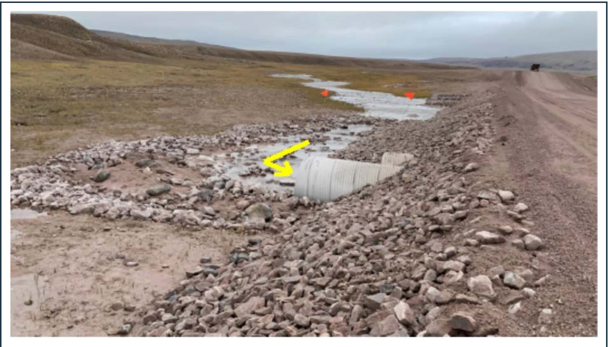
Figure 106: View of the inlet of the twin culverts at KM 36+000, in good condition.
