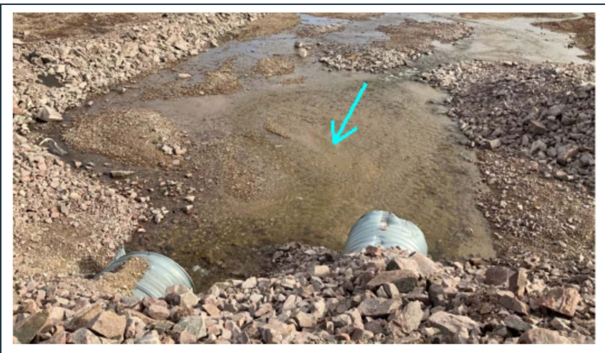
Figure 76: View of the P-SWD-7 surface water collection ditch and culverts (inlet).
