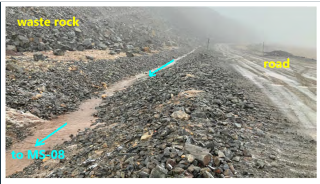
Figure 29: View of the well-maintained drainage ditch around the west side of the waste rock disposal facility, leading to the MS-08 pond.
