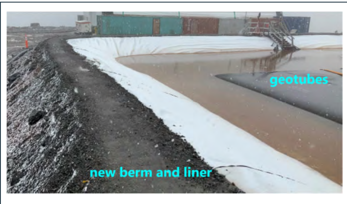
Figure 31: View of the completely refurbished perimeter berm and new liner at the geotube pond, located adjacent to the treatment plant.
