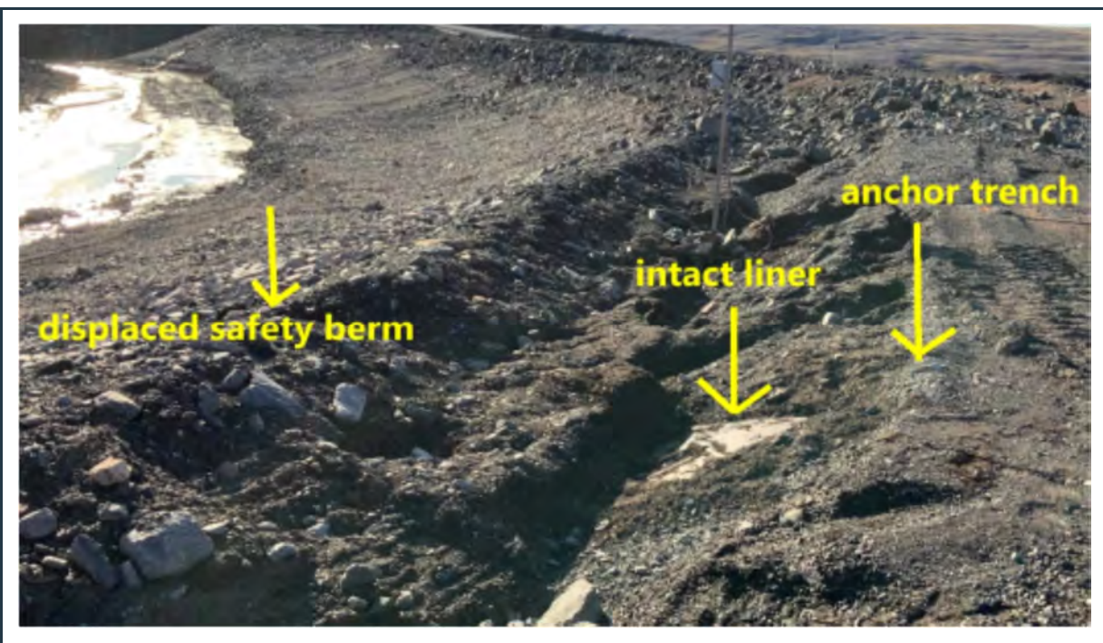
Figure 36: View of the displaced safety berm and the intact liner at the south pond (image was taken on August 26, 2024).
