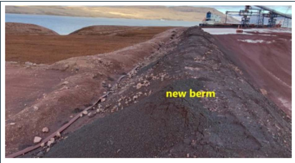
Figure 67: View of the 2024 condition of the “west” surface water collection ditch adjacent to the ore storage area. Note the new, widened berm along the ditch, partly constructed within the ditch.
