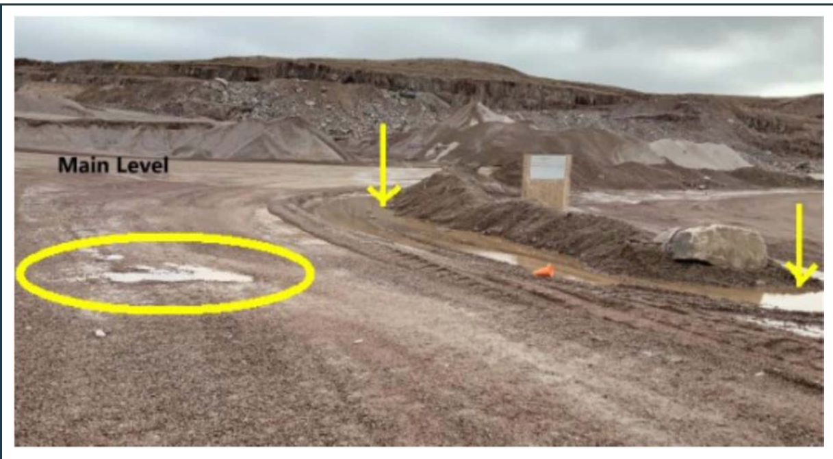
Figure 68: View of ponding and flowing water at may areas of the lower (main) level of the Q01 rock quarry. The drainage problem should be rectified prior to restarting the operation in the quarry.
