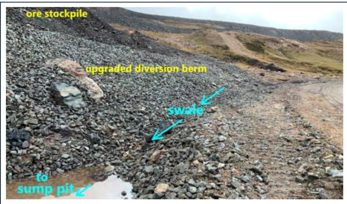
Figure 51: View of the new, recently upgraded diversion berm and drainage ditch/swale south of the ore stockpile area.
