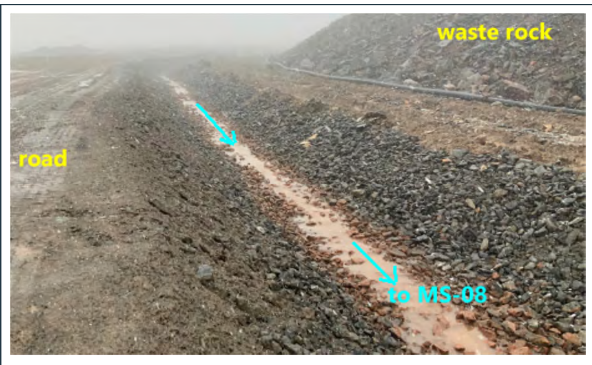
Figure 30: View of the well-maintained drainage ditch around the east side of the waste rock facility, leading to the MS-08 pond.
