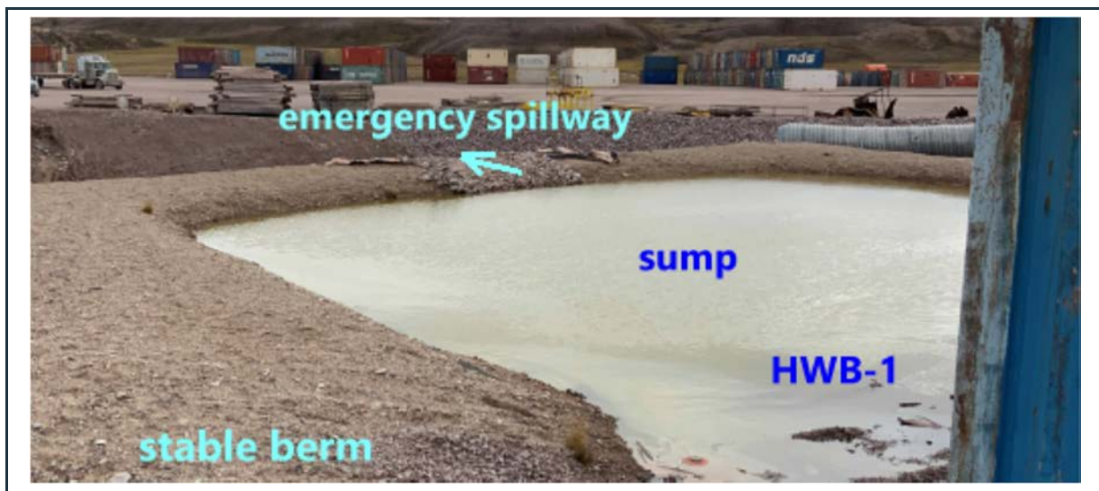
Figure 54: View of the sump and emergency spillway at the back of the HWB-1 cell with stable berm.
