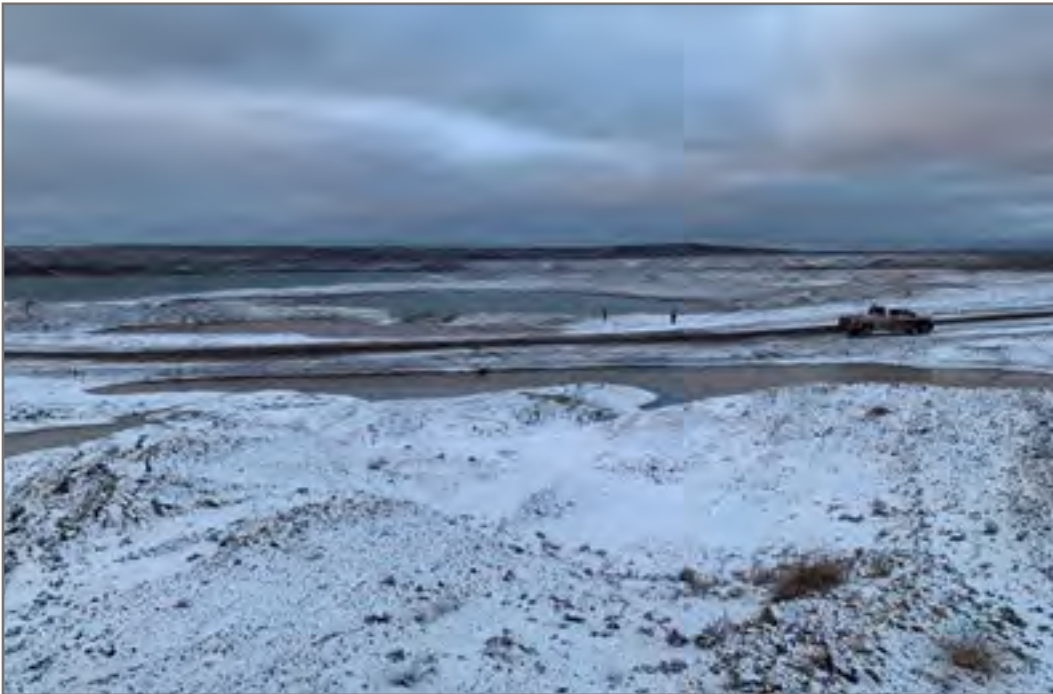
Photo 2 (Point 10-Priority B): Thaw settlement, excessive water pooling and dysfunctional drainage system
