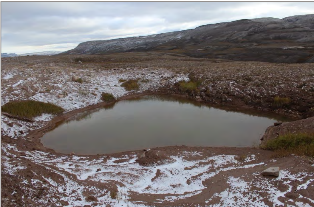
Photo 50 (Point 79.1-Priority A): Large sinkhole filled by water near the right (heading north) toe of the roadway embankment
