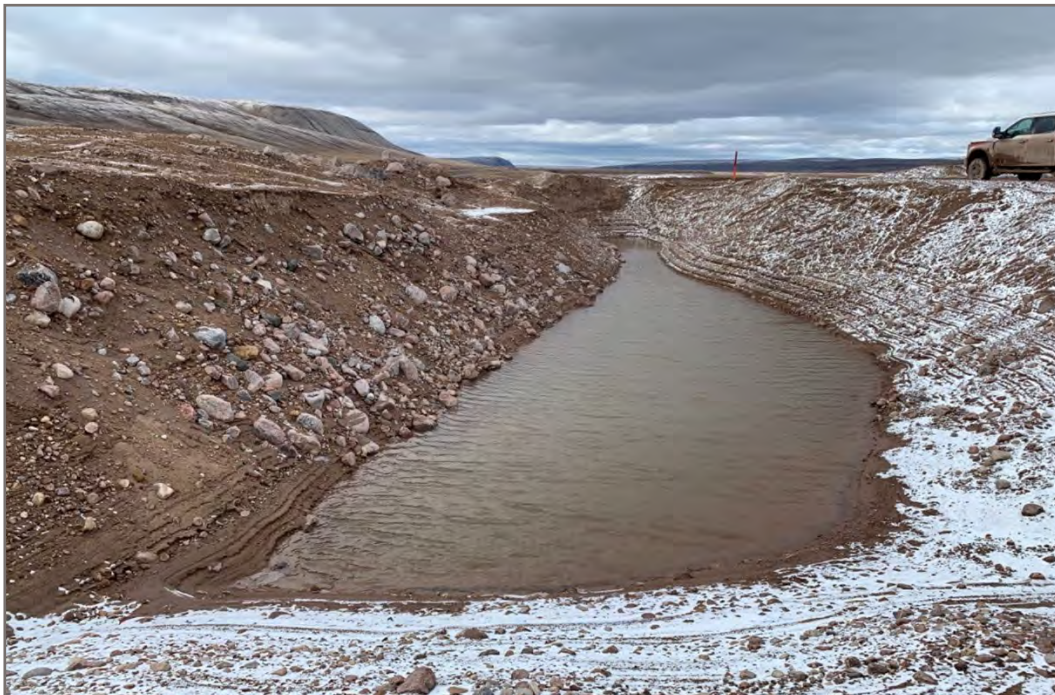
Photo 44 (Point 71-Priority A++++): Steep slope, deep water, and evidence of continuing permafrost degradation
