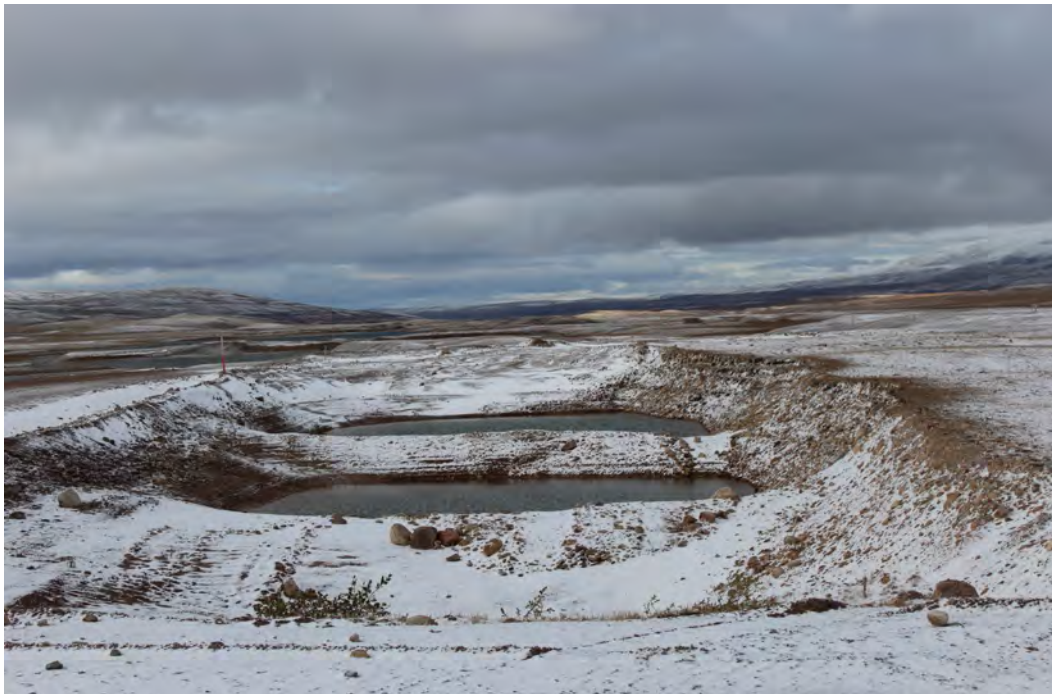
Photo 36 (Point 62A-Priority A+): Water pooling and evidence of permafrost degradation
