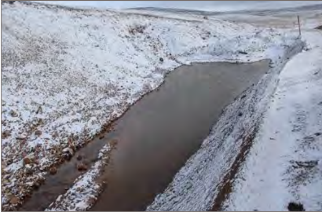
Photo 35 (Point 62-Priority B): Steep embankment and pooled water at the embankment
