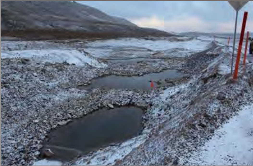
Photo 7 (Point 14 (QIA-02)-Priority A++++): Steep embankment, deep water pooling, and evidence of instability
