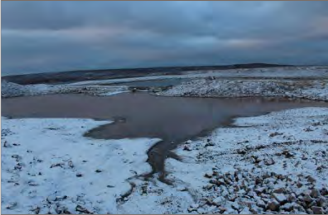
Photo 3: (Point 11-Priority B) Excessive water pooling and dysfunctional drainage
