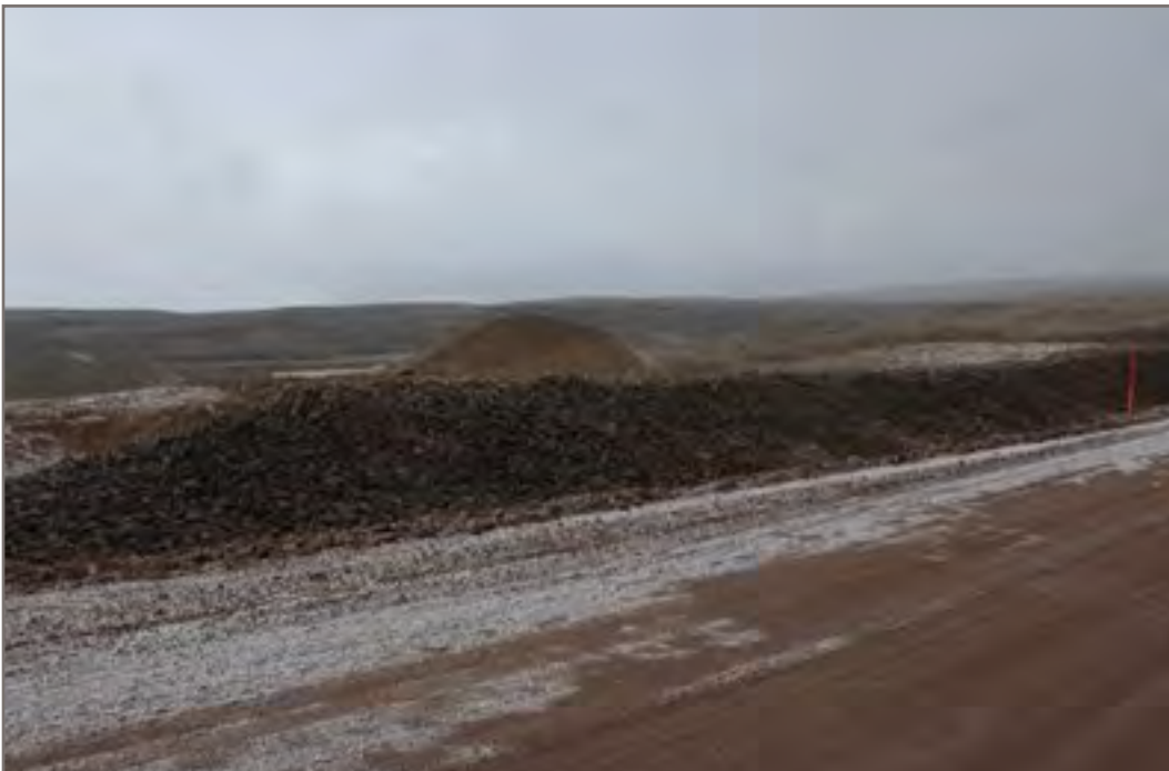
Photo 20 (Point 40-Priority C): Completed filling activities (filled with 150 mm minus material)
