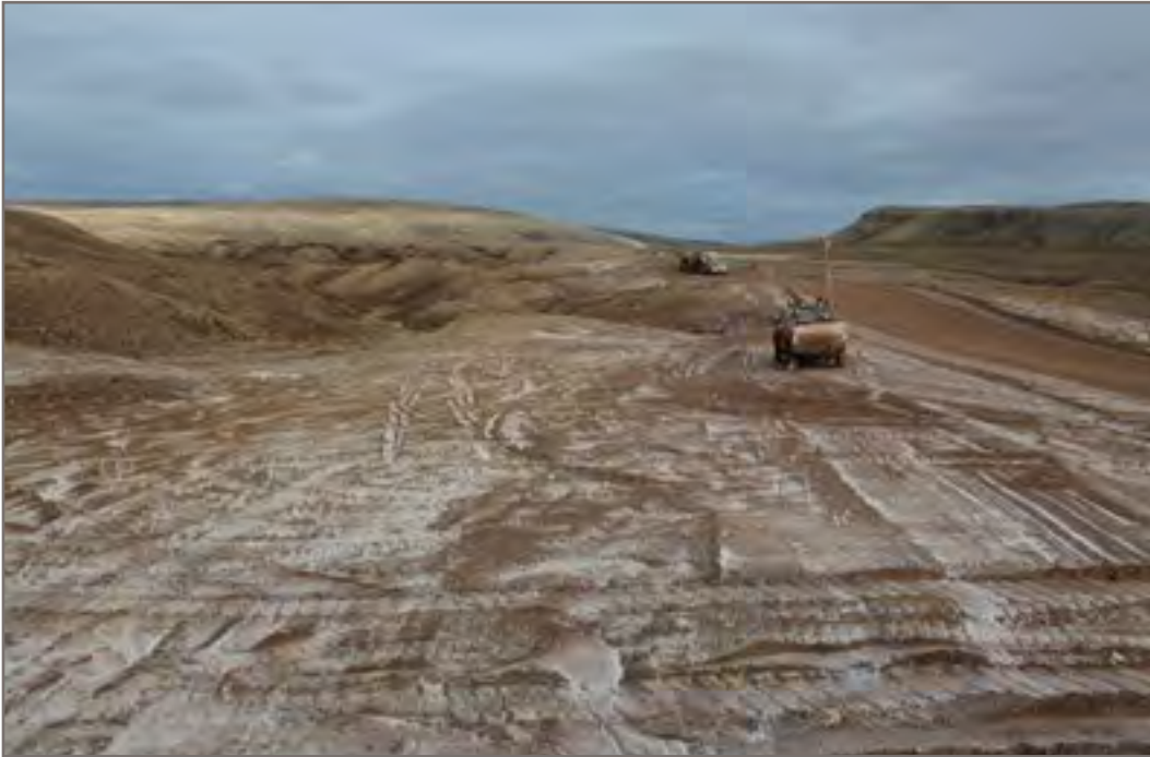
Photo 11 (Point 29-Priority B): Partially filled, need more filling, grading, and dressing
