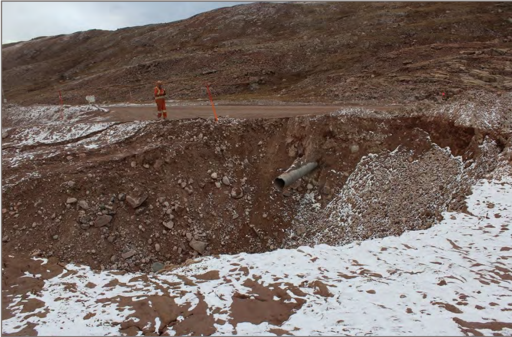
Photo 55 (Point 85-Priority A++++): Slope failure along the right (heading north) edge of the Tote Road
