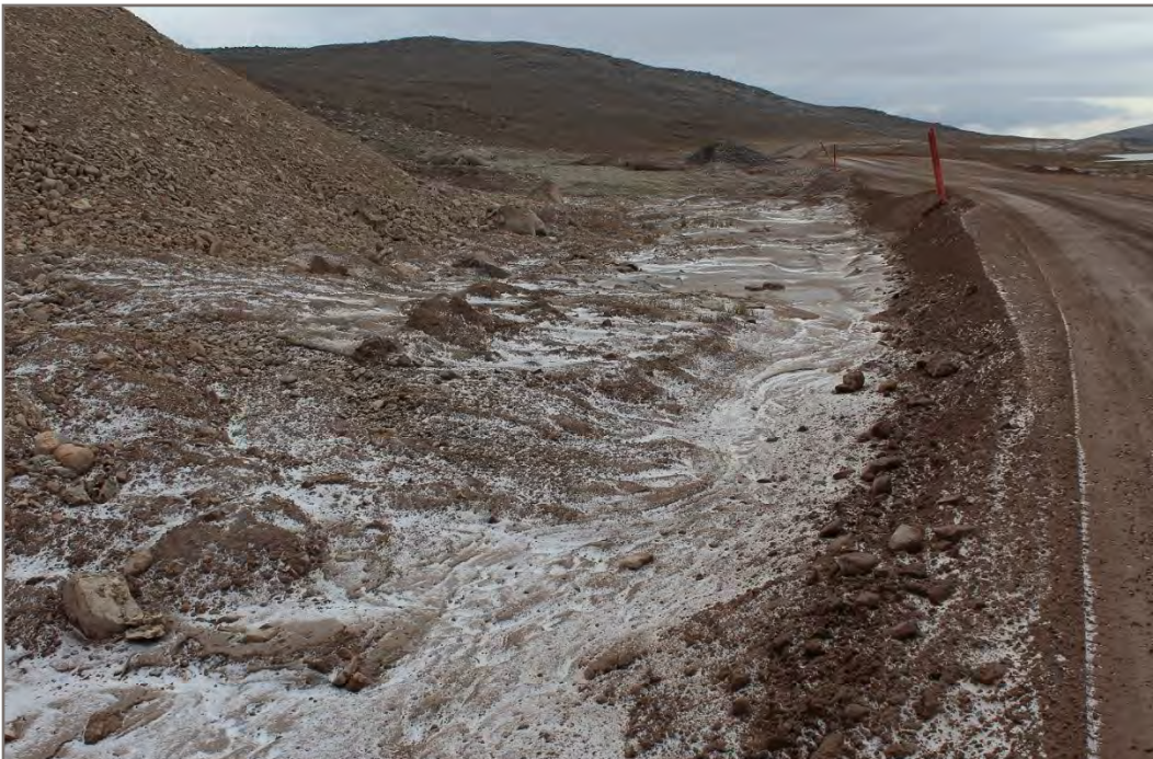
Photo 16 (Point 35A-Priority B): Dysfunctional drainage system and poor erosion protection measures
