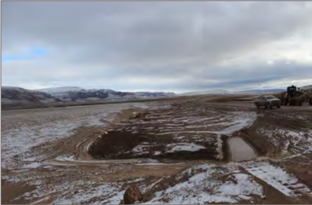
Photo 43 (Point 70-Priority B): Wet bottom, settlement, and evidence of continuing permafrost degradation
