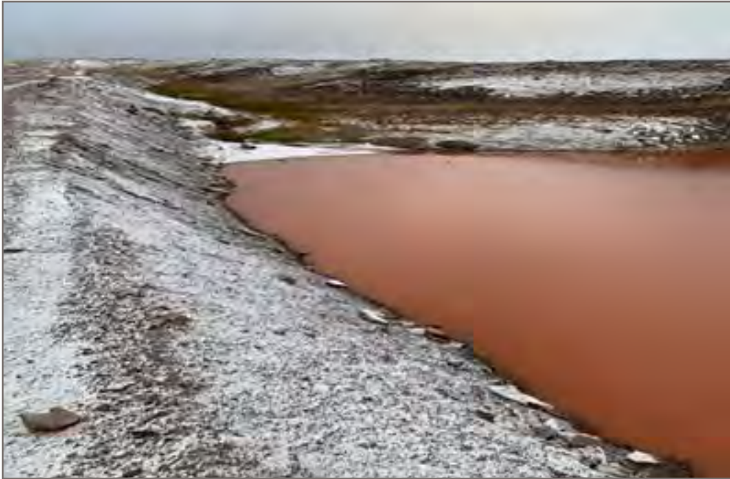
Photo 5 (Point-QIA-01): Water pooling at several locations along the north edge of the road
