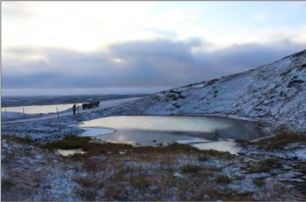
Photo 9 (Point 16-Priority B): Dysfunctional drainage system and water pooling at the toe of the embankment
