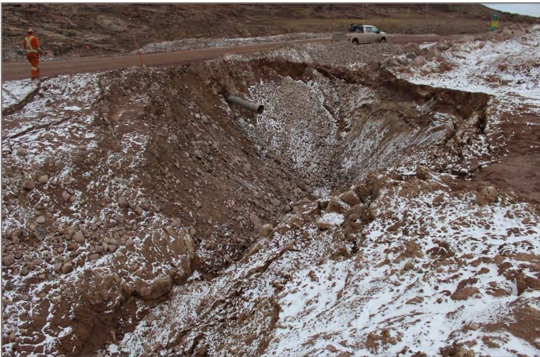
Photo 56 (Point 85-Priority A++++): Slope failure along the right (heading north) edge of the Tote Road
