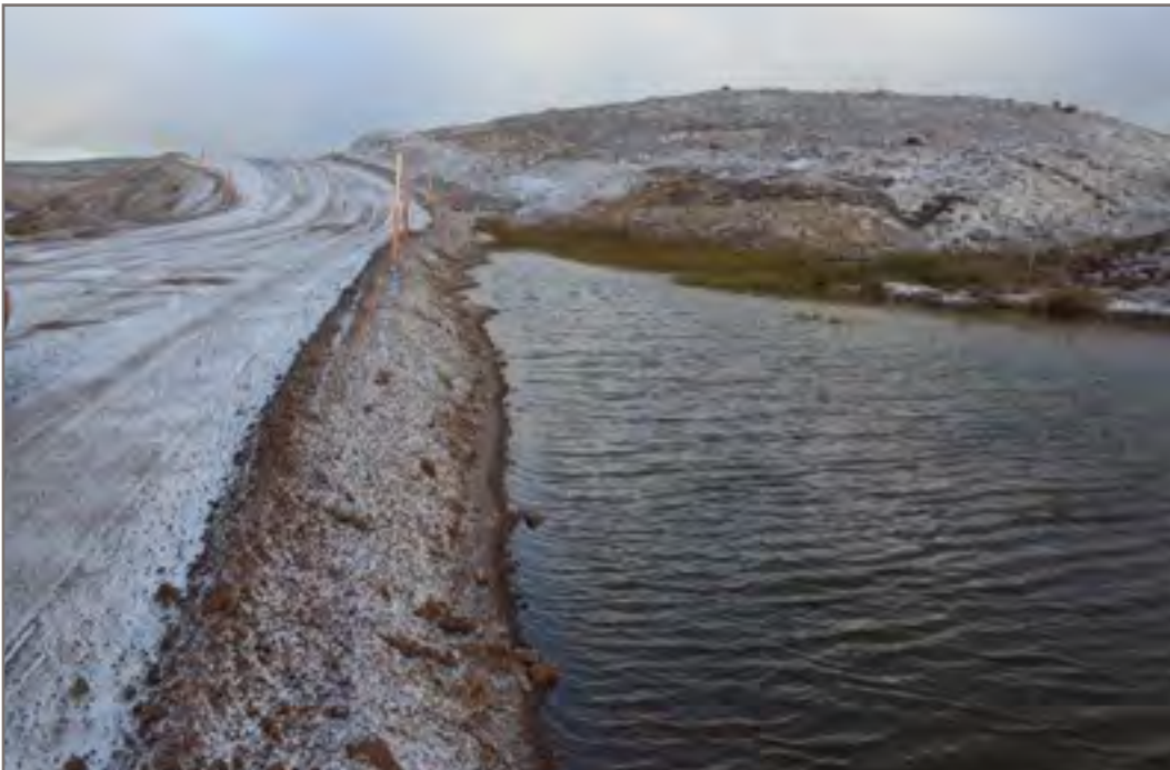
Photo 10 (Point 16.1-Priority C): Dysfunctional drainage system and water pooling at the toe of the embankment
