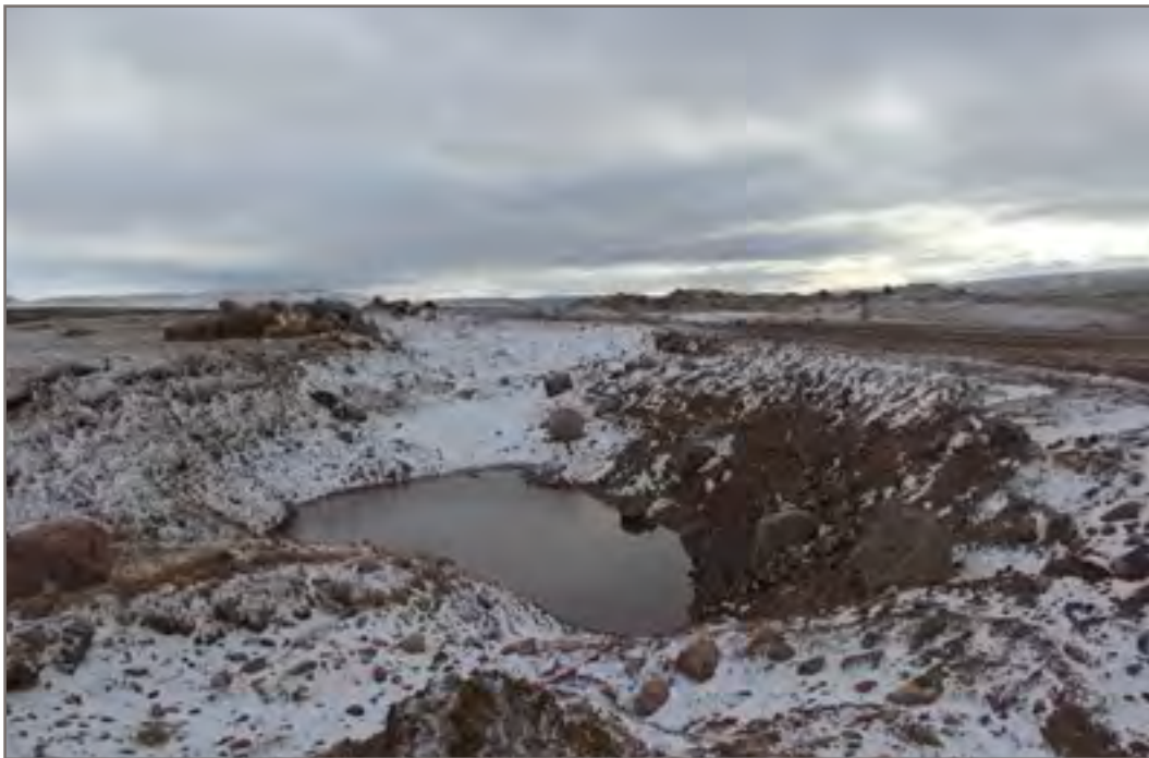
Photo 40 (Point 67-Priority B): Deep water and evidence of continuing permafrost degradation (north end of the pit)
