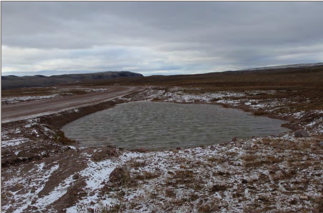
Photo 48 (Point 75-Priority A): Right (heading north) pit filled and graded. Deep pooled water in the left (heading north) pit
