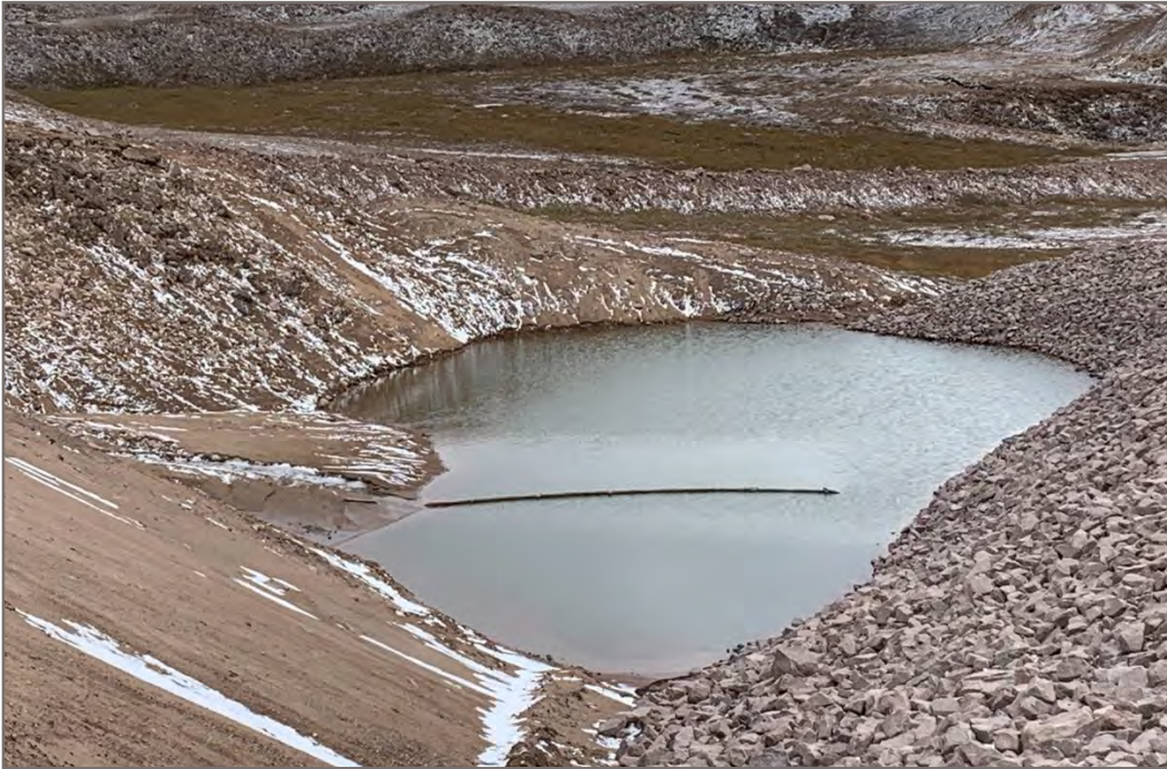
Photo 51 (Point 82A-Priority A): Old borrow area with deep standing water near the left edge of the embankment
