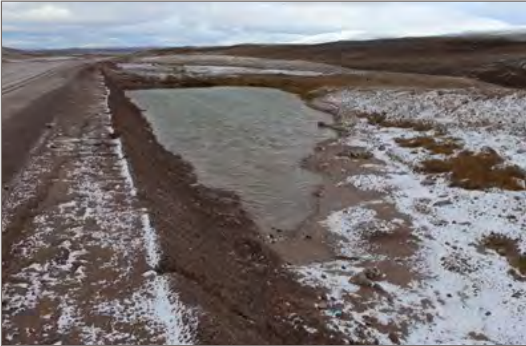
Photo 39 (Point 66-Priority A+): Pooled water and evidence of continuing permafrost degradation (left pit heading north)
