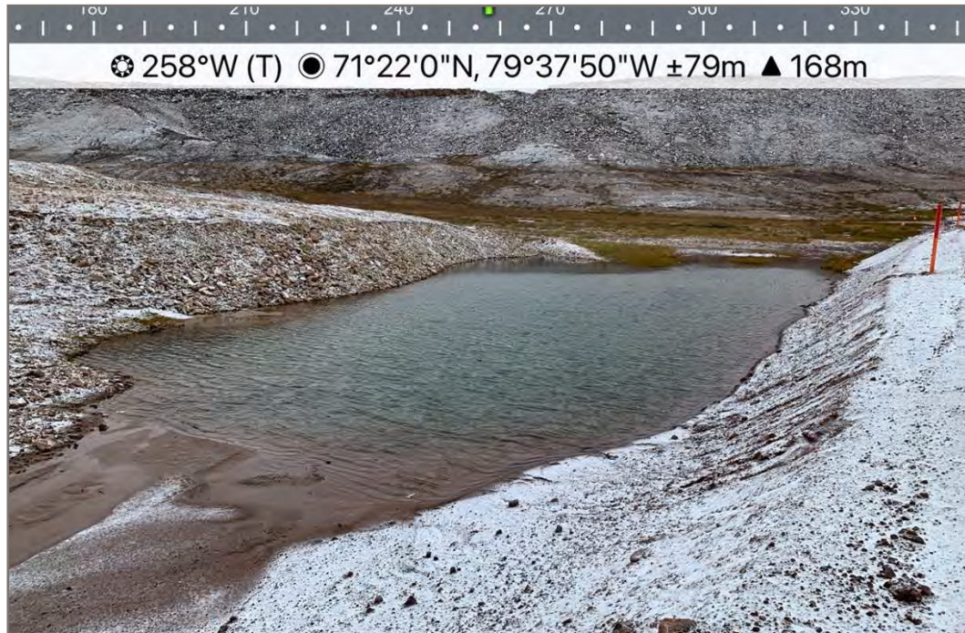
Photo 13 (Point 33- Priority A+++): Water pooling, ground settlement, dysfunctional drainage system
