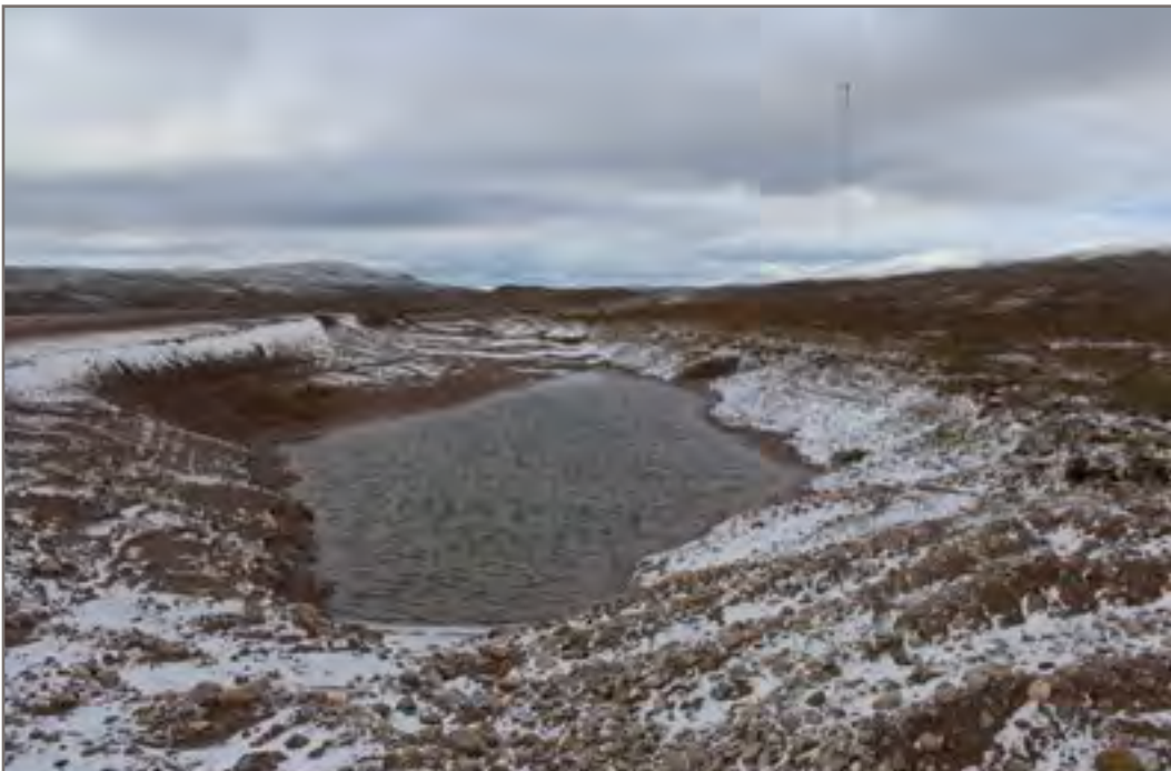
Photo 38 (Point 65-Priority A+): Pooled water and evidence of permafrost degradation (left pit heading north)
