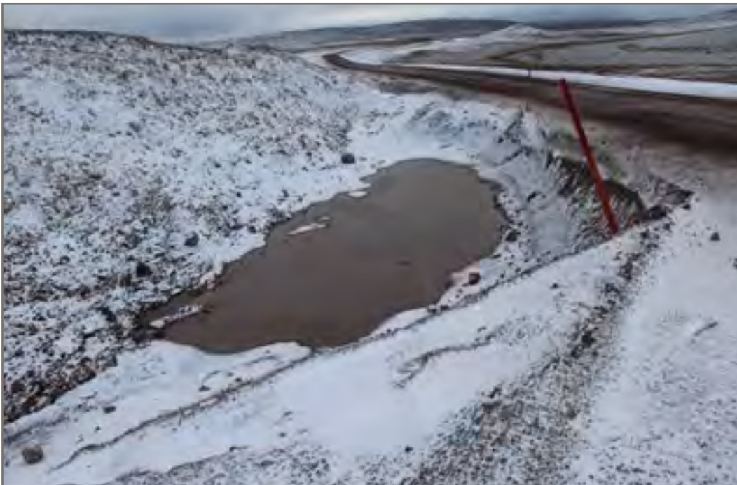
Photo 34 (Point 61B (QIA-09)-Priority A++++): Steep and high embankment, presence of water at the toe of the slope
