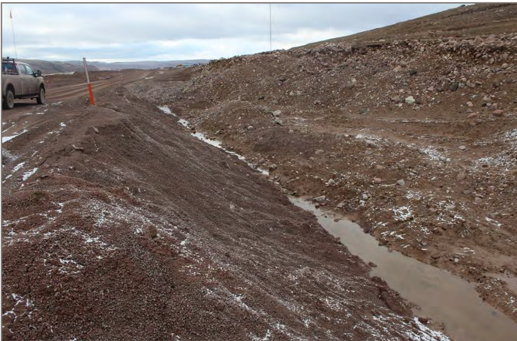
Photo 54 (Point 83A (QIA-11)-Priority B): Left borrow area was partially filled in 2021, needs more grading
