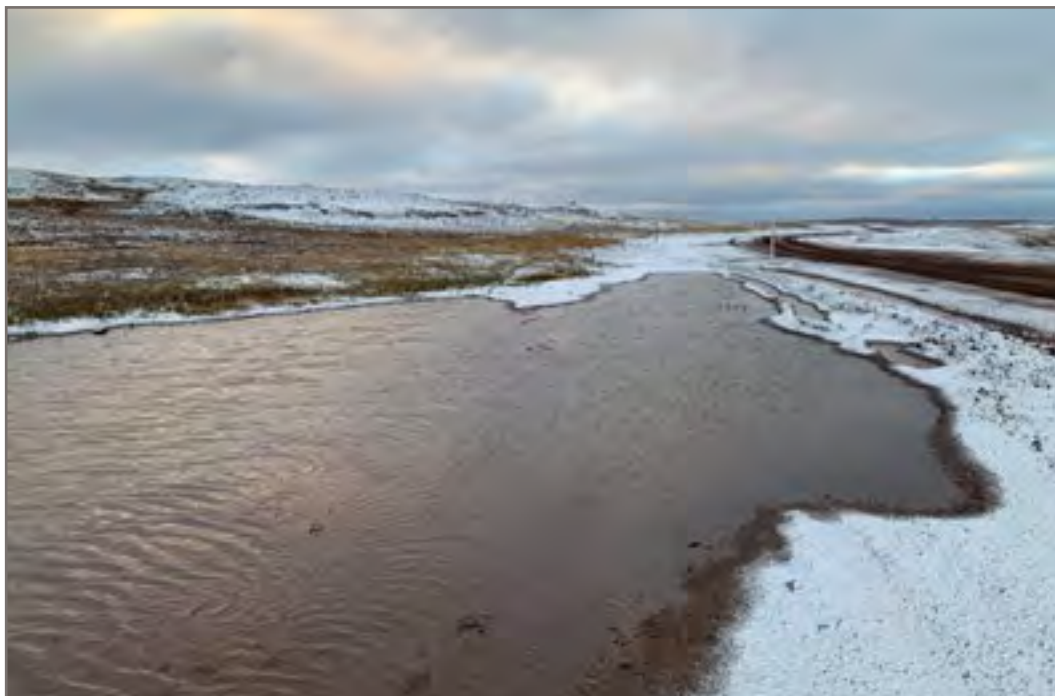
Photo 4 (Point 12A-Priority B): Water pooling adjacent to the north edge of the road
