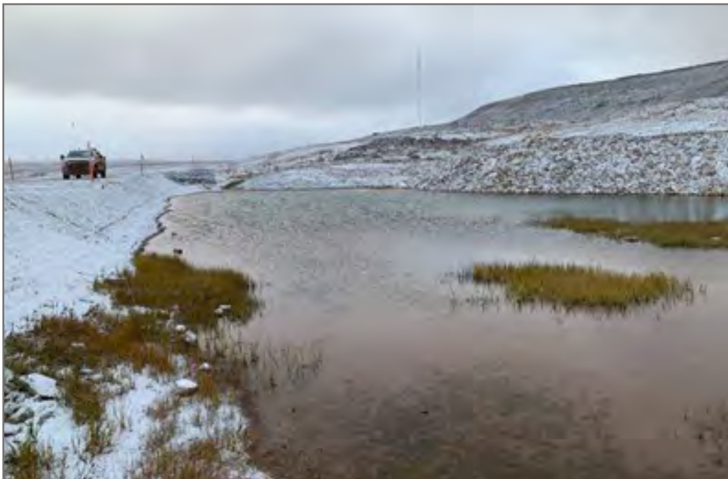
Photo 8 (Point 15-Priority B): Dysfunctional drainage system and water pooling at the toe of the embankment
