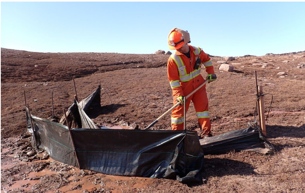
Photo 85. Maintaining ESC Silt Fence – April
